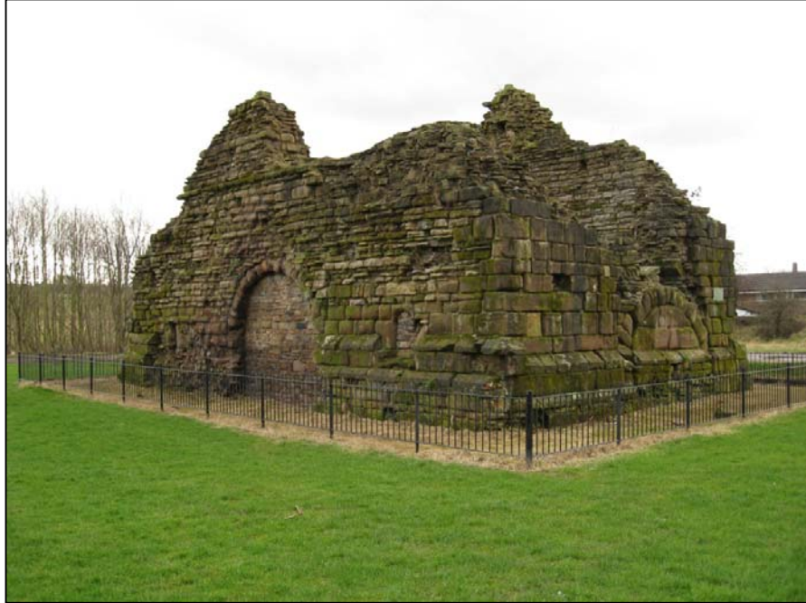
Fig 24: The northern and eastern elevations of Radcliffe Tower in 2008.
