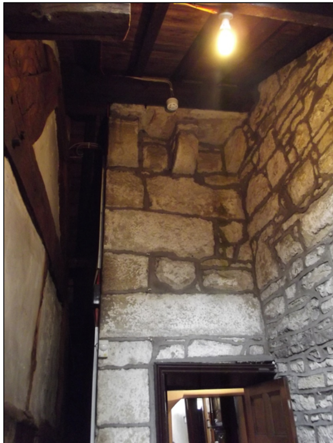
Fig 54: The stair tower at Turton Tower with corbelling to support the roof line. A possible parallel for the stair tower at Radcliffe.
