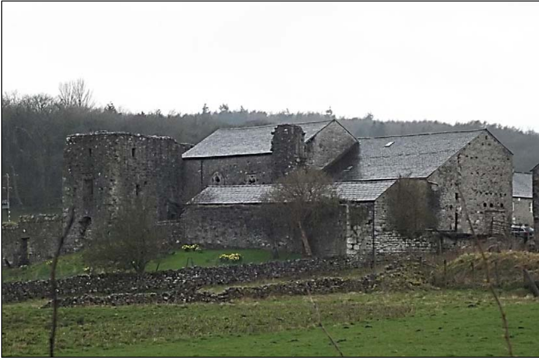
Fig 55: The late medieval tower (left) at Beetham Hall, Cumbria.
