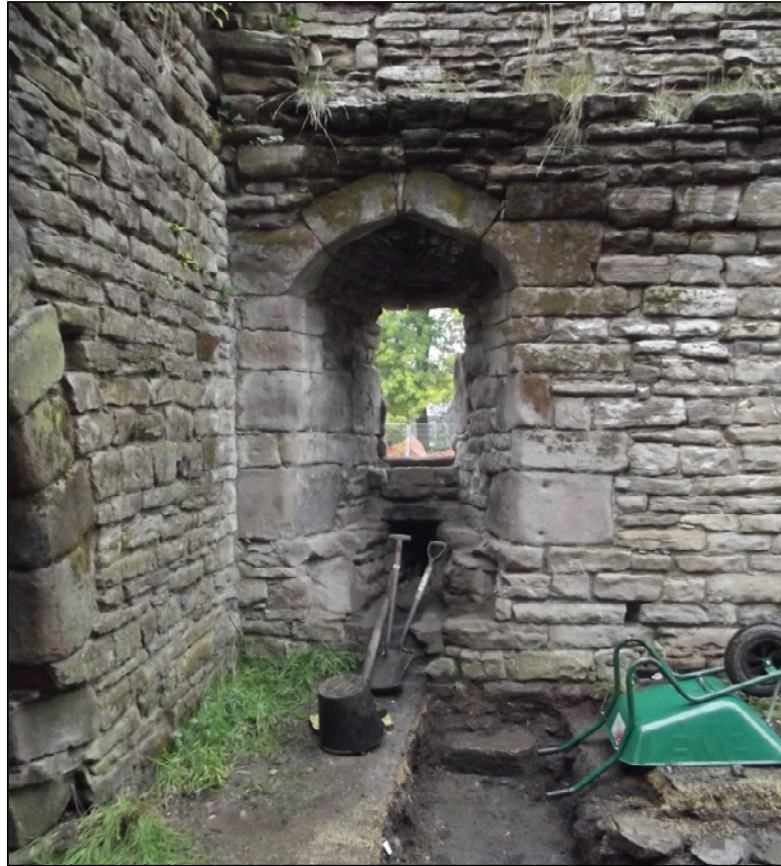
Fig 38: Excavations in October 2014 showing the north-eastern interior corner of Radcliffe Tower, with the medieval drain. Note the remains of the barrel vaulting surviving above the window.
