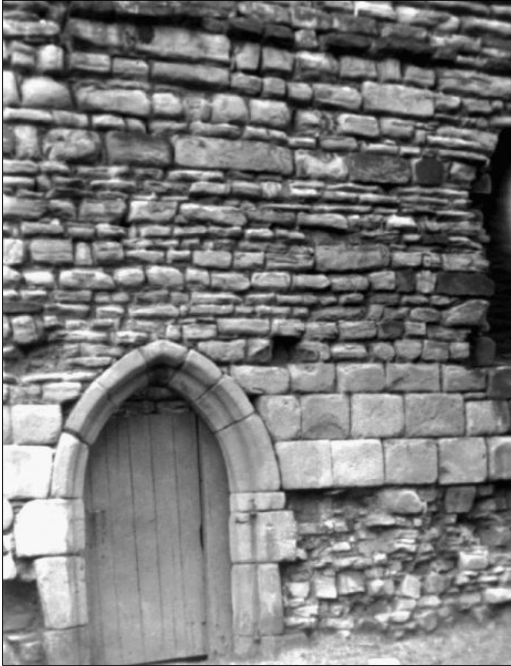
Fig 21: Radcliffe Tower western doorway and the edge of the tower doorway (right) in 1902. Copyright Bury Archives.
