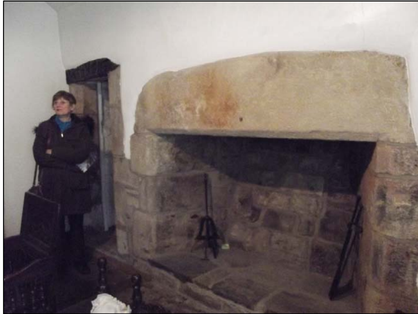
Fig 53: A first-floor fireplace at Turton Tower – a possible parallel for the first floor fireplace at Radcliffe Tower.
