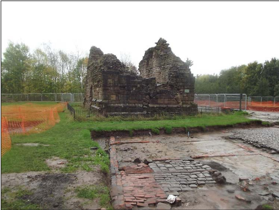
Fig 37: Excavations in October 2014 showing the foundations of farm buildings and behind the northern gable of the Radcliffe Tower.
