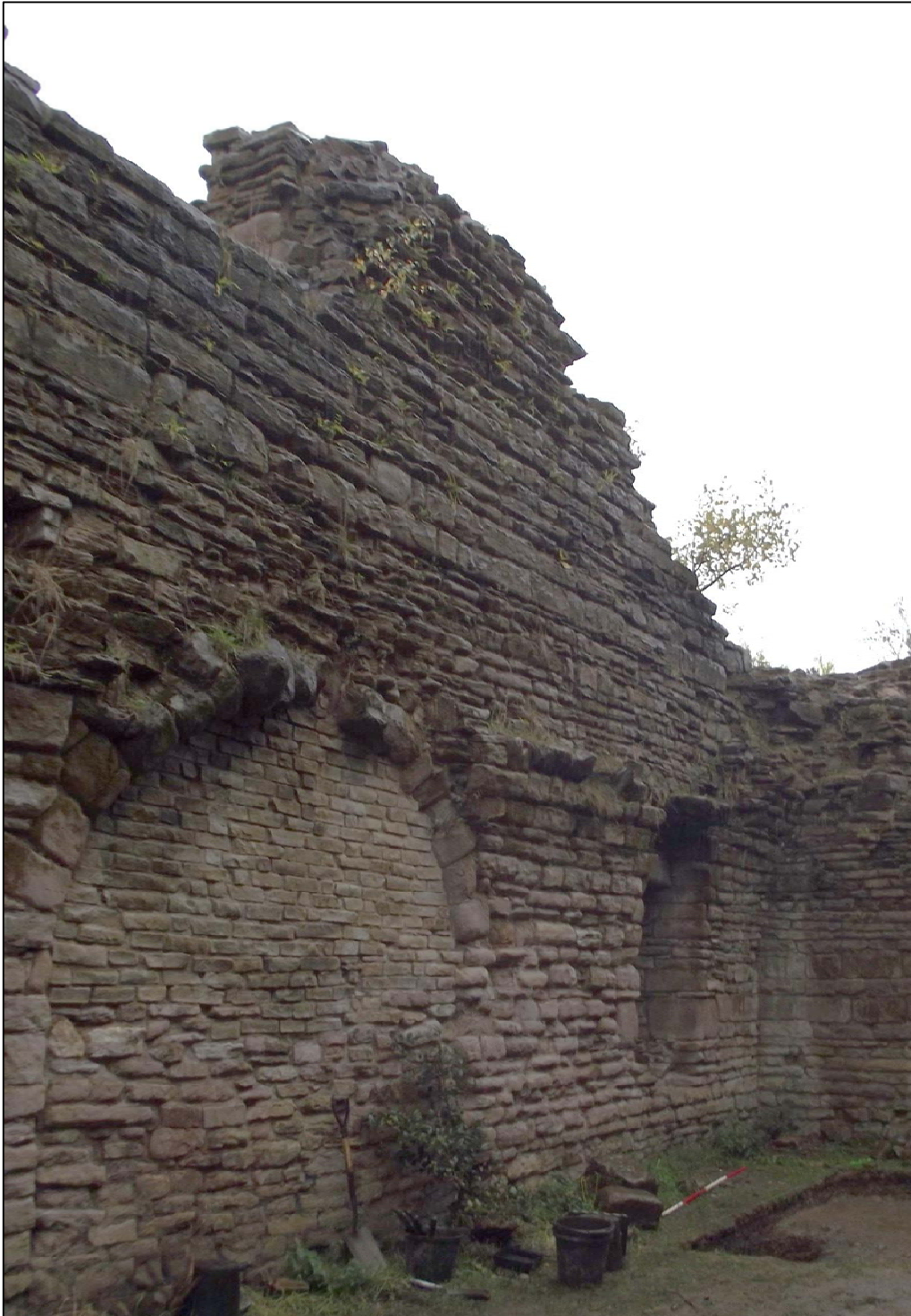
Fig 42: Interior of Radcliffe Tower, looking at the eastern elevation. The apex of the archway breaks the line of the barrel vaulting suggesting that it is a later insert. Note the remains of the window above the arch.
