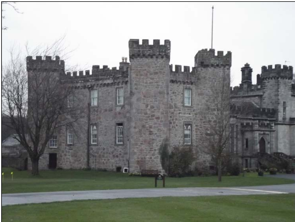
Fig 60: Ashton Hall which its late medieval peel tower which has stair turrets to each corner..
