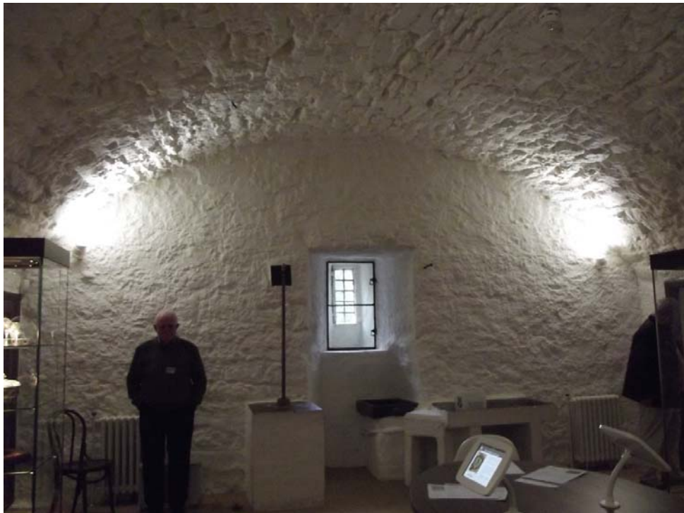
Fig 50: The ground floor barrel vaulting at Sizergh castle with a splayed central window of the style seen at Radcliffe Tower.
