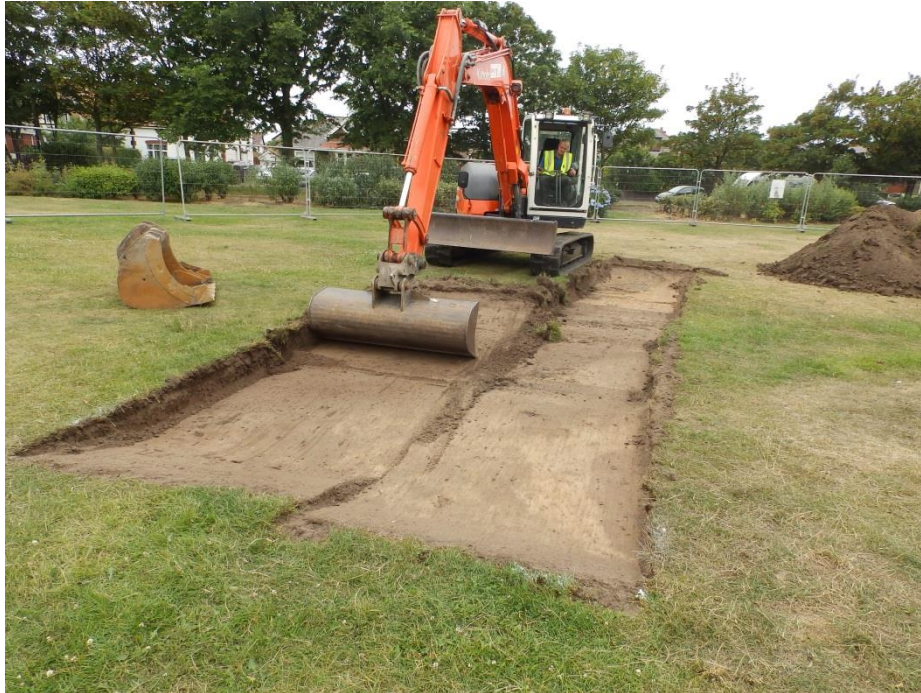
Figure 17: showing the machine excavation of T1.
