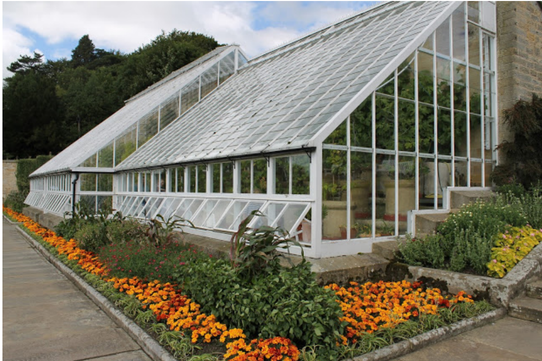
Fig 40. Glasshouses at Cragside. These were built in 1870 and typically had low walls supporting the iron and glass framework (image: http://www.jibberjabberuk.co.uk/2015/10/the-formal-garden-cragside.html )
