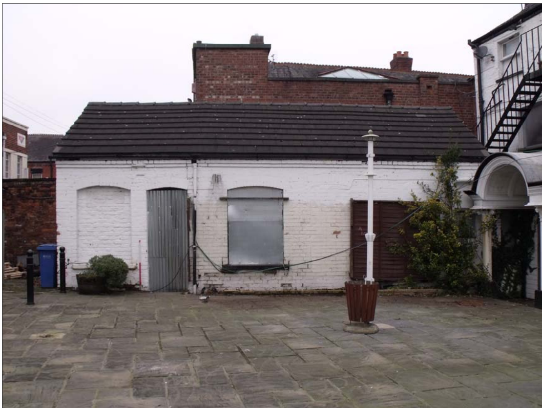
Fig 5: The south-western wing of the George & Dragon Hotel showing the blocked openings. The blocked window on the left will be knocked through.
