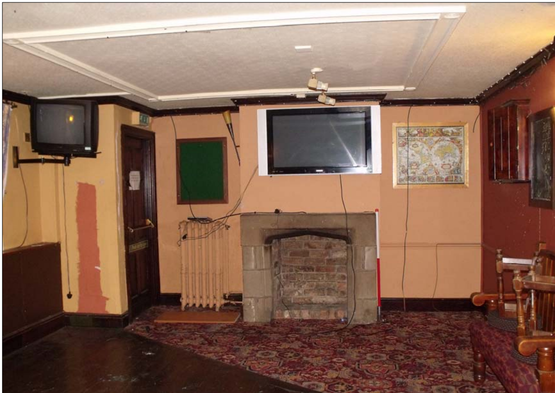
Fig 9: George & Dragon Hotel GF1, showing the eastern fireplace bay with to the left (north) the north-eastern entrance. This is intended to be the site of a new staircase which will involve the removal of the fireplace.
