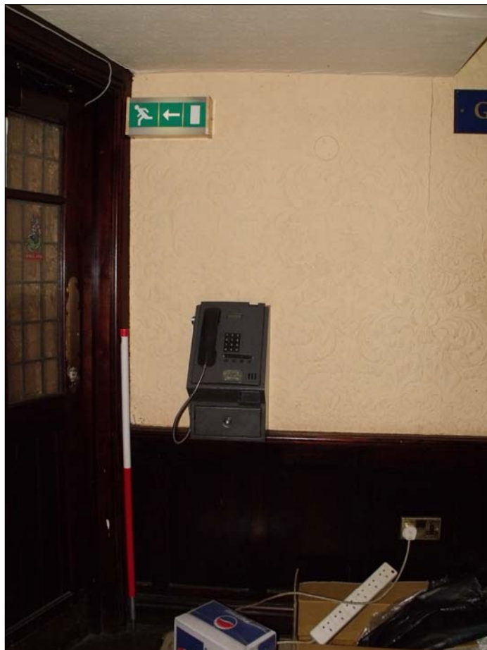
Fig 7: George & Dragon Hotel GF6 looking at the southern wall into the toilet area (GF9) which will be knocked through.
