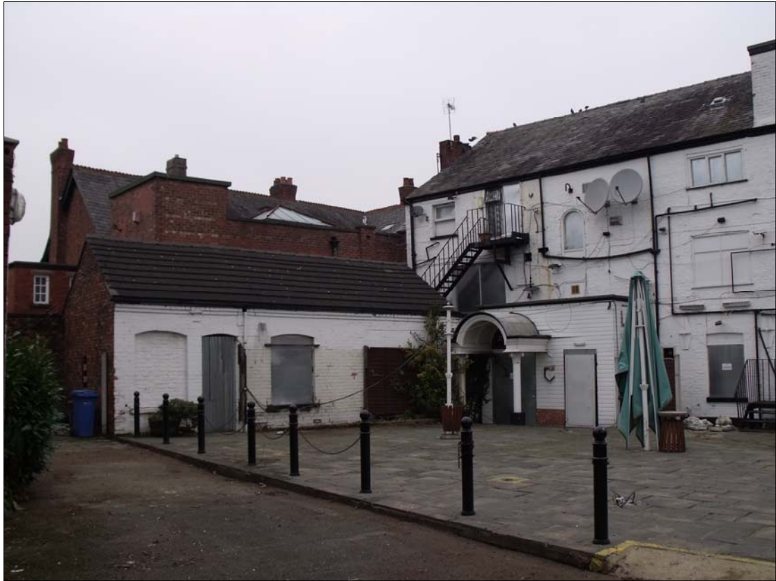
Fig 4: The single-storey south-western wing of the George & Dragon Hotel.
