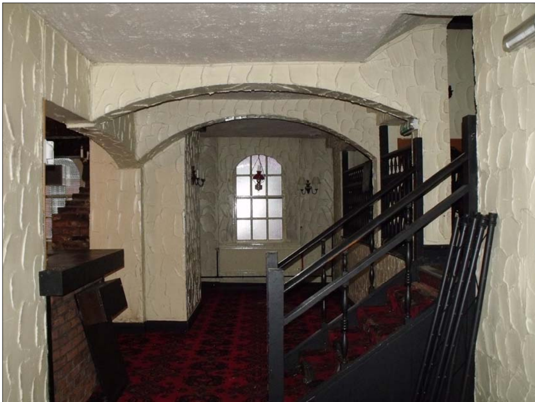
Fig 13: George & Dragon Hotel room FF7 looking north the window where the new staircase will be inserted.
