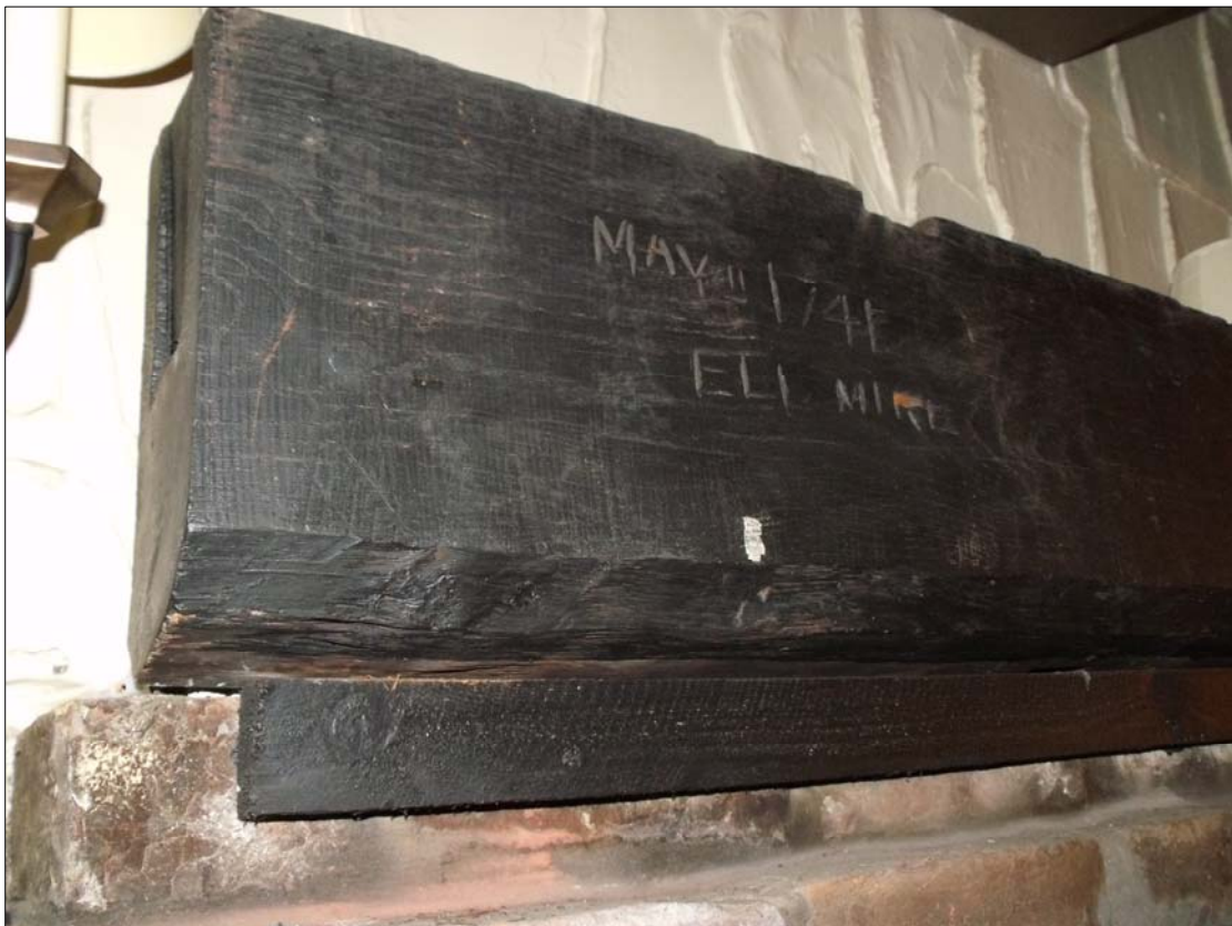
Fig 15: George & Dragon Hotel room FF6 looking at the inscription on the re-used purlin, dated '1741', above the fireplace.
