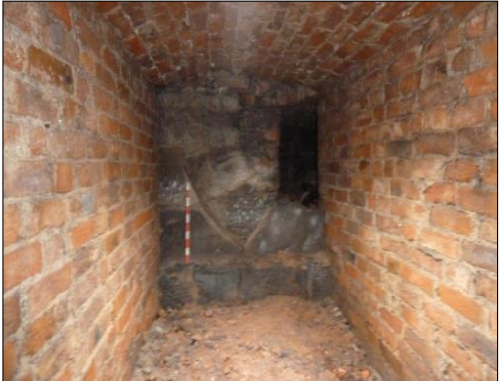
Fig 16: View of Room C10 looking south at another inverted stone arch.
