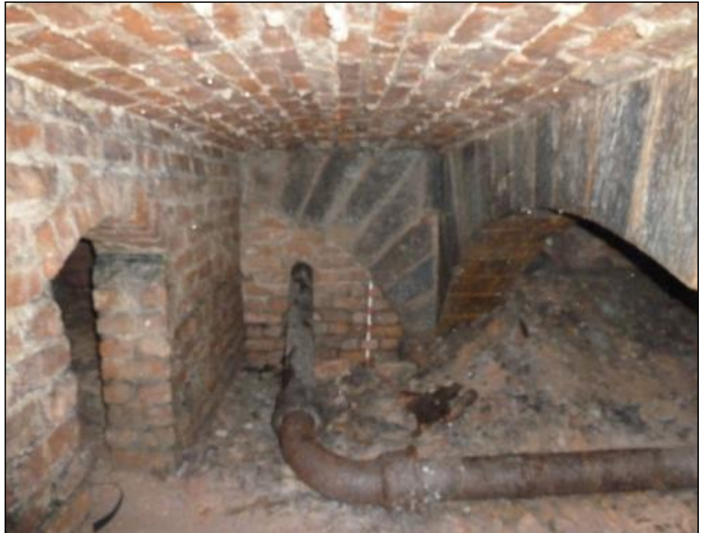
Fig 14: View of Room C7 looking north at the stone arches with brick blocking into which a heating pipe runs.
