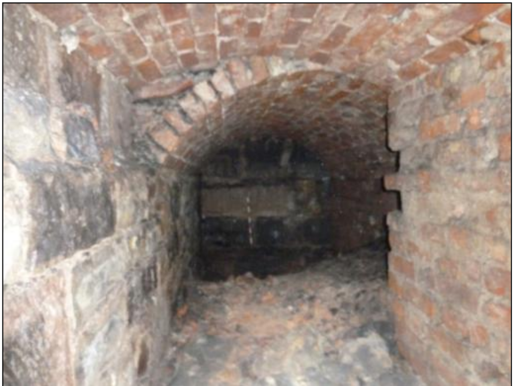
Fig 19: View of Room C12 looking southwards at the stonework beneath the brick barrel vaulting.
