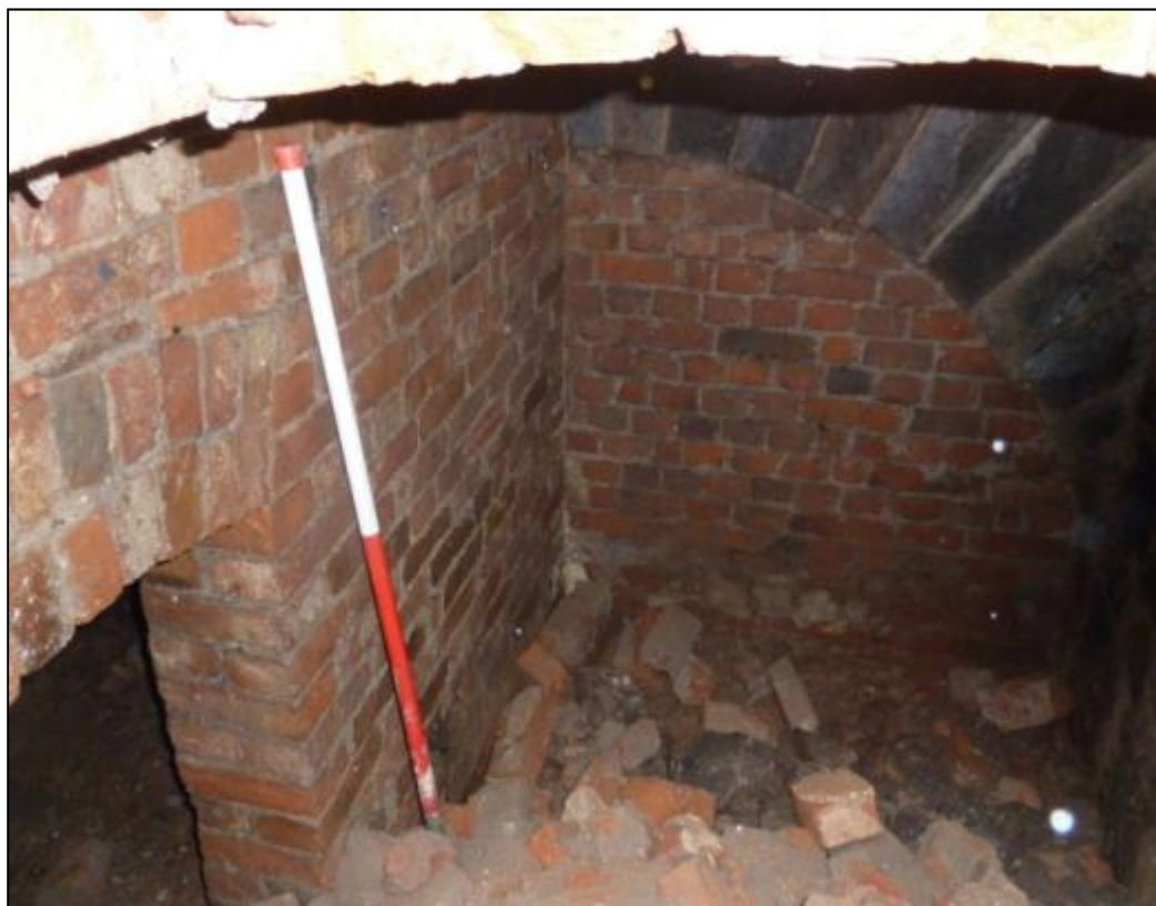
Fig 27: View of Room C25 looking north at a stone arch.
