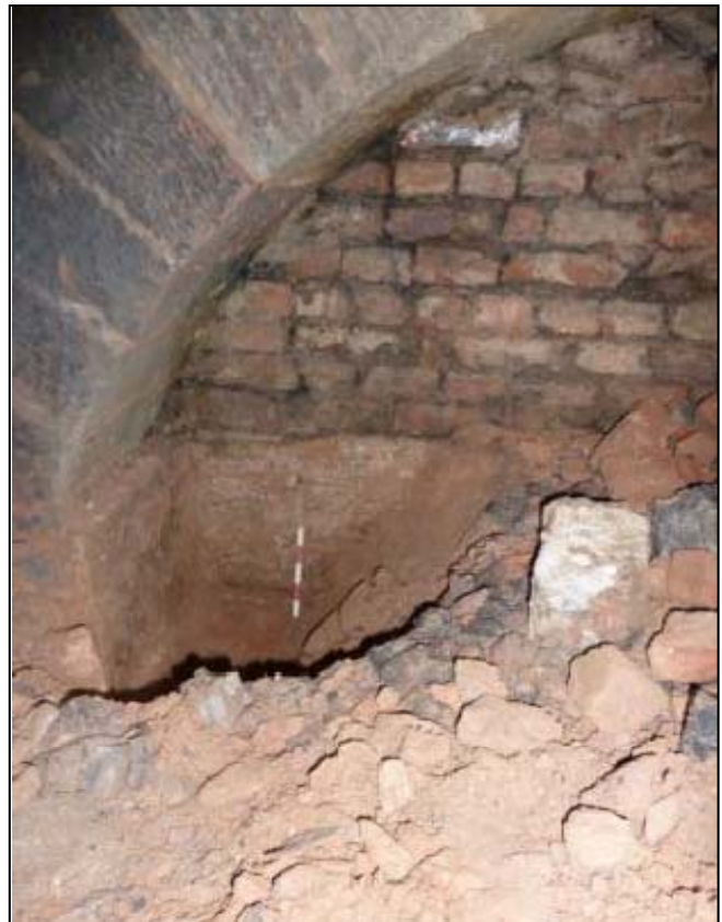
Fig 33: View of Room C16 showing Test Pit 3 against the western wall. Note the depth of the stone foundations.
