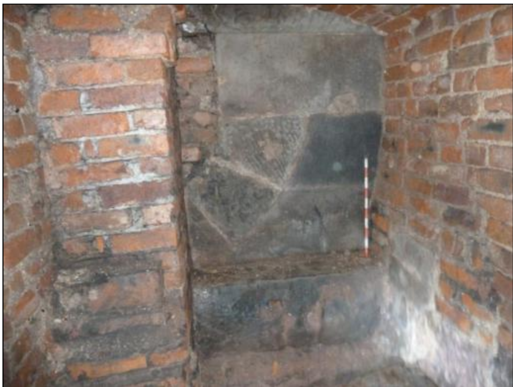
Fig 25: View of Room C22 looking east at an inverted stone arch.
