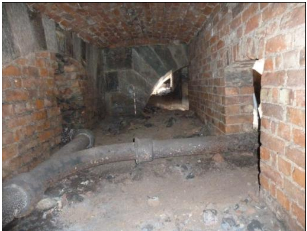
Fig 11: View of Room C4 looking north showing the two stone arches set at right-angles to each other.
