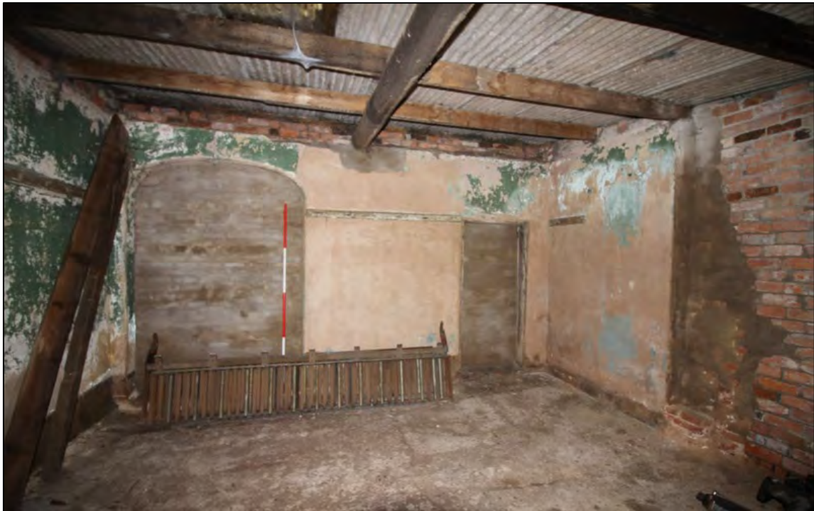
Plate 48: Room G3, looking north, with inserted corrugated sheet roof
