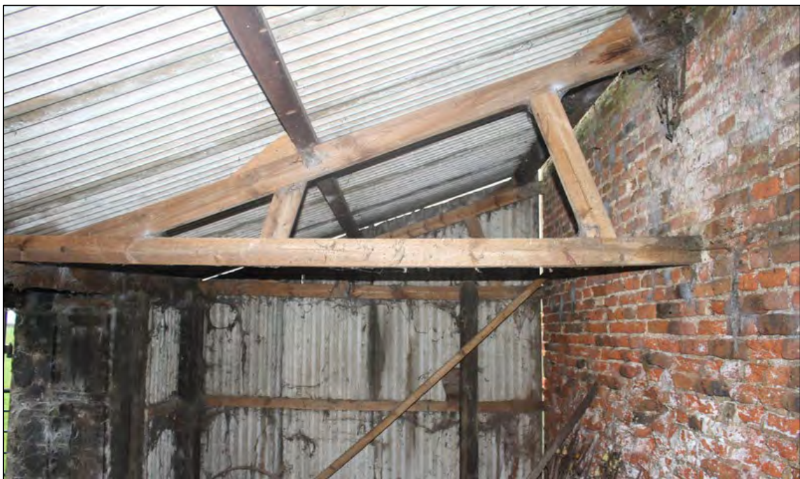
Plate 61: Detail of truss within cart shed G7
