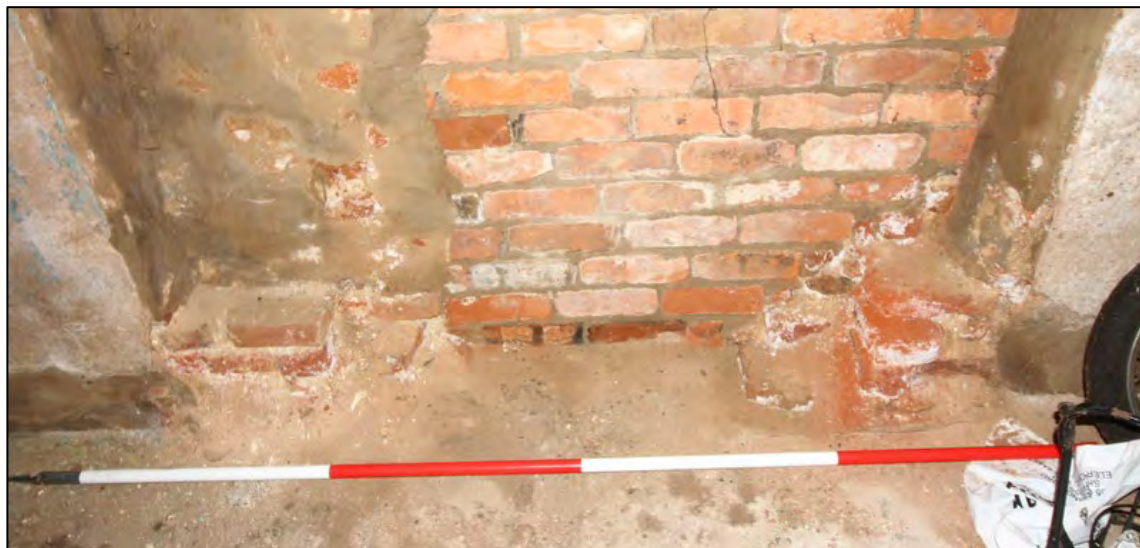
Plate 54: Remnants of fireplace cheeks in east wall, Room G3
