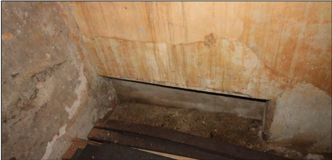
Plate 52: Rebate of former door head of stairs into cellar, Room G3
