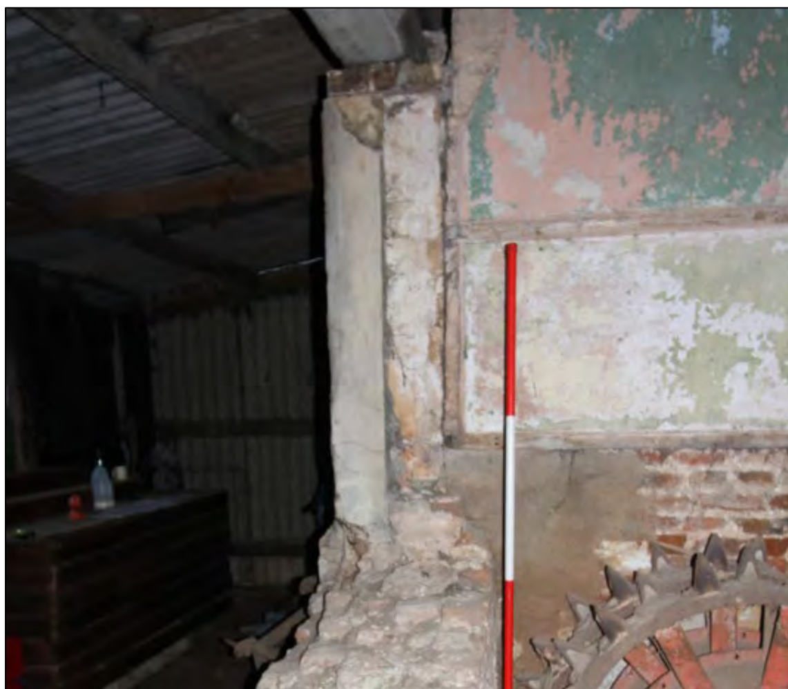
Plate 27: Rendered door jamb for the entrance into the post-monastic house
