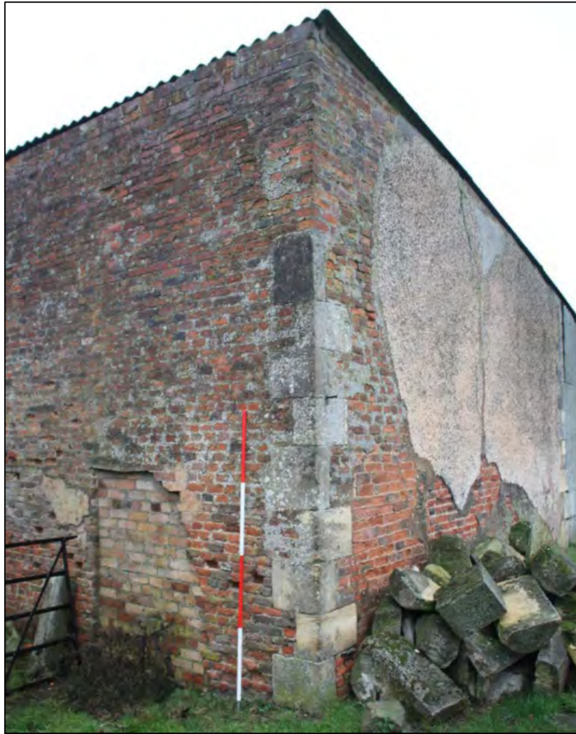
Plate 18: Eastern return of the west section of the north wall, with stepped quoins but no plinth
