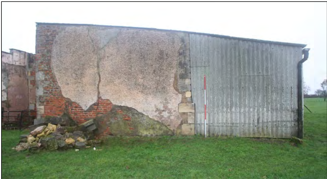
Plate 17: Western section of the north elevation, with large quoins forming the plinth at the western edge
