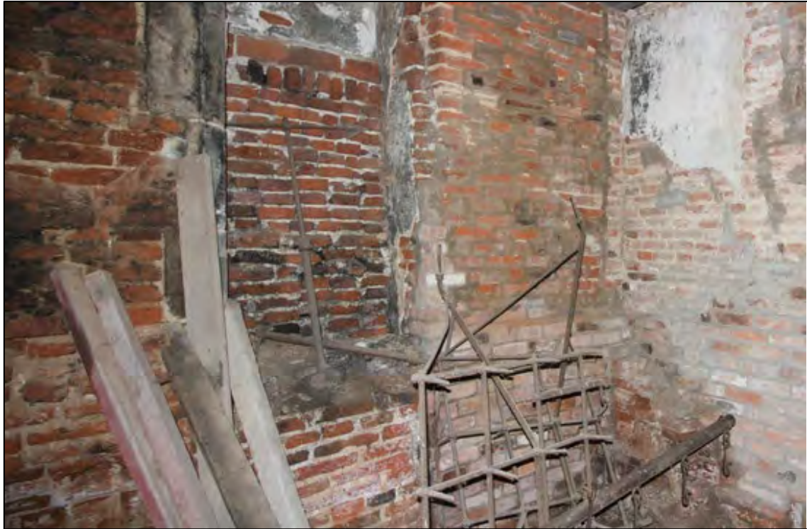
Plate 31: Junction of west and south walls, Room G1
