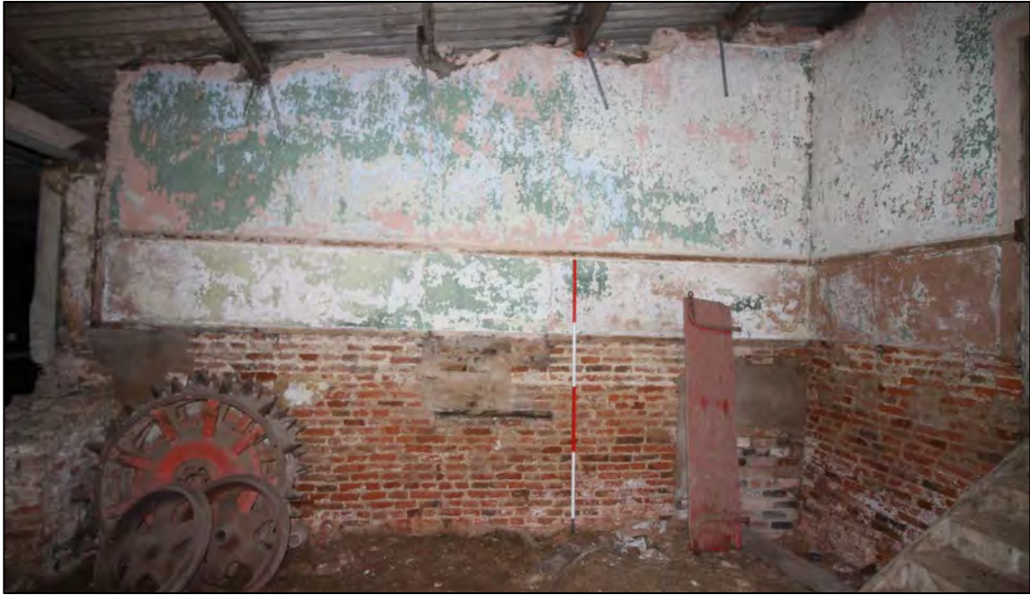
Plate 36: North elevation of Room G1
