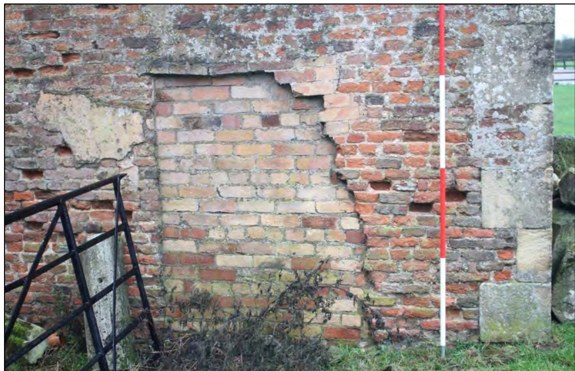
Plate 20: Blocked ragged doorway at the north end of the return of the west section of the north wall
