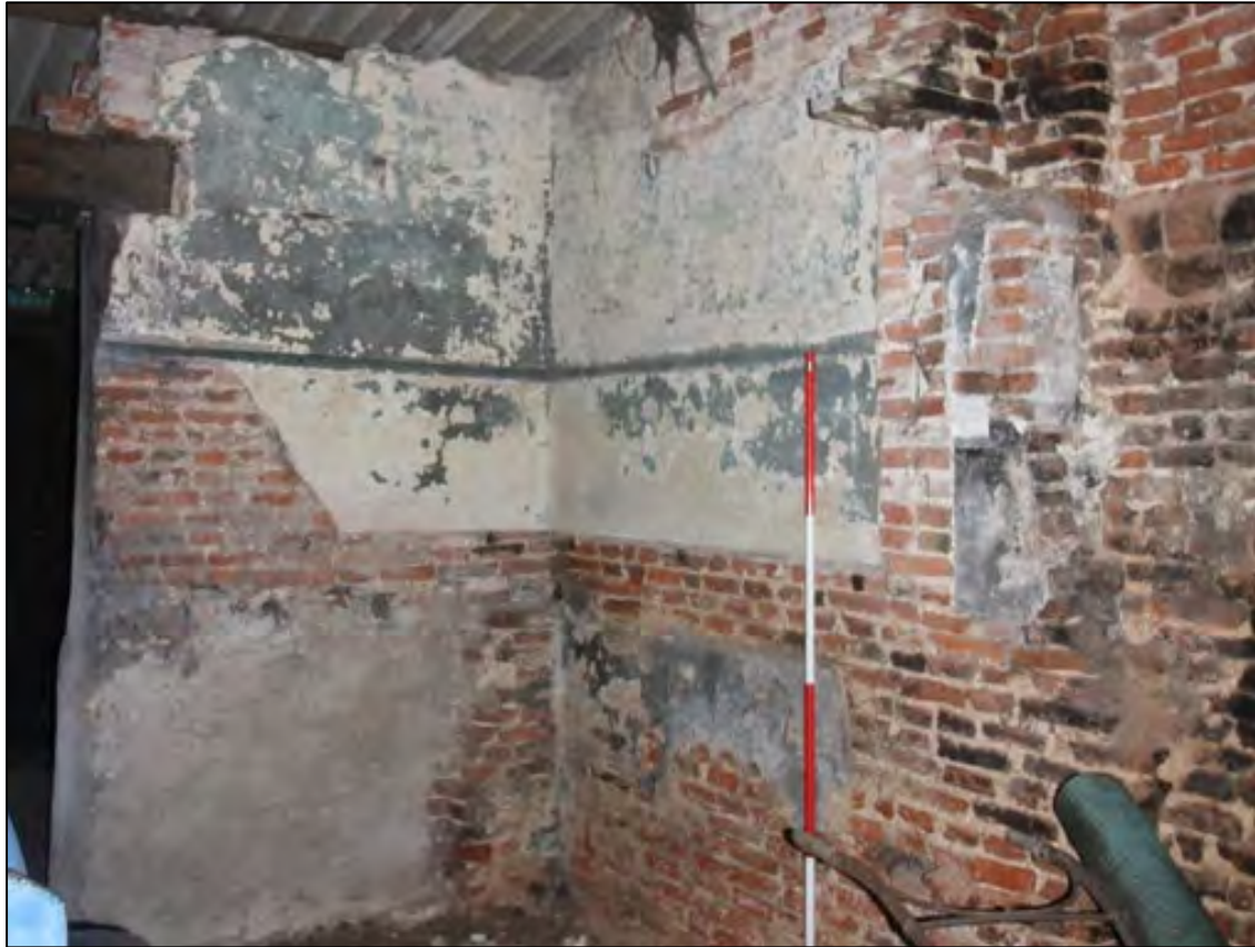
Plate 39: Junction of west and north elevations, Room G2
