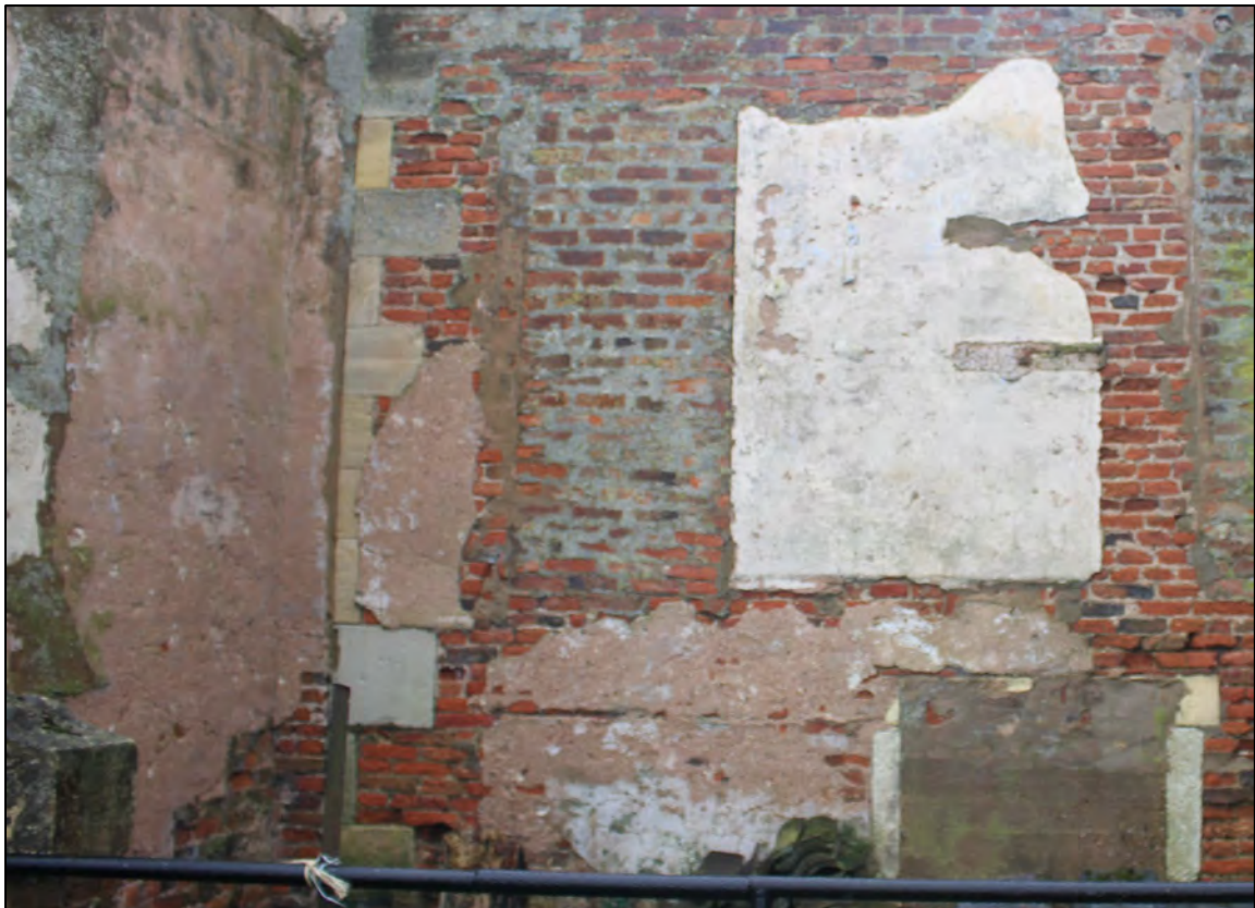
Plate 22: Blocked doorway between Rooms G3 and G5
