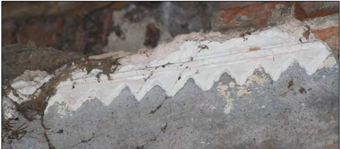
Plate 44: Detail of decorative plaster cornice, Room G2
