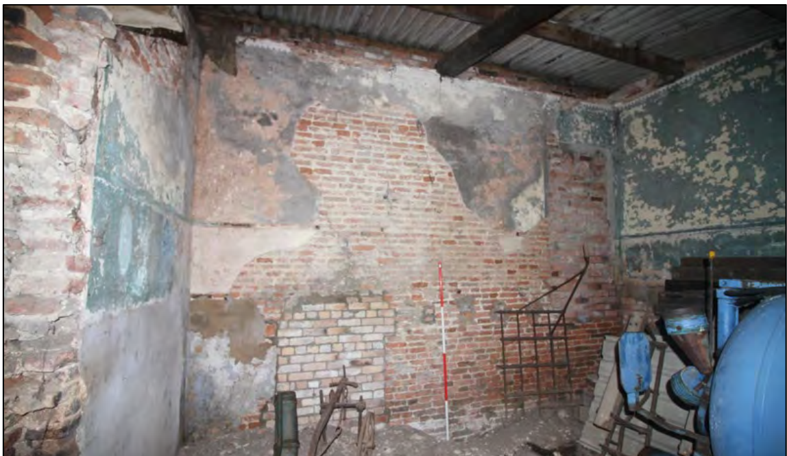
Plate 43: East elevation of Room G2
