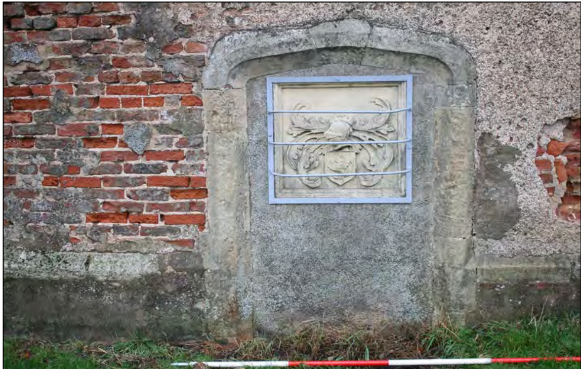
Plate 13: Detail of decorative doorway in the southern façade, latterly housing the Mowbray coat of arms
