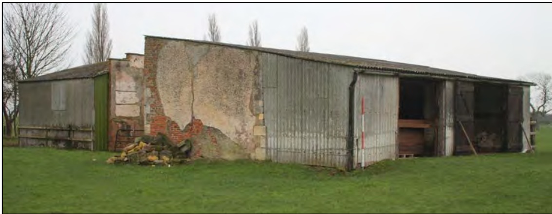
Plate 9: Extant building complex within the study area from the north-west
