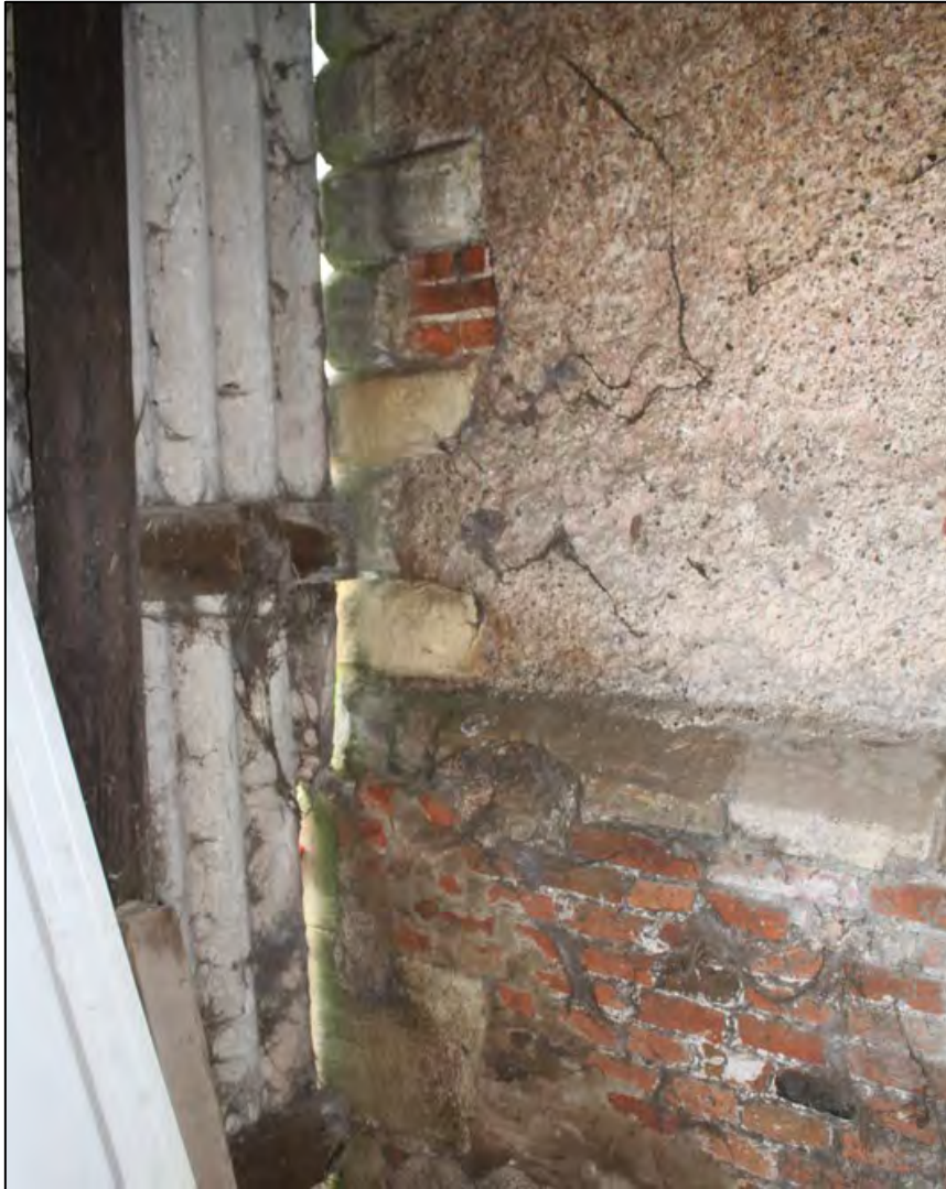
Plate 29: Rusticated quoins above plinth and flush quoins below
