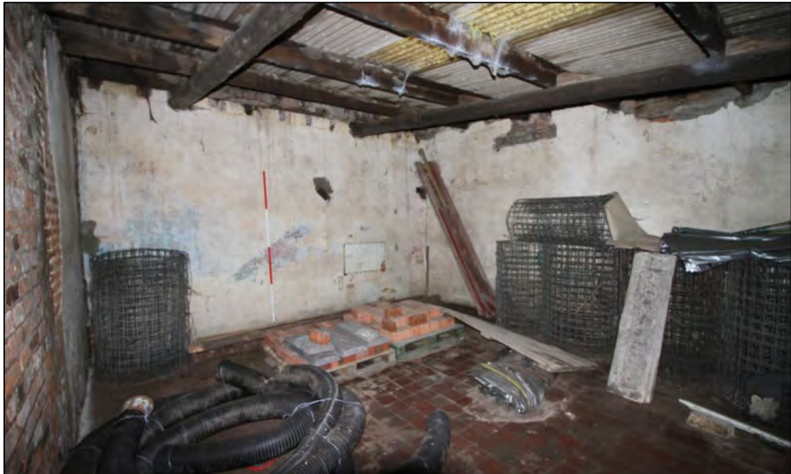
Plate 55: Room G4, looking north-east
