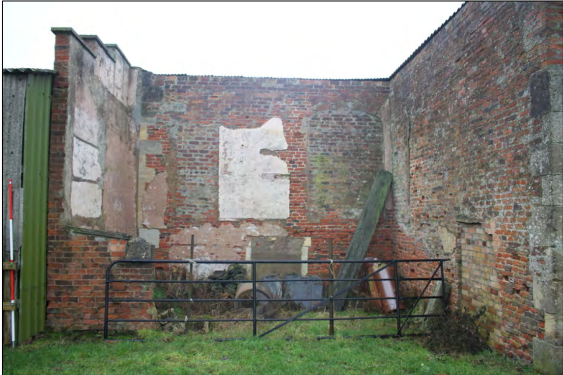
Plate 19: Recessed central section of the northern façade
