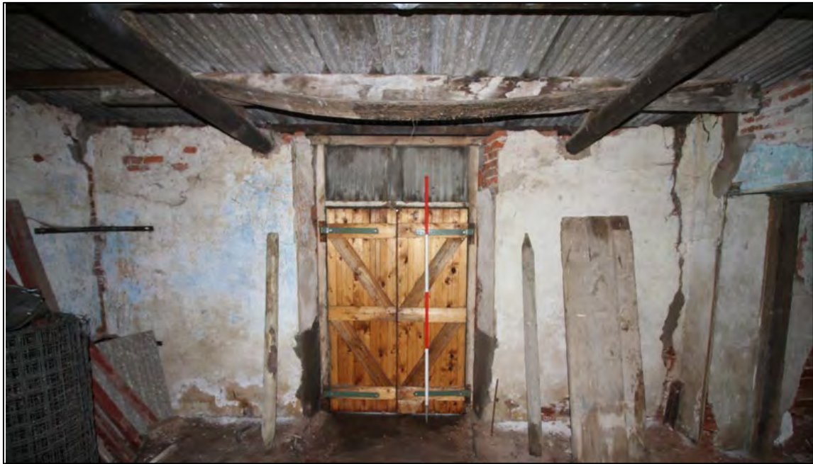
Plate 57: South elevation of Room G4
