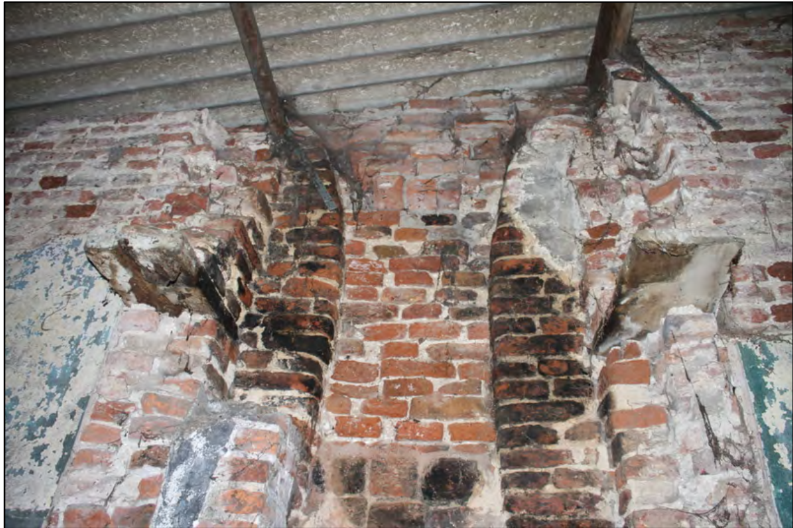
Plate 42: Detail of fireplace cheeks and flue, Room G2
