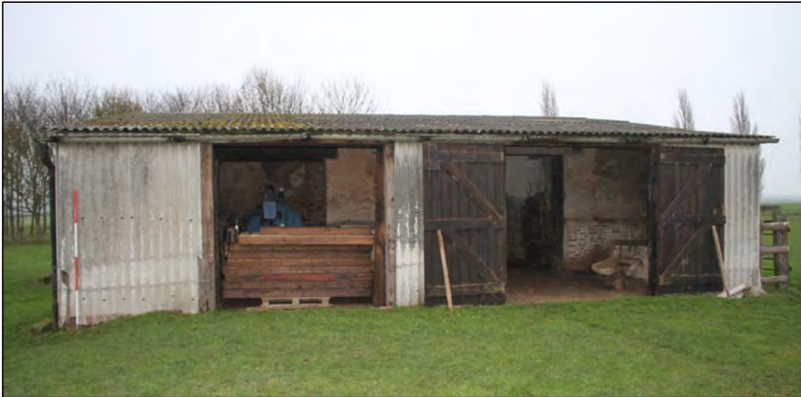
Plate 11: Twentieth-century addition to the western façade of the original structure
