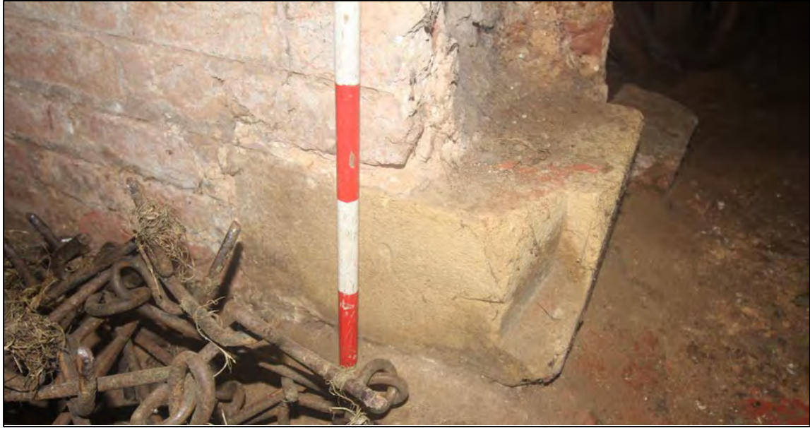
Plate 28: Moulded sandstone block forming part of window jamb at cellar level
