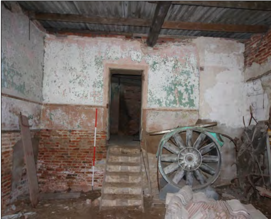
Plate 35: East elevation of room G1
