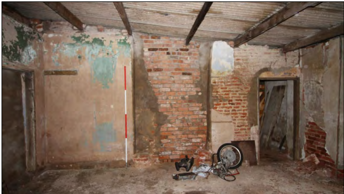
Plate 53: East elevation, Room G3, with inserted door and removed chimney breast
