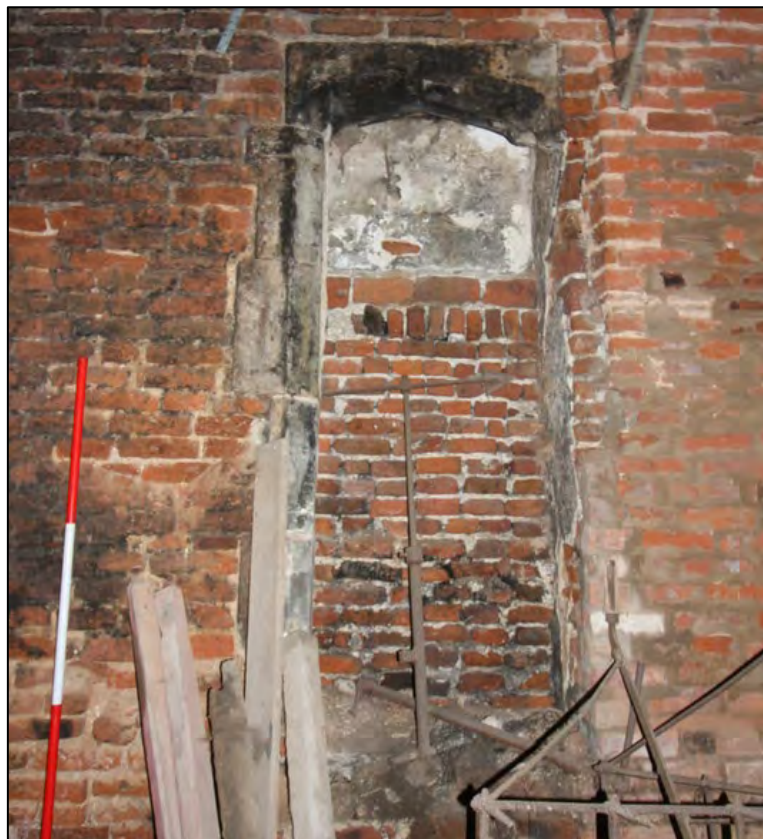
Plate 32: Moulded sandstone surround of narrow aperture in south wall, Room G1
