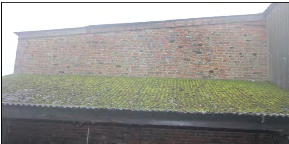
Plate 16: Eastern elevation above the single-storey cart shed
