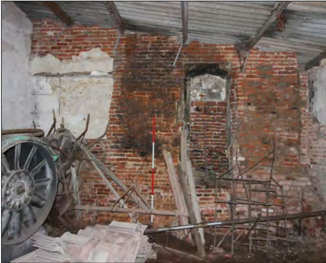
Plate 33: South elevation of Room G1, with sooting to left of blocked window
