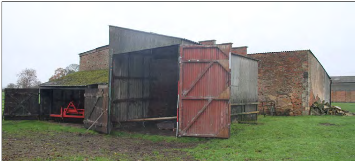
Plate 15: Corrugated sheet timber framed sheds to the east of the brick-built structure
