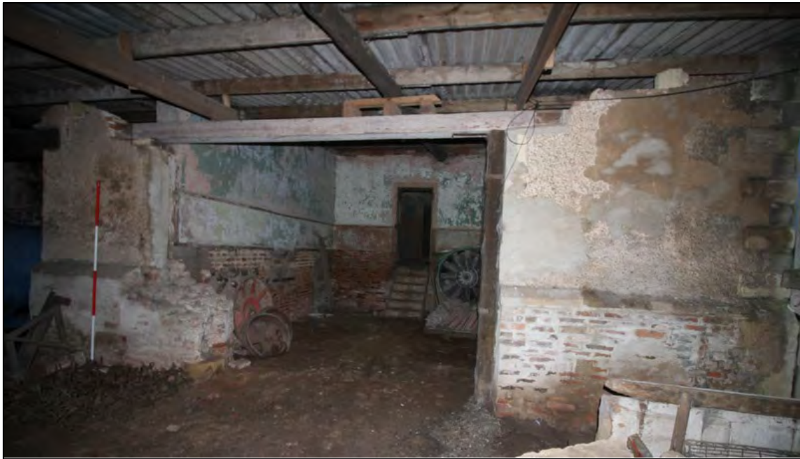
Plate 24: Southern and central sections of the east wall of Room G8
