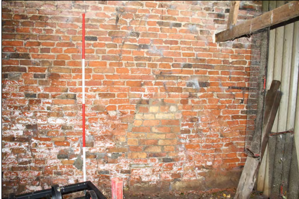
Plate 62: Blocked possible keeping hole within cart shed G7
