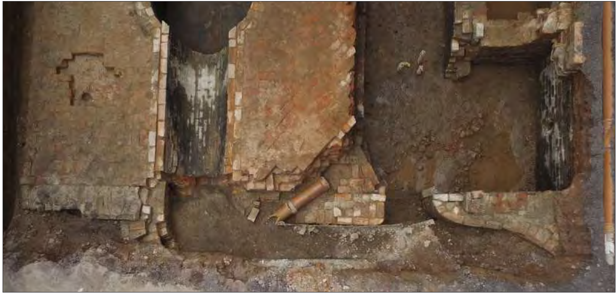
Plate 25: Flues to the north of the chimney, partly forming the south gable of the northern boiler house
