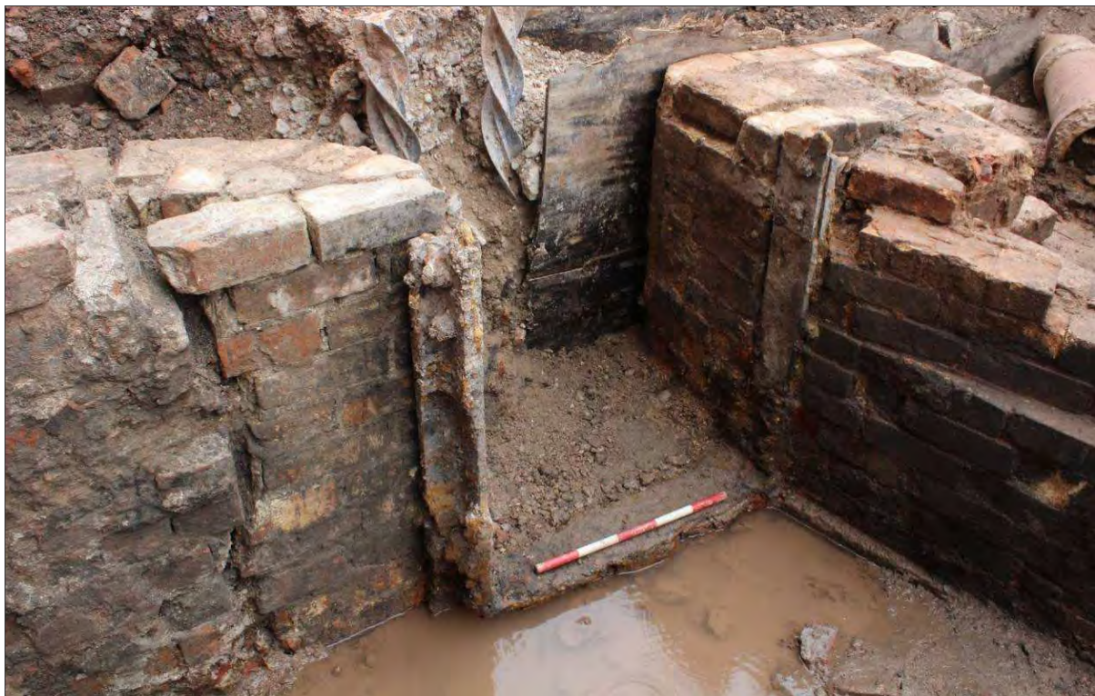
Plate 29: Metal damper constructed against the opening on the south-east side of walls 010 and 014 (0.50m scale)
