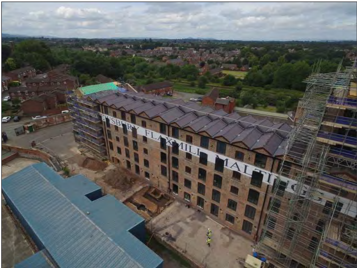
Plate 1: Recent aerial view across the Main Mill and excavation area
