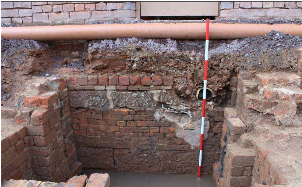
Plate 14: North-west elevation of the foundation of the Main Mill, wall 019 (2m scale, 20cm increments) Note the stone courses, brick infill and later truncations
