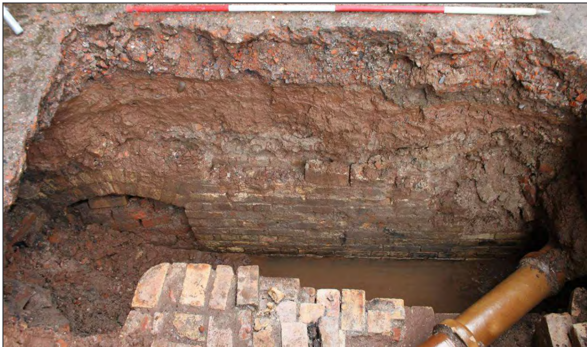
Plate 5: Watching brief trench showing remains of the flue located to the north of the chimney
