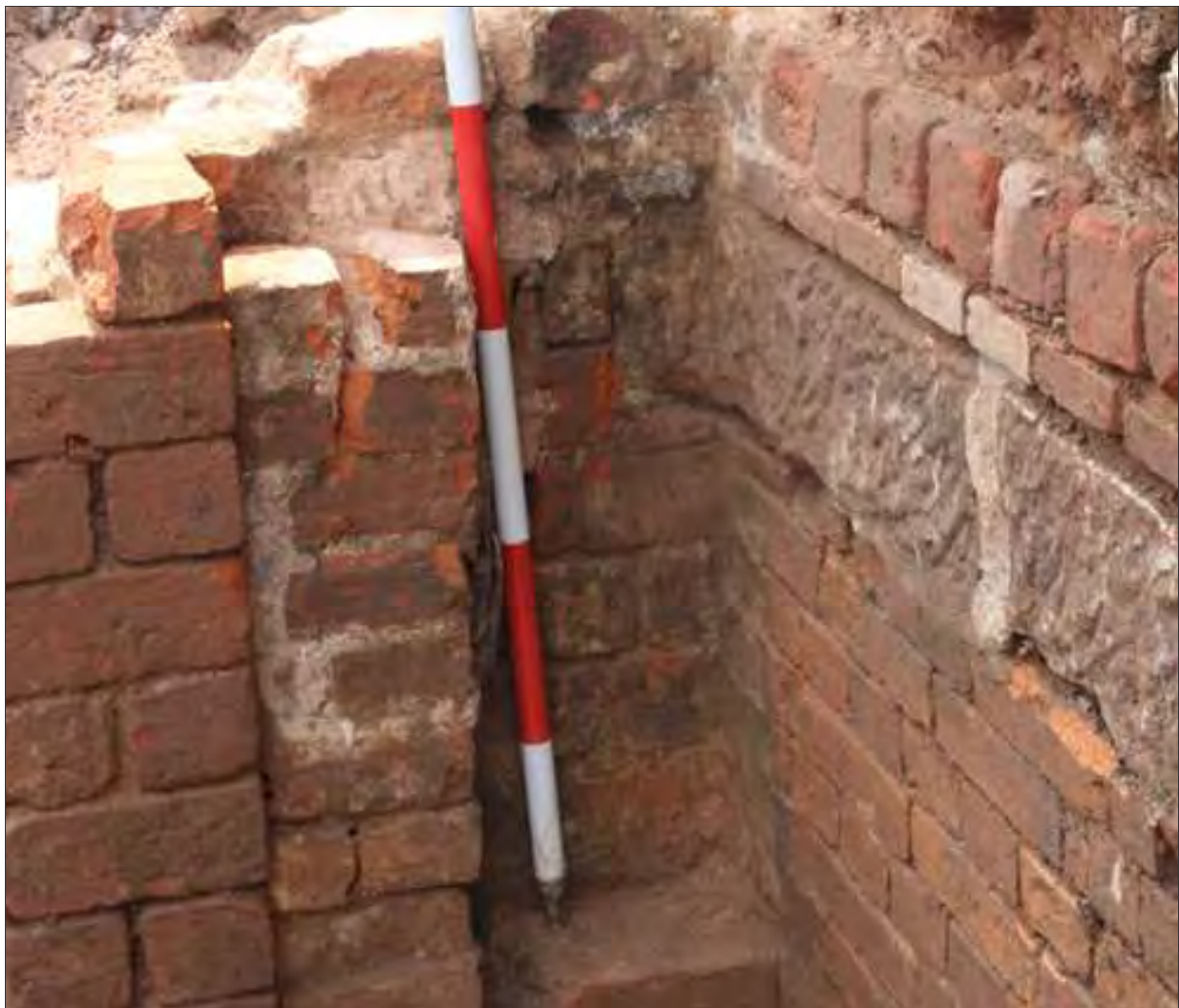
Plate 11: Walls 016 after removing the brick infill (022) to reveal the rebated stone block
