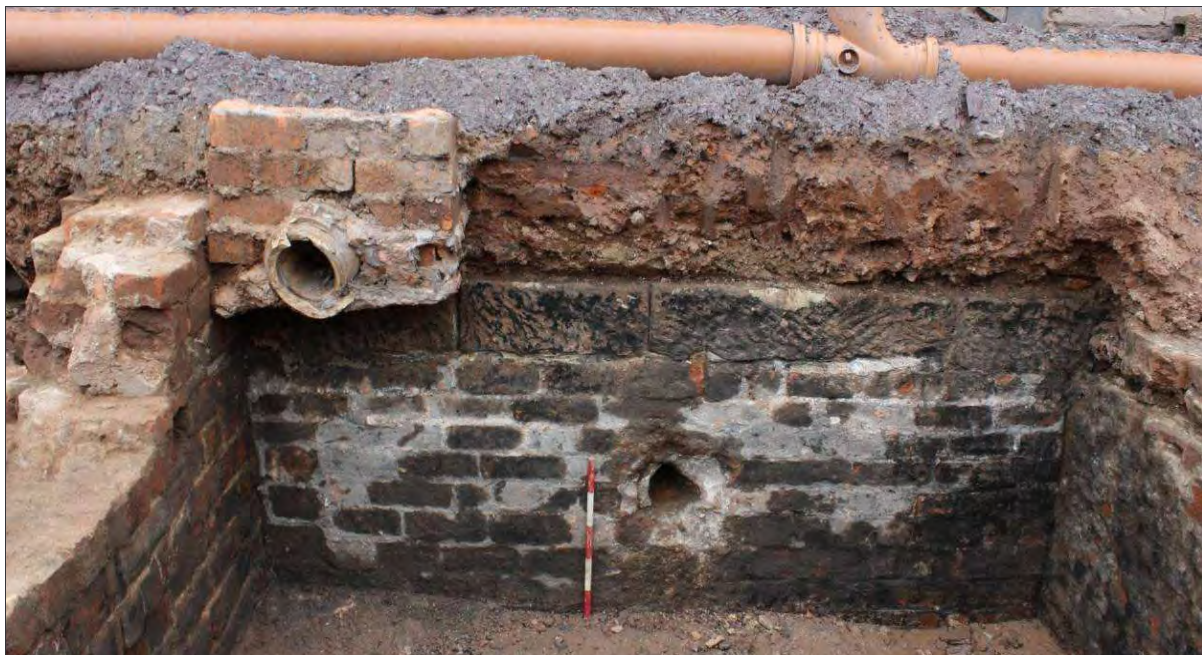
Plate 15: North-west elevation of the mill foundation visible to the north of the privy tower. Note the soot-staining on the face of the wall
