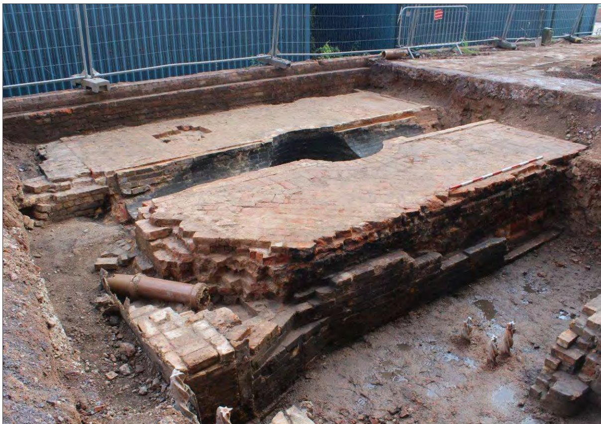
Plate 31: General view of the north-west side of the chimney base, looking over the economiser bed
