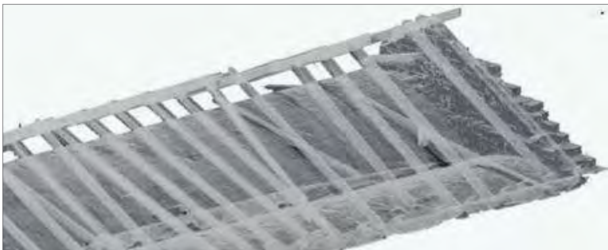
Plate 33: Extract from point cloud model showing the pitched roof spanning two brick vaults at the junction between the original and extended mill
