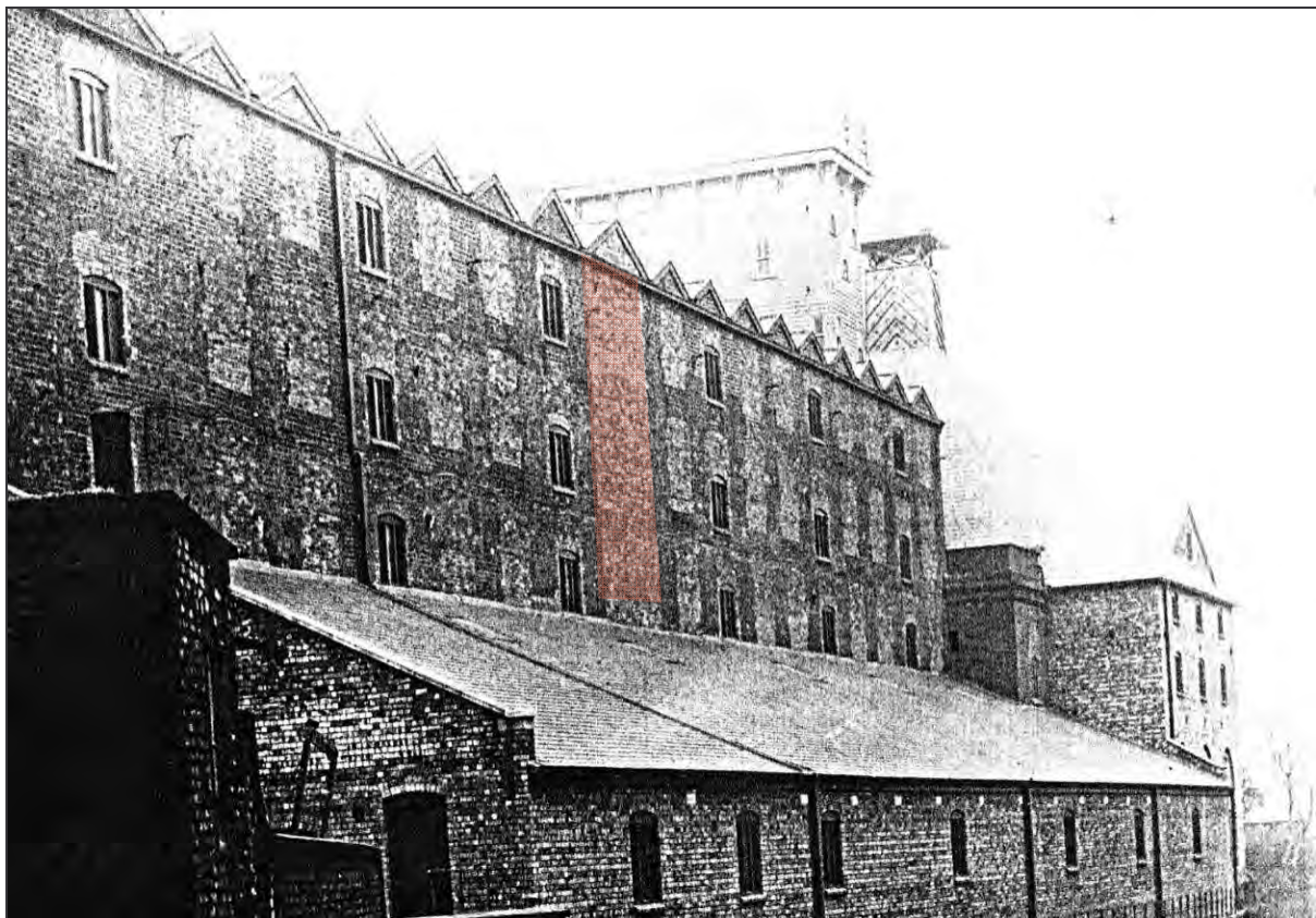
Plate 42: View of the eastern wall of the Main Mill; the scar-line of privy tower is highlighted in pink
