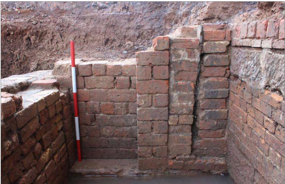
Plate 10: South-west elevation of wall 016 (1m scale) Note the position of the projecting brick piers and later infill
