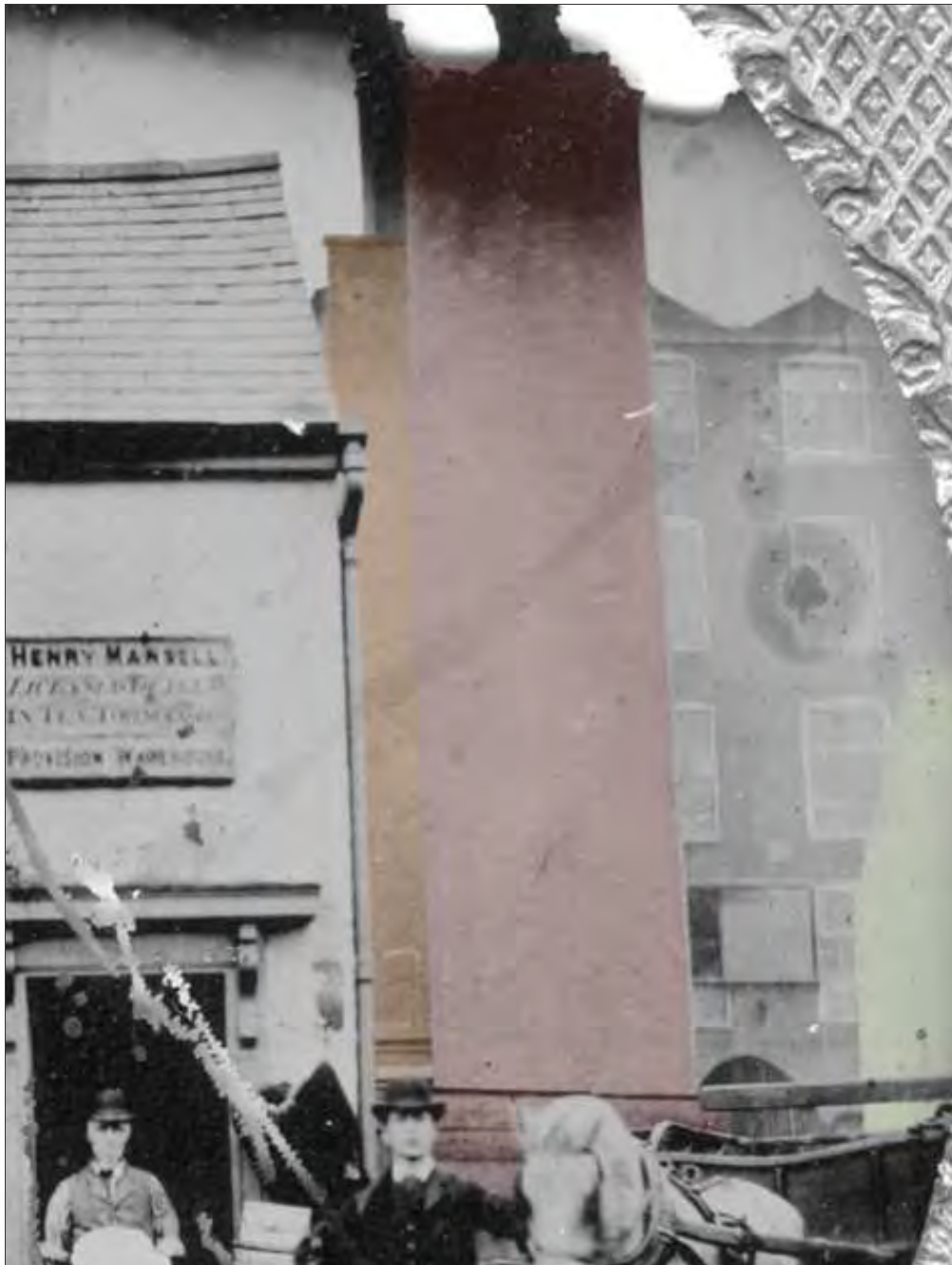
Plate 34: Photograph from the late nineteenth century showing privy tower (orange), chimney (red) and boiler house (green) positioned in front of the Main Mill
