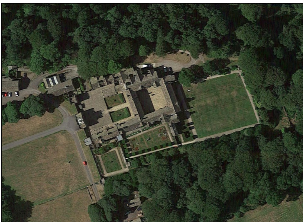
Plate 3: Recent aerial view across Hoghton Tower.
