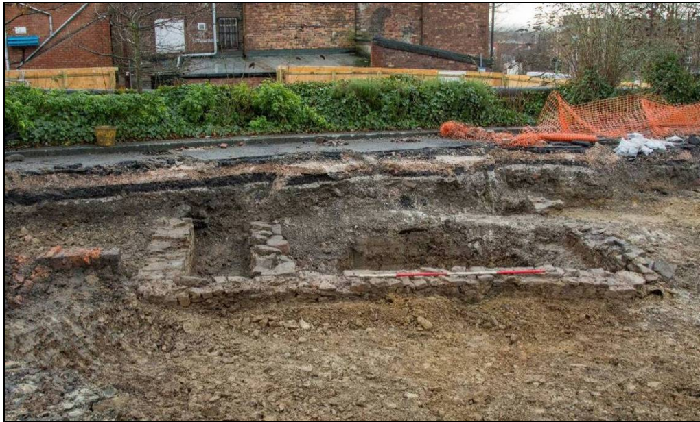
Plate 8: Foundations of stone structure 049, situated in the south-eastern part of the site, looking south
