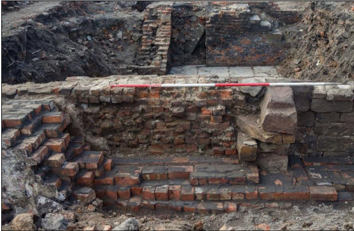
Plate 27: Walls 232 and 232 representing the Chetham Arms and the 20 th -century warehouse, looking south-west. Scale 2m
