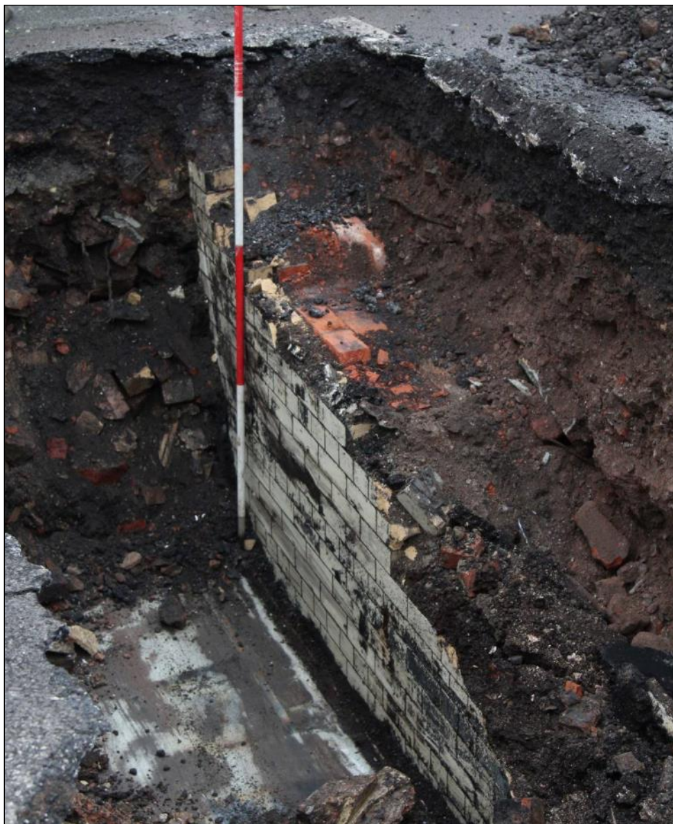
Plate 32: 20 th -century basement partition wall in Trench 3, looking south-east. Scale 2m
