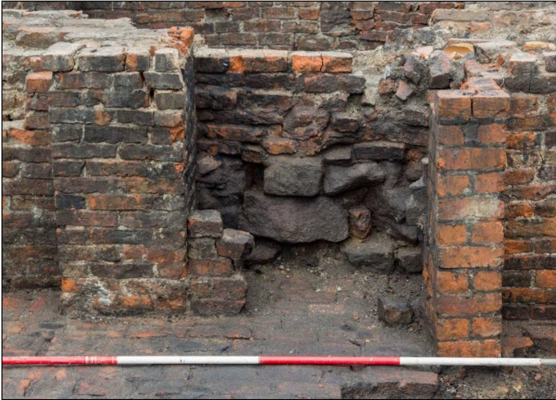
Plate 17: Detailed view of fireplace 211, showing the stone wall foundations, looking north-east. Scale 2m
