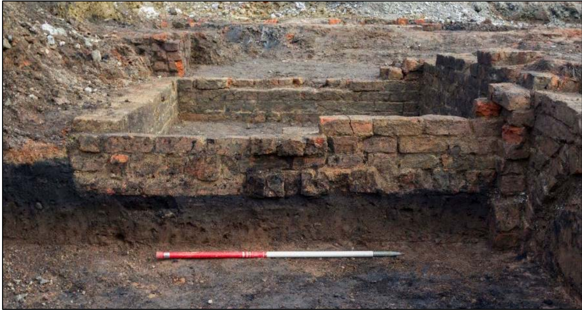
Plate 43: Wall 112, forming the north-western side of the square outbuilding, looking south-east. Scale 1m
