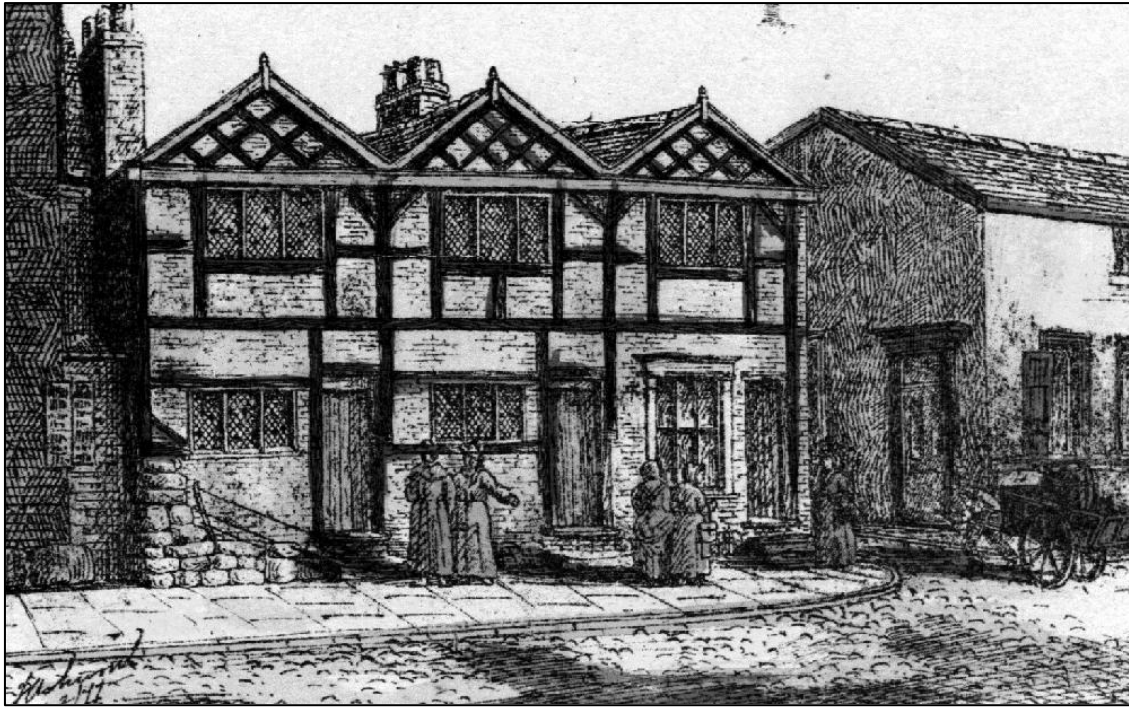
Plate 52: Stone foundations and brick superstructure visible in 17 th -century cottages on Long Millgate on a drawing produced in c. 1850, showing part of the Chetham Arms on the right
