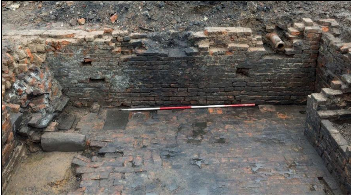
Plate 10: The south-western wall (202), looking south-east. Scale 2m
