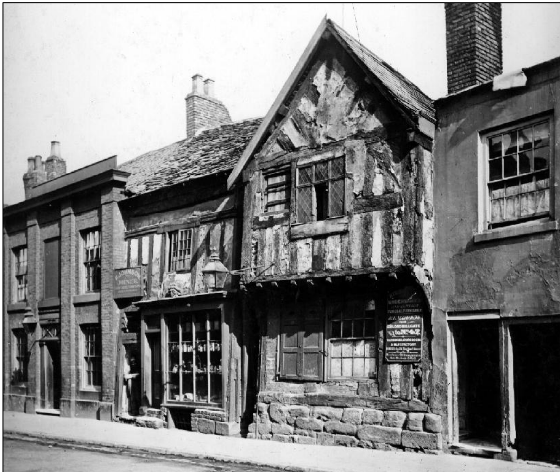
Plate 53: Commercial properties on Long Millgate in c. 1870, clearly displaying stone foundations
