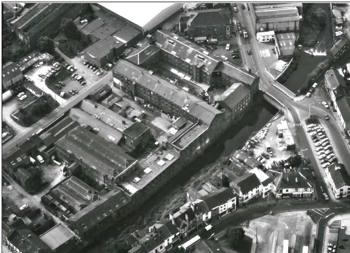
Plate 5: Aerial photograph of Castle Street Mills taken in 1988 (reproduced courtesy of GMAAS)
