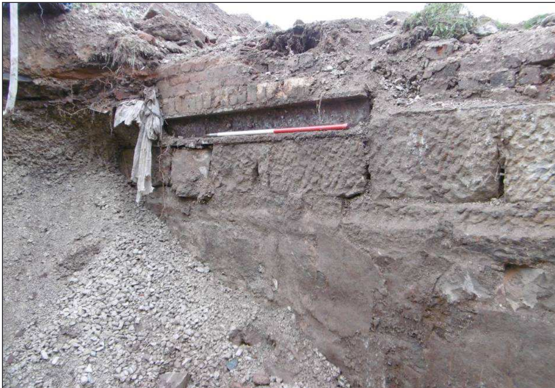
Plate 9: Brick and stone wall 111/125, looking north-east. Joist and re-build at top left
