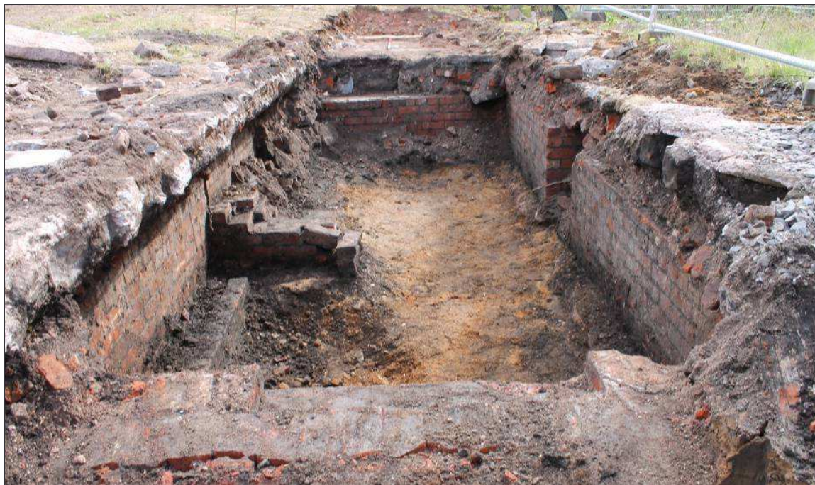
Plate 22: Basement room, looking south
