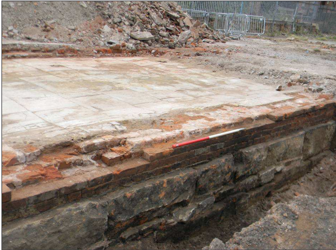
Plate 7: The south wall ( 103 ) and stone foundation ( 112 ) of the spinning block, looking north-east
