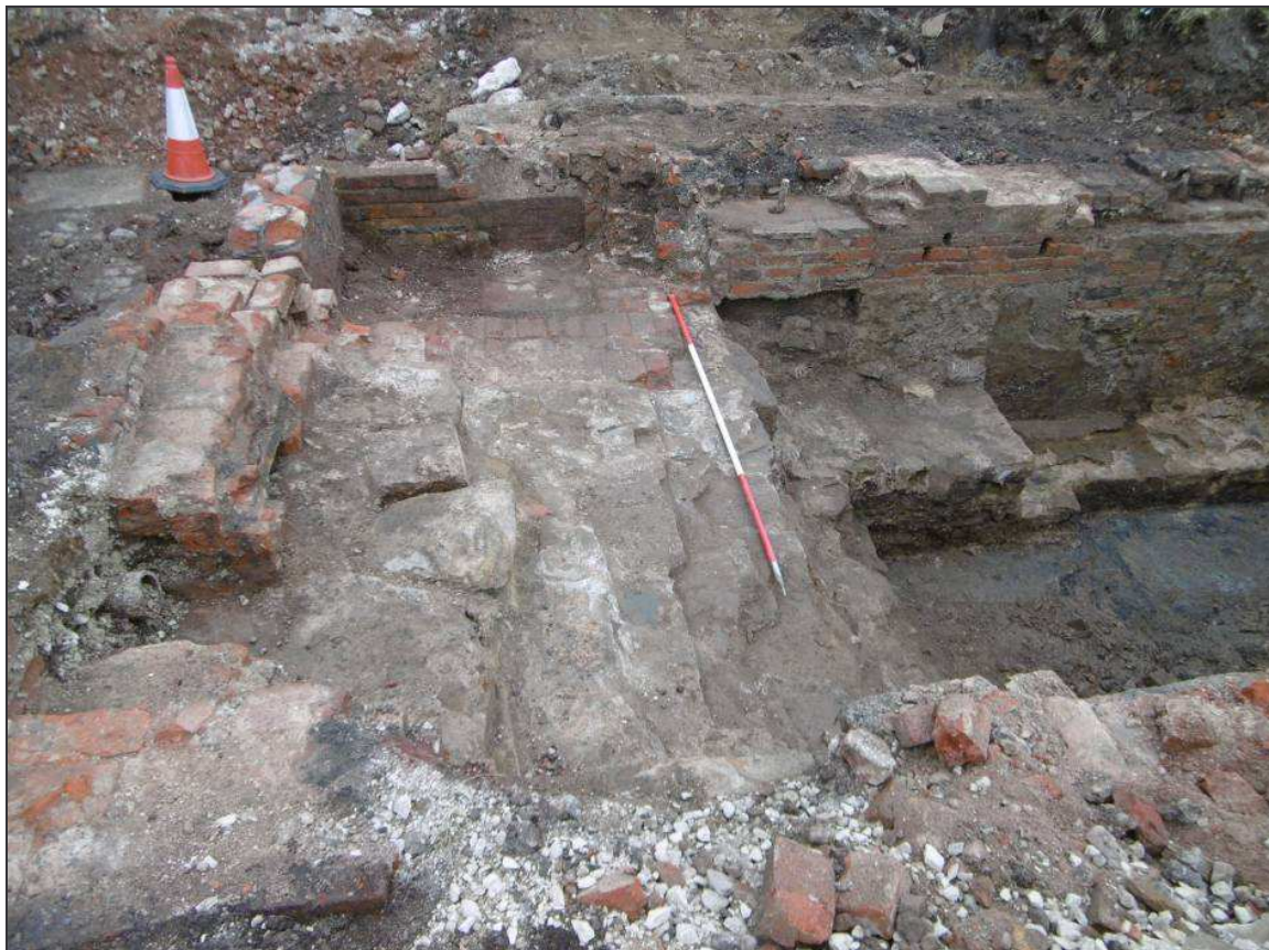
Plate 13: Brick chimney 118 to north of the stone base, looking west. Modern brick blocking at left
