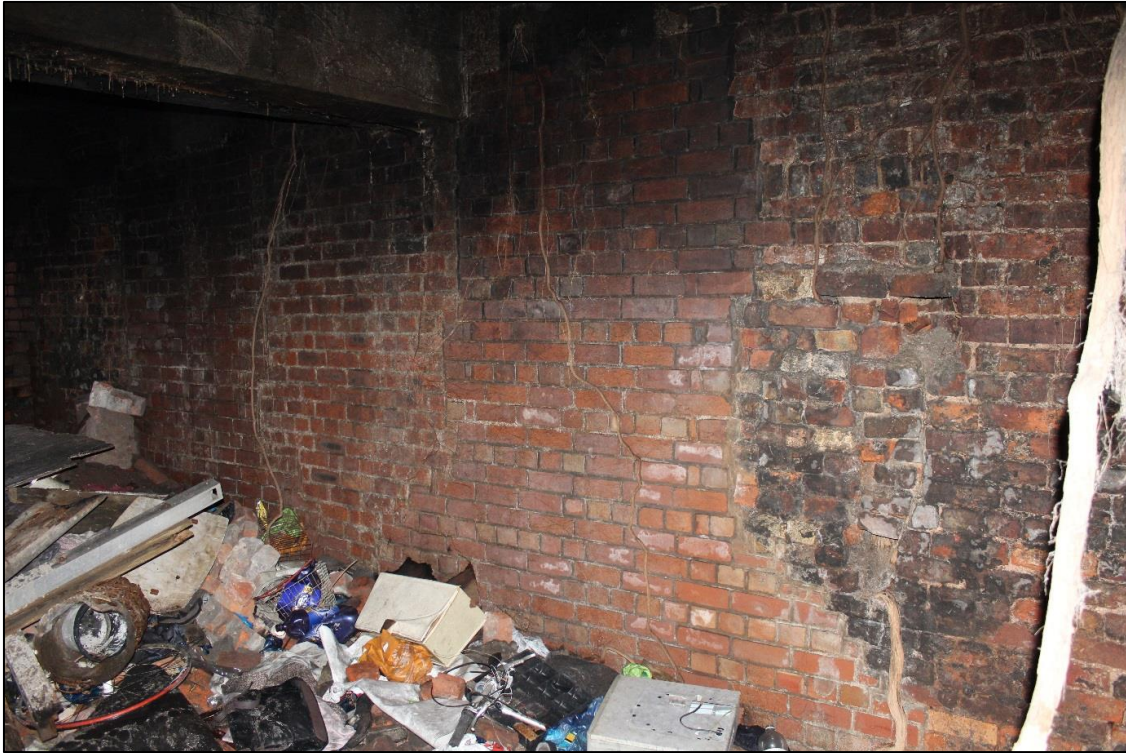
Plate 13: Repaired section of the south-eastern wall
