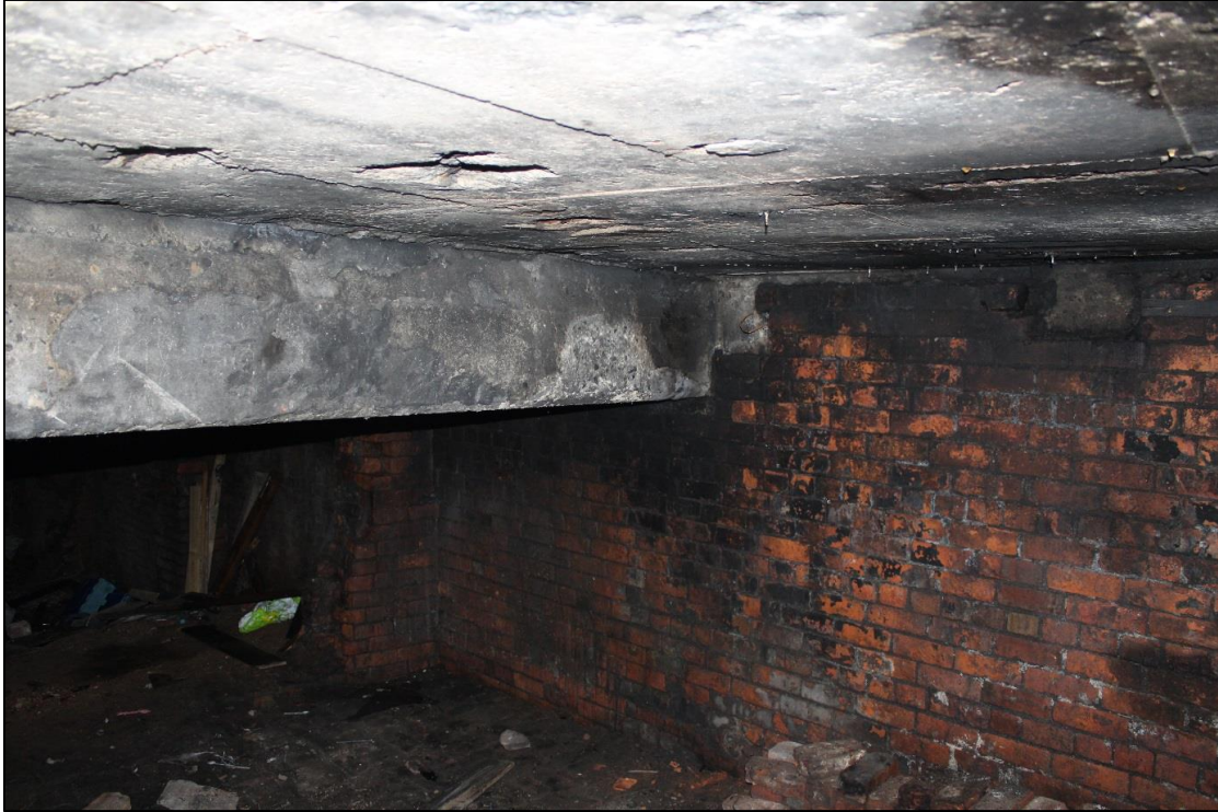
Plate 11: Concrete beam of supporting the concrete section ceiling of the remains of the boiler house
