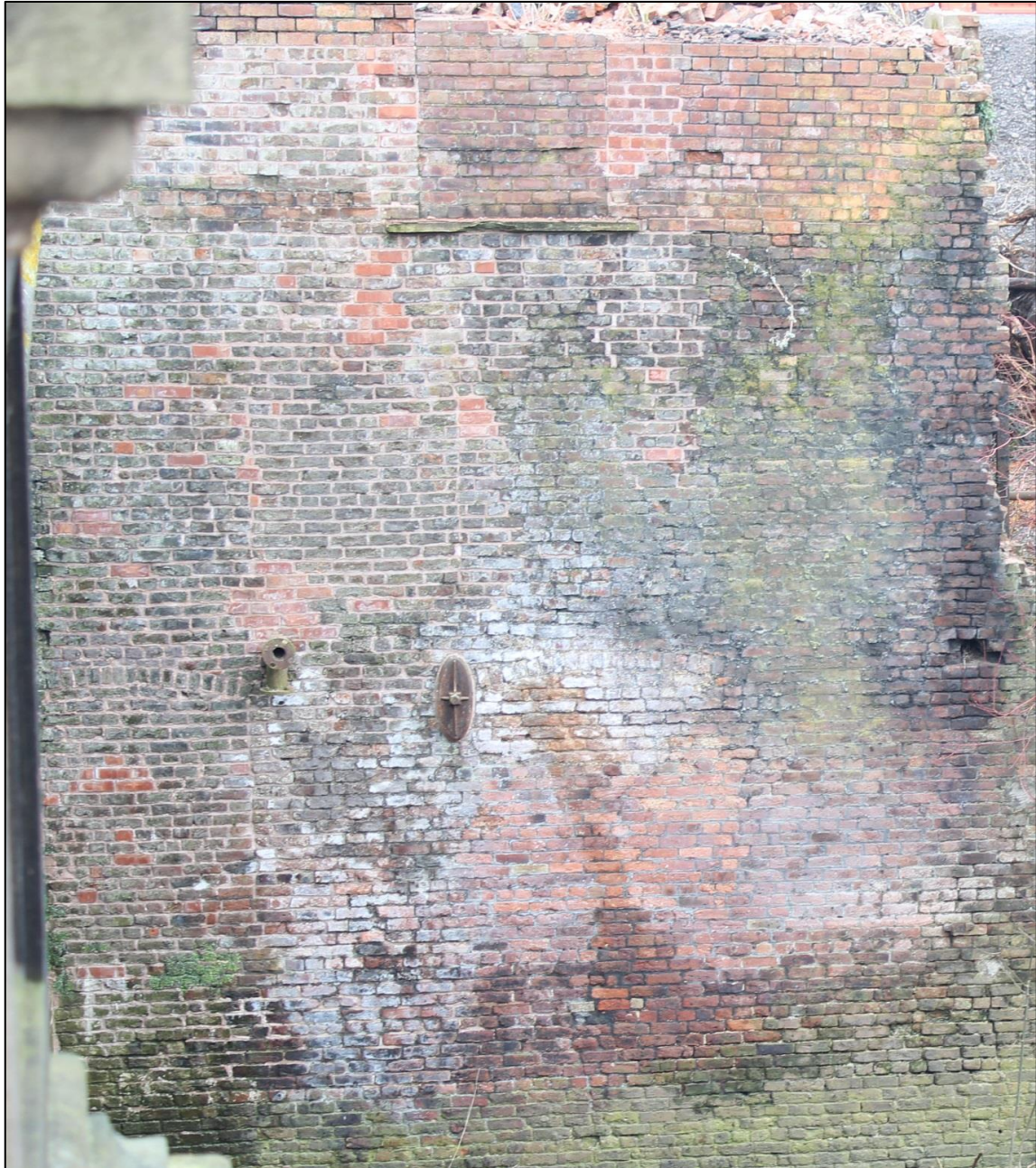
Plate 9: Blocked windows within the north-eastern façade
