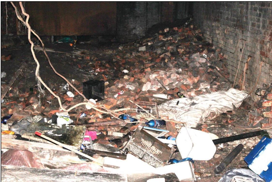
Plate 12: Modern rubbish obscuring the floor of the boiler house
