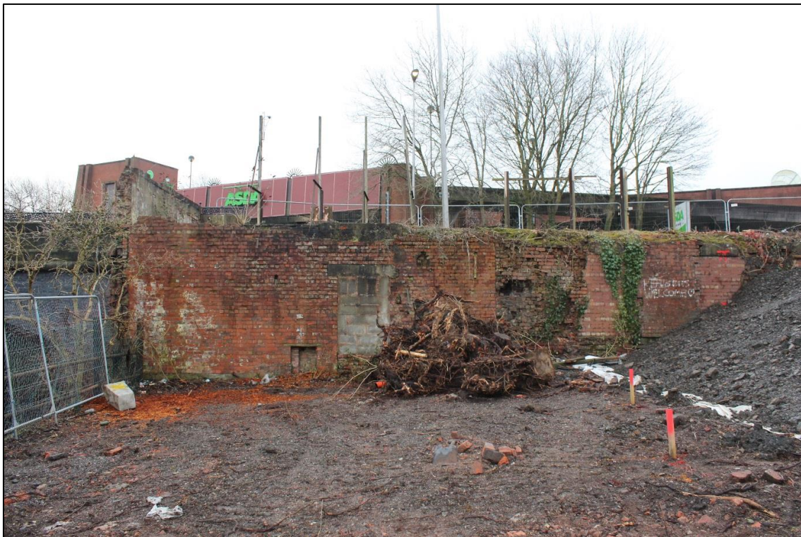
Plate 5: General view of the north-western façade
