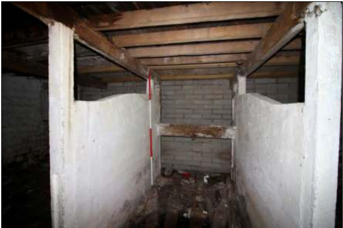
Gleaves Hill Barn 149: Central stall of northern cow house with retained feeding trough
