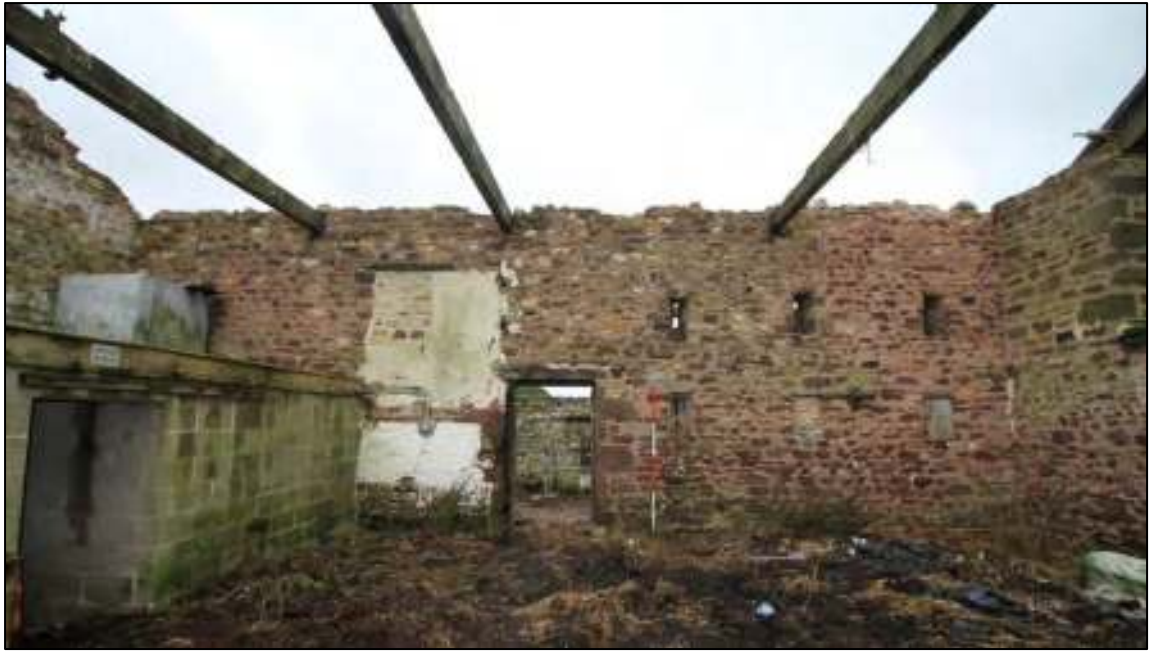
Gleaves Hill Barn 83: West internal wall of original threshing barn
