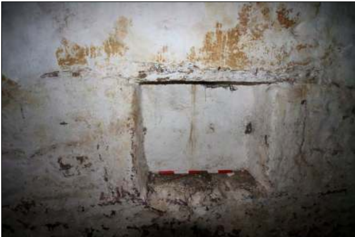
Gleaves Hill Barn 160: Keeping hole in dividing wall
