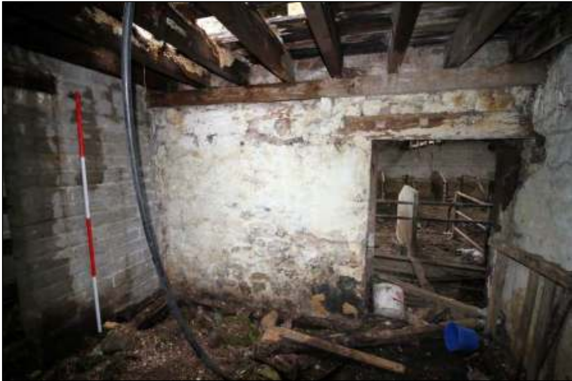
Gleaves Hill Barn 66: South wall of original barn, in west bay
