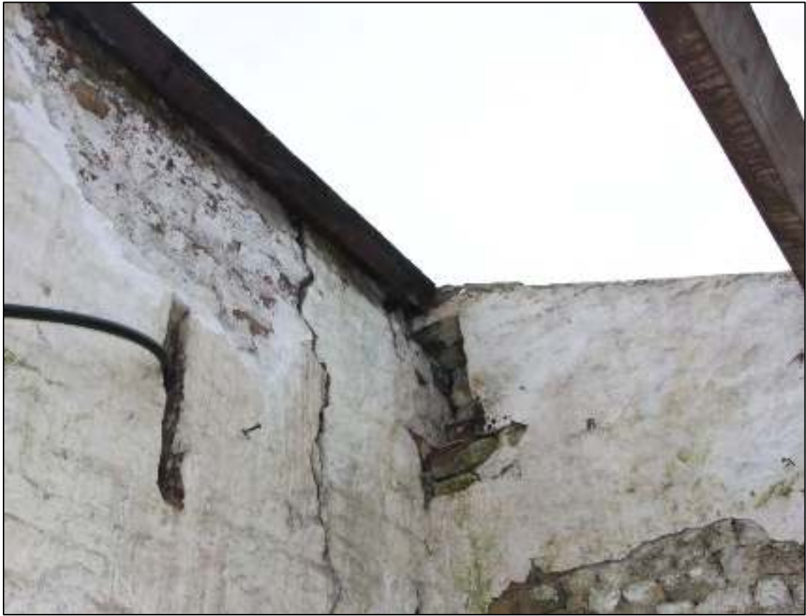
Gleaves Hill Barn 119: Owl hole in south gable of single-storey outshut
