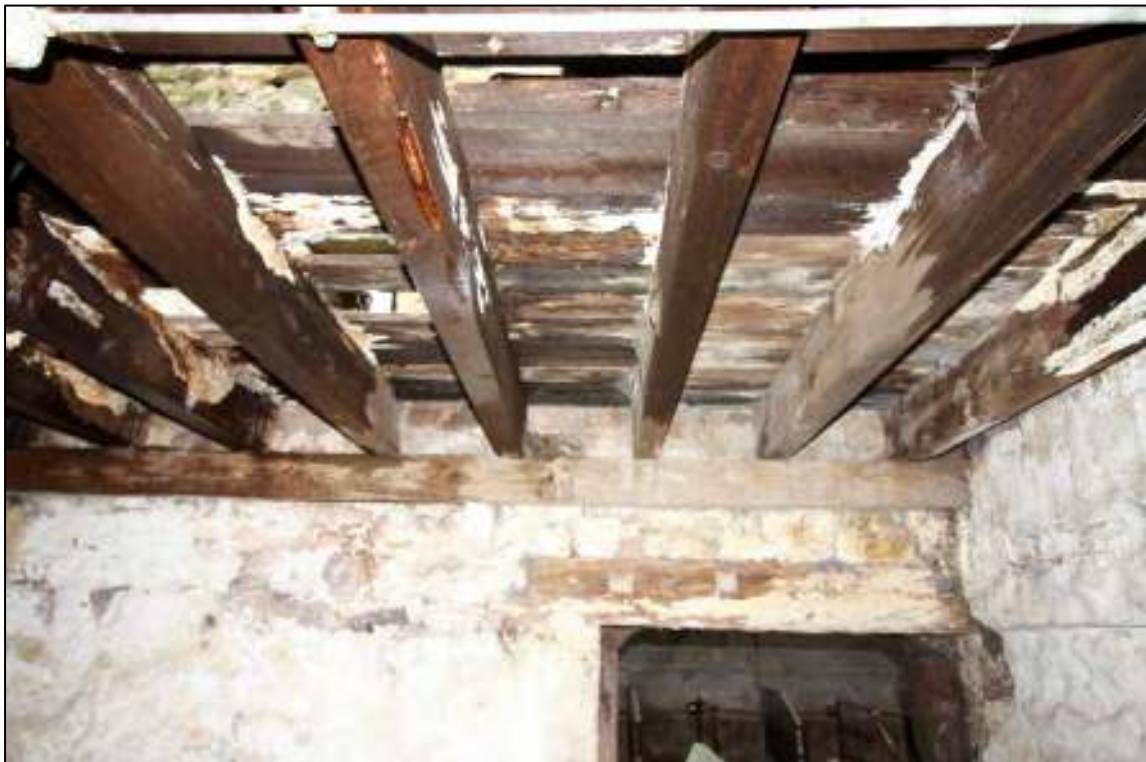
Gleaves Hill Barn 67: Ceiling detail in south cowhouse of original barn
