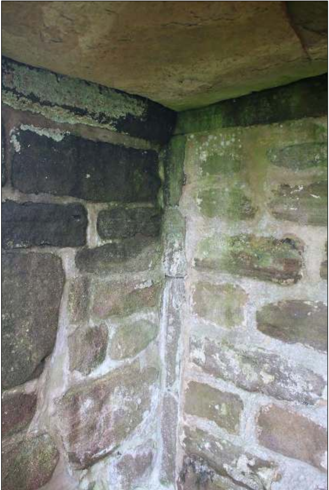
Gleaves Hill Barn 25: Quoins of lower doorway behind wall of stairs
