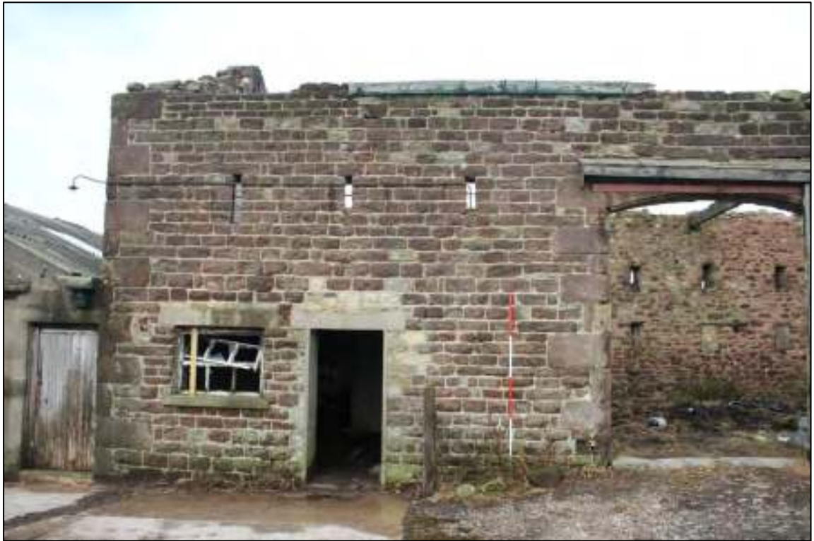
Gleaves Hill Barn 05: Southern bay of original barn
