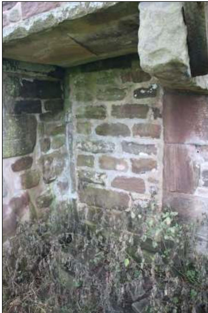
Gleaves Hill Barn 24: Detail of blocked lower doorway, north gable
