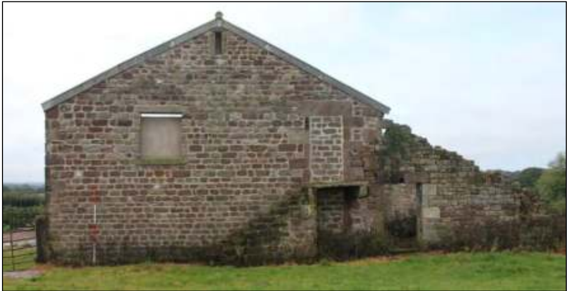
Gleaves Hill Barn 16: North elevation of Gleaves Hill Barn
