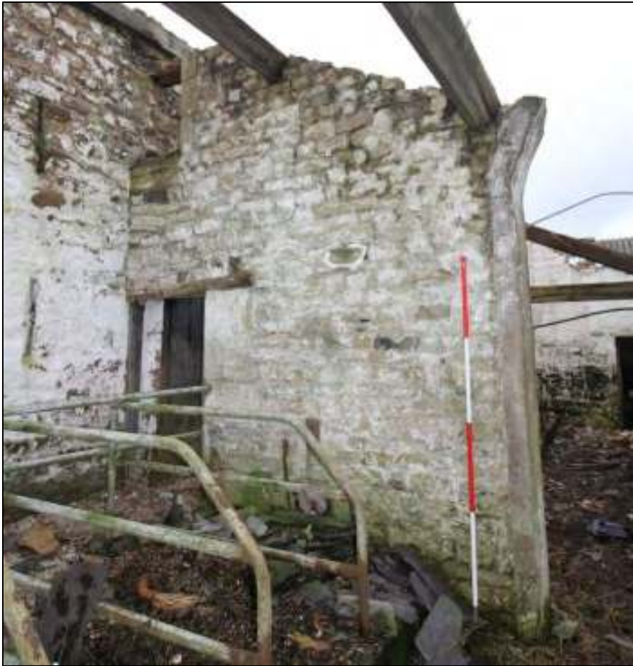
Gleaves Hill Barn 121: Stone dividing wall within single-storey outshut, looking south
