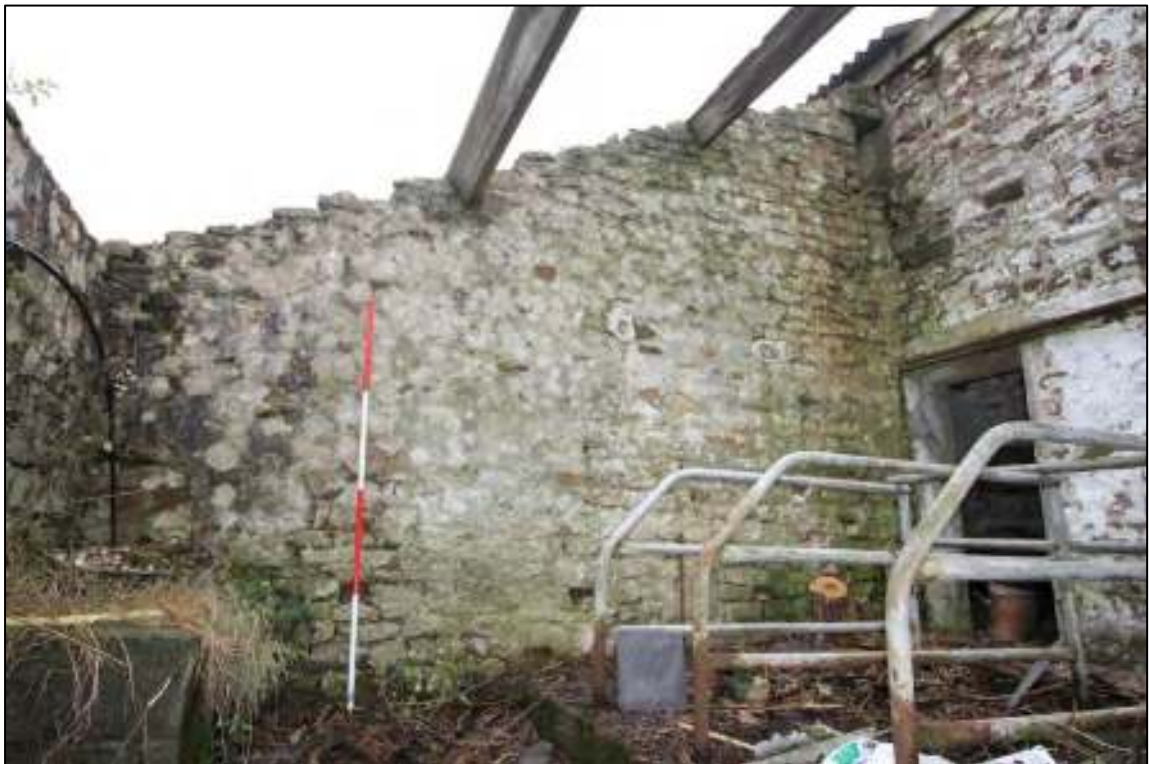
Gleaves Hill Barn 124: North wall of single-storey outshut
