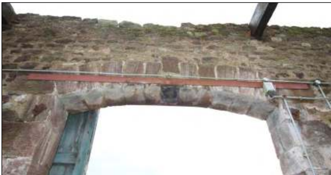
Gleaves Hill Barn 108: Quoined arch of threshing door
