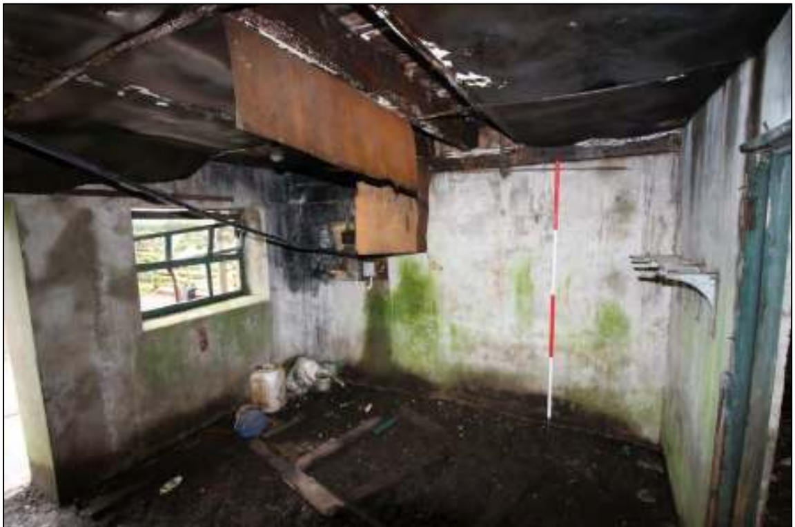
Gleaves Hill Barn 74: Rendered bay in southern cowhouse, looking south
