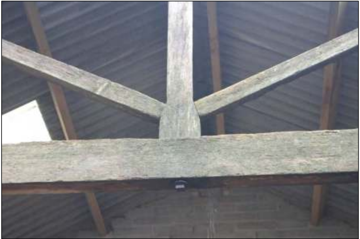
Gleaves Hill Barn 93: Roof truss detail with iron fastening bolt
