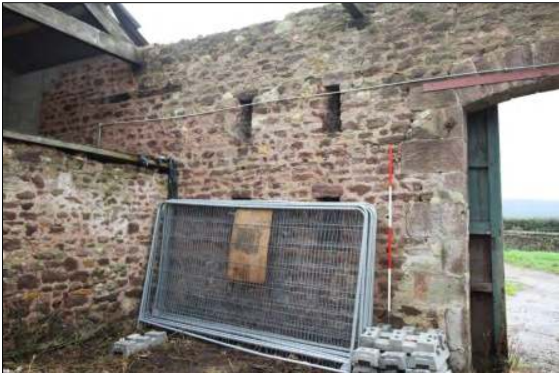
Gleaves Hill Barn 104: Front, eastern wall of threshing barn
