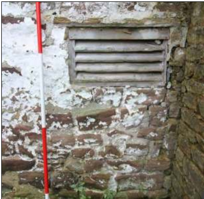
Gleaves Hill Barn 172: Timber louvre inserted into earlier window
