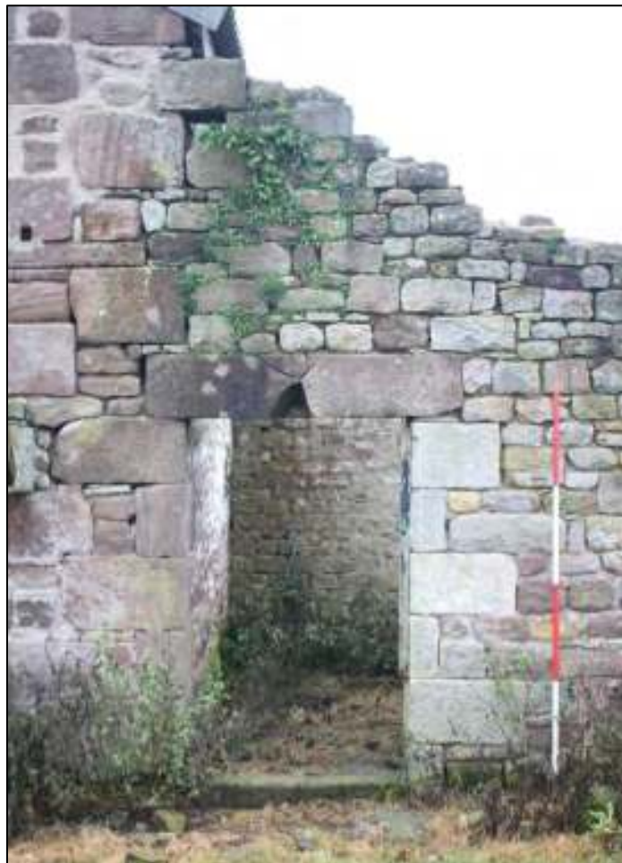
Gleaves Hill Barn 28: Detail of doorway into extension, north gable
