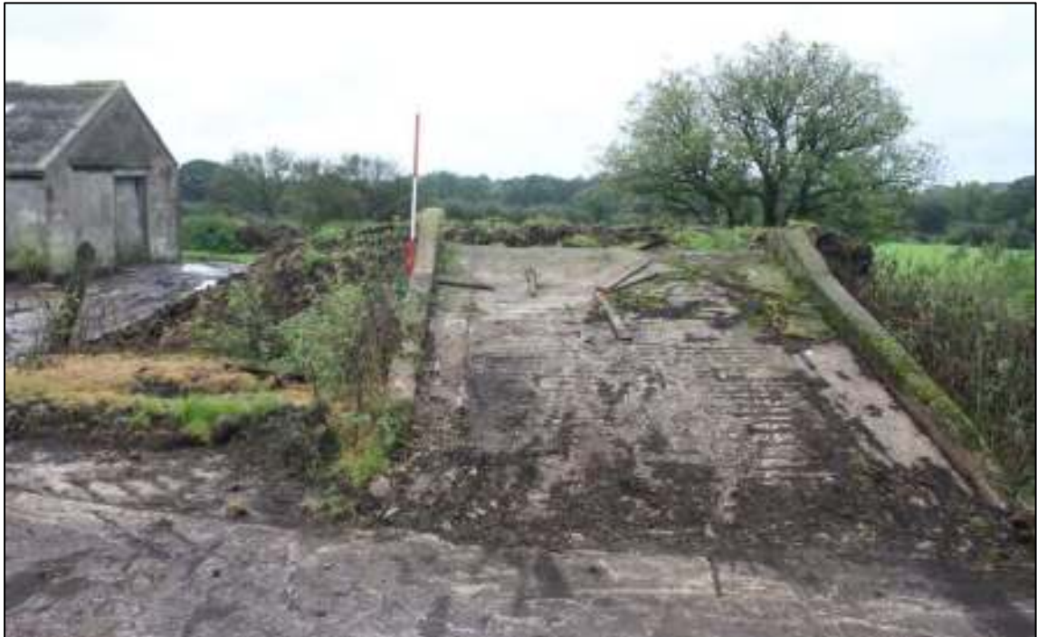
Gleaves Hill Barn 49: Concrete ramp to north-west of barn
