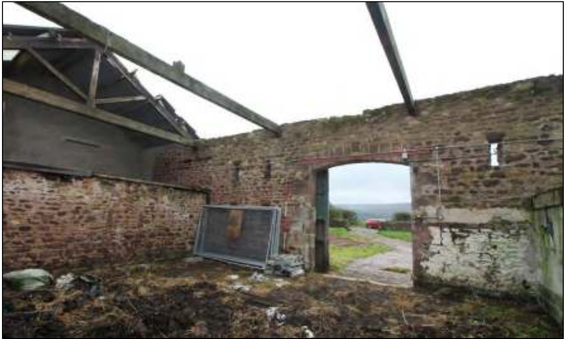
Gleaves Hill Barn 103: Front, eastern wall of threshing barn
