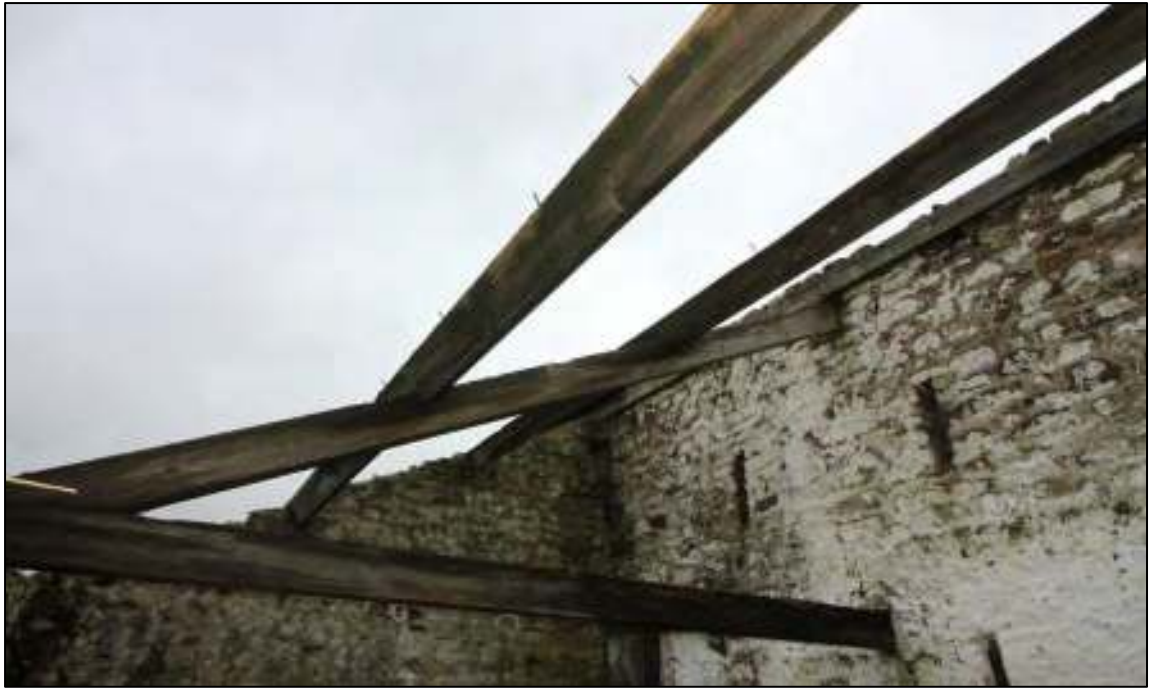
Gleaves Hill Barn 133: Roof truss detail within single-storey outshut
