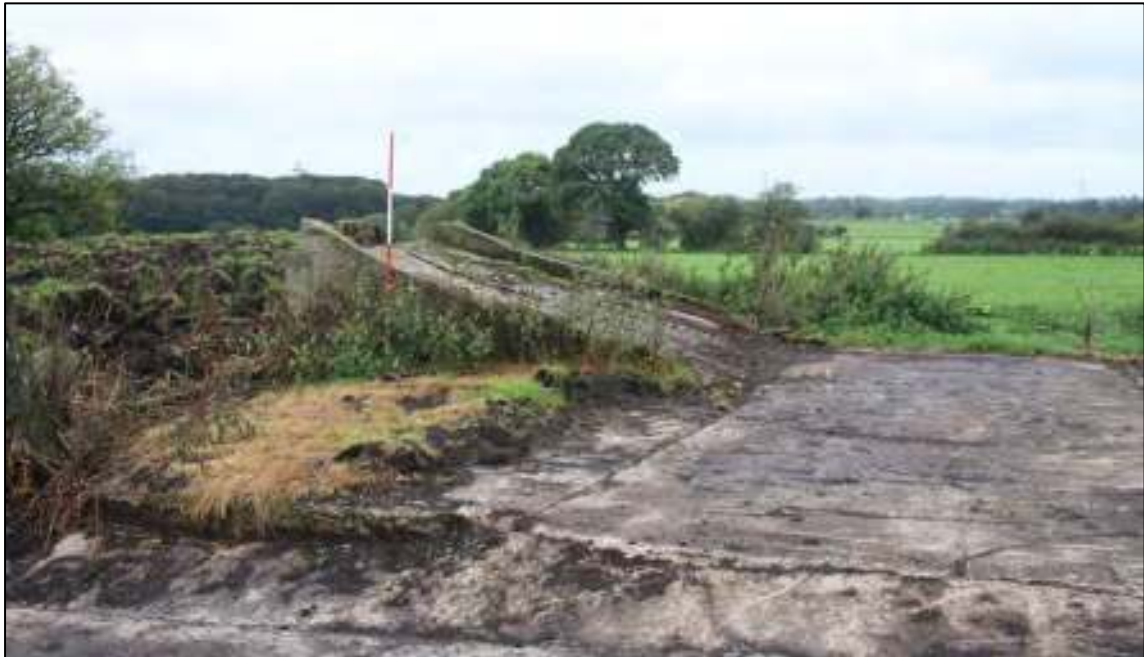
Gleaves Hill Barn 47: Concrete ramp to north-west of barn
