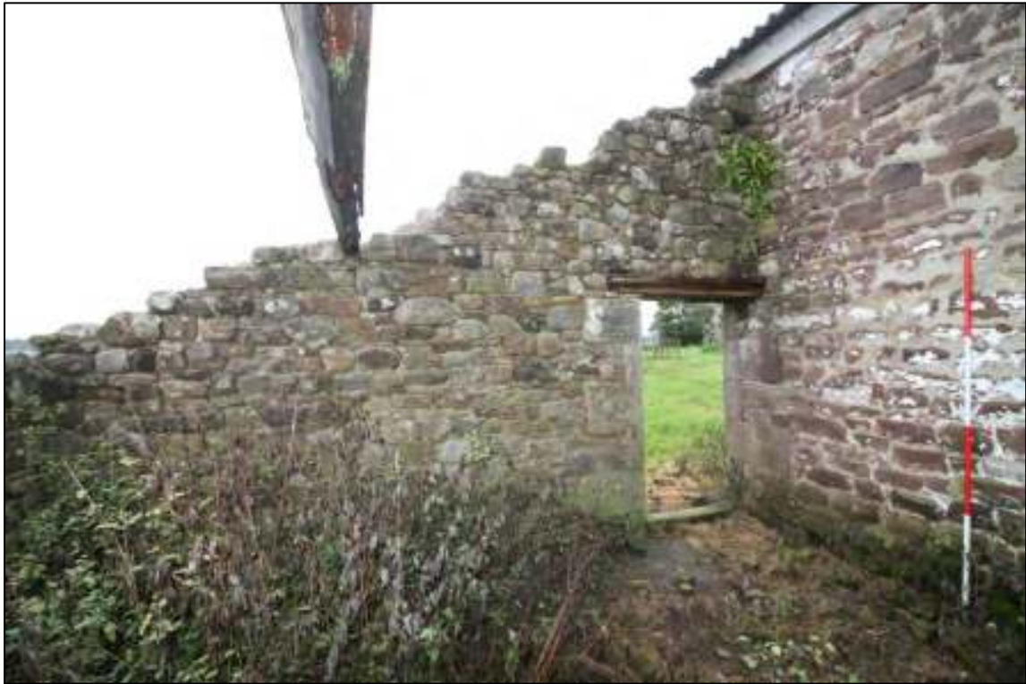
Gleaves Hill Barn 167: North wall of single-storey extension
