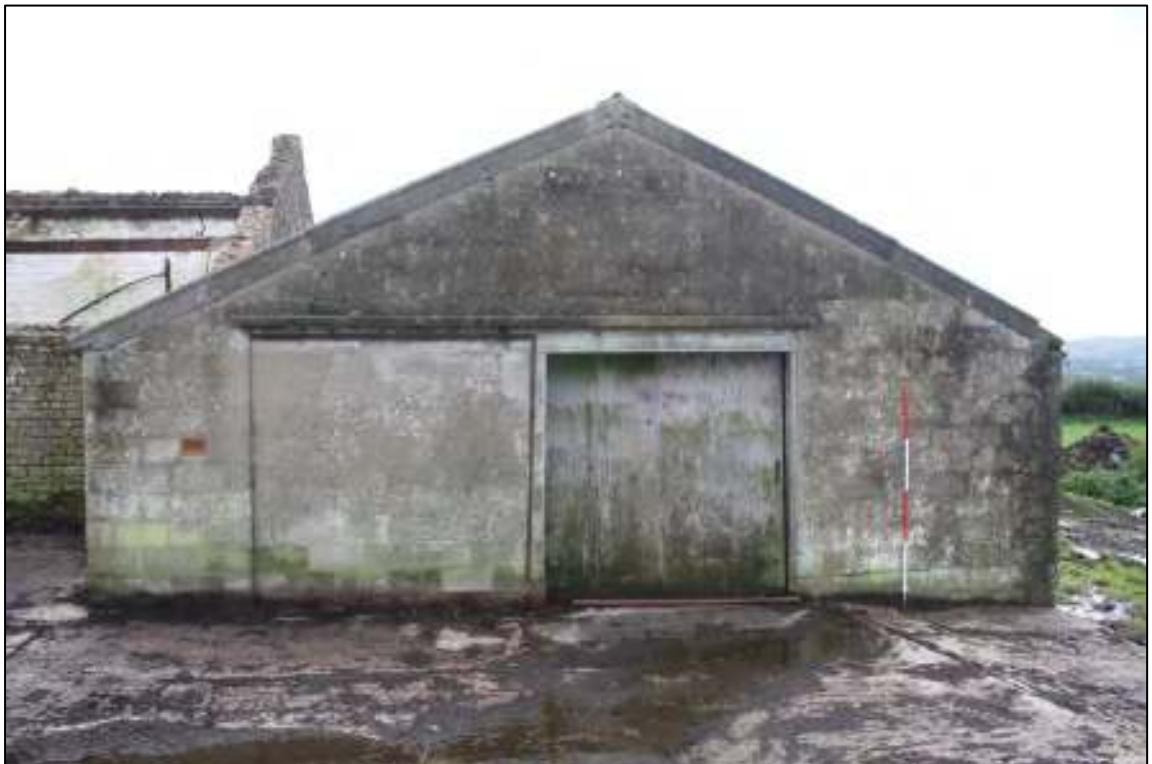
Gleaves Hill Barn 36: West elevation of mid/late-twentieth century southern extension
