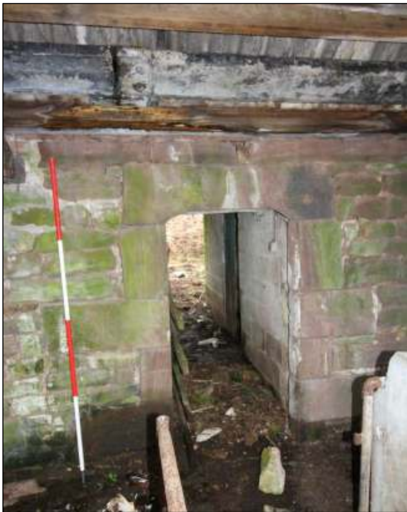
Gleaves Hill Barn 59: Detail of central doorway in original south wall
