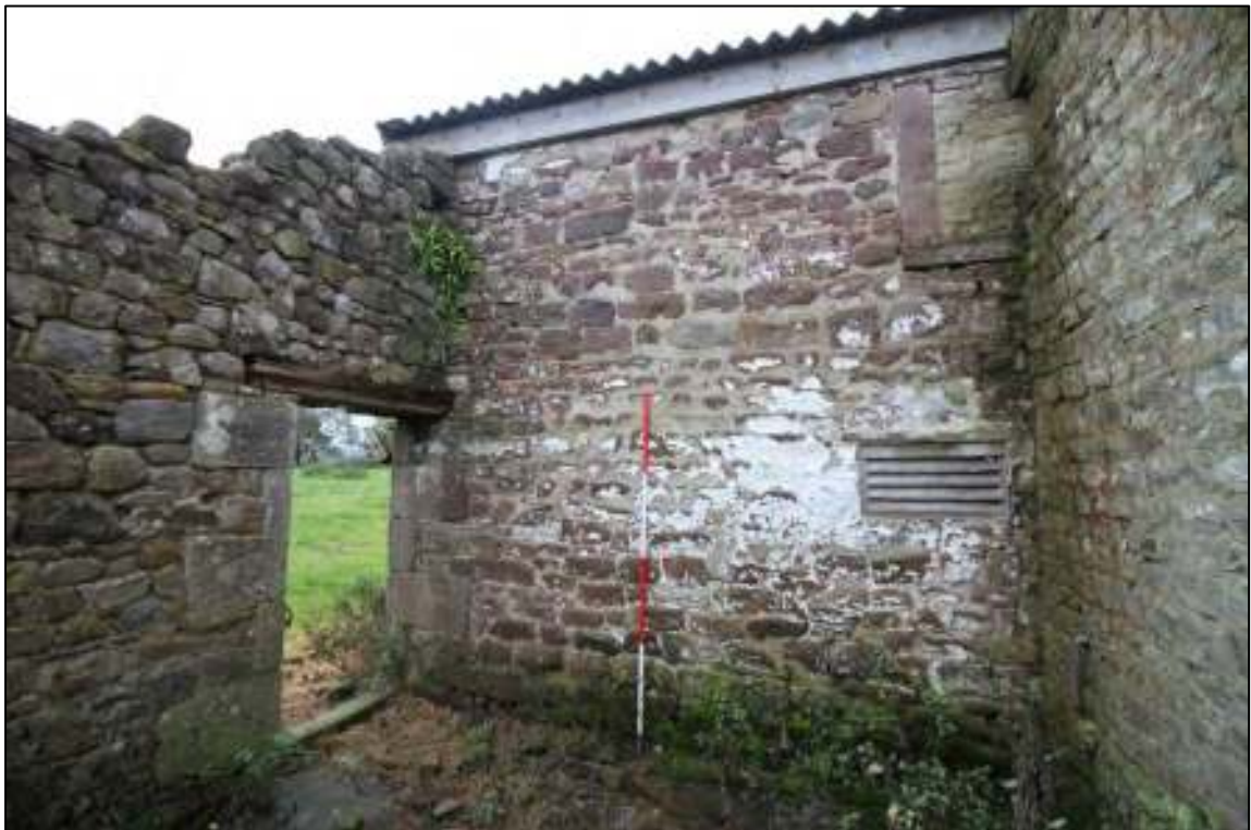
Gleaves Hill Barn 166: Original west wall of barn, butted by extension
