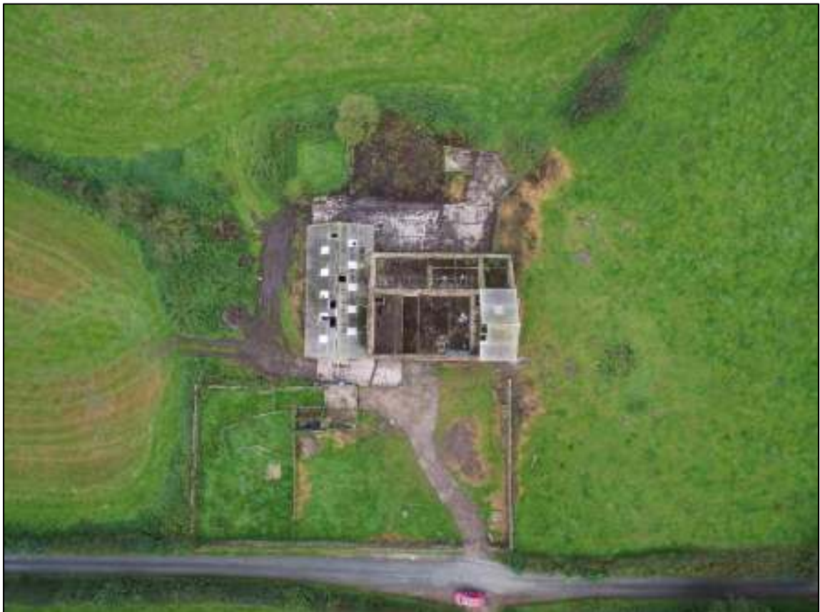
Gleaves Hill Barn UAV 17: Vertical view of the entire complex from the south-east
