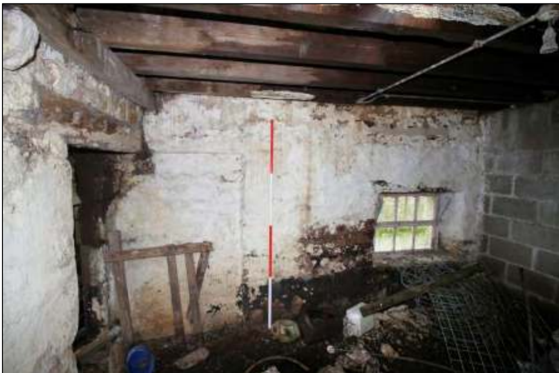
Gleaves Hill Barn 63: North stable of original barn, looking north-west
