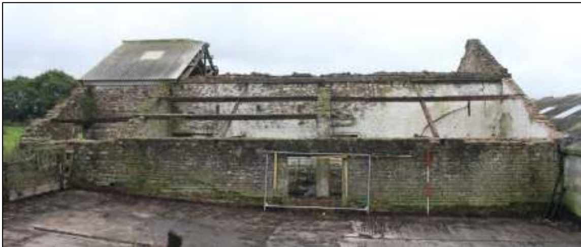
Gleaves Hill Barn 38: West single-storey extension from the rear
