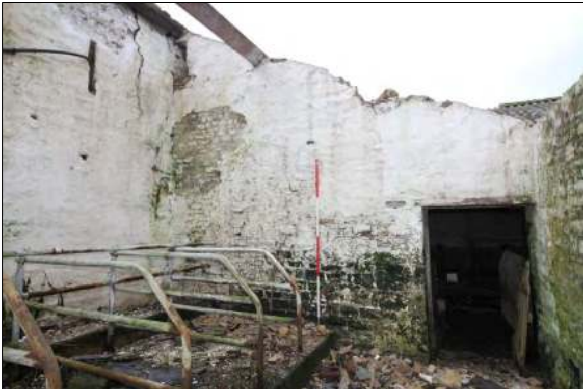
Gleaves Hill Barn 110: South wall of single-storey western cowhouse extension
