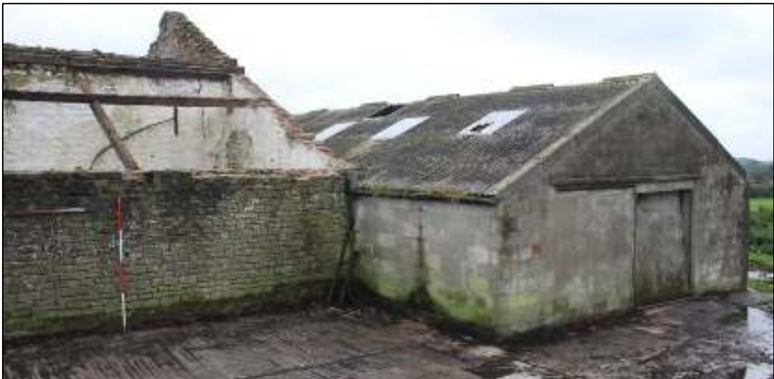
Gleaves Hill Barn 43: Southern extension from the north
