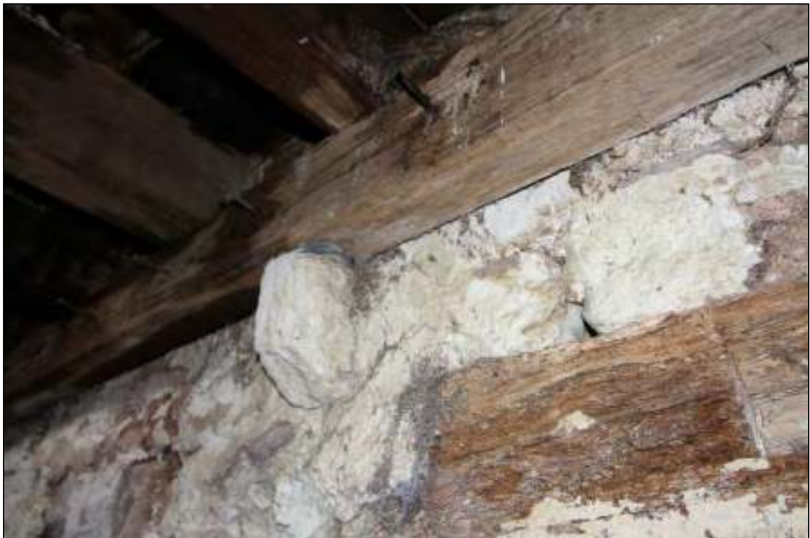
Gleaves Hill Barn 69: Stone corbel carrying ceiling joist, west bay
