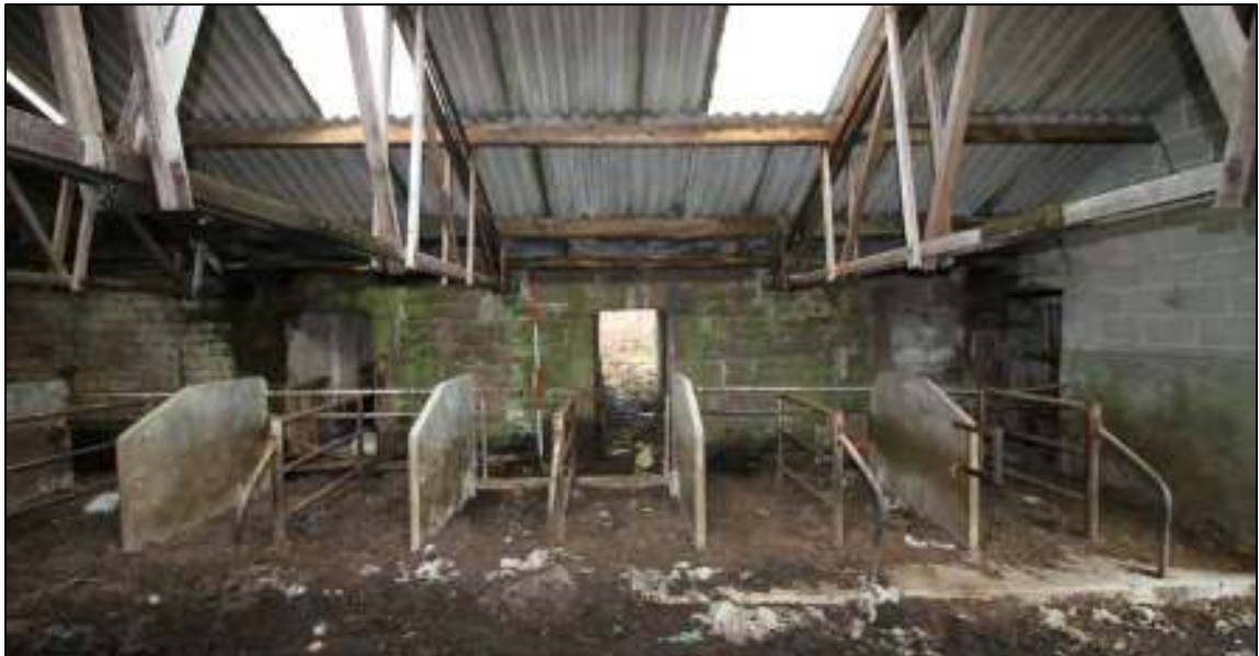
Gleaves Hill Barn 56: Doorways in south wall of original barn
