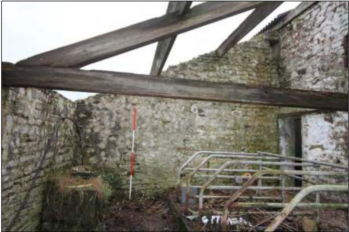
Gleaves Hill Barn 123: North wall of single-storey outshut
