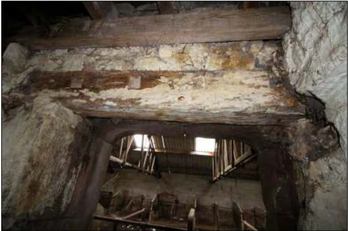
Gleaves Hill Barn 68: Internal door lintel detail, south wall, west bay
