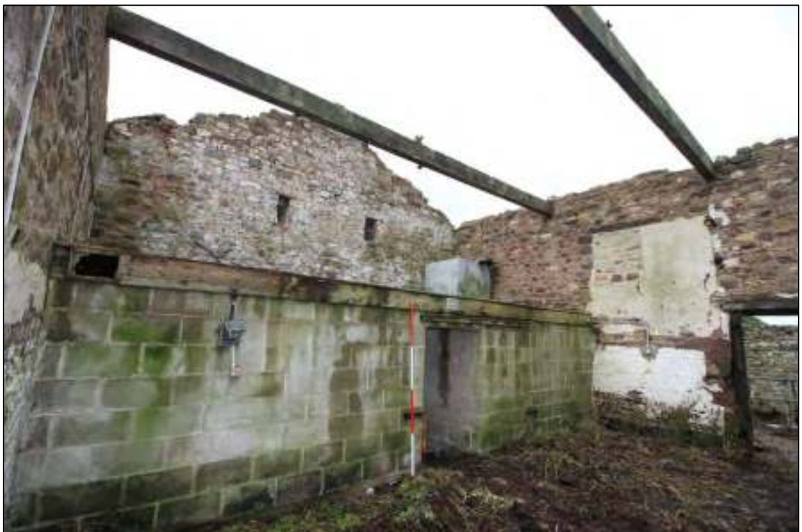
Gleaves Hill Barn 82: Interior of threshing barn looking west
