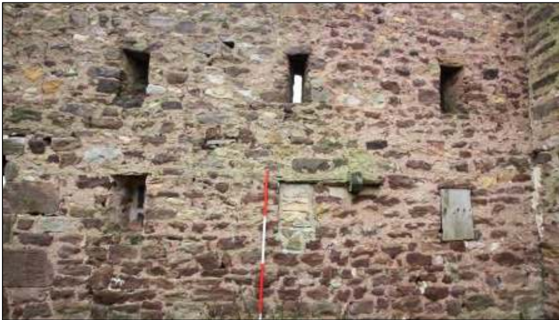
Gleaves Hill Barn 98: extant and blocked ventilators in west wall of threshing barn
