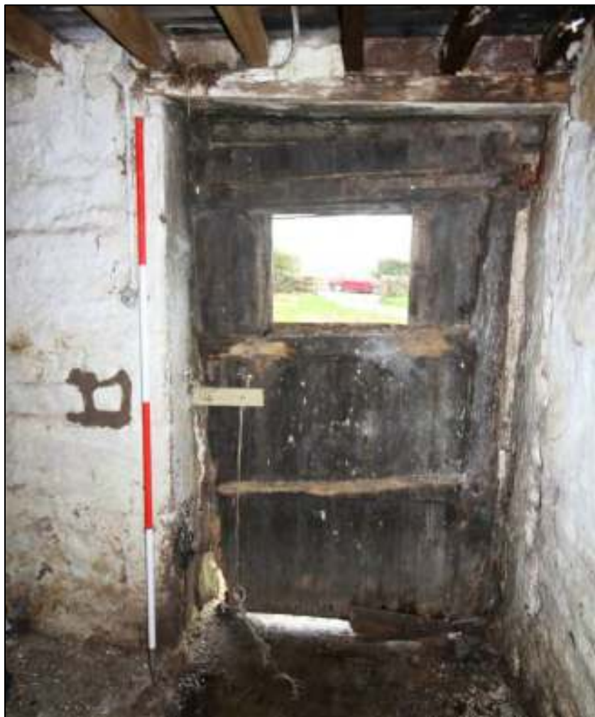
Gleaves Hill Barn 162: Wide doorway in east wall into northern cowhouse
