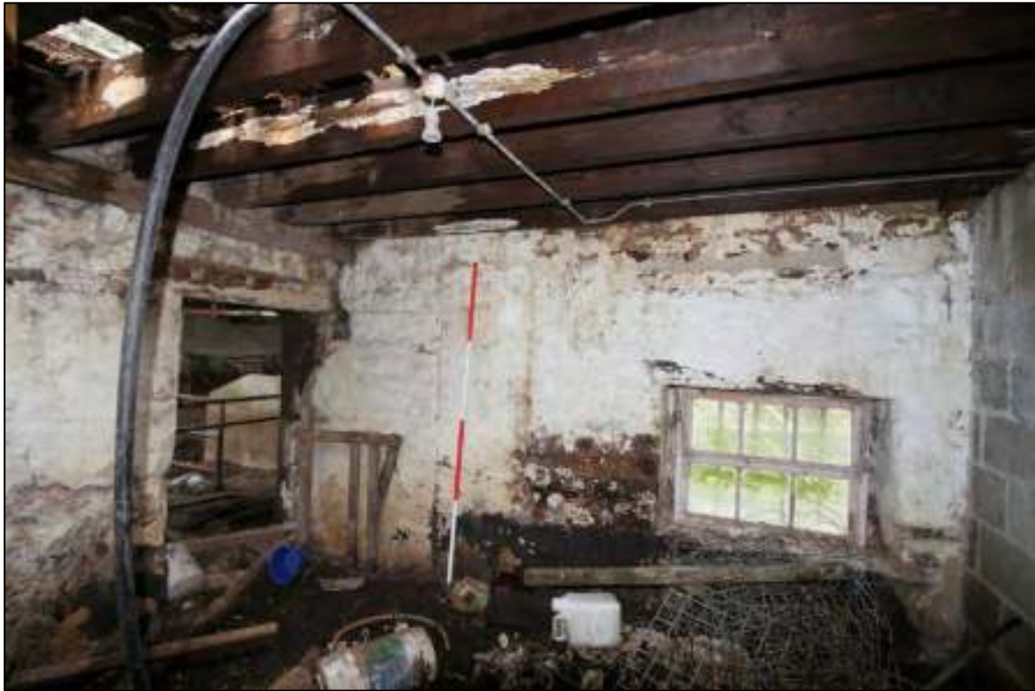
Gleaves Hill Barn 64: West bay of original southern cowhouse, looking west
