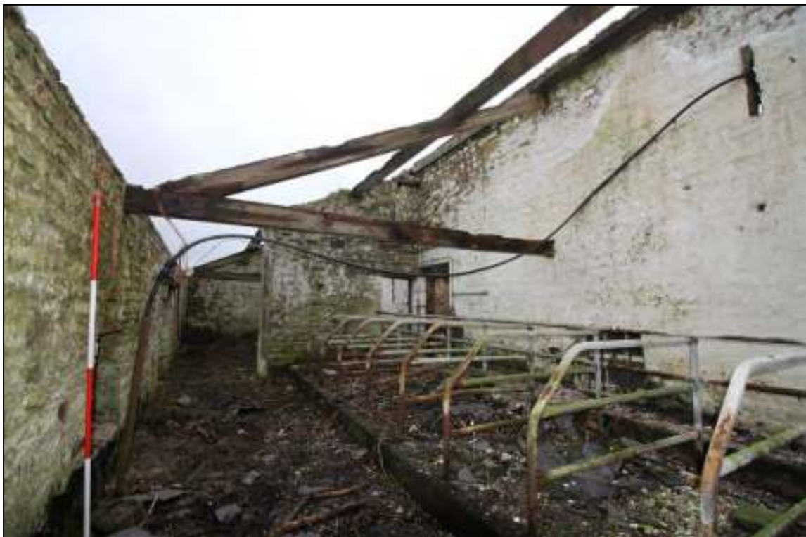
Gleaves Hill Barn 116: Single-storey cowhouse extension, looking north-east
