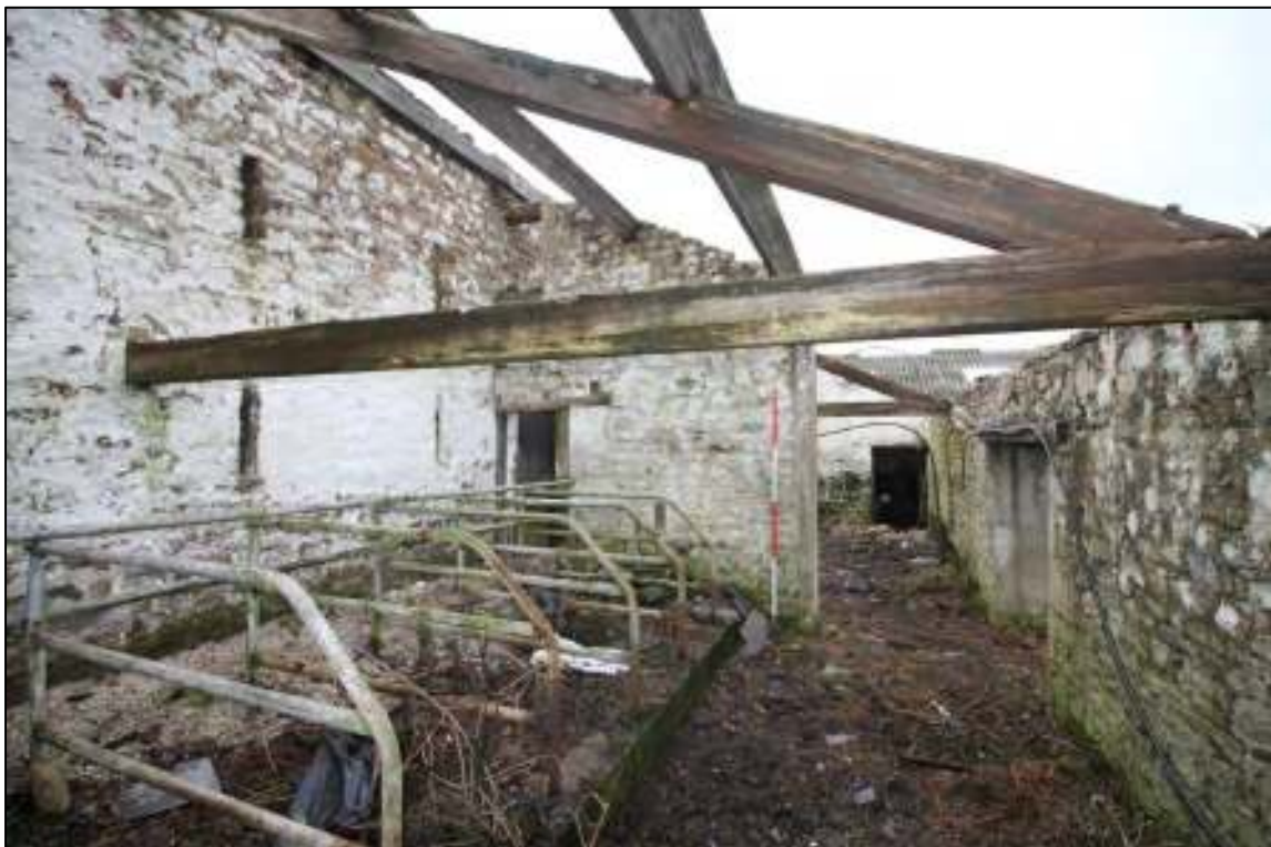
Gleaves Hill Barn 112: Single-storey cowhouse extension, looking south
