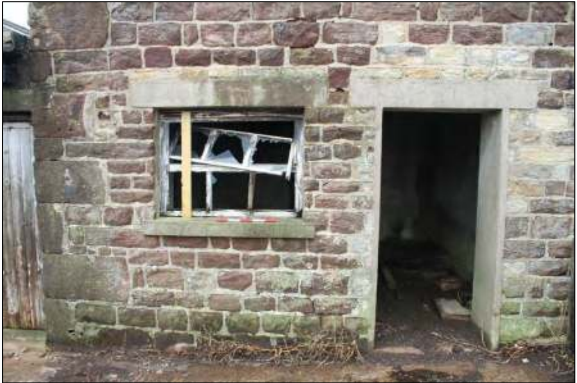
Gleaves Hill Barn 07: Detail of entrance into stables in southern bay
