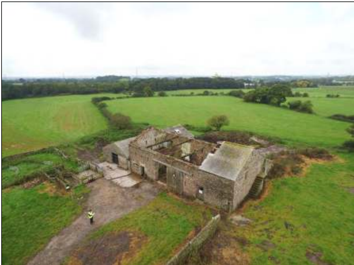
Gleaves Hill Barn UAV 15: Landscape view of the complex from the east
