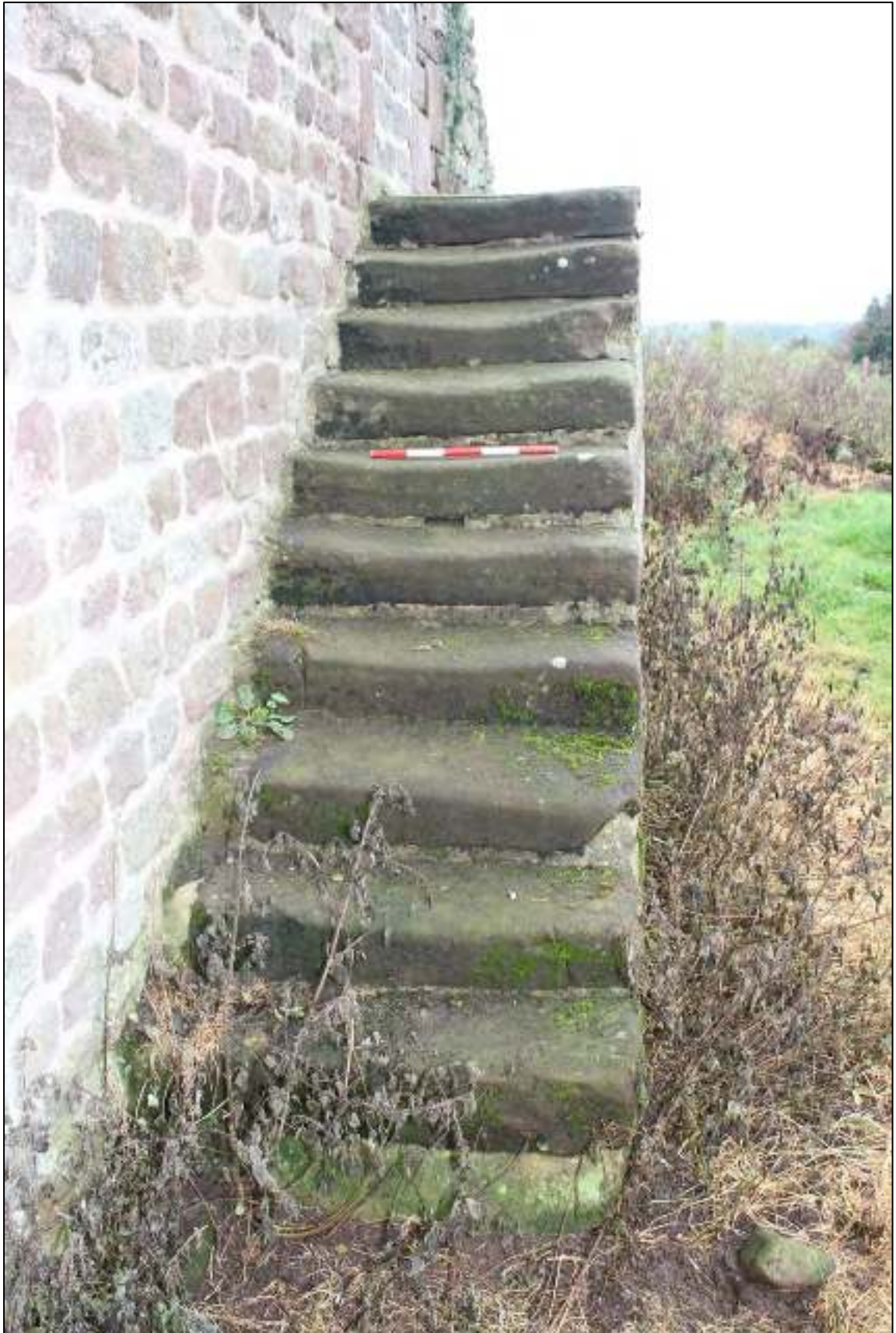
Gleaves Hill Barn 26: Detail of external stone stair, north gable
