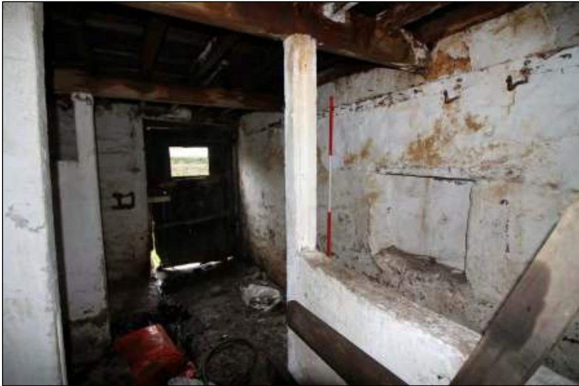
Gleaves Hill Barn 159: Stone dividing wall between cowhouse and threshing barn
