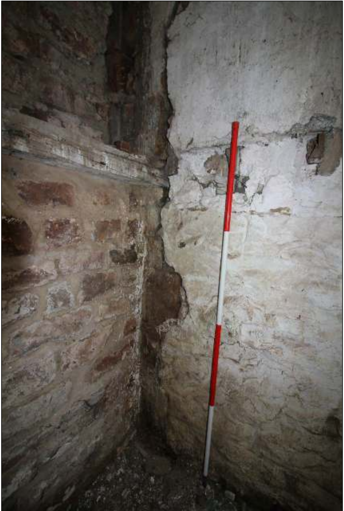
Gleaves Hill Barn 139: Quoin door jambs of doors in north passage
