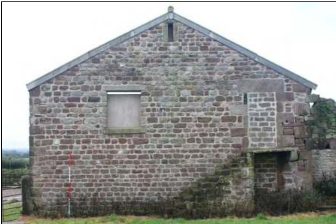
Gleaves Hill Barn 17: Detail of original north gable
