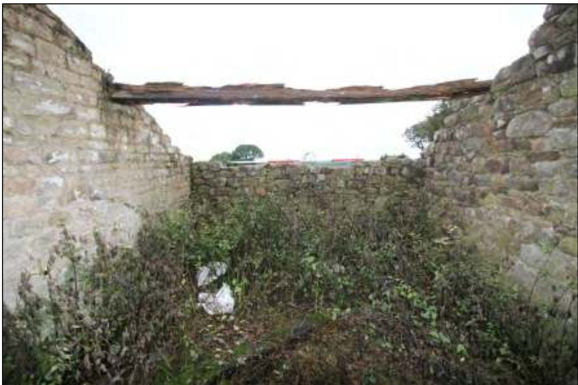
Gleaves Hill Barn 168: Loose box in single-storey extension, looking west
