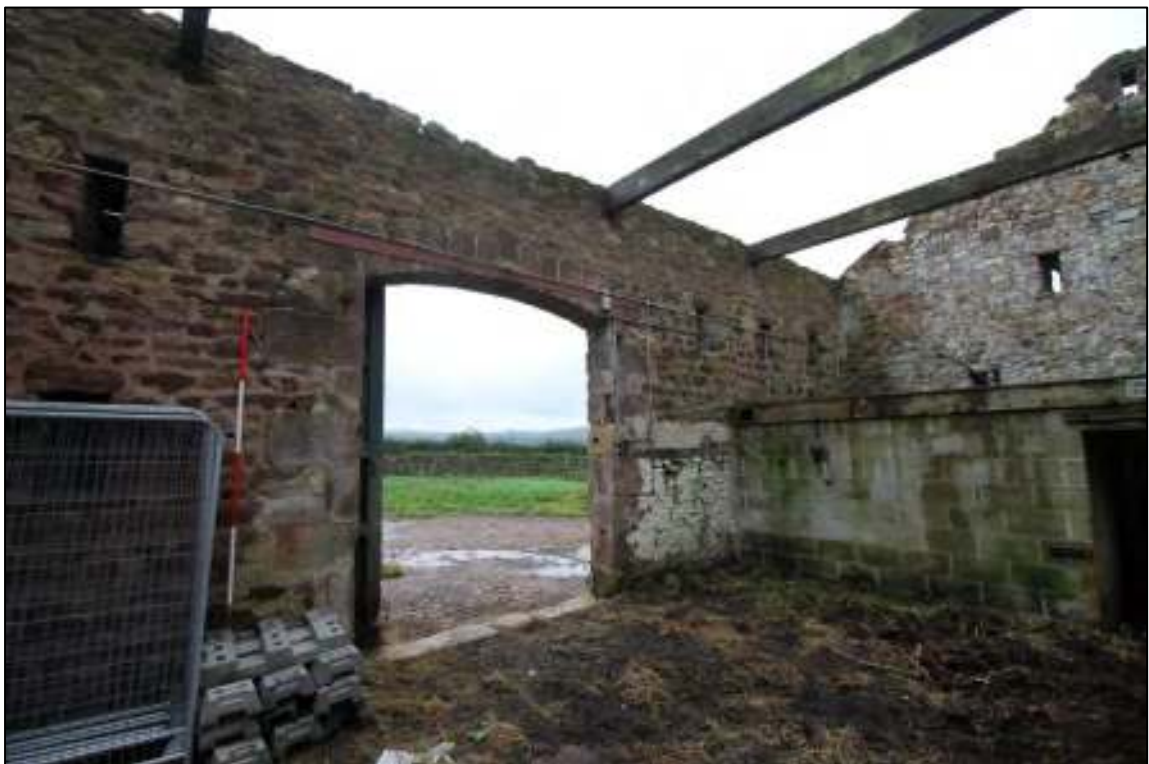
Gleaves Hill Barn 106: Front, eastern wall of threshing barn
