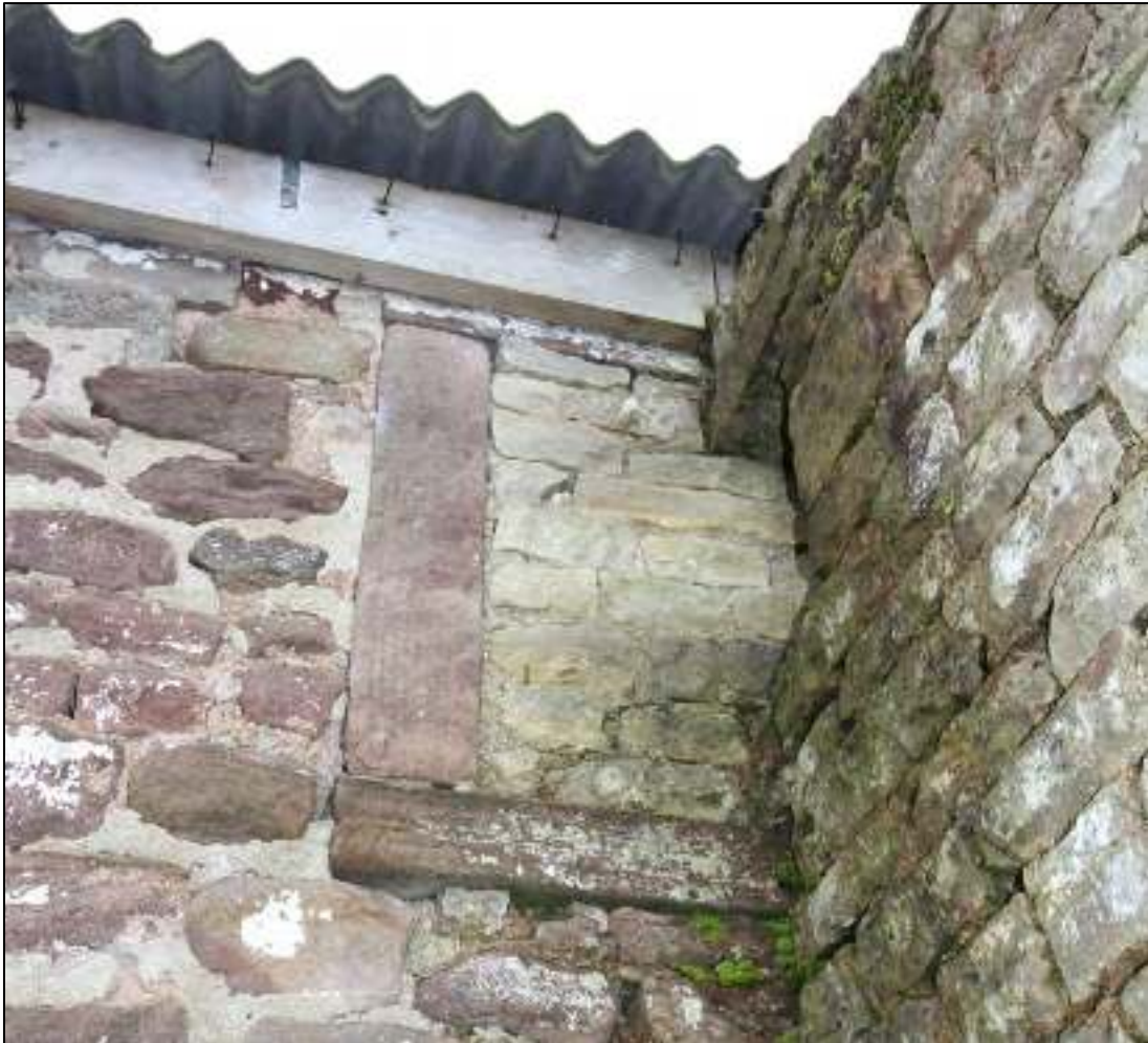
Gleaves Hill Barn 173: Cross wall within western extension blocking original window
