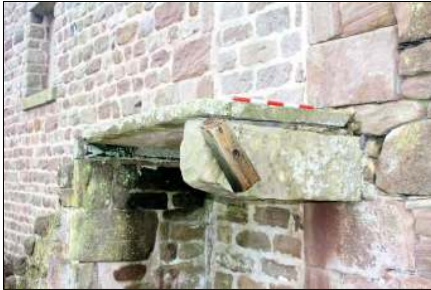
Gleaves Hill Barn 23: Detail of stone pad supporting landing
