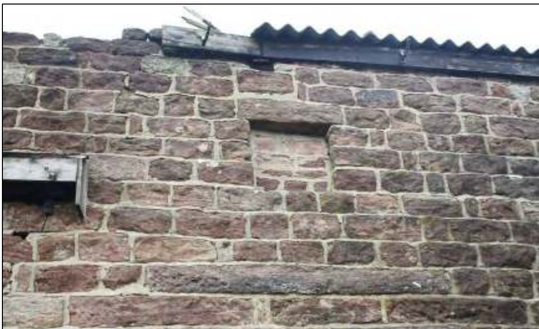
Gleaves Hill Barn 15: Detail of small blocked aperture above doorway
