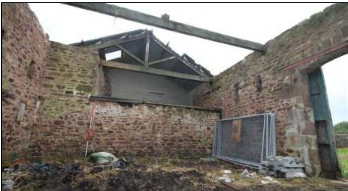
Gleaves Hill Barn 100: Interior of threshing barn, looking north-east
