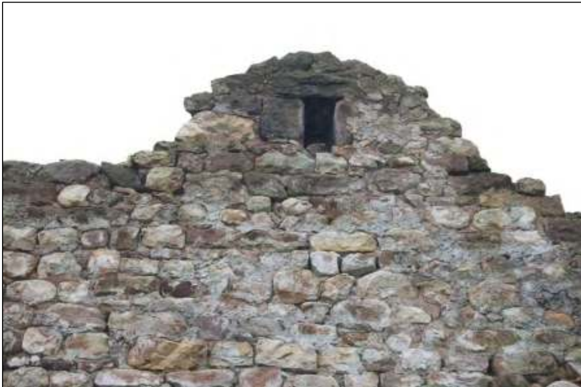
Gleaves Hill Barn 80: Owl hole in loft of southern gable
