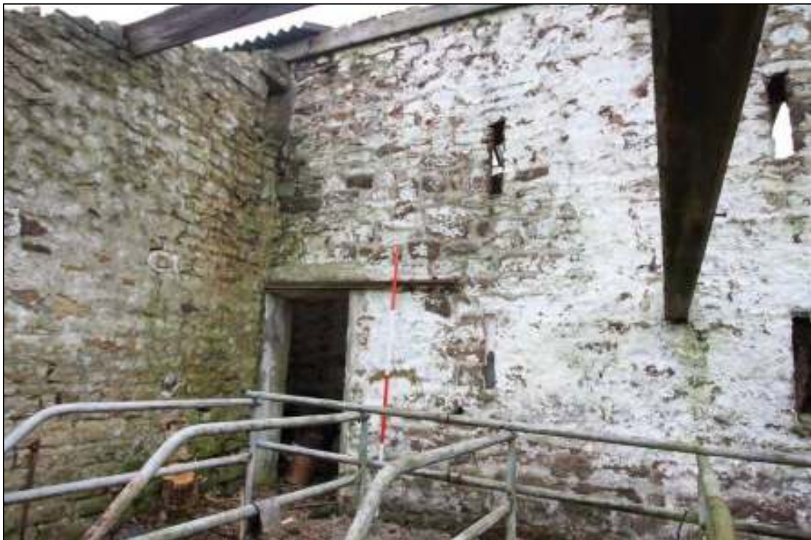
Gleaves Hill Barn 130: Doorway in west wall of original barn
