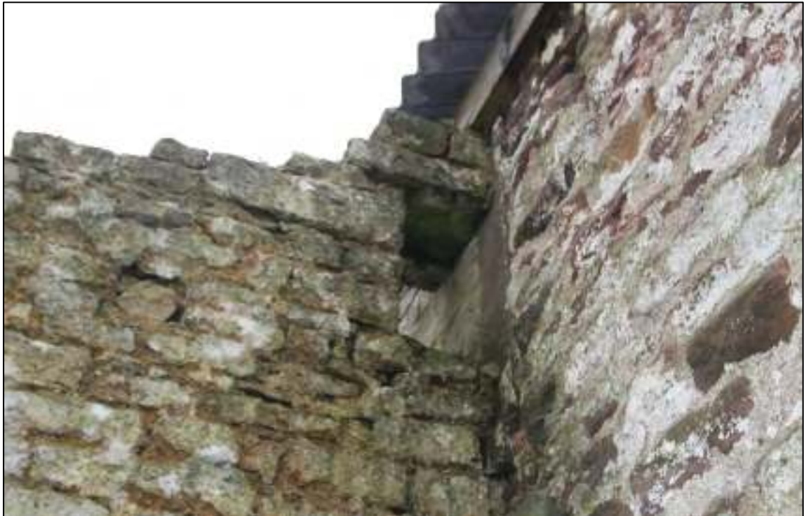
Gleaves Hill Barn 127: Owl hole in north gable of single-storey outshut
