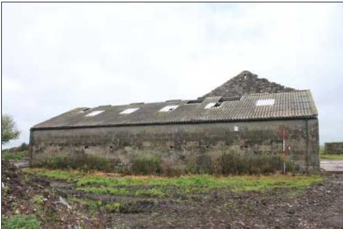
Gleaves Hill Barn 34: South elevation of south extension
