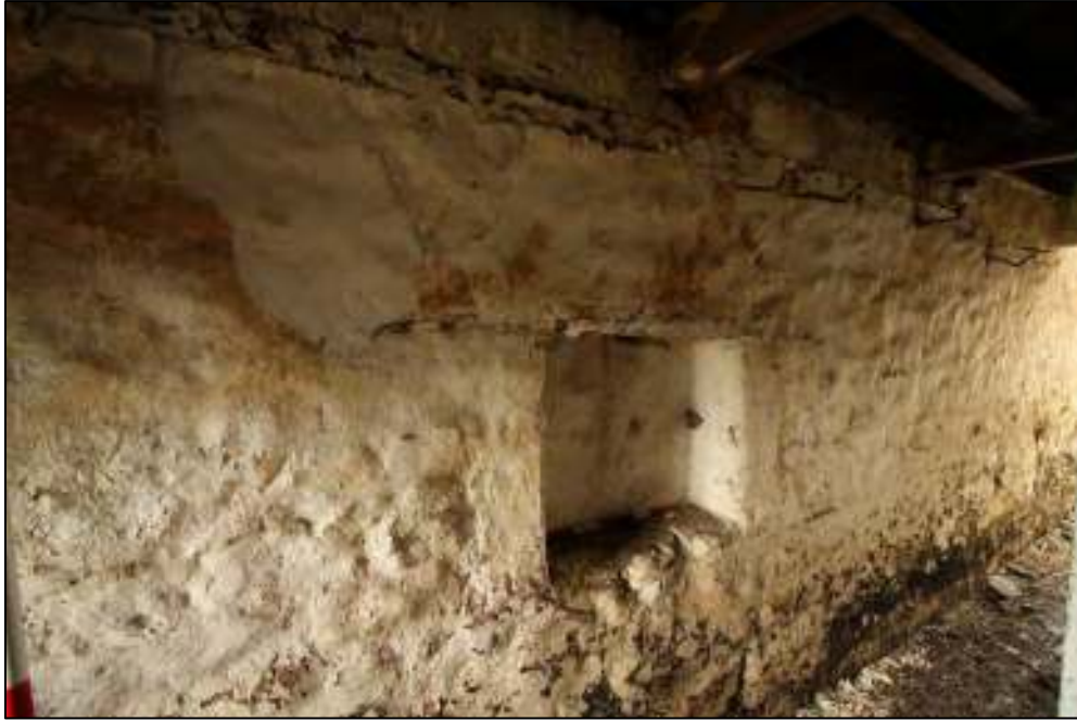
Gleaves Hill Barn 161: Keeping hole in dividing wall
