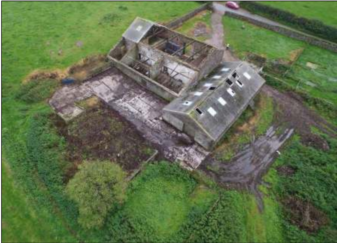
Gleaves Hill Barn UAV 06: General view of the complex from the west
