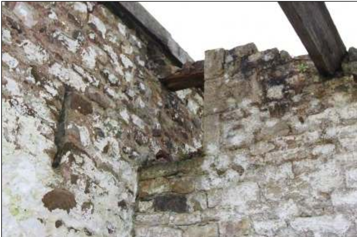
Gleaves Hill Barn 122: Quoined aperture in dividing wall within single-storey outshut,
