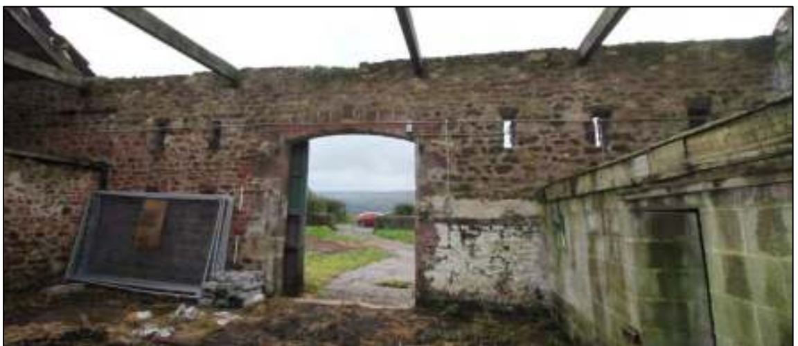
Gleaves Hill Barn 102: Front, eastern wall of threshing barn
