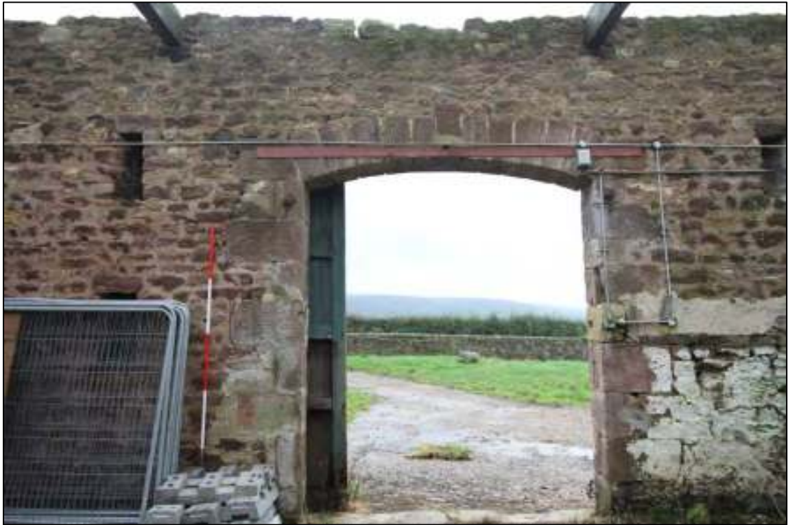
Gleaves Hill Barn 105: Threshing door in east wall
