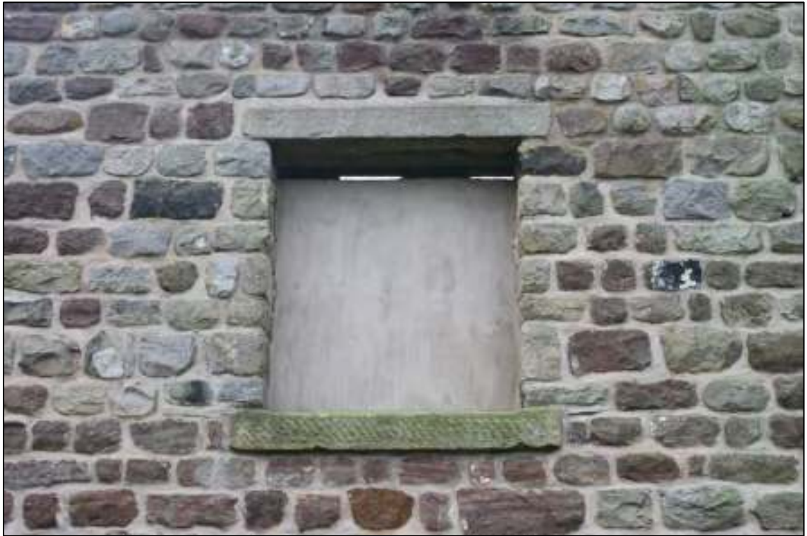
Gleaves Hill Barn 18: Window/pitching eye into north loft of barn
