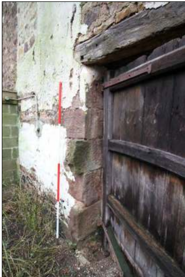
Gleaves Hill Barn 86: Detail of southern jamb of winnowing door
