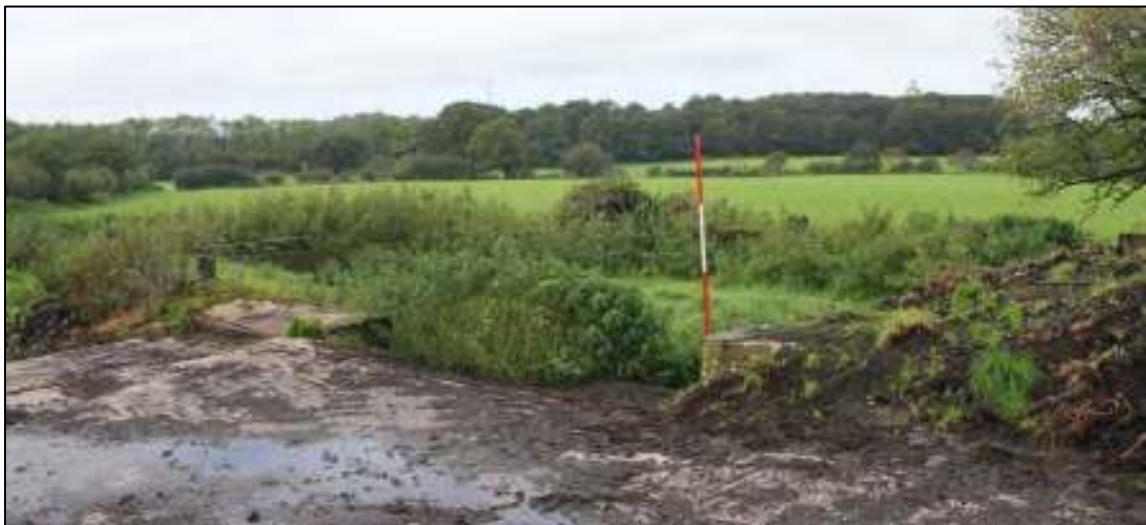
Gleaves Hill Barn 50: Concrete tank to south-west of barn
