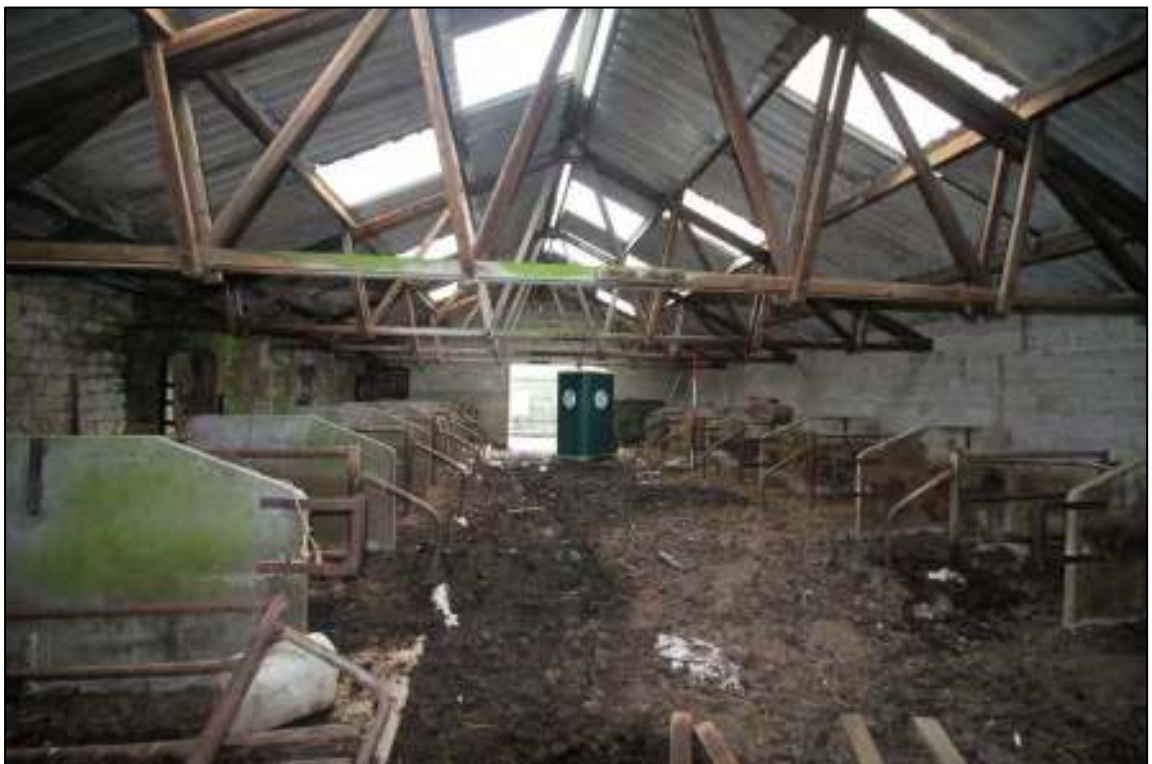
Gleaves Hill Barn 54: Mid/late-twentieth century cowhouse looking east
