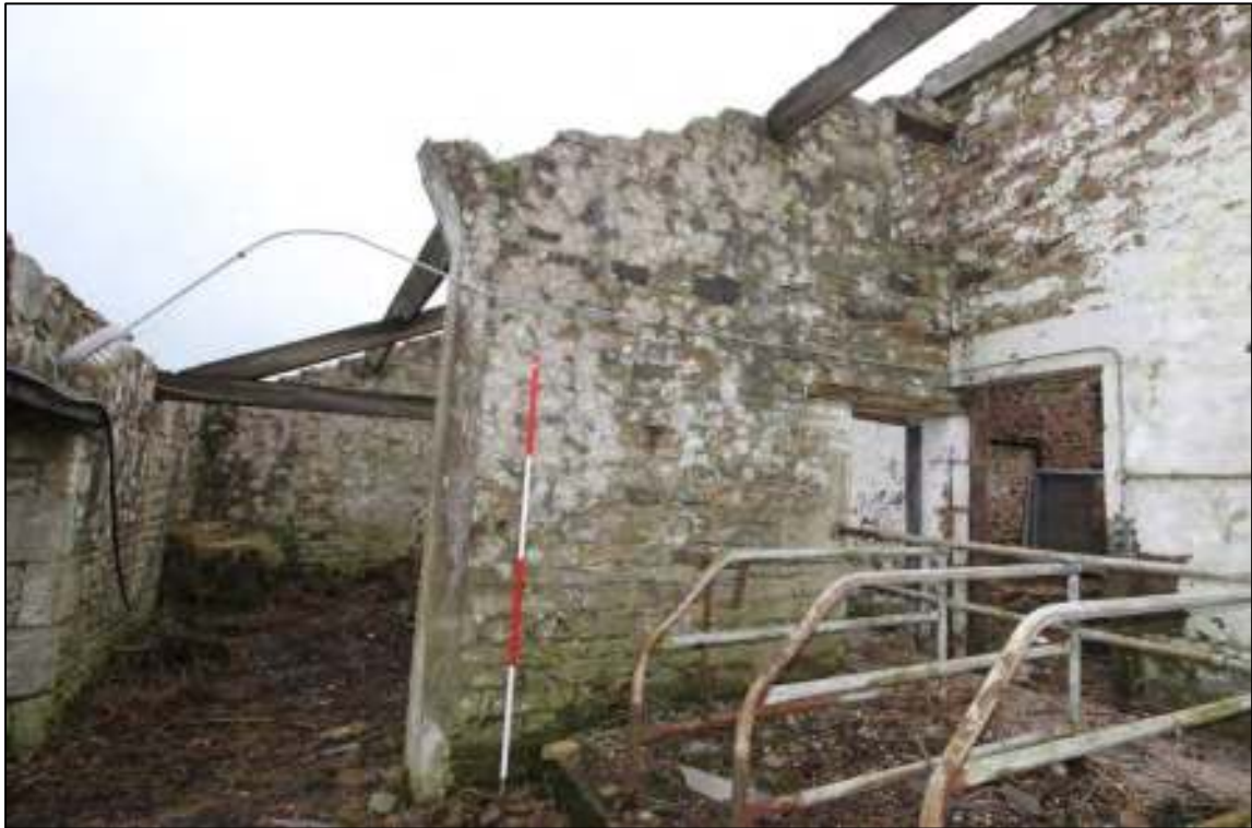
Gleaves Hill Barn 117: Single-storey cowhouse extension, looking north-east
