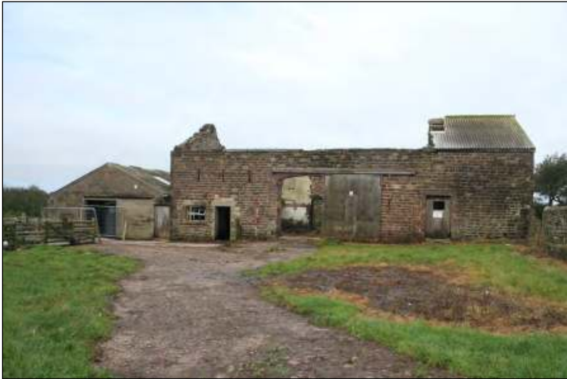
Gleaves Hill Barn 03: Eastern front façade of extant complex
