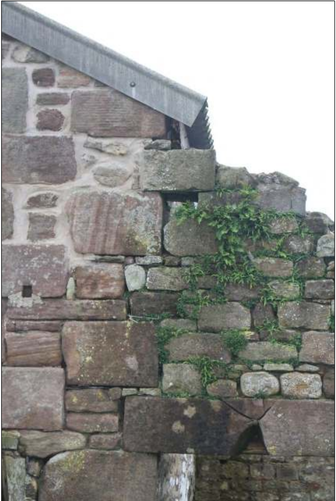
Gleaves Hill Barn 29: Detail of rough keying of extension, north gable
