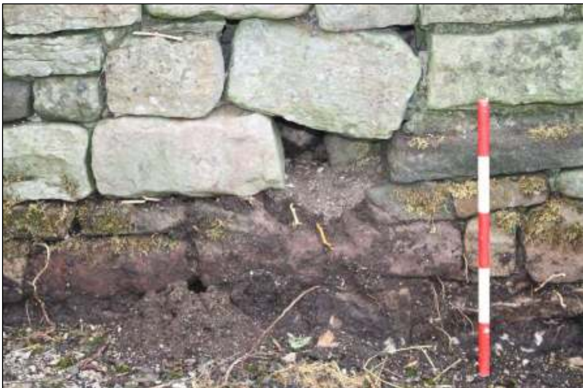
Gleaves Hill Barn 46: Detail of drain aperture
