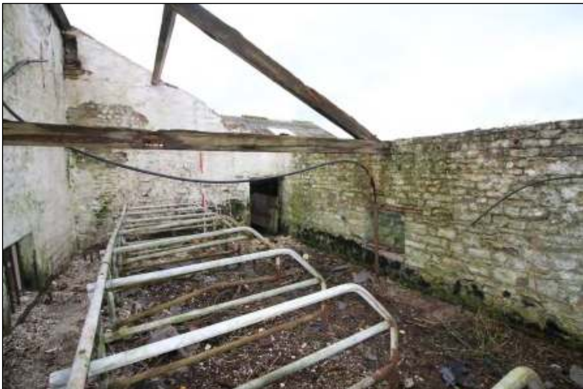
Gleaves Hill Barn 114: Single-storey cowhouse extension, looking south-west
