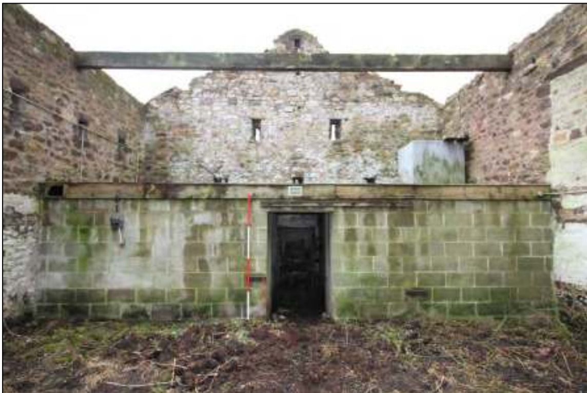
Gleaves Hill Barn 78: Inserted clinker-block wall to southern cowhouse, almost certainly replacing a timber partition
