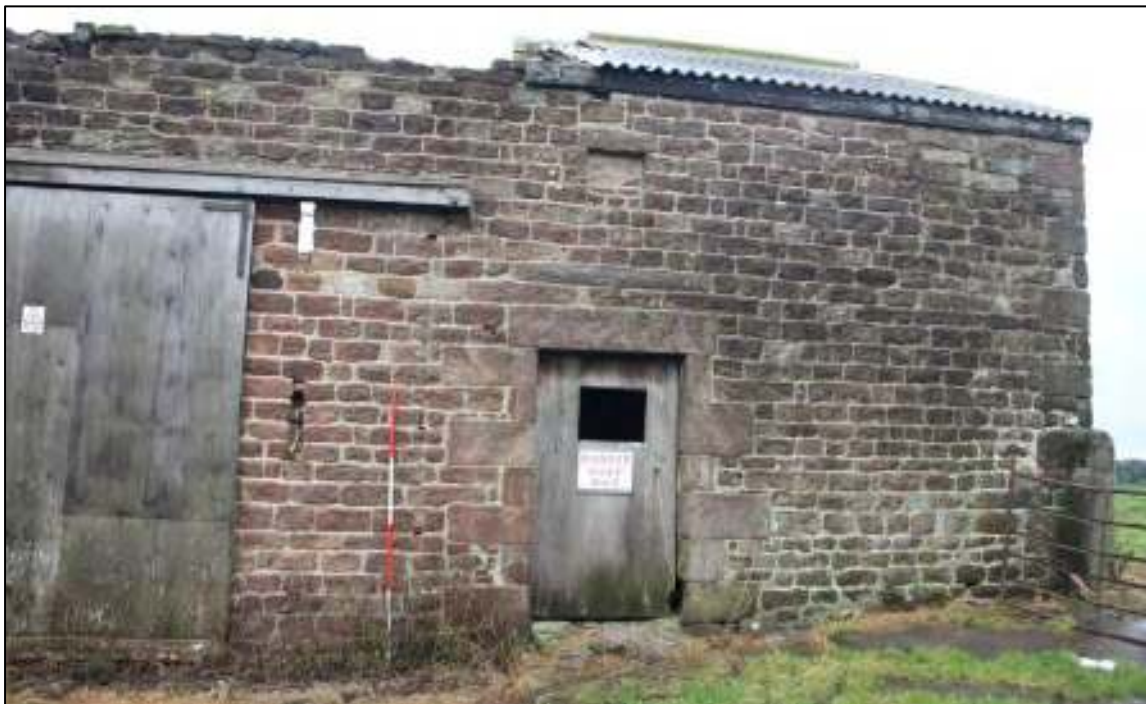
Gleaves Hill Barn 13: Northern bay of original barn
