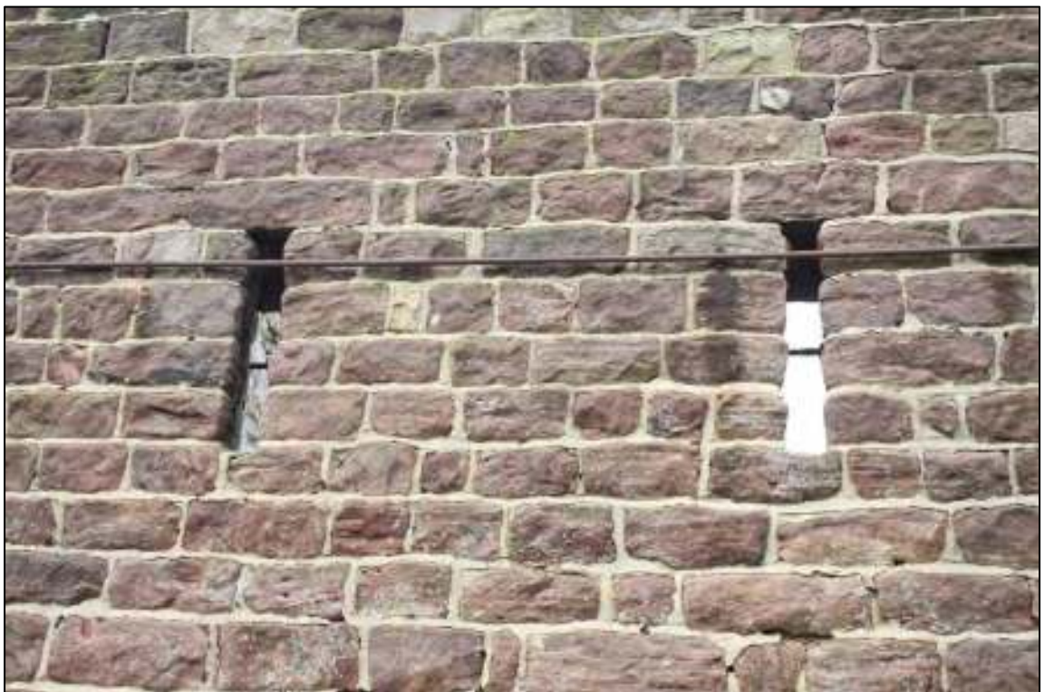
Gleaves Hill Barn 06: Detail of ventilators in hayloft
