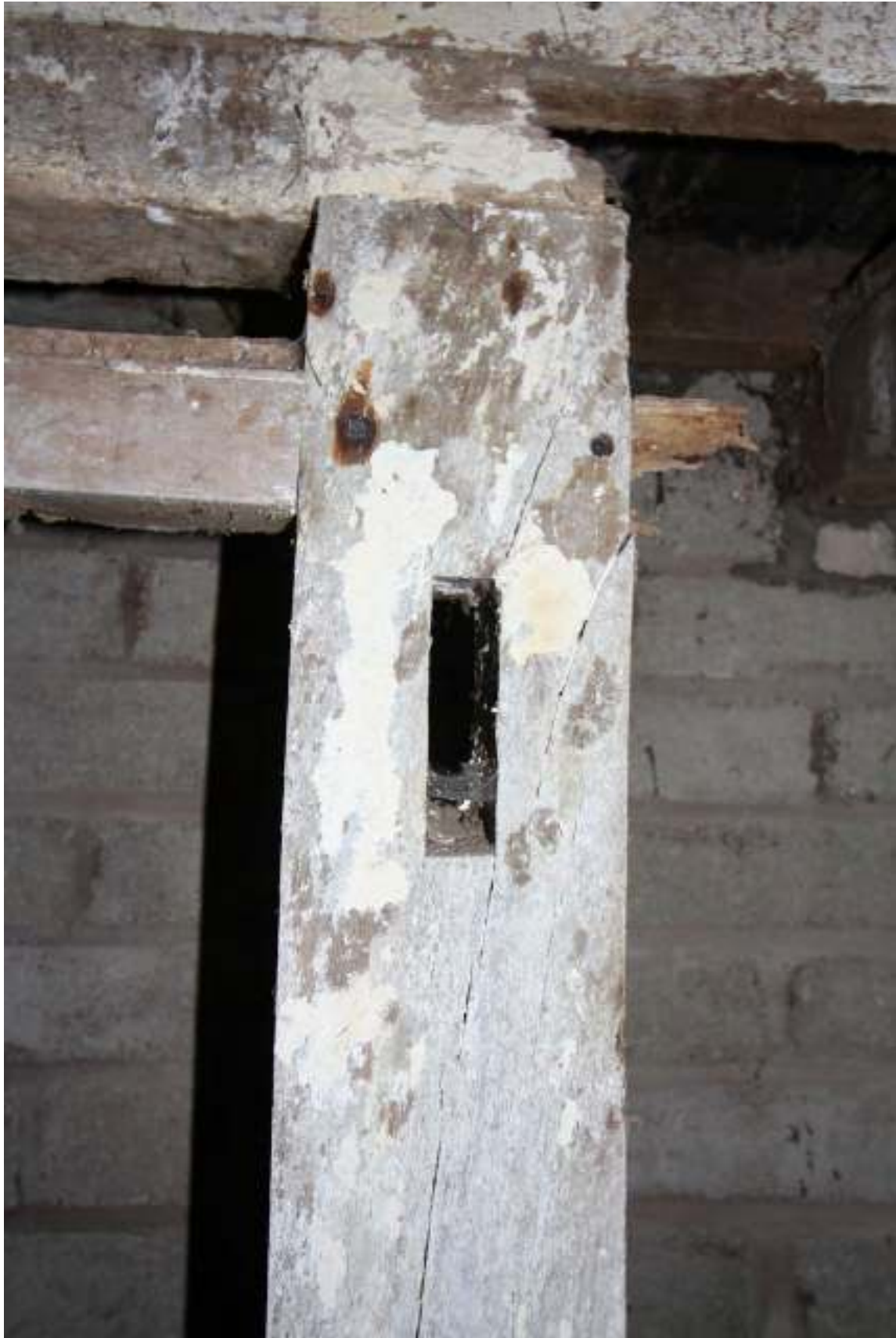
Gleaves Hill Barn 156: Detail of mortise in hay feeder
