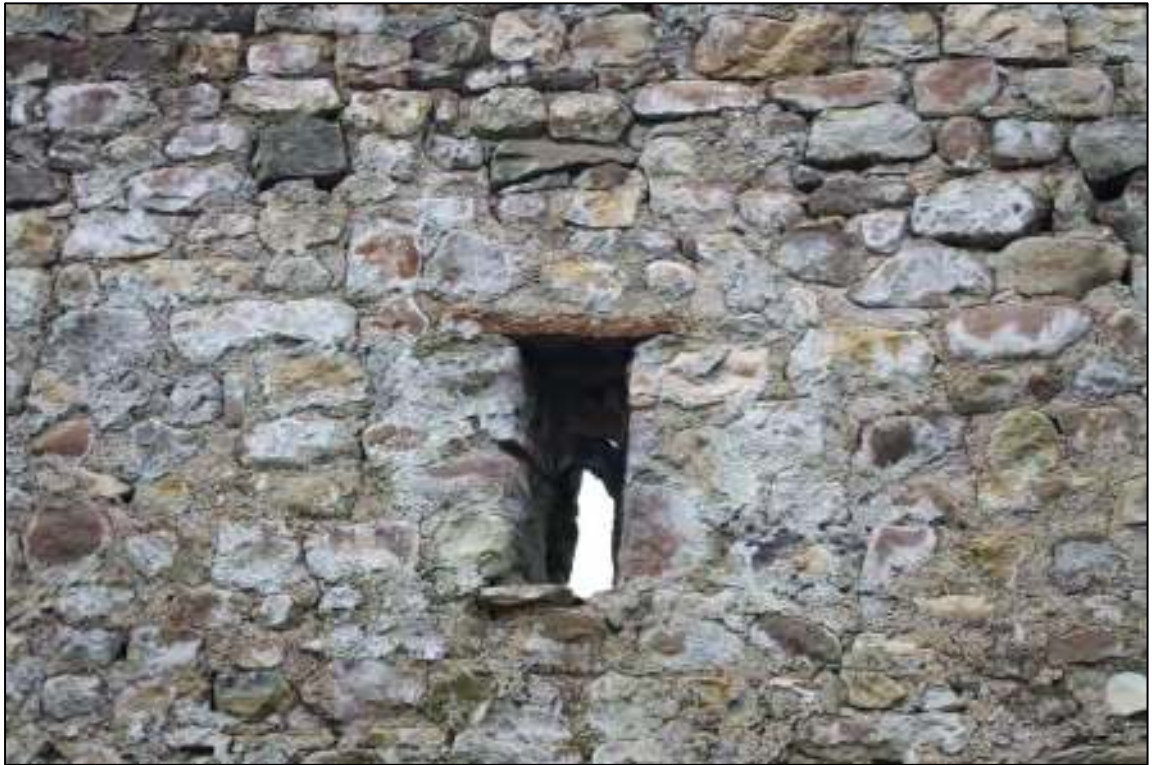
Gleaves Hill Barn 81: Detail of ventilator in loft of southern gable
