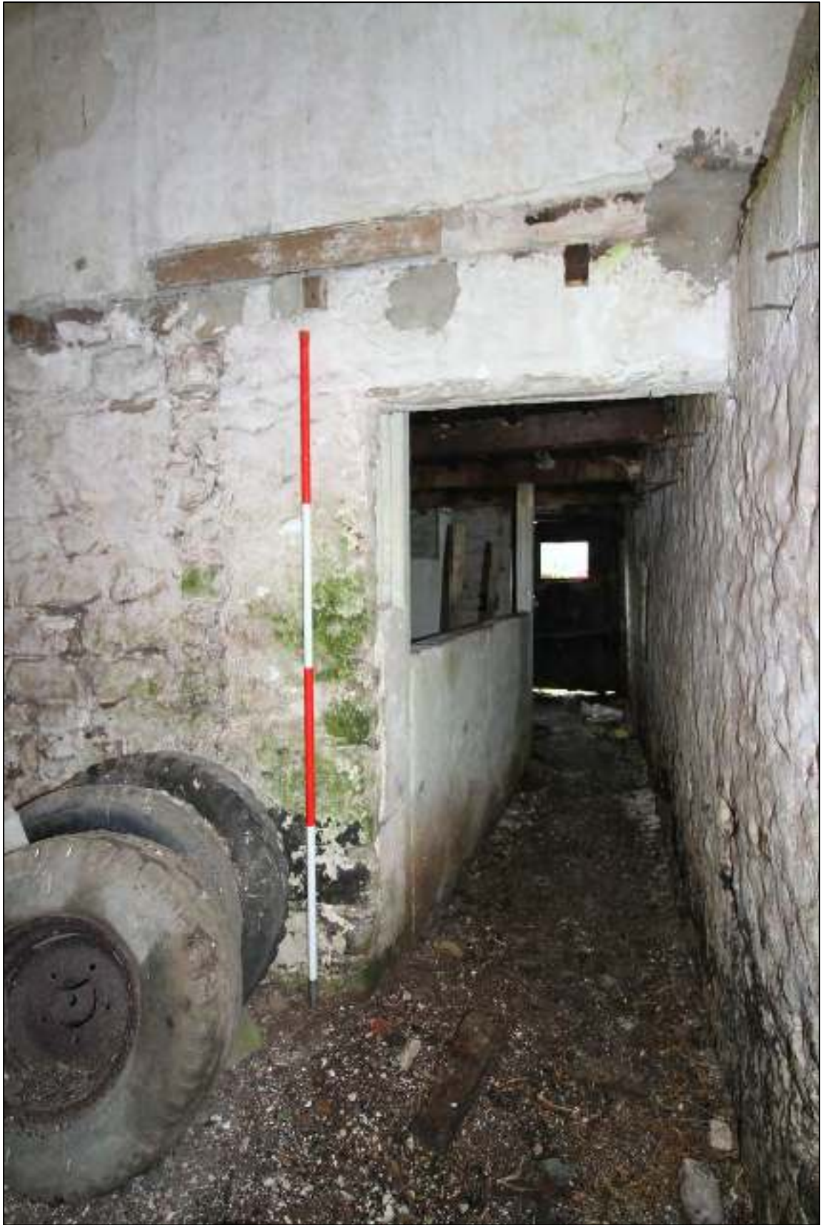
Gleaves Hill Barn 135: Passage within northern stables
