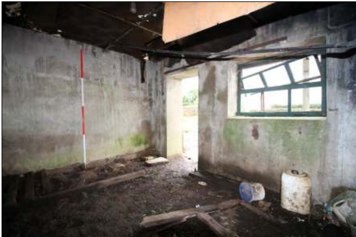
Gleaves Hill Barn 75: Rendered bay in southern cowhouse, looking east
