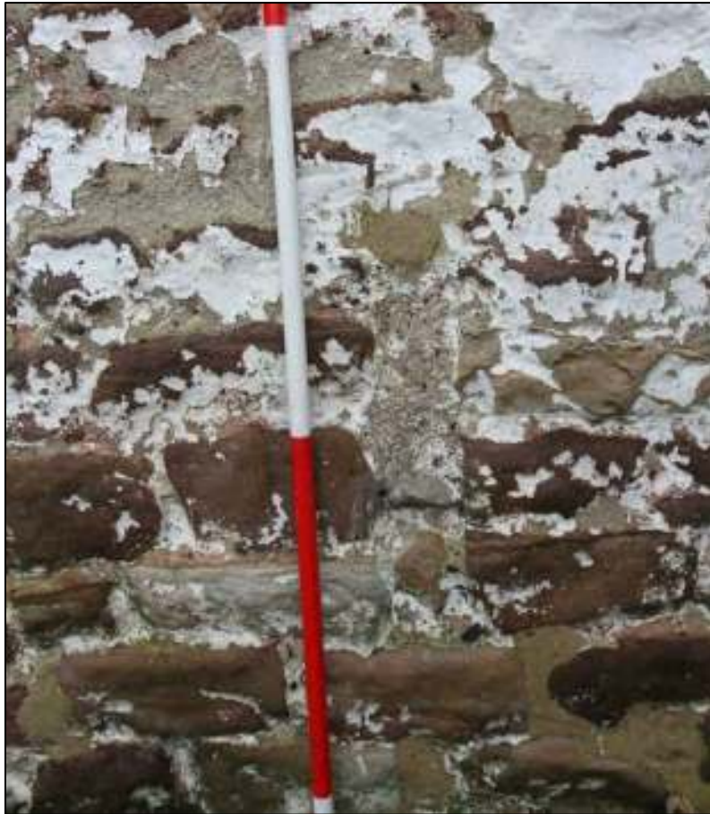
Gleaves Hill Barn 171: Blocked ventilator in original west wall
