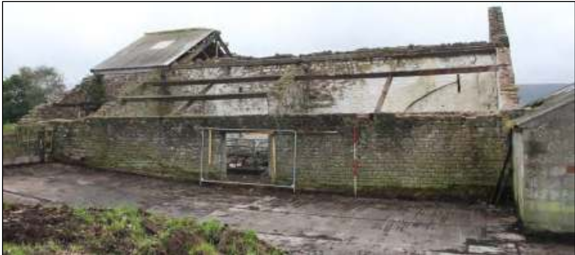
Gleaves Hill Barn 37: West single-storey extension from the rear
