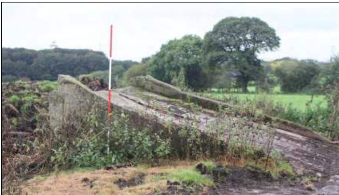
Gleaves Hill Barn 48: Concrete ramp to north-west of barn
