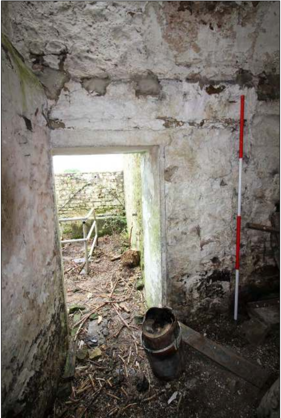
Gleaves Hill Barn 141: Door in west wall of original barn
