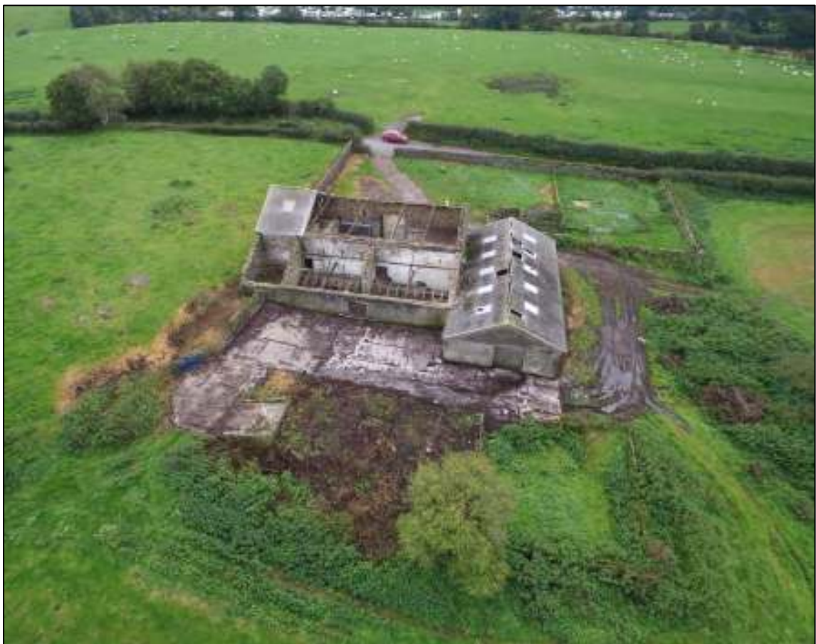
Gleaves Hill Barn UAV 07: General view of the complex from the north-west
