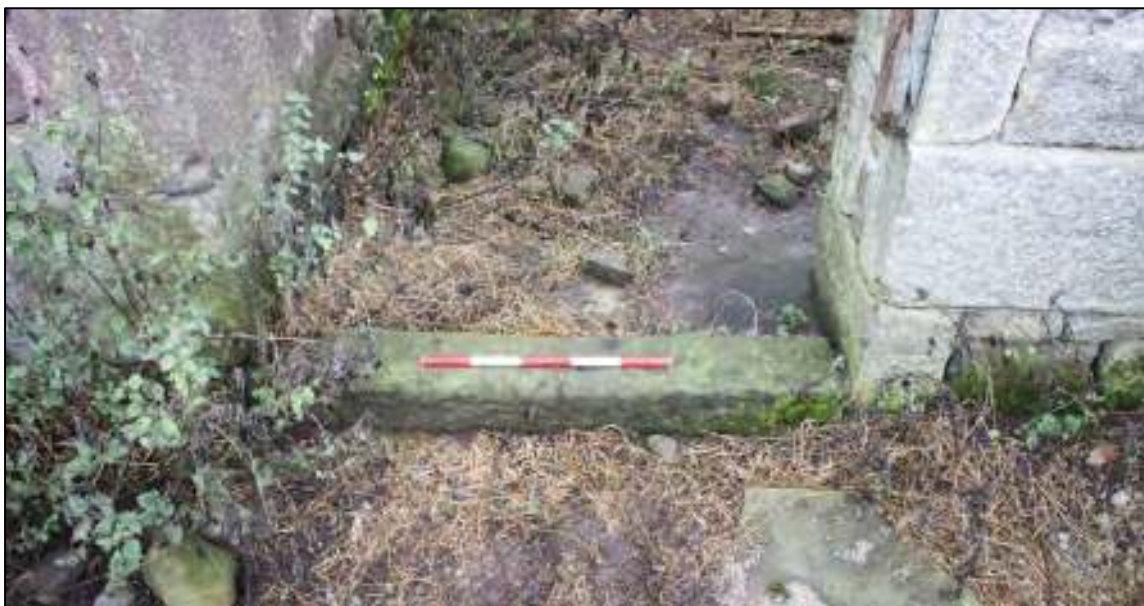
Gleaves Hill Barn 32: Threshold step into north extension
