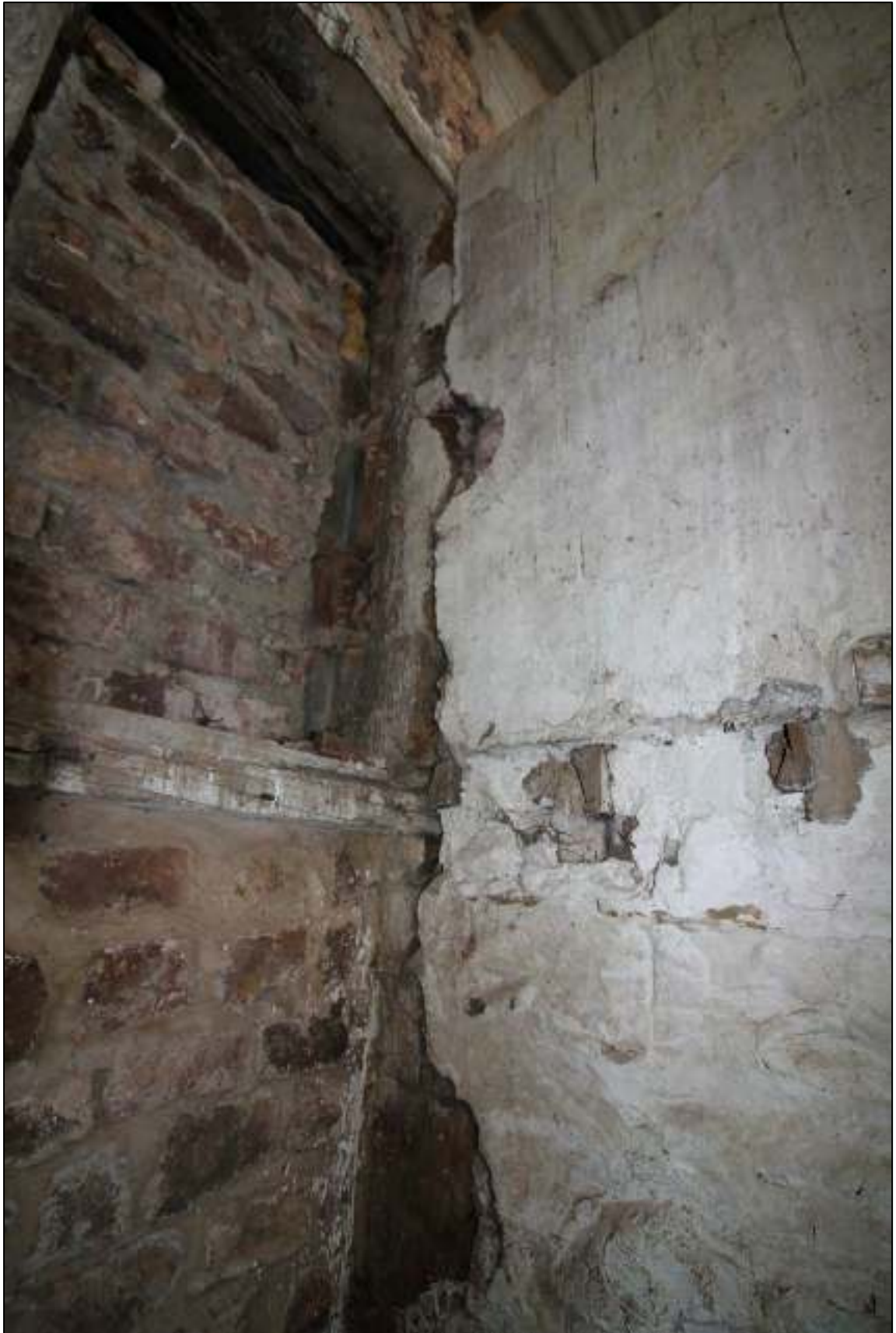
Gleaves Hill Barn 140: Quoin door jambs of doors in north passage
