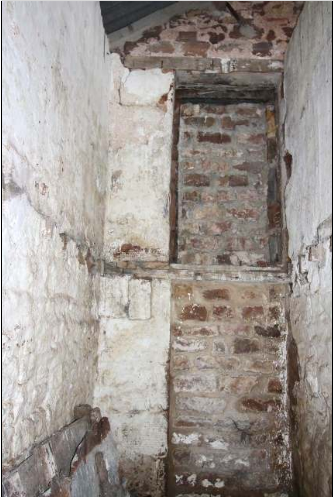
Gleaves Hill Barn 137: Doorways in north passage
