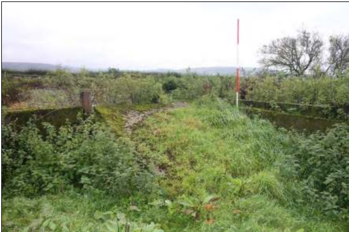
Gleaves Hill Barn 52: Concrete ramp within concrete tank to south-west of barn
