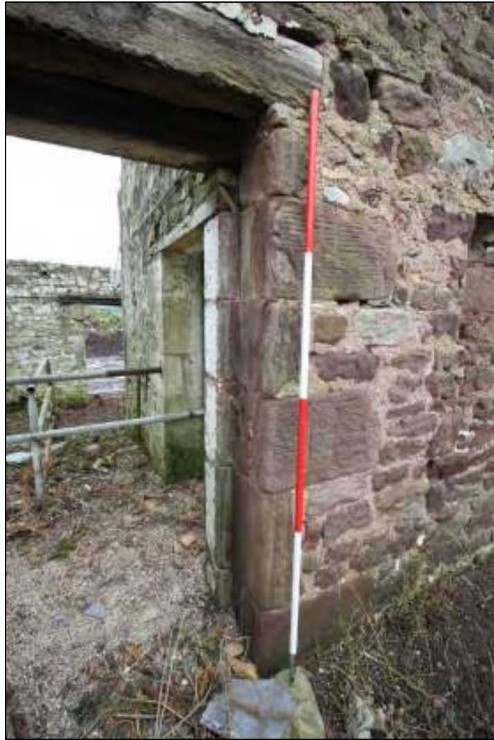
Gleaves Hill Barn 89: Detail of northern jamb of winnowing door
