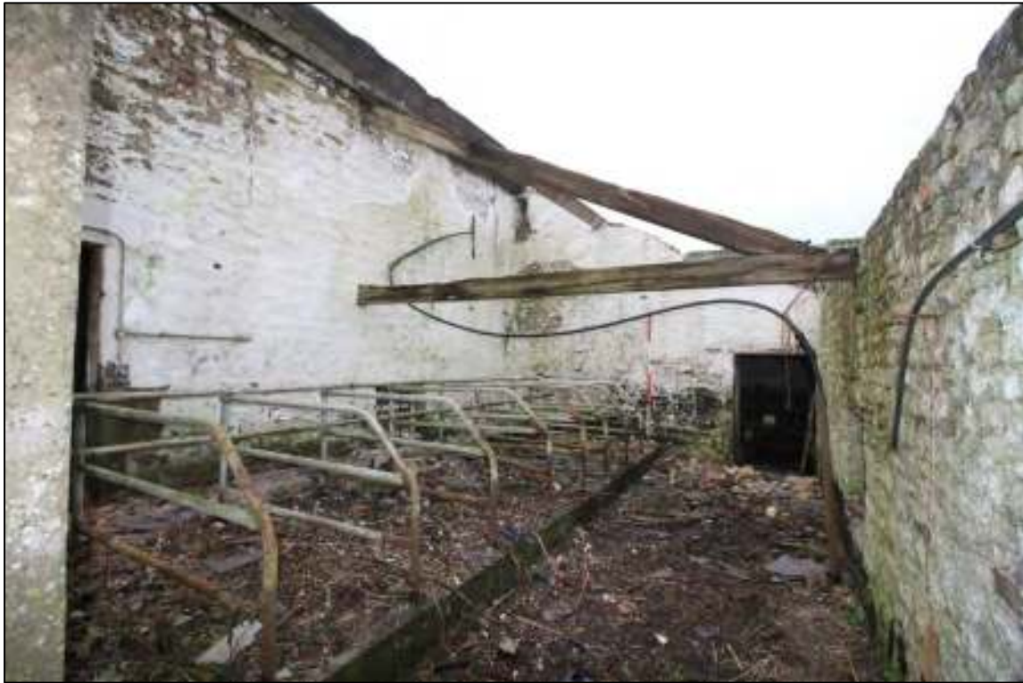
Gleaves Hill Barn 113: Single-storey cowhouse extension, looking south
