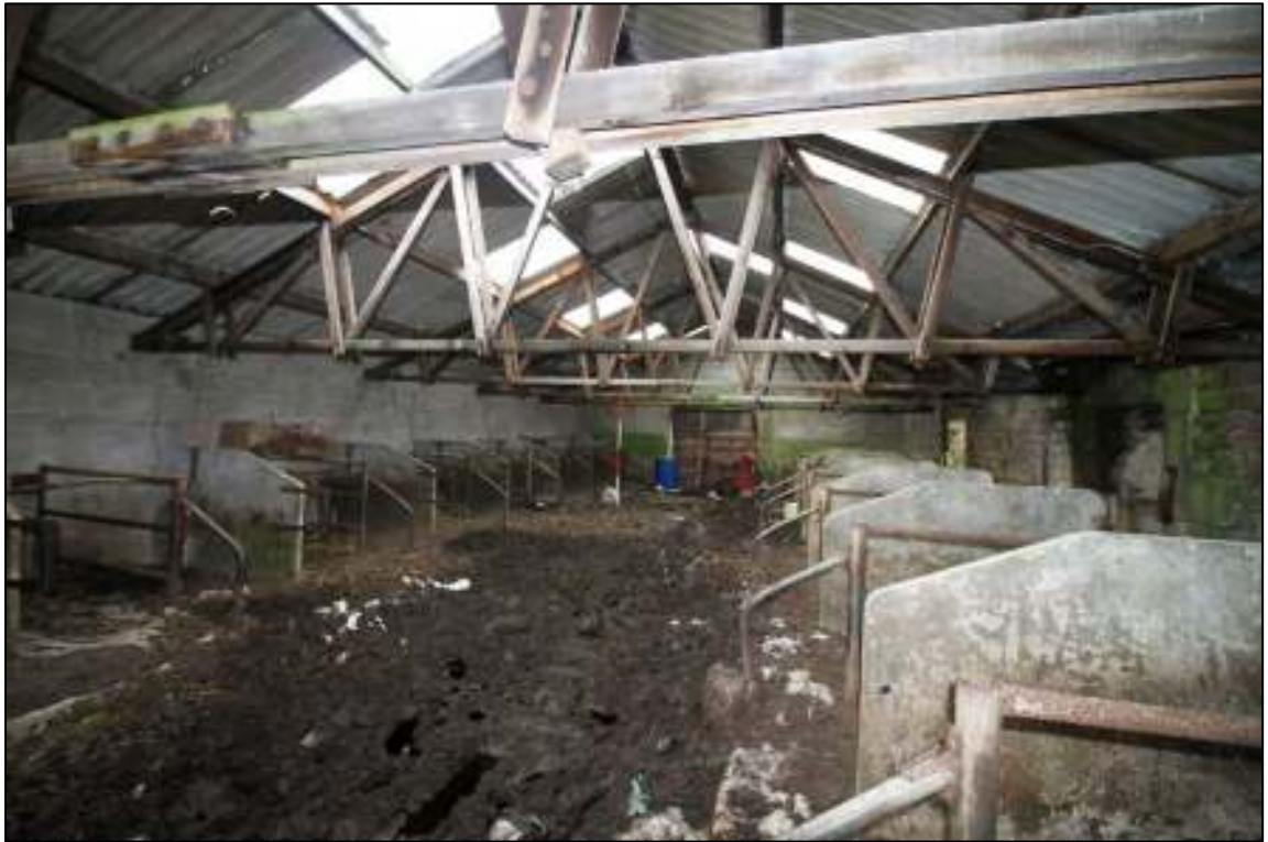
Gleaves Hill Barn 53: Mid/late-twentieth century cowhouse looking west
