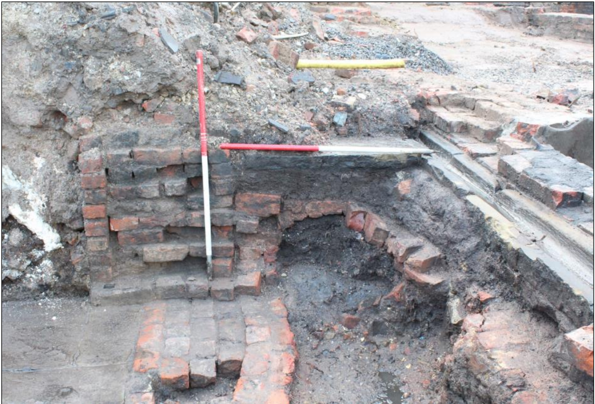
Plate 24: Detail of brick-vaulted flue 068 with wall 067, looking south-east. Scale 1m
