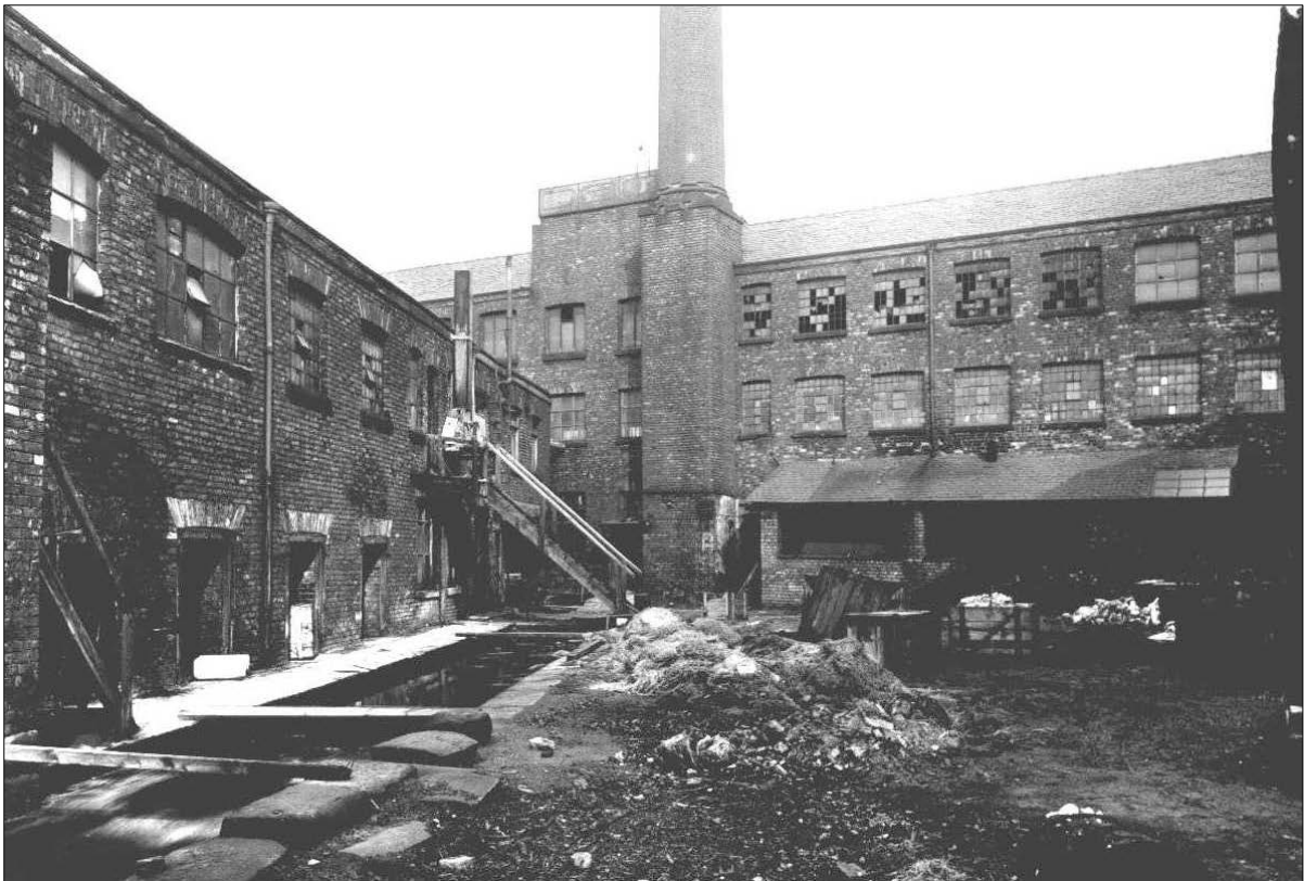
Plate 7: View of the glassworks shortly before demolition
