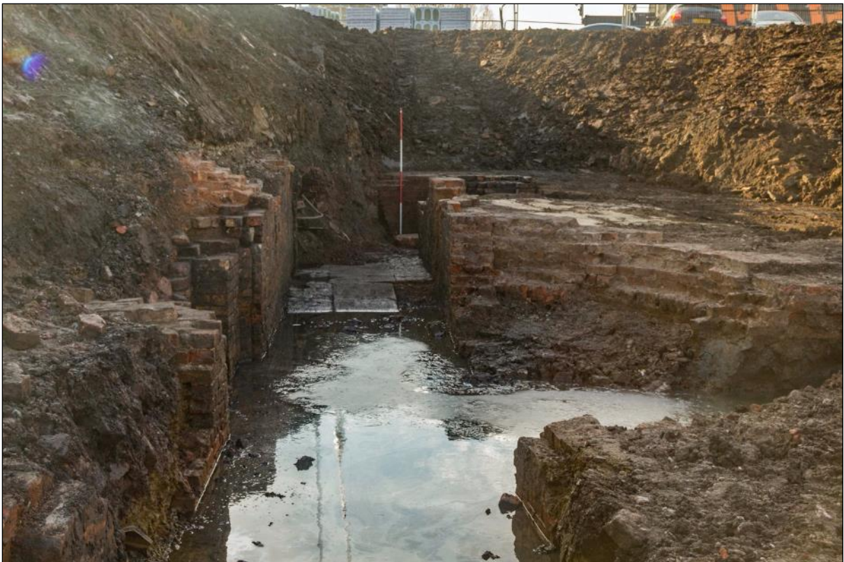
Plate 16: Furnace wall 006 (right) and the central flue, looking south-west. Scale 2m
