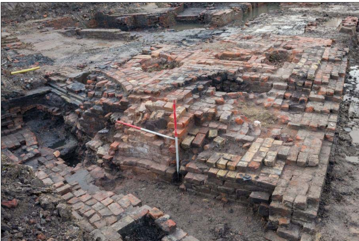
Plate 23: The remains of the annealing house, showing refractory brick wall 051, chimney and associated flue, looking south-west. Scale 1m
