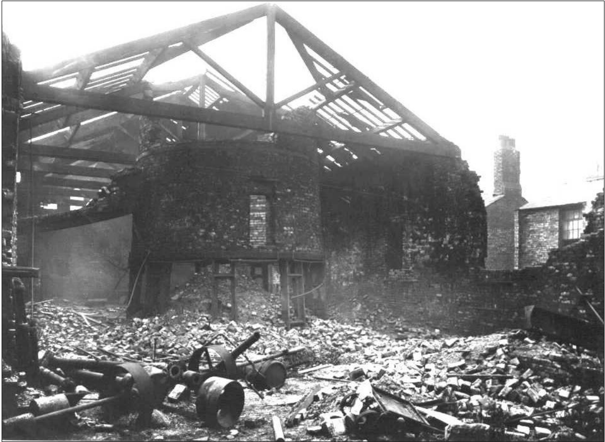
Plate 6: View of a glass-melting furnace during demolition
