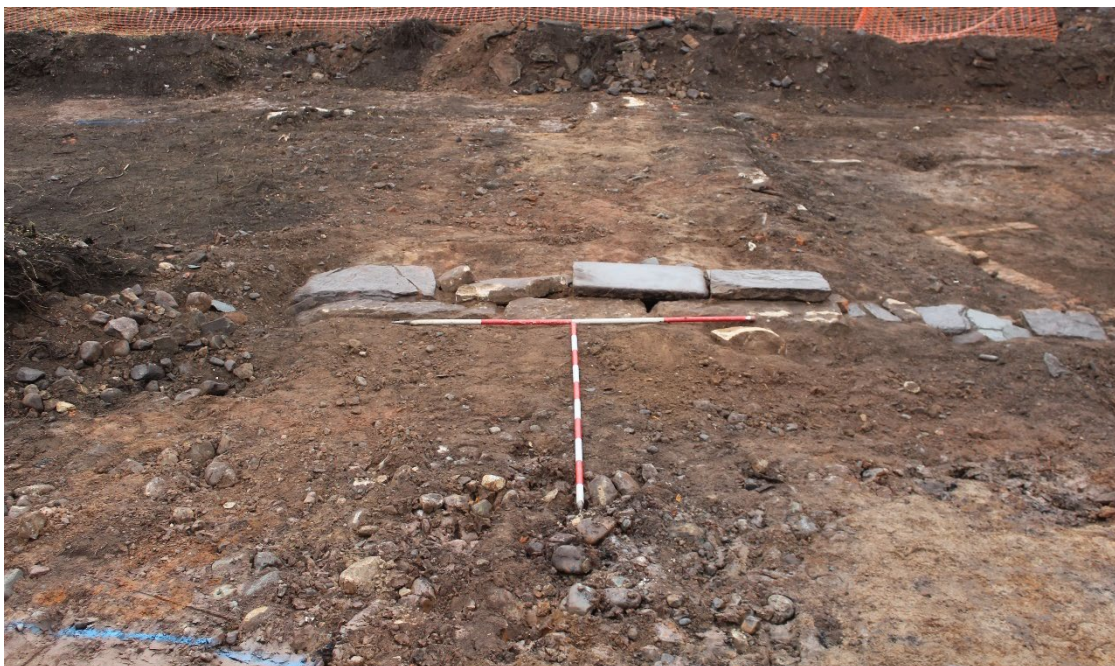
Plate 32: Area 1 looking east, a mid-excitation shot of the causeway after the removal of surface [133], bedding layer [137] and partial excavation of [172], scales: 2m horizontal; 2m vertical
