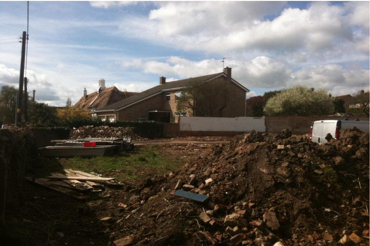
Plate 4: Site view looking south.
