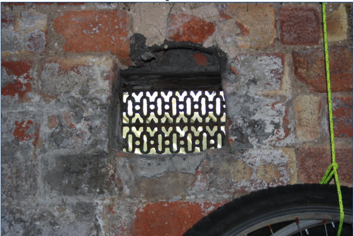
Plate 15: Air vent in Room 1 looking north.
