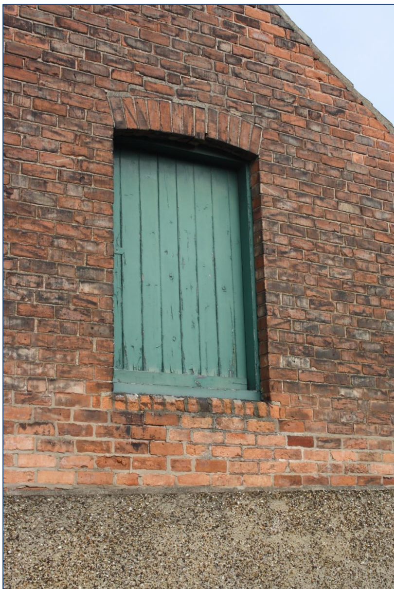
Plate 19: Pitch-hole south elevation looking north.
