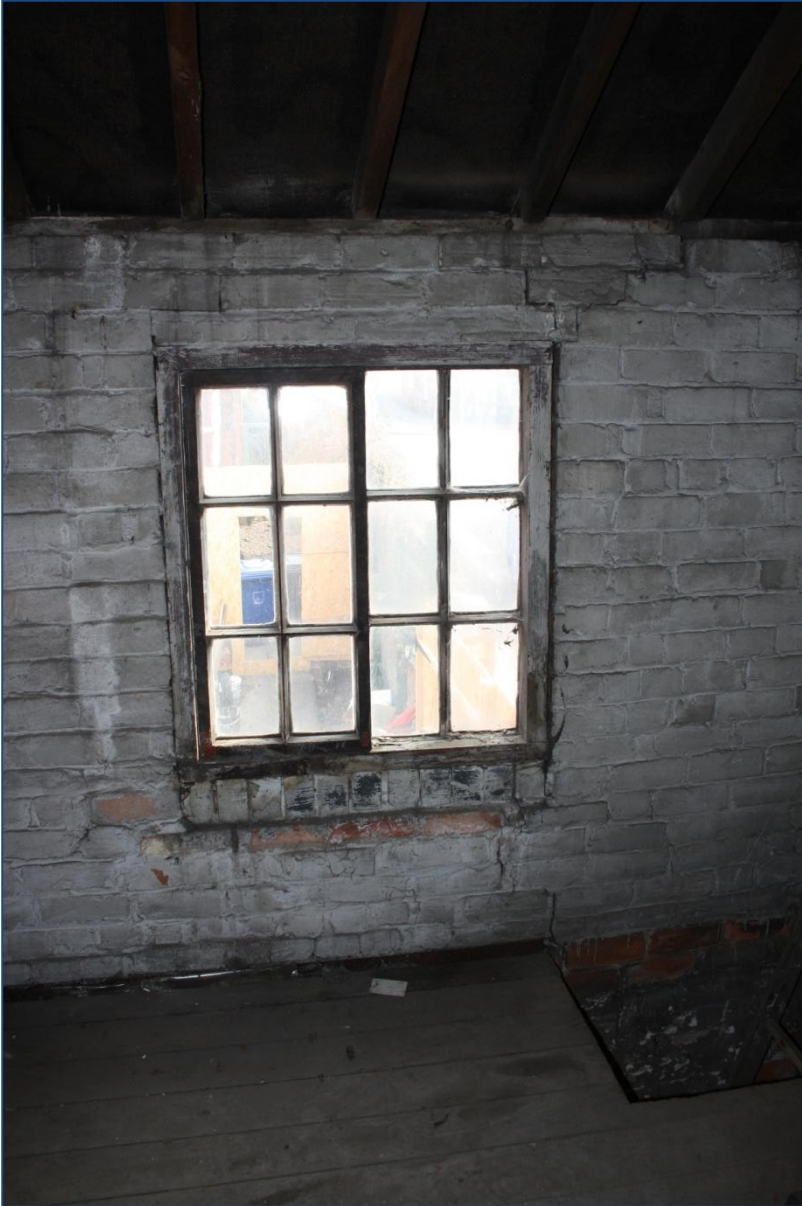
Plate 18: Sliding sash in Room 3 looking east.
