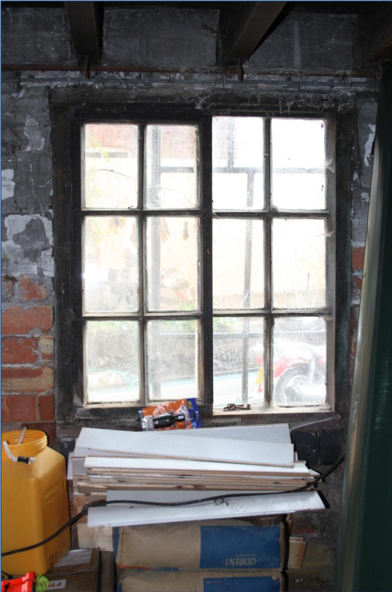
Plate 16: Sliding sash window in Room 1 looking east.
