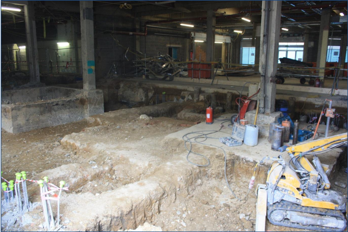
Plate 3: Location of lift pits Area 2 looking north-east.
