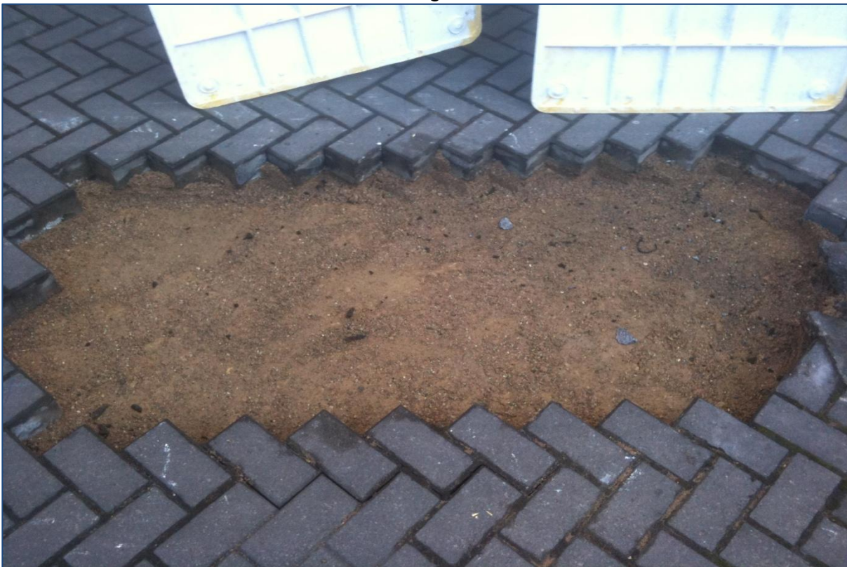
Plate 2: Test-hole looking north-east.
