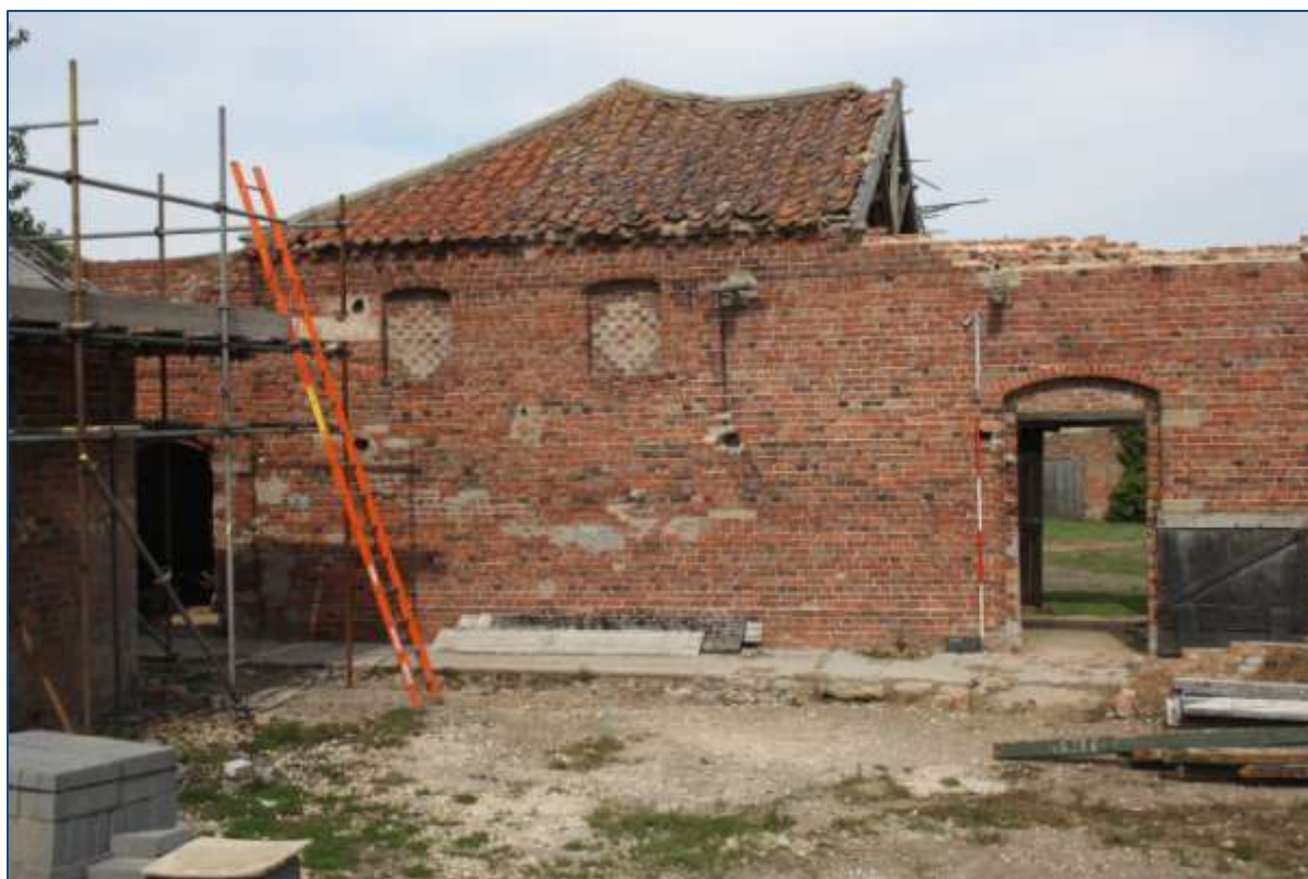
Plate 28: G1 showing false pitch-holes ‘ventilators’ in south-east elevation.
