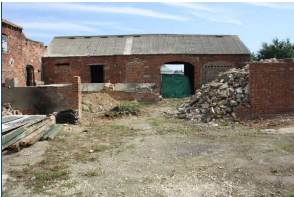
Plate 24: G5 and G6 showing blocked openings in south-west facing.
