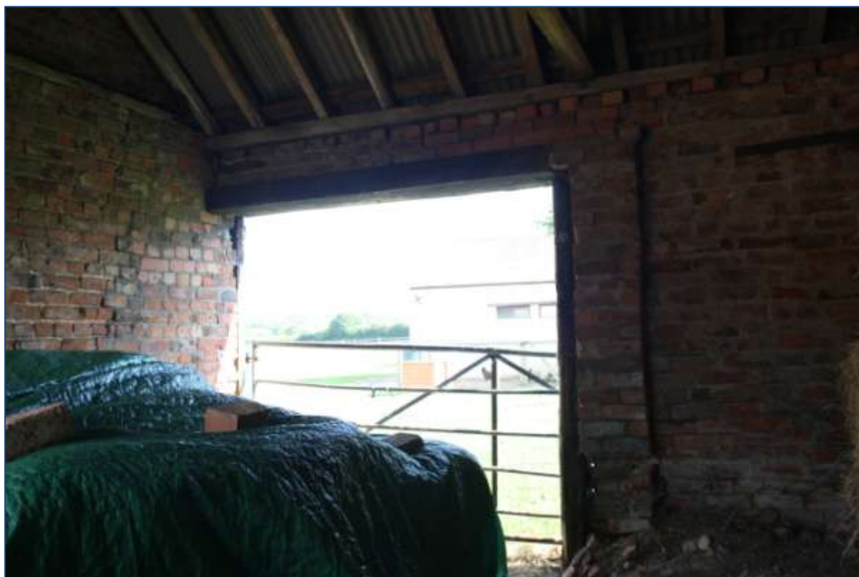
Plate 16: G6 interior looking north.
