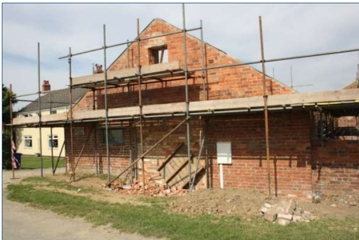
Plate 4: Block 2 south-east facing elevation looking north-west.
