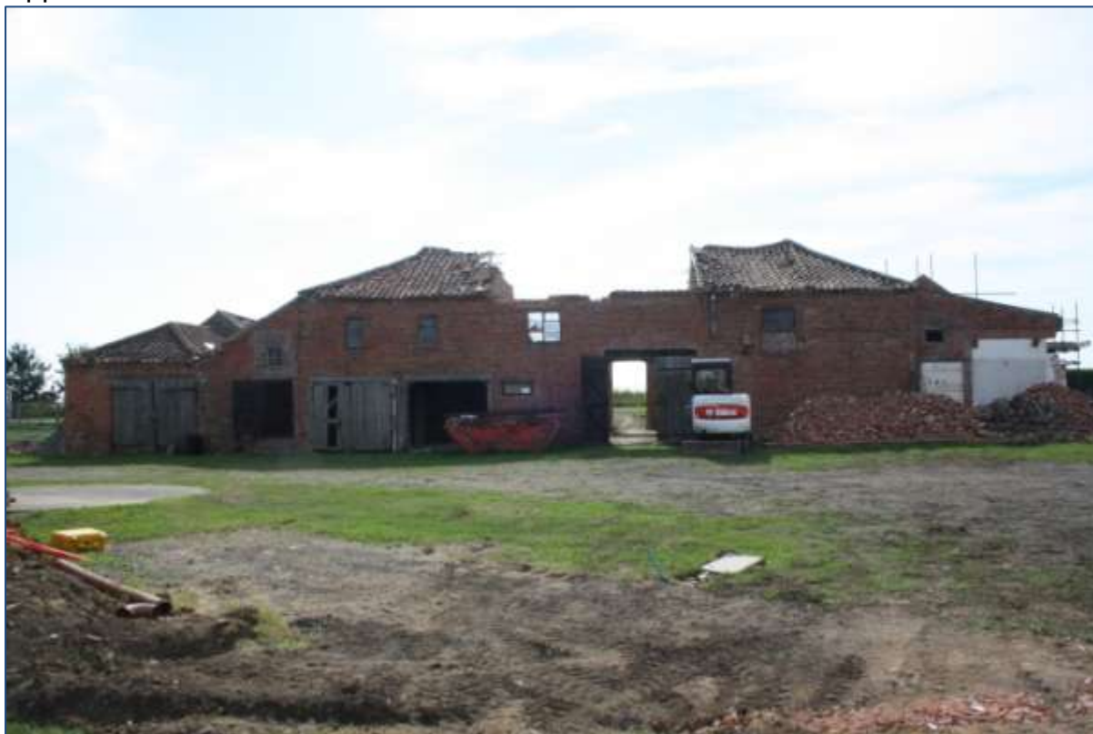
Plate 2: Block 1 north-west elevation looking south-east.
