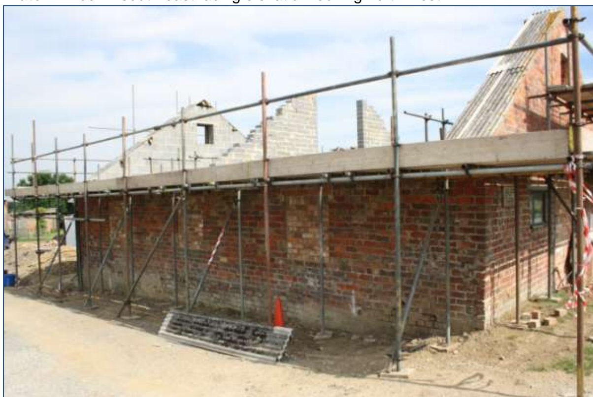
Plate 5: Block 2 south-west elevation looking north.
