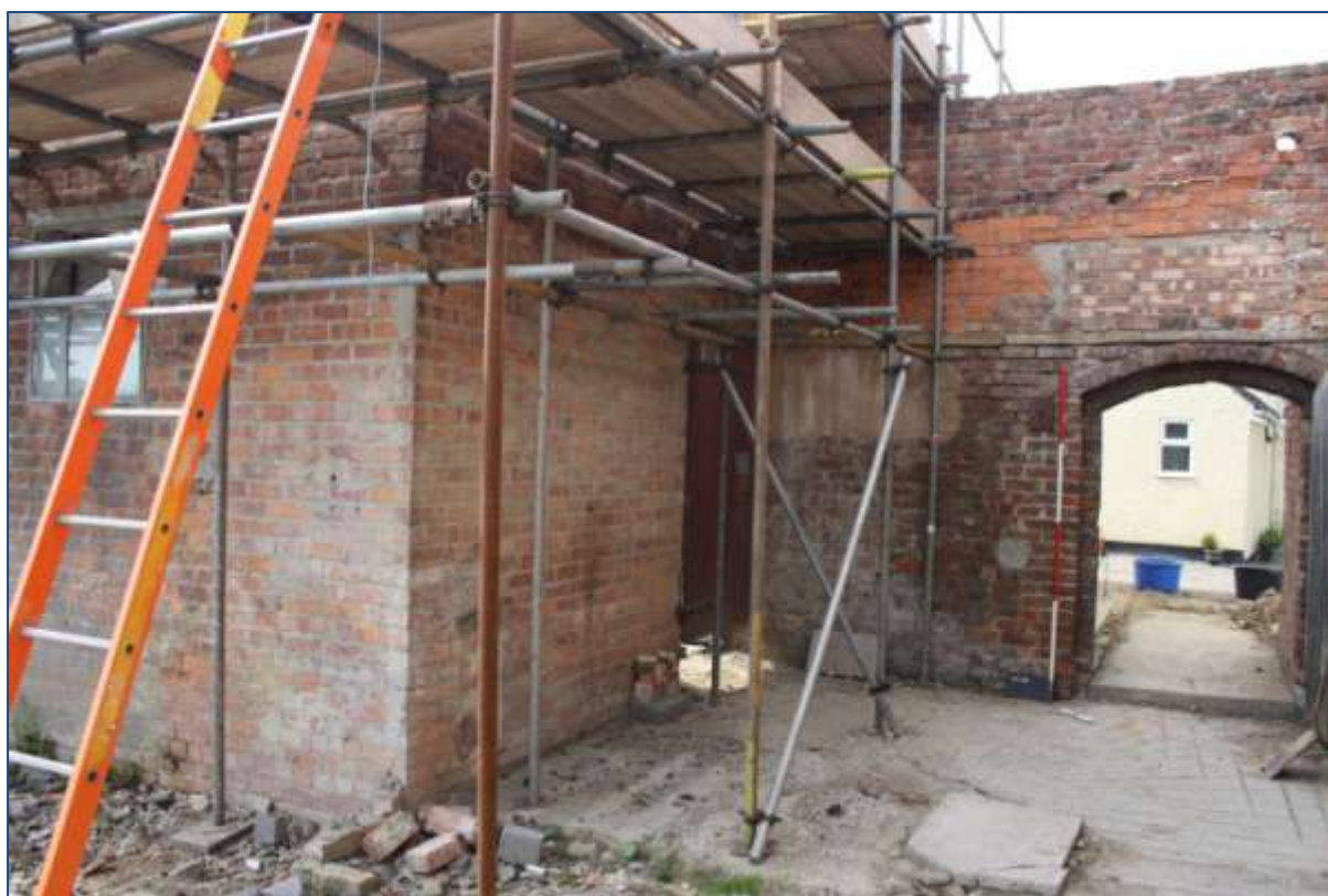
Plate 20: Access through wall towards farmhouse with G9 left and G8 right.
