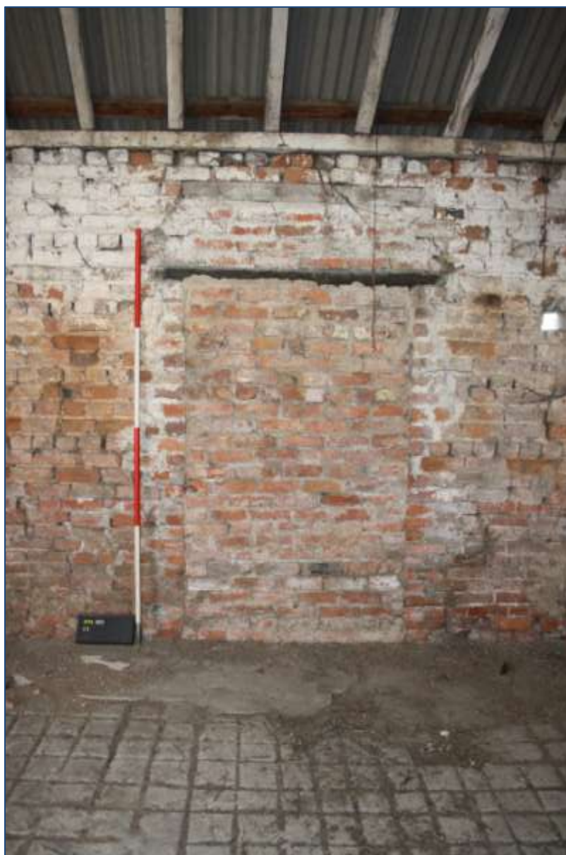
Plate 23: G5 blocked opening in north-east elevation interior view looking north-east.
