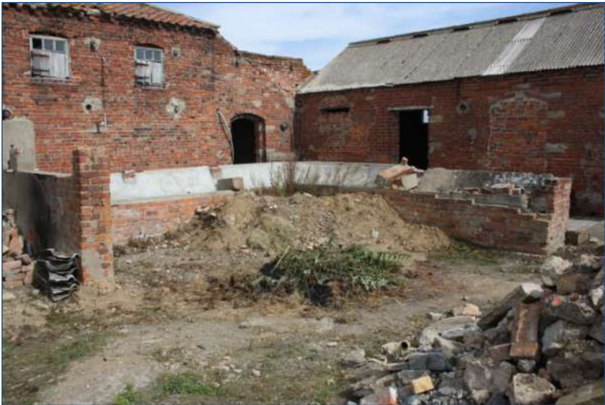
Plate 22: G5 blocked openings in south-west elevation looking north.
