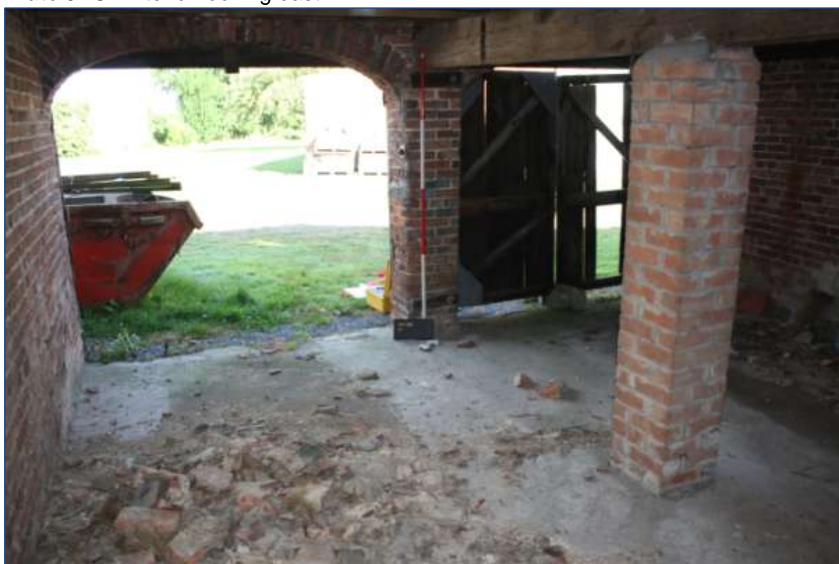
Plate 10: G2 interior looking north.
