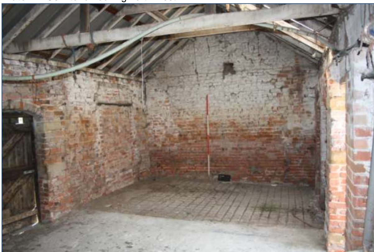
Plate 13: G5 interior looking south-east.
