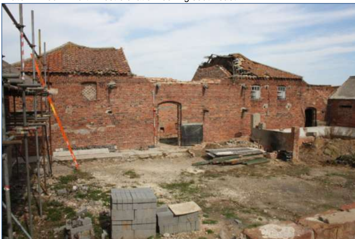
Plate 3: Block 1 south-east facing elevation looking north.
