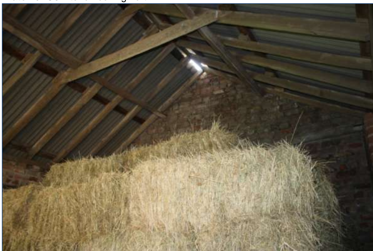
Plate 17: G6 roof structure looking south-east.
