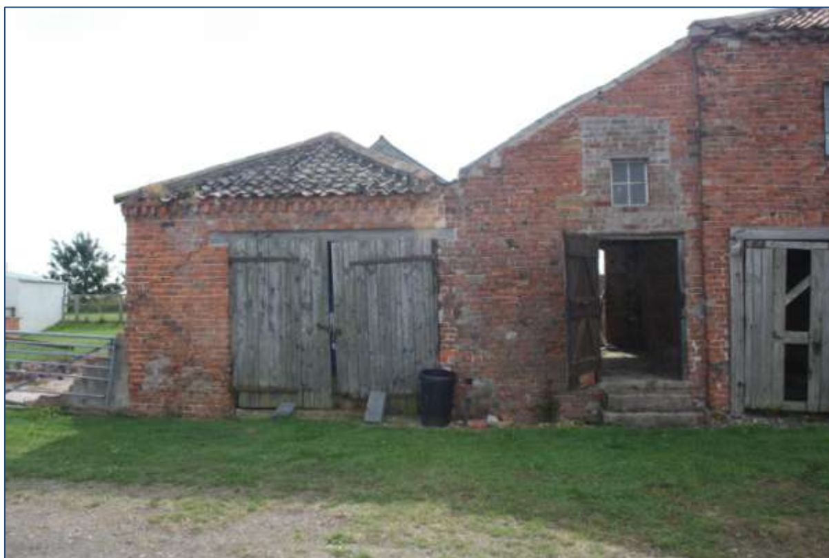
Plate 25: G4/G3 north-west elevation showing altered pitch-hole looking south-east.
