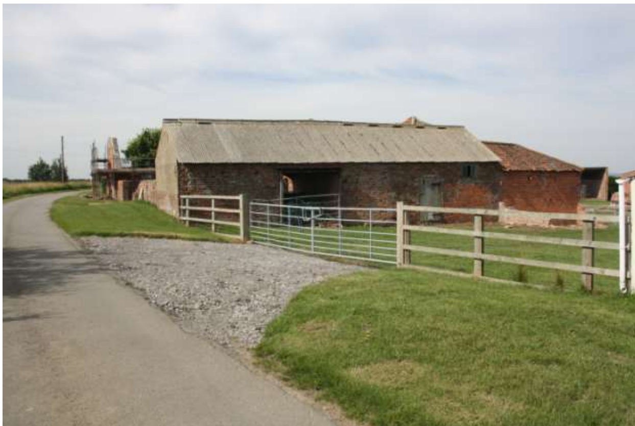
Plate 6: Block 1 south-east elevation looking north-west.
