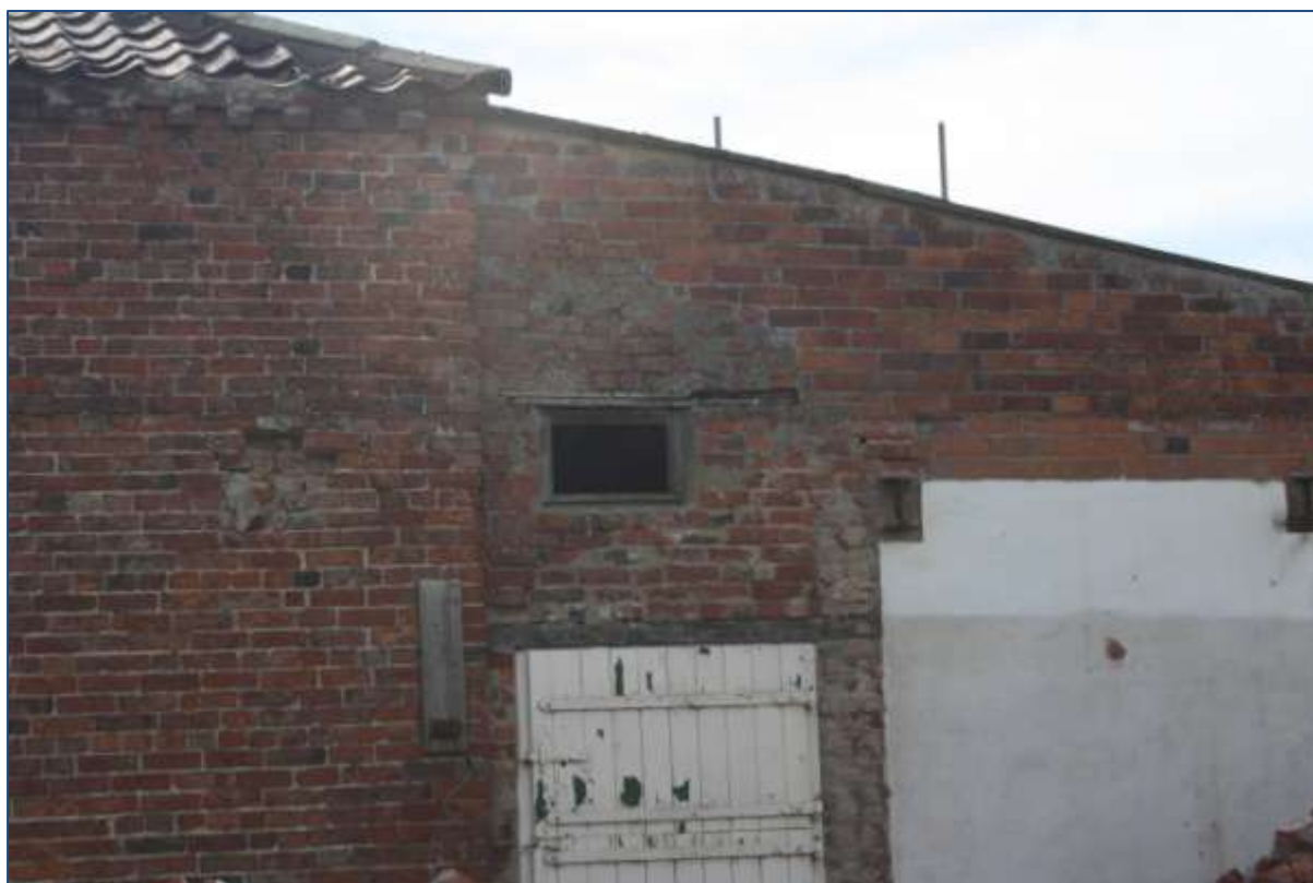
Plate 26: G8 showing opening in north-west elevation looking south-east.
