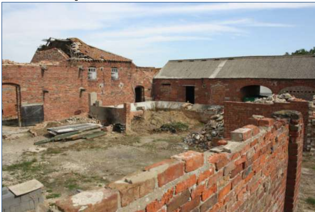
Plate 1: Site looking north-east.
