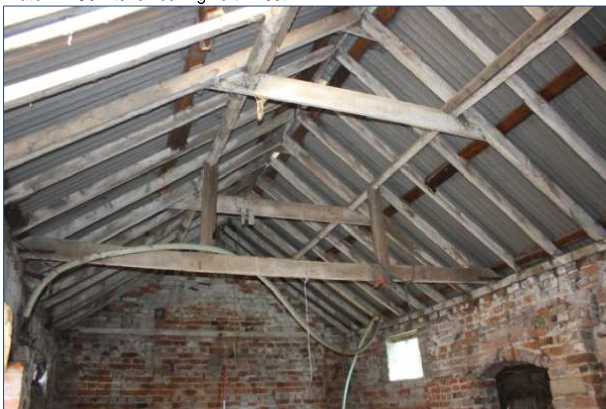
Plate 15: G5 Roof structure looking north-west.
