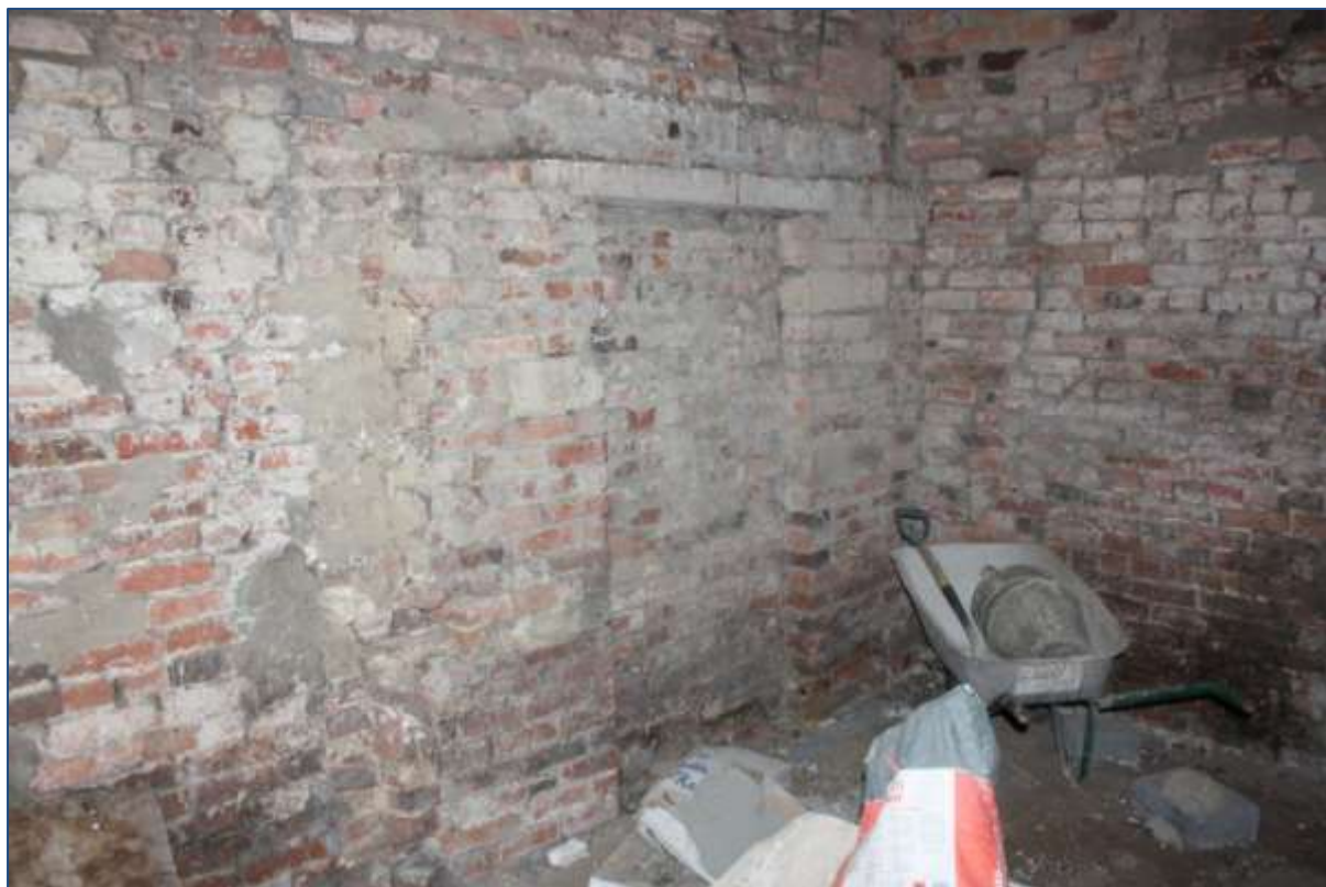
Plate 32: G8 blocked opening in north-west corner looking west.
