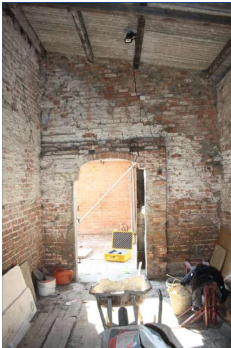
Plate 19: G8 interior looking south-east.
