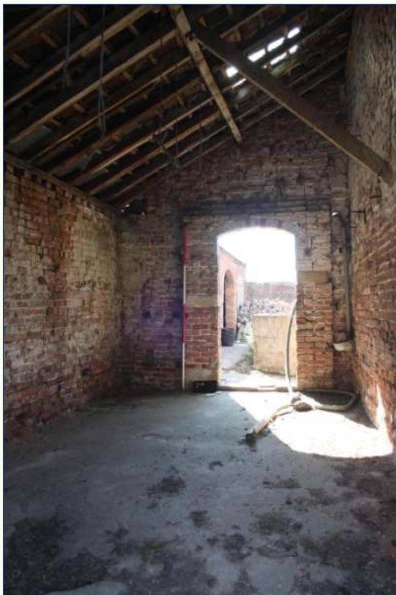
Plate 11: G3 interior looking south-east.
