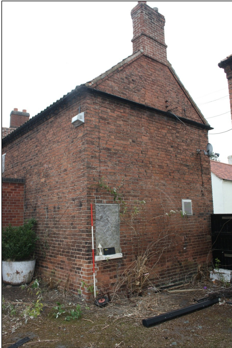
Plate 73: Old Greyhound Inn S facing elevation.
