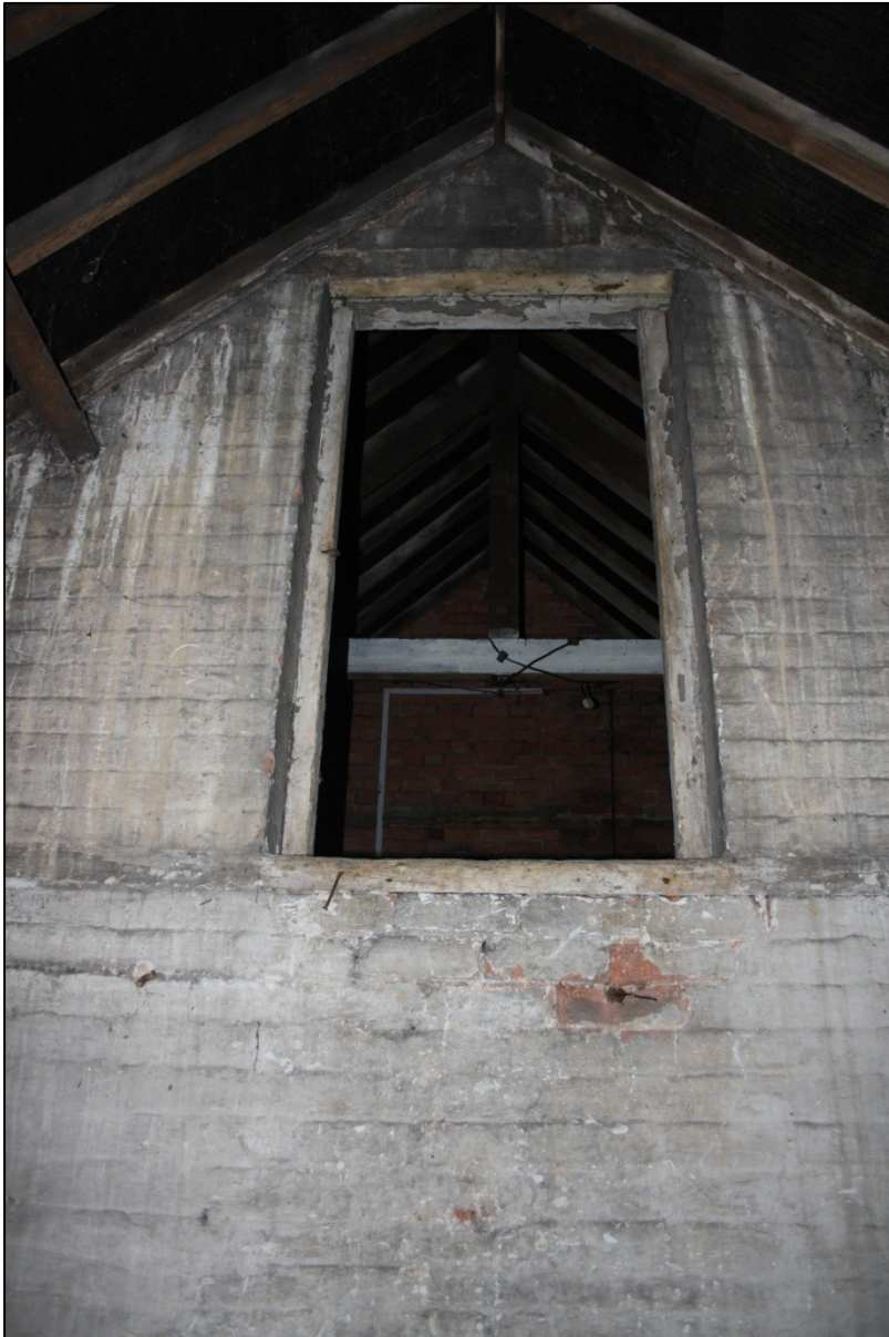
Plate 36: G17 access to loft looking N/E.
