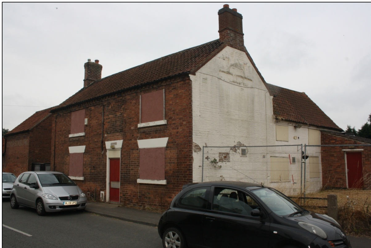
Plate 76: Old Greyhound Inn N facing elevation.
