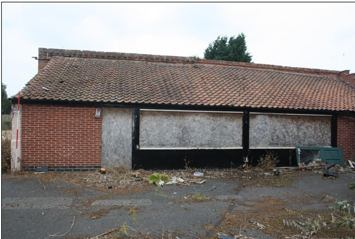
Plate 78: Old Greyhound Inn E facing elevation.
