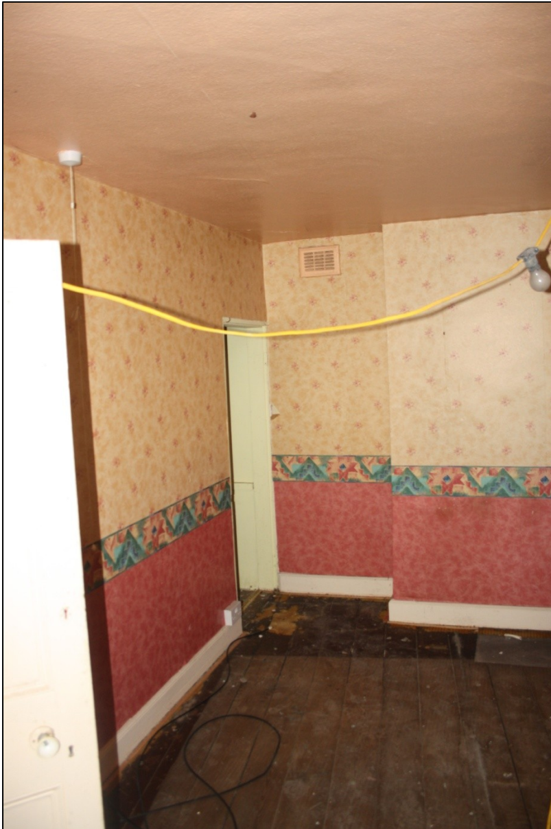
Plate 53: F20 looking N/W.
