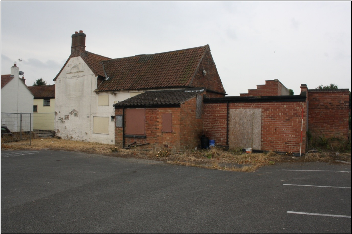
Plate 74: Old Greyhound Inn N facing elevation.
