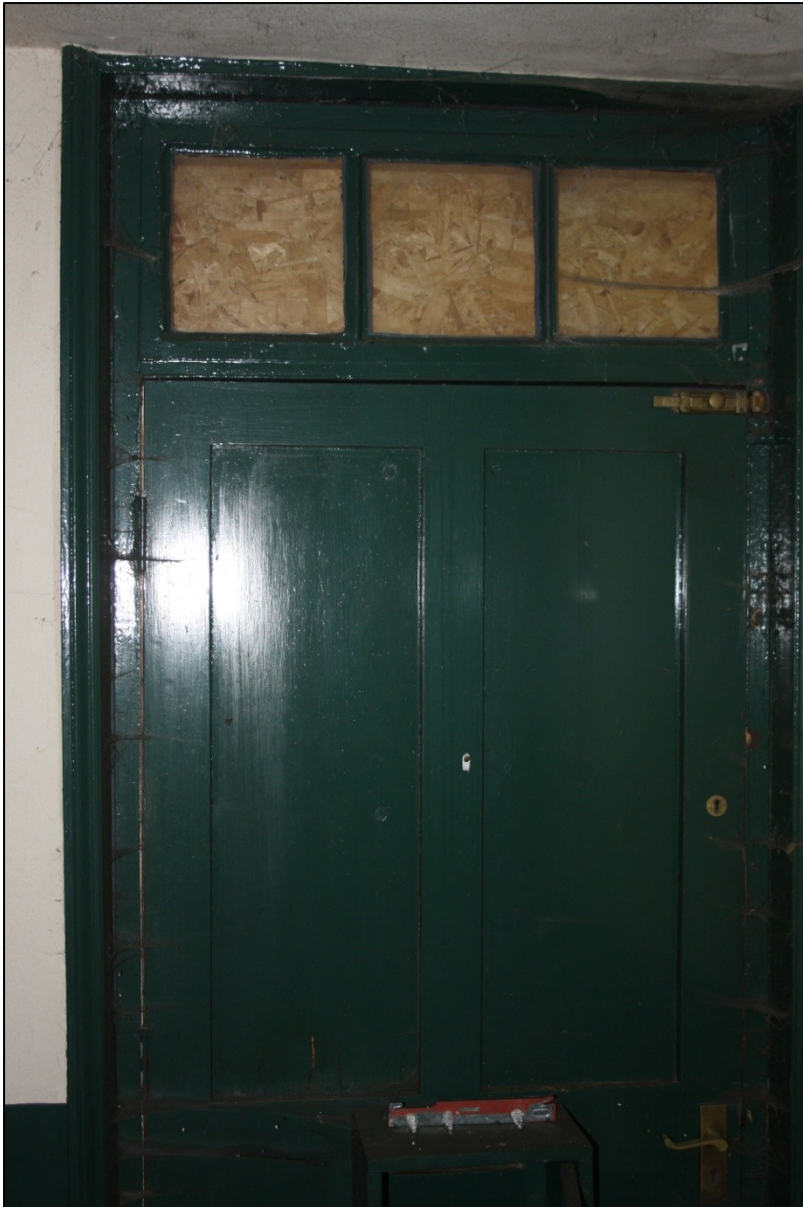
Plate 15: G7 looking S/E towards main entrance.
