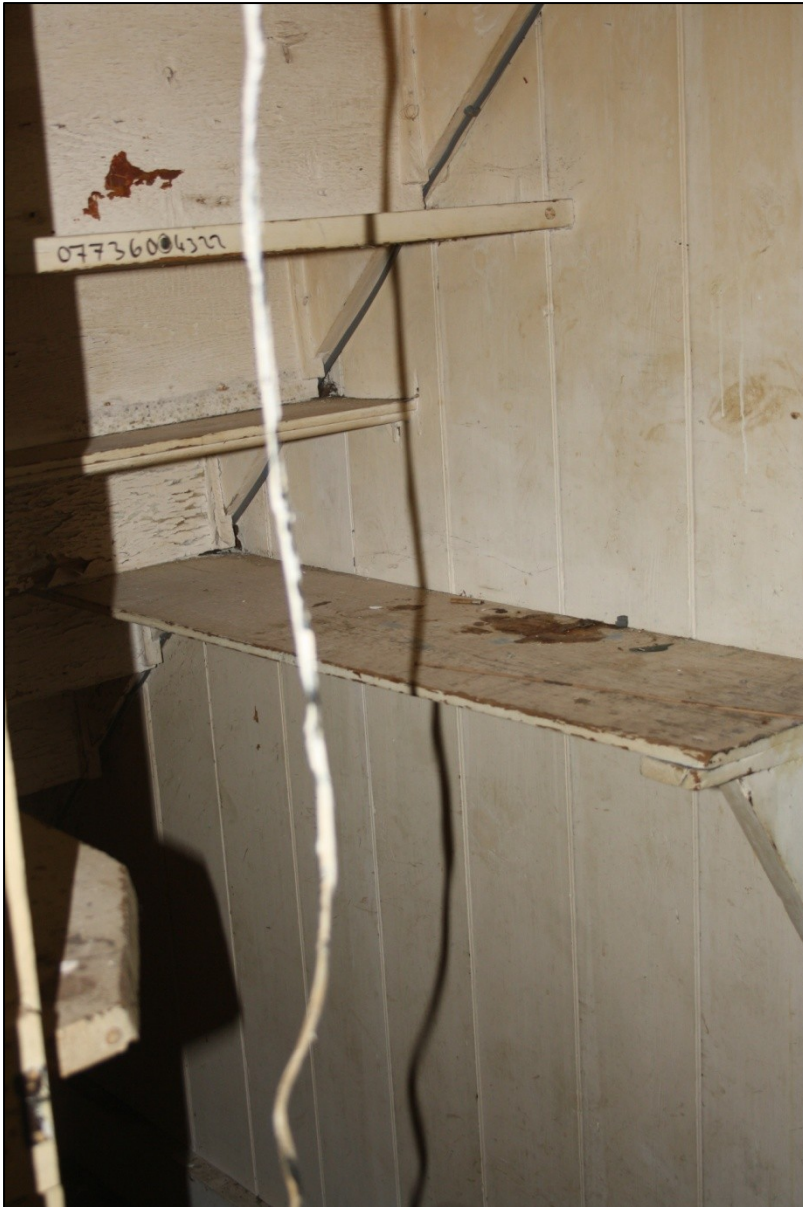
Plate 12: G6 under stair cupboard looking S/E.
