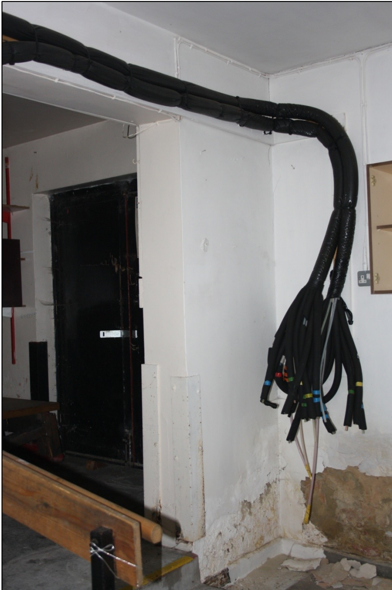
Plate 28: G12 looking N/W.
