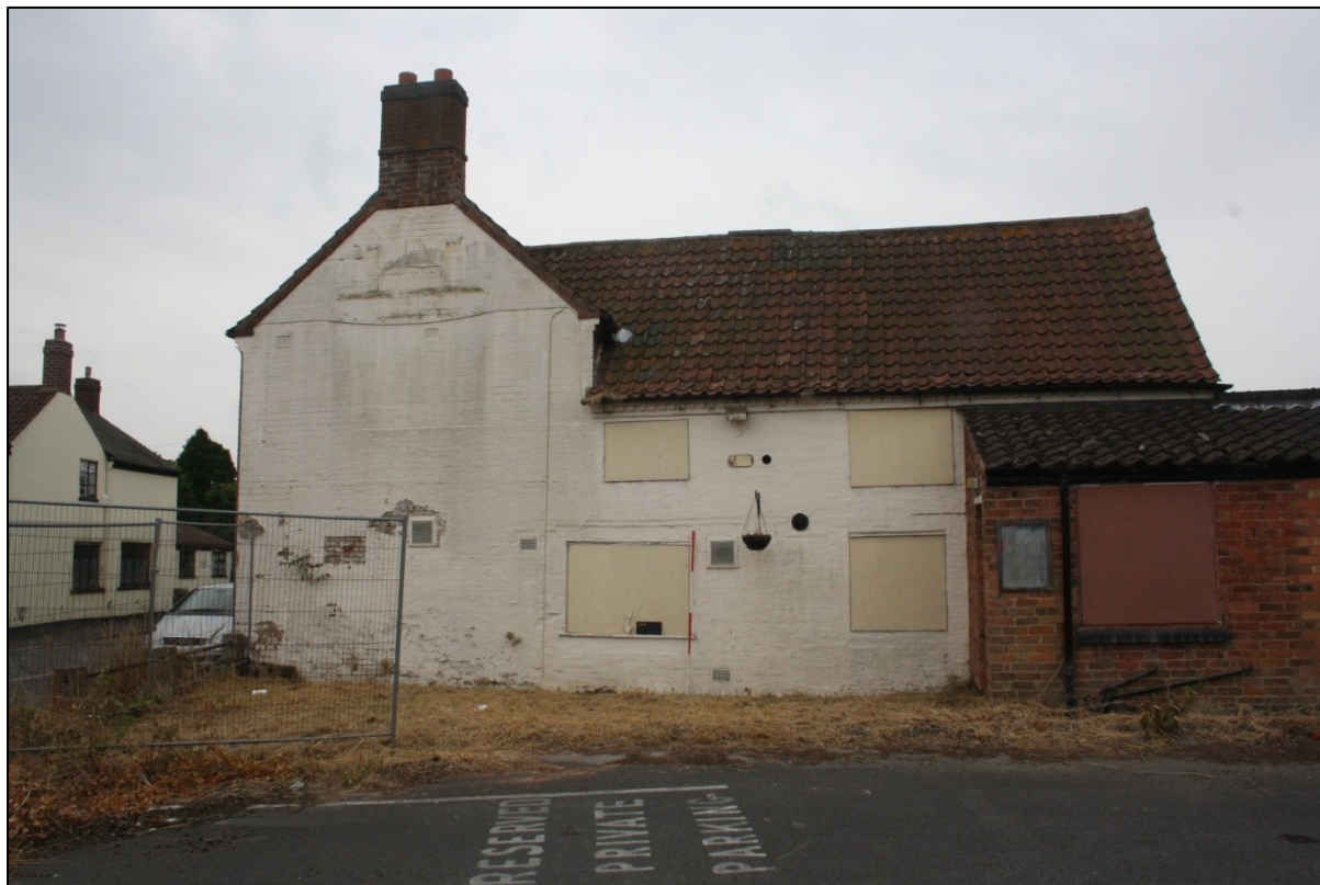
Plate 69: Old Greyhound Inn N facing elevation.
