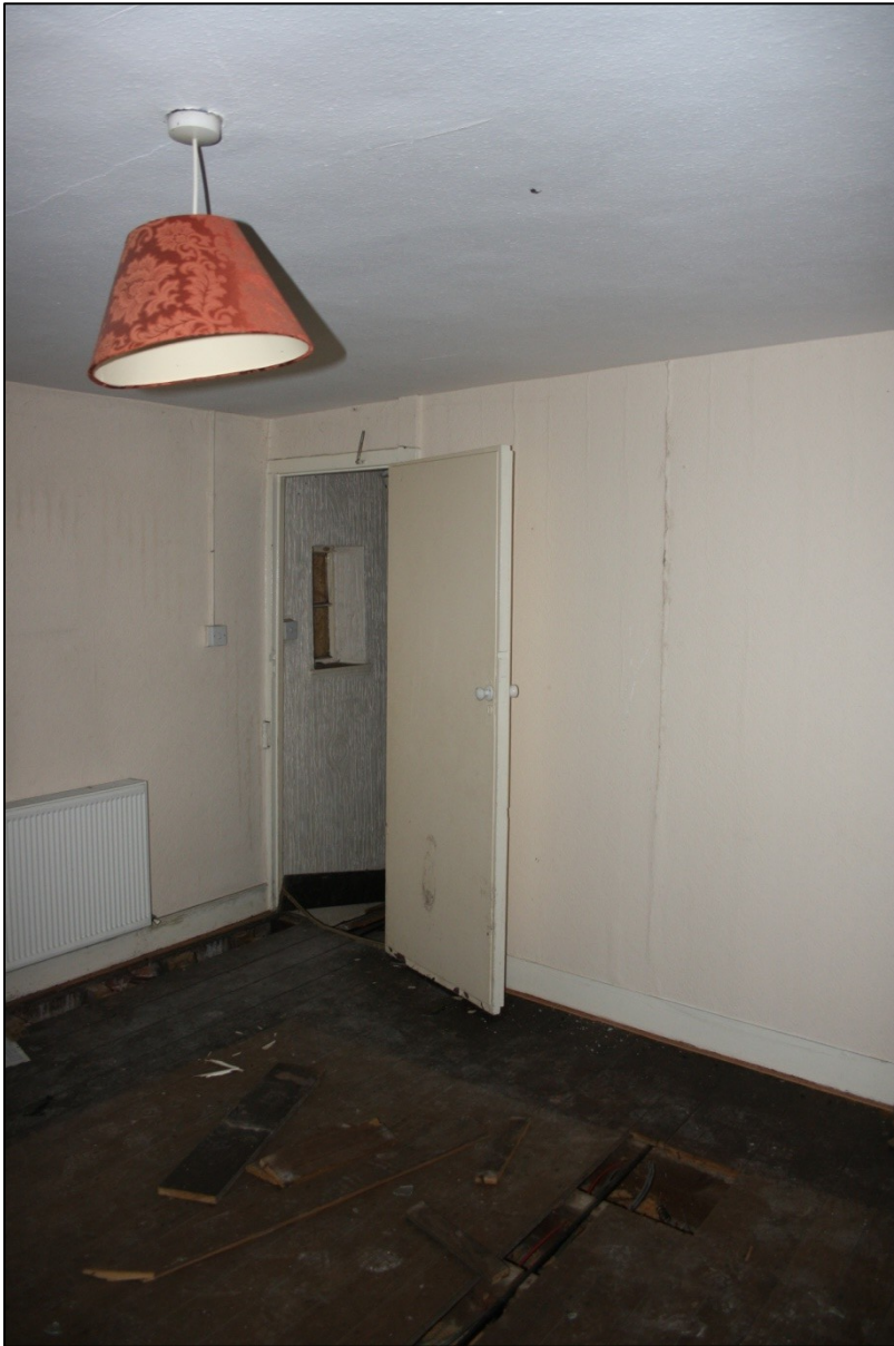
Plate 51: F19 looking N/W to entrance.
