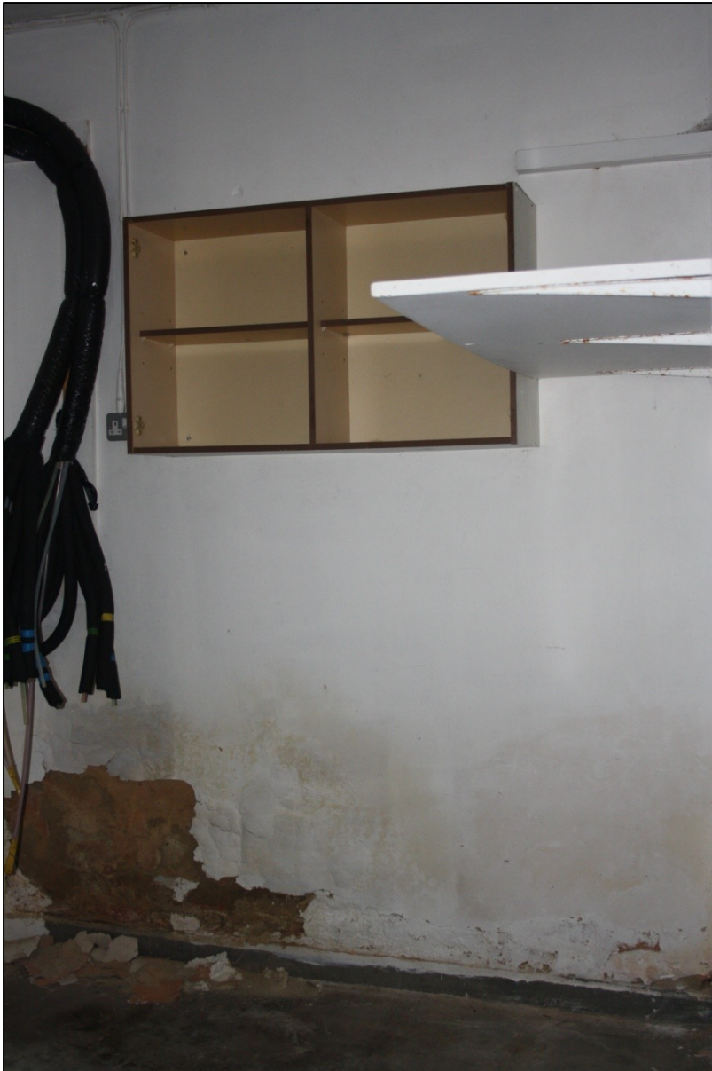
Plate 29: G12 looking N/W.
