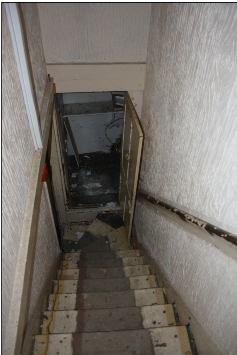
Plate 57: F22 looking S/E down stairs.
