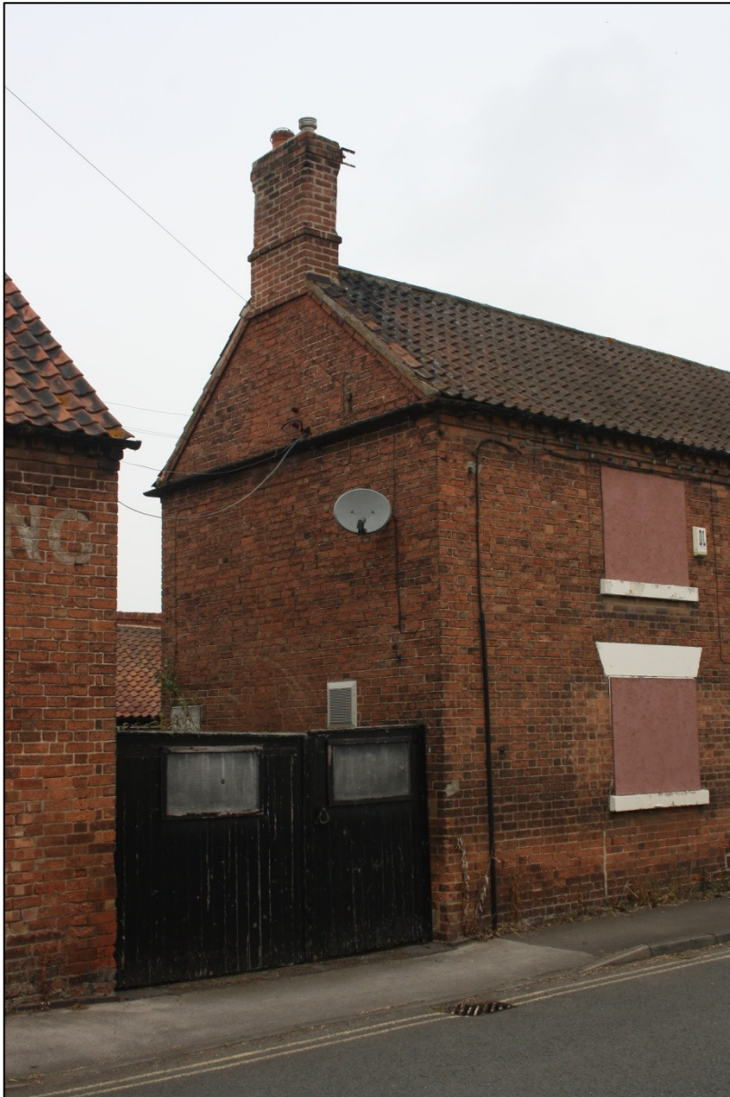
Plate 71: Old Greyhound Inn E facing elevation.
