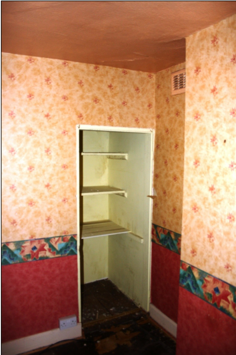
Plate 55: F20 looking N/W towards cupboard.
