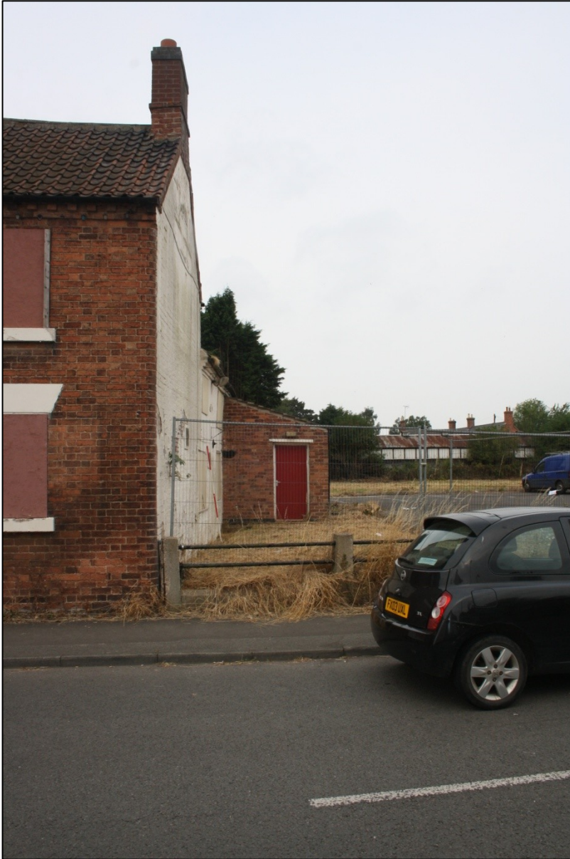
Plate 75: Old Greyhound Inn E facing elevation.
