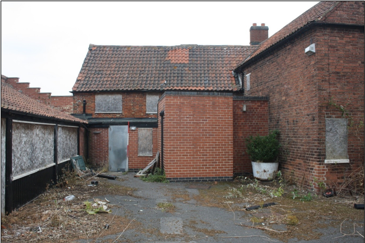
Plate 72: Old Greyhound Inn S facing elevation.
