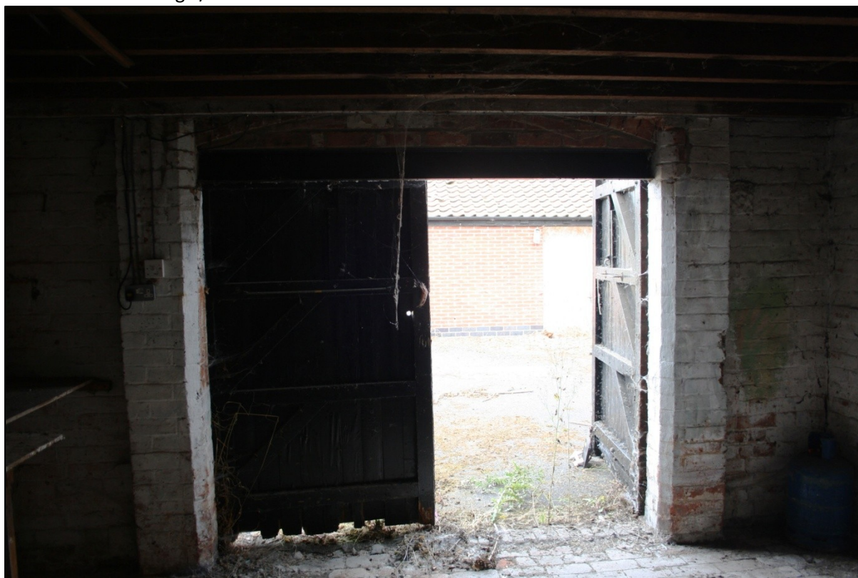
Plate 48: G18 looking N/W.
