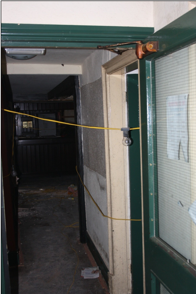
Plate 14: G7 looking N/W.
