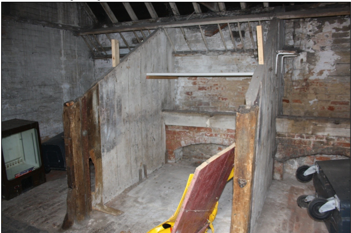
Plate 38: G17 stalling looking N/E.
