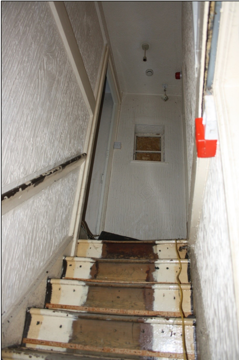
Plate 16: G7 looking N/W up stairs
