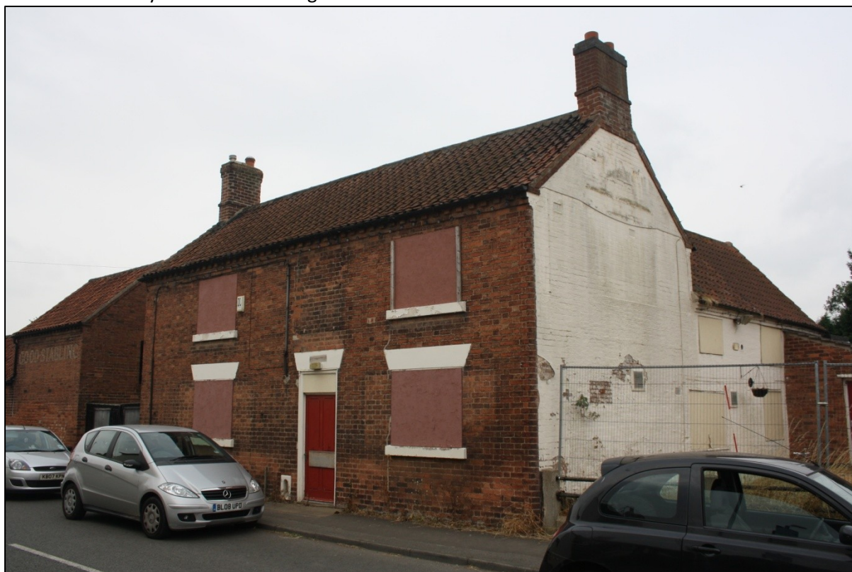
Plate 70: Old Greyhound Inn E facing elevation.
