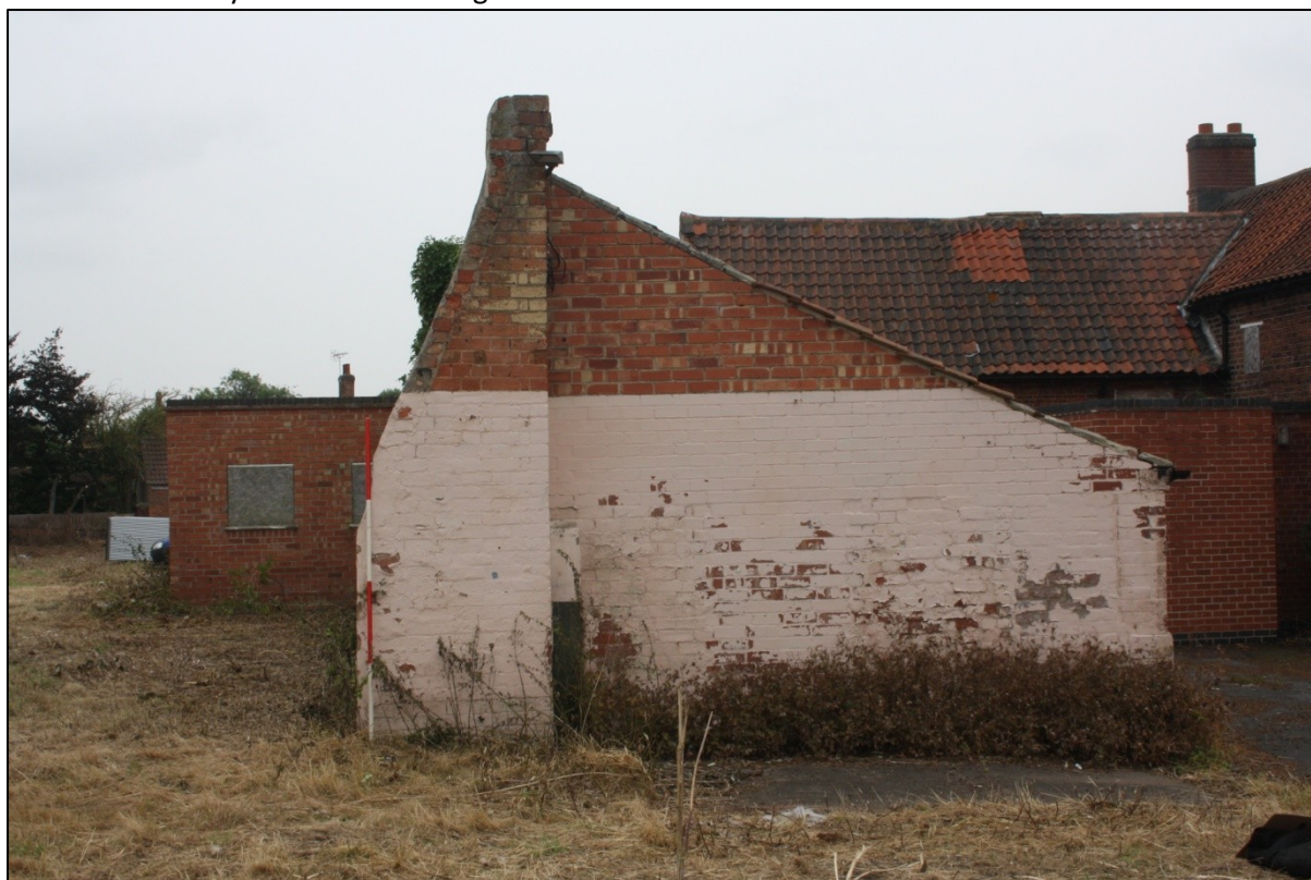
Plate 77: Old Greyhound Inn S facing elevation.
