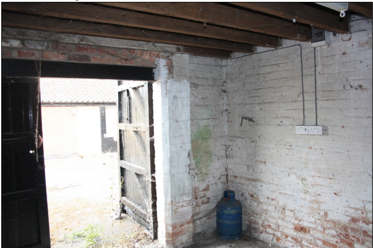
Plate 46: G18 looking N/W.
