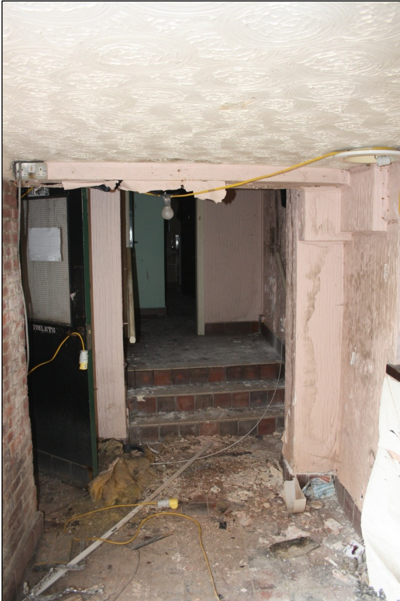
Plate 2: G1 looking N/W.
