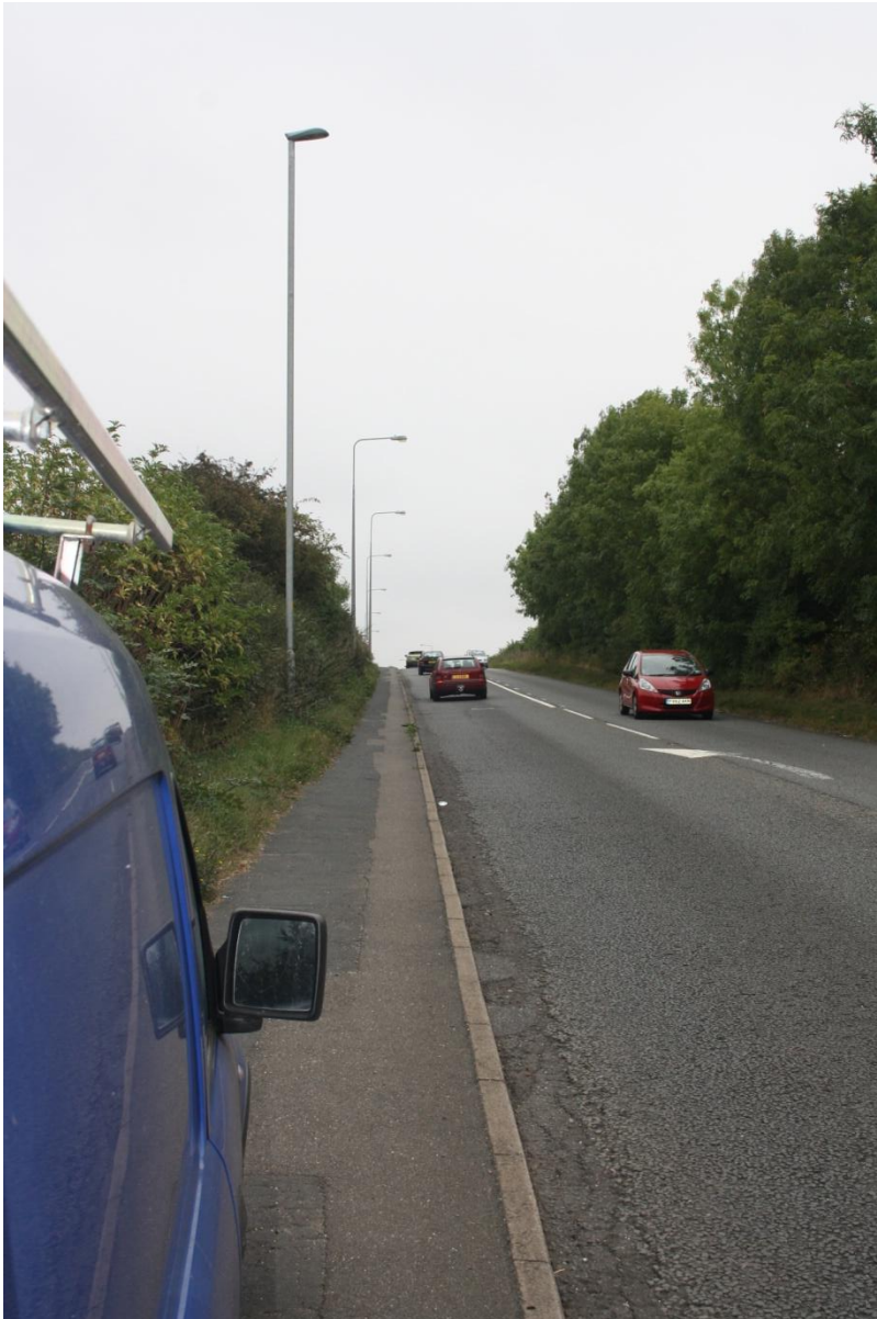
Plate 1: View looking S/E along site boundary with A52.
