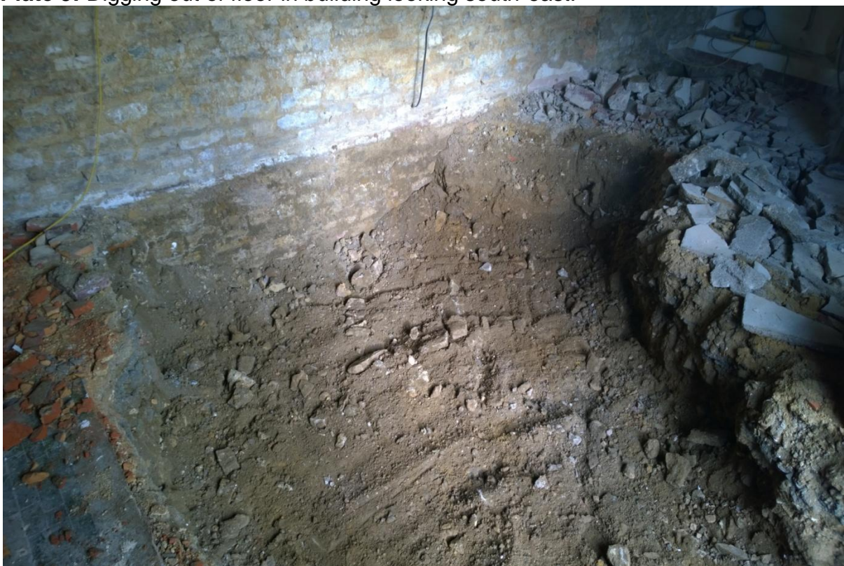
Plate 4: Interior of building after digging out looking north-east.
