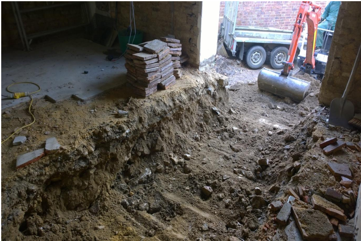
Plate 3: Digging out of floor in building looking south-east.
