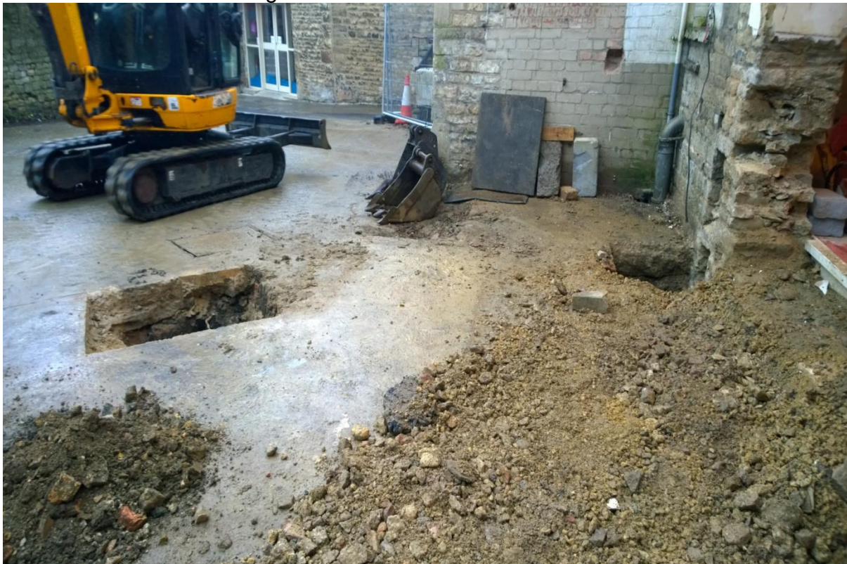
Plate 6: Pier bases 2 and 3 looking west.
