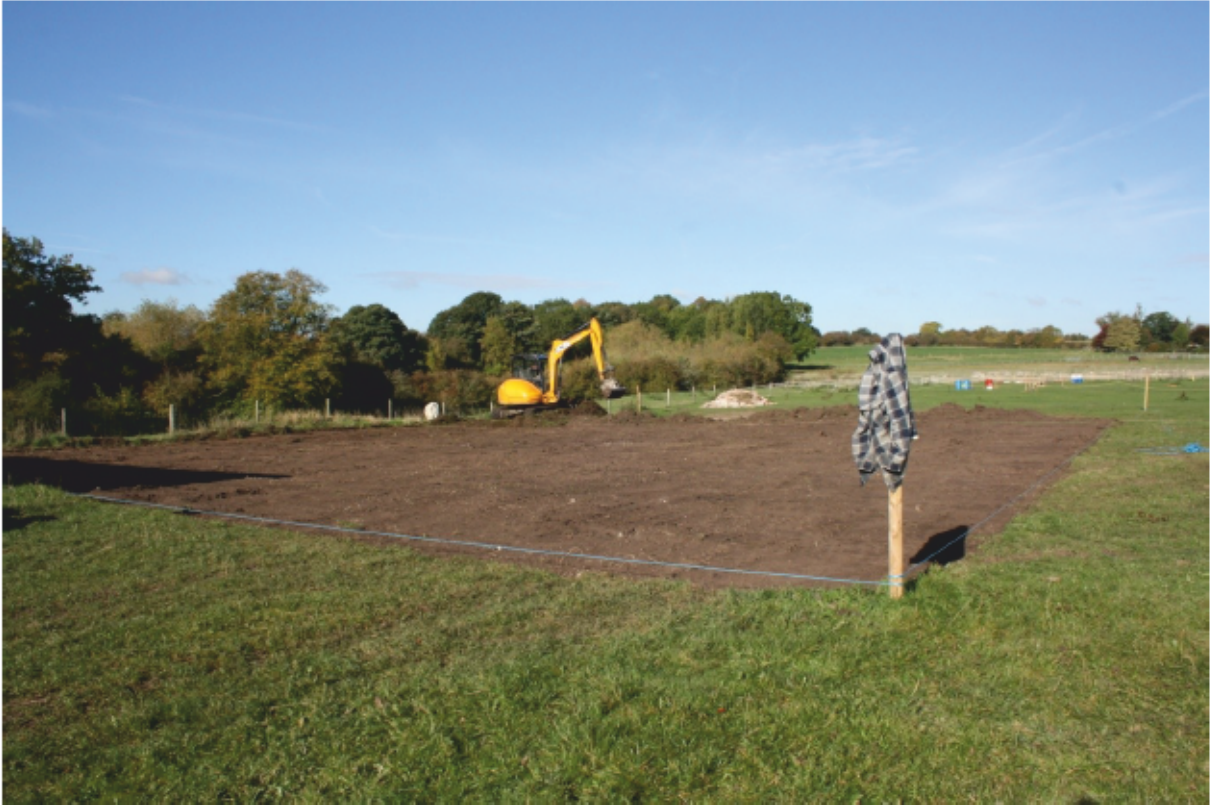
Plate 7: Ménage area fully machined looking north west.
