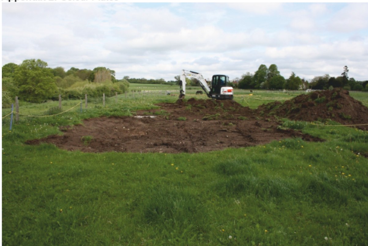
Plate 1: Site area looking north.
