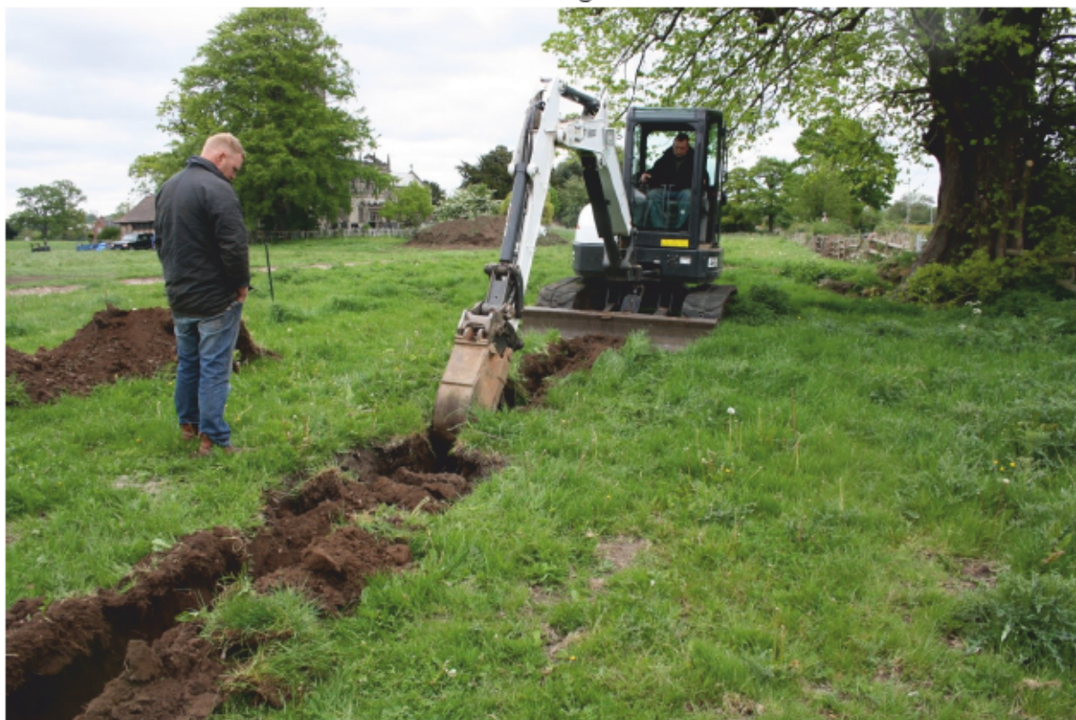
Plate 4: Service trench looking east.
