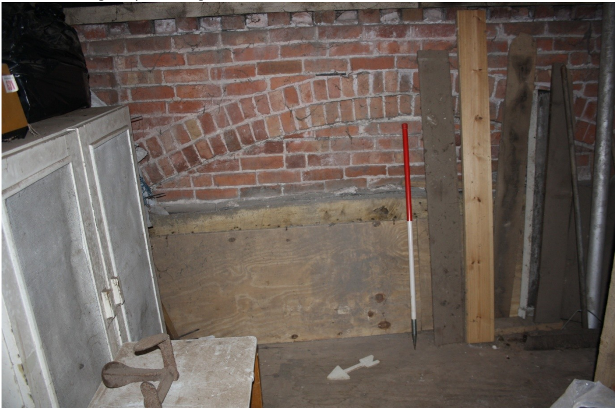
Plate 33: Landing/access area 10 looking SE.
