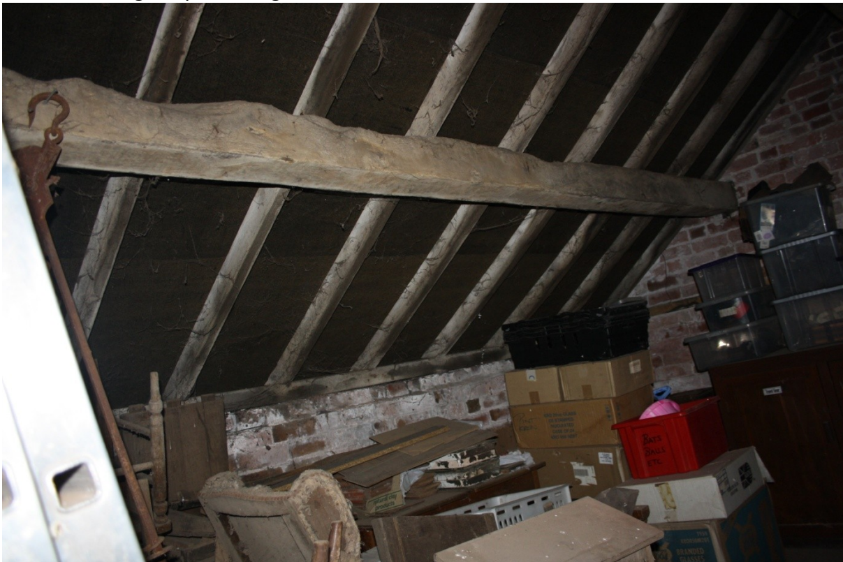
Plate 31: Storage Bay 6 looking N.
