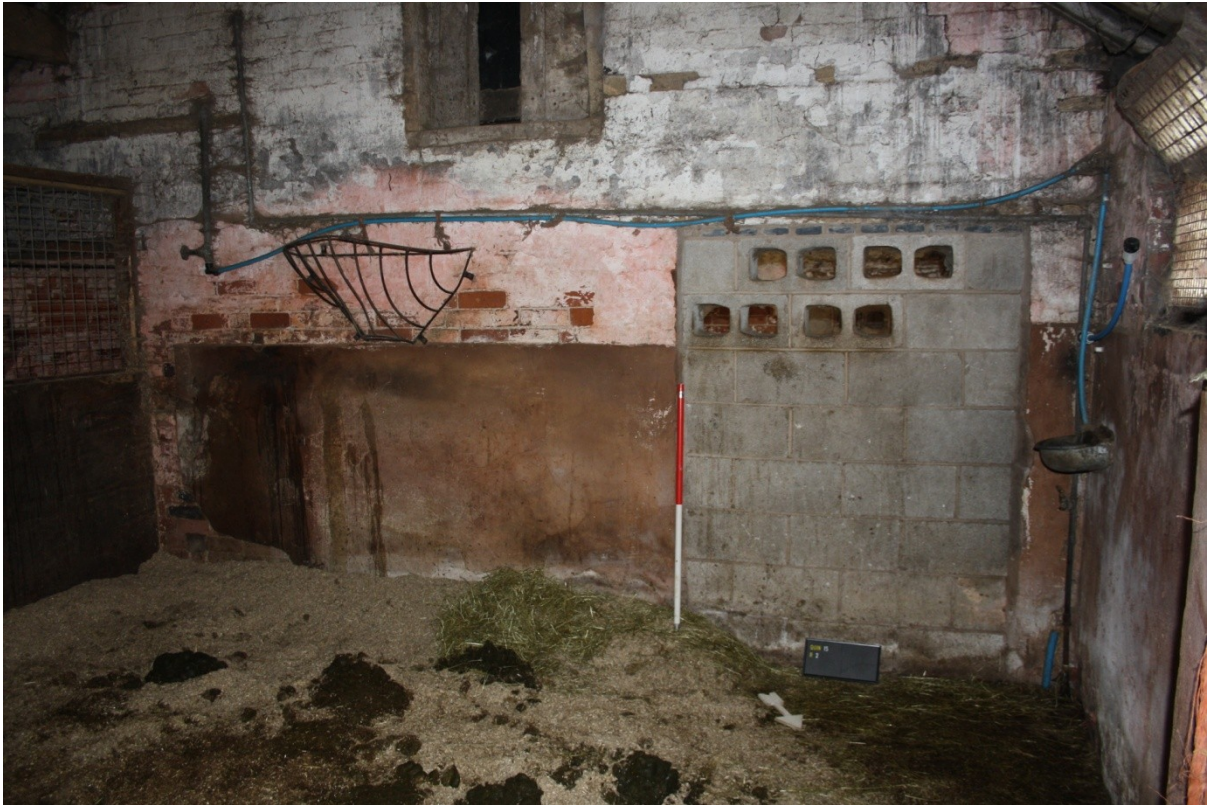
Plate 11: Cow Housing 1 looking SW
