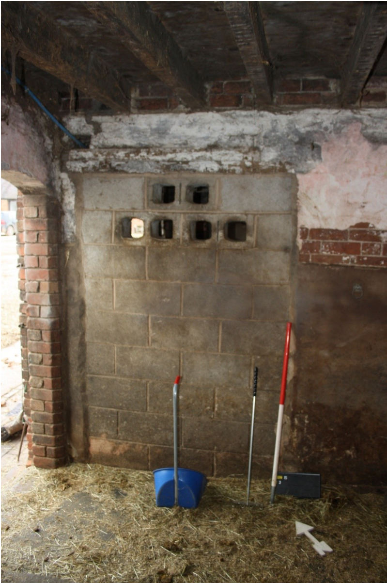
Plate 23: Cow Housing 3 looking NE.
