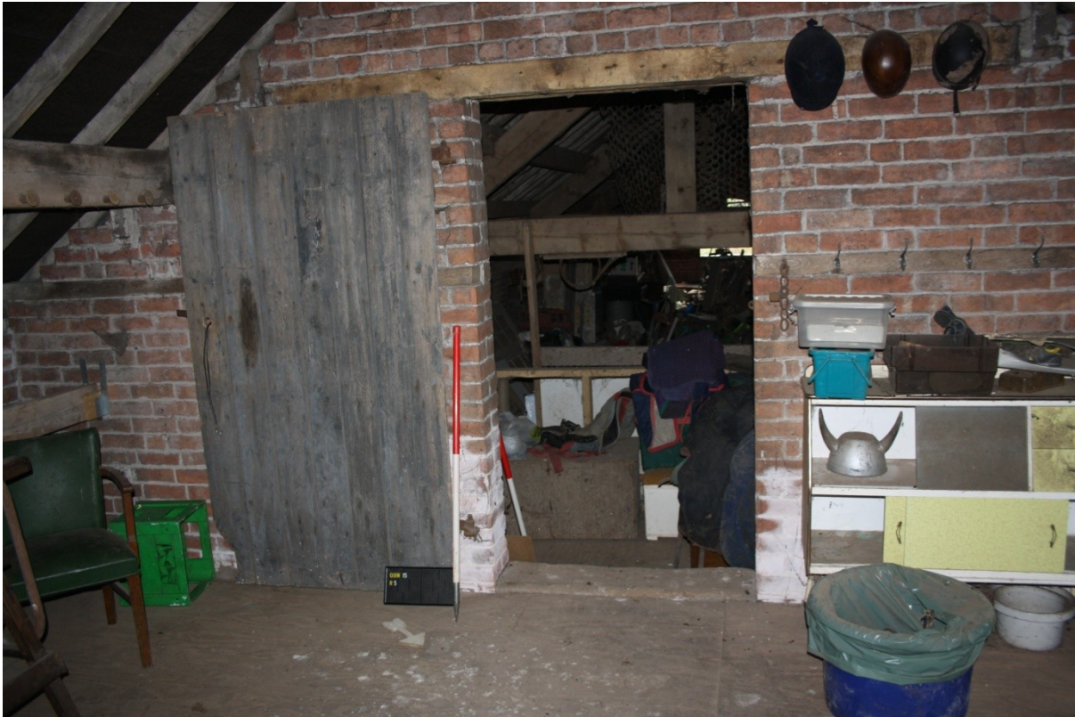
Plate 29: Storage Bay 5 looking SE.
