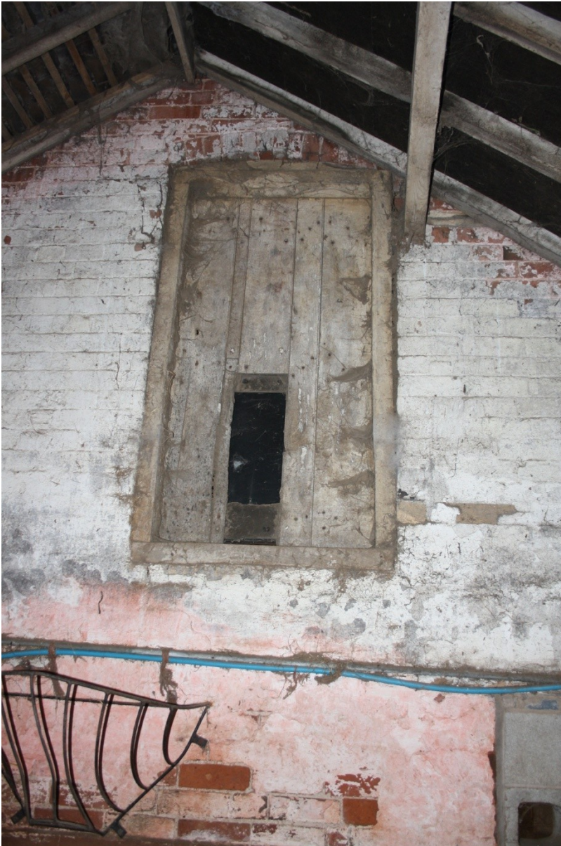
Plate 12: Cow Housing 1 looking SW.
