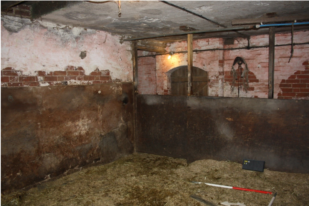
Plate 19: Cow Housing 3 looking E.
