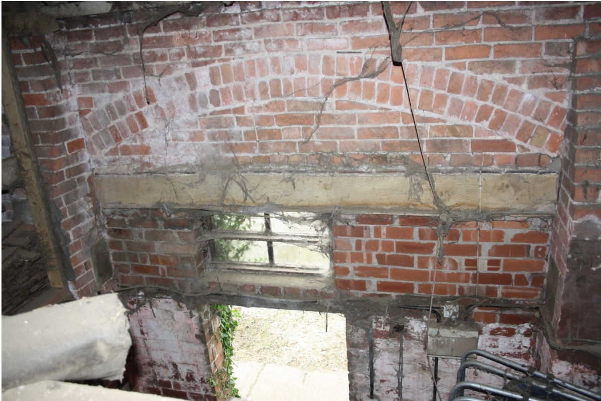
Plate 34: Landing/access area 10 looking NW.
