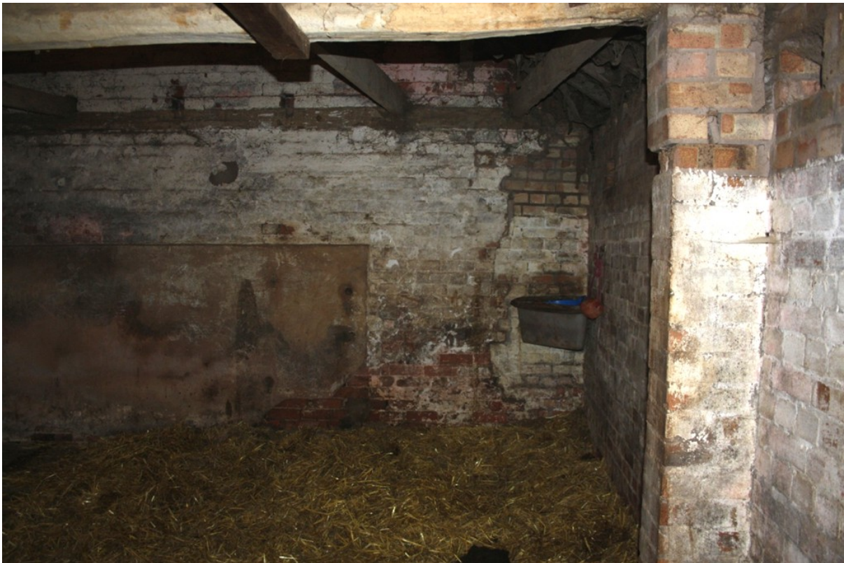
Plate 8: Cow Housing 1 looking NE.
