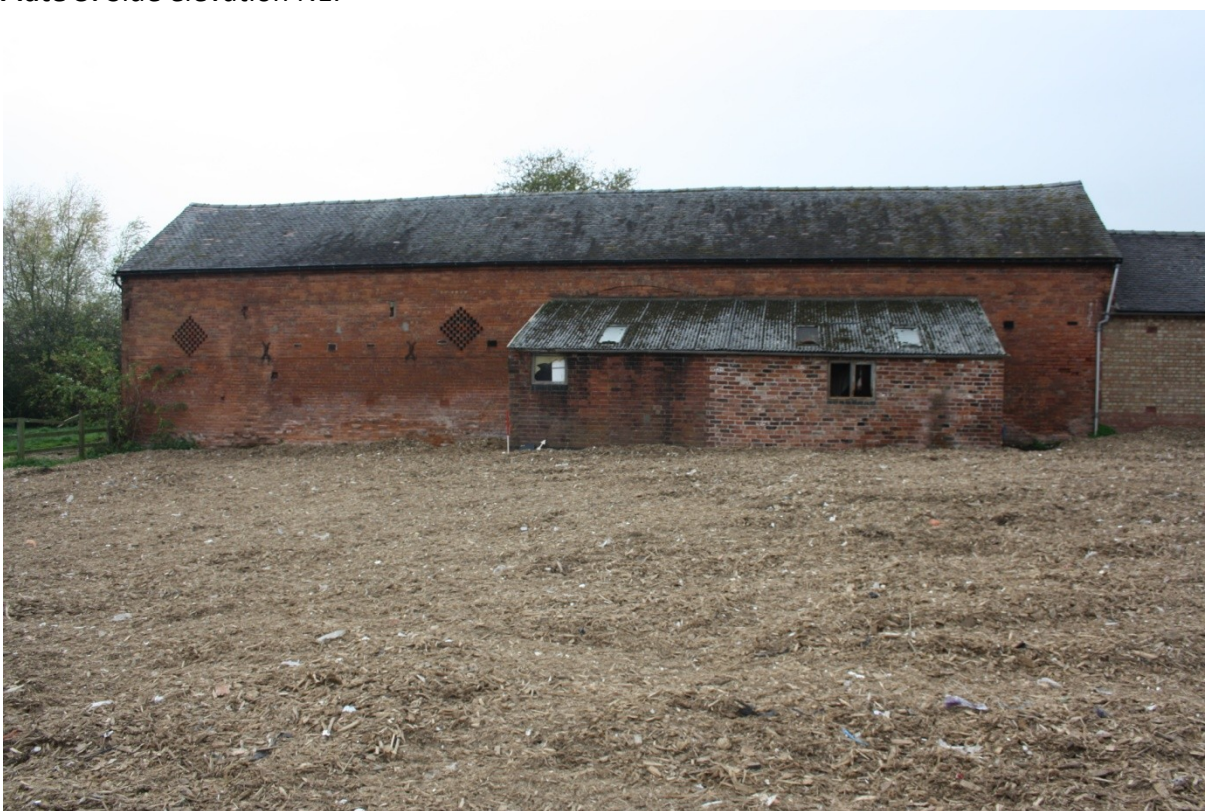
Plate 4: Rear elevation SE.
