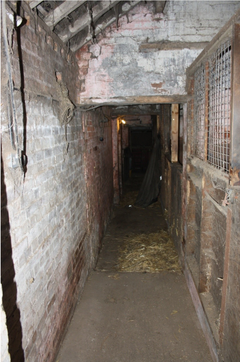
Plate 13: Corridor/feed passage ground floor looking SW.
