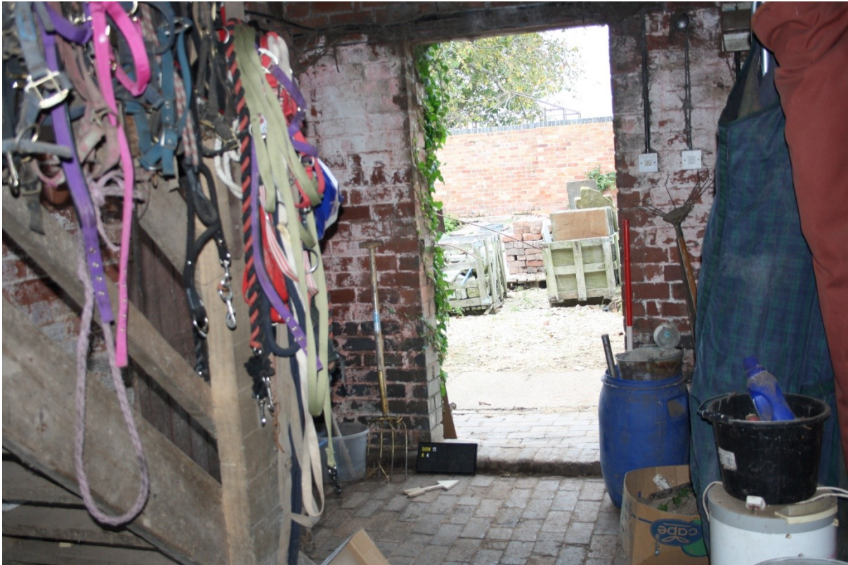
Plate 24: Threshing Barn 4 looking NW.
