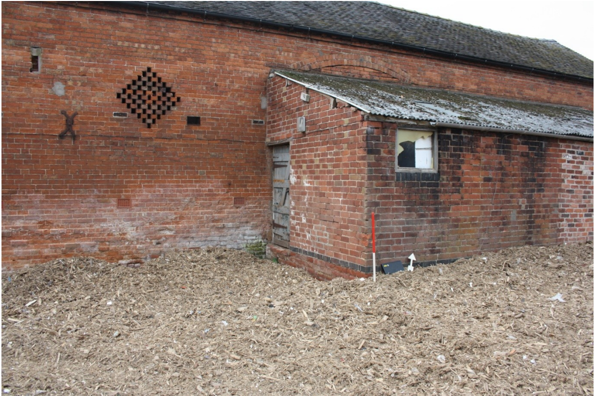
Plate 5: Side elevation SW.
