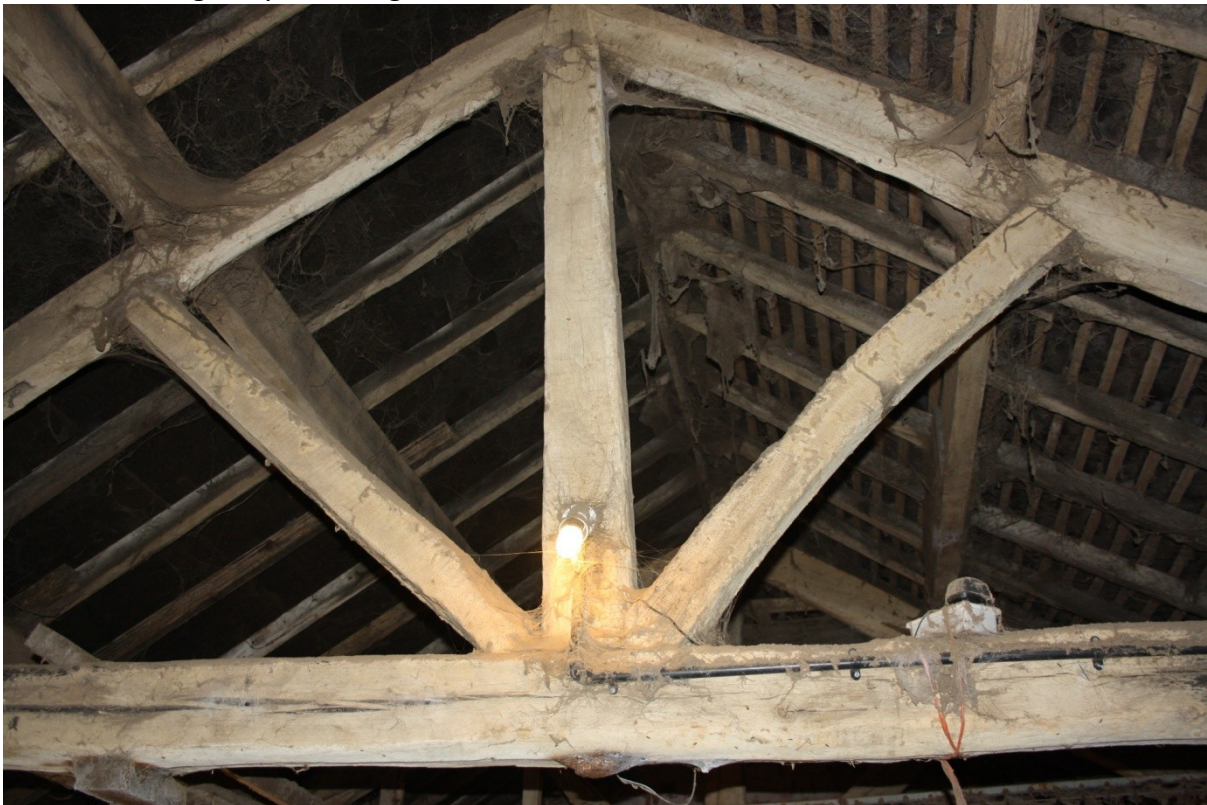
Plate 38: Cow Housing 1 looking NE.
