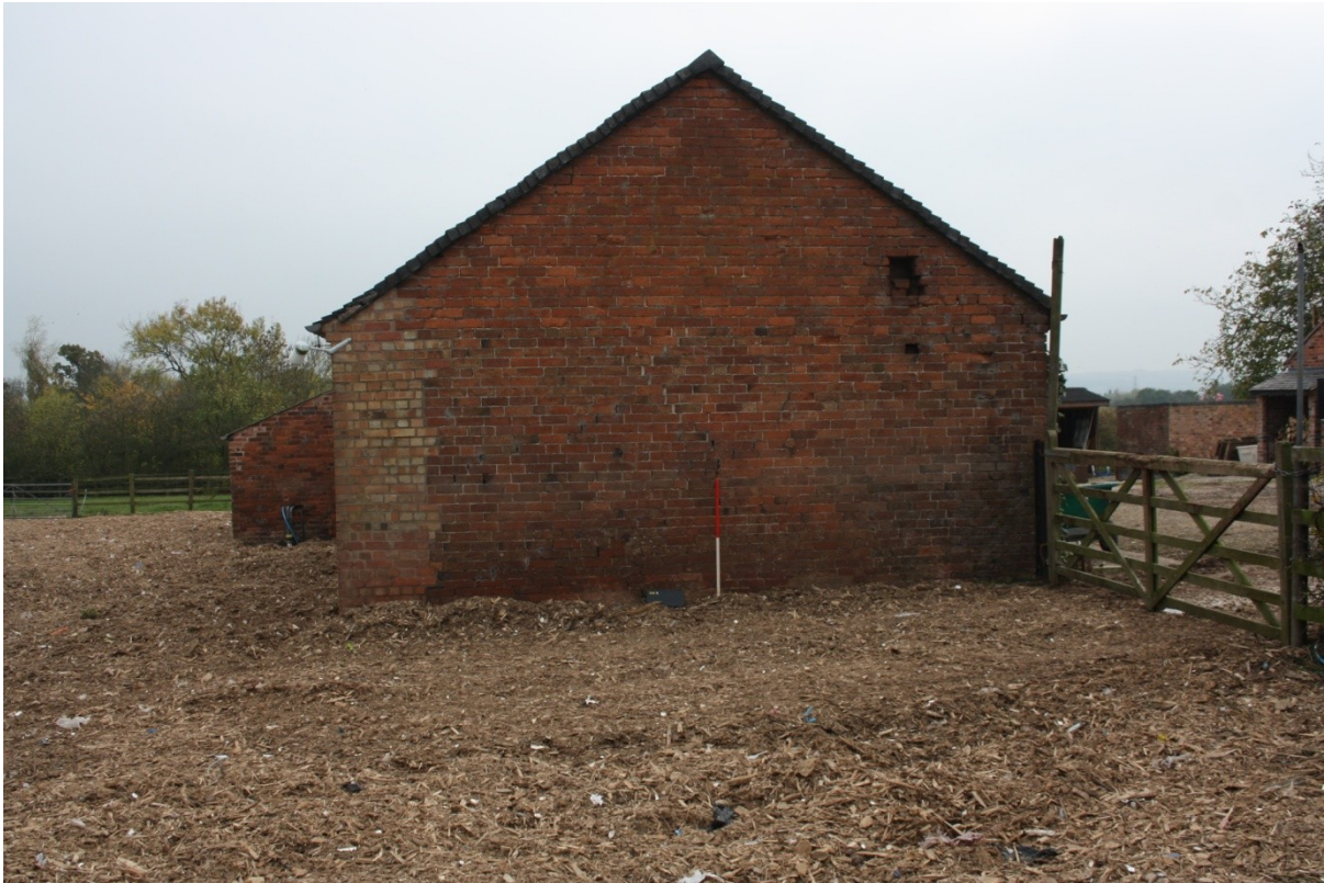
Plate 3: Side elevation NE.
