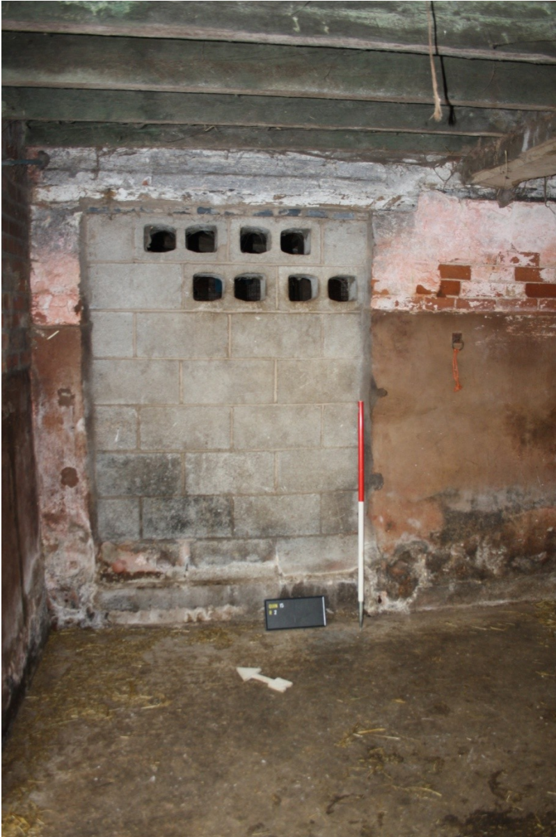
Plate 14: Cow Housing 2 looking NE.
