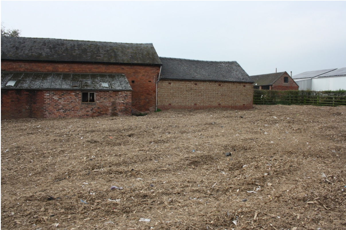
Plate 7: Side elevation SW.
