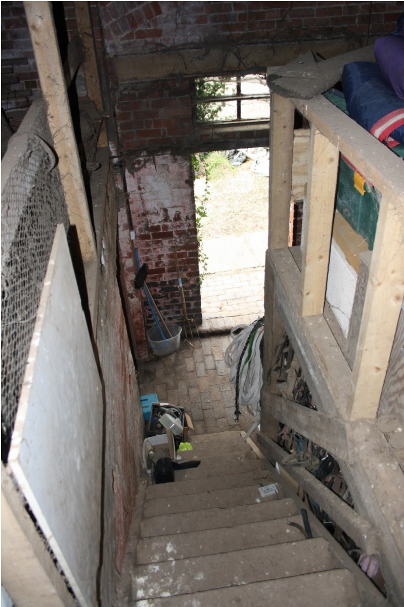
Plate 41: Landing/access area 10 stairs looking NW.
