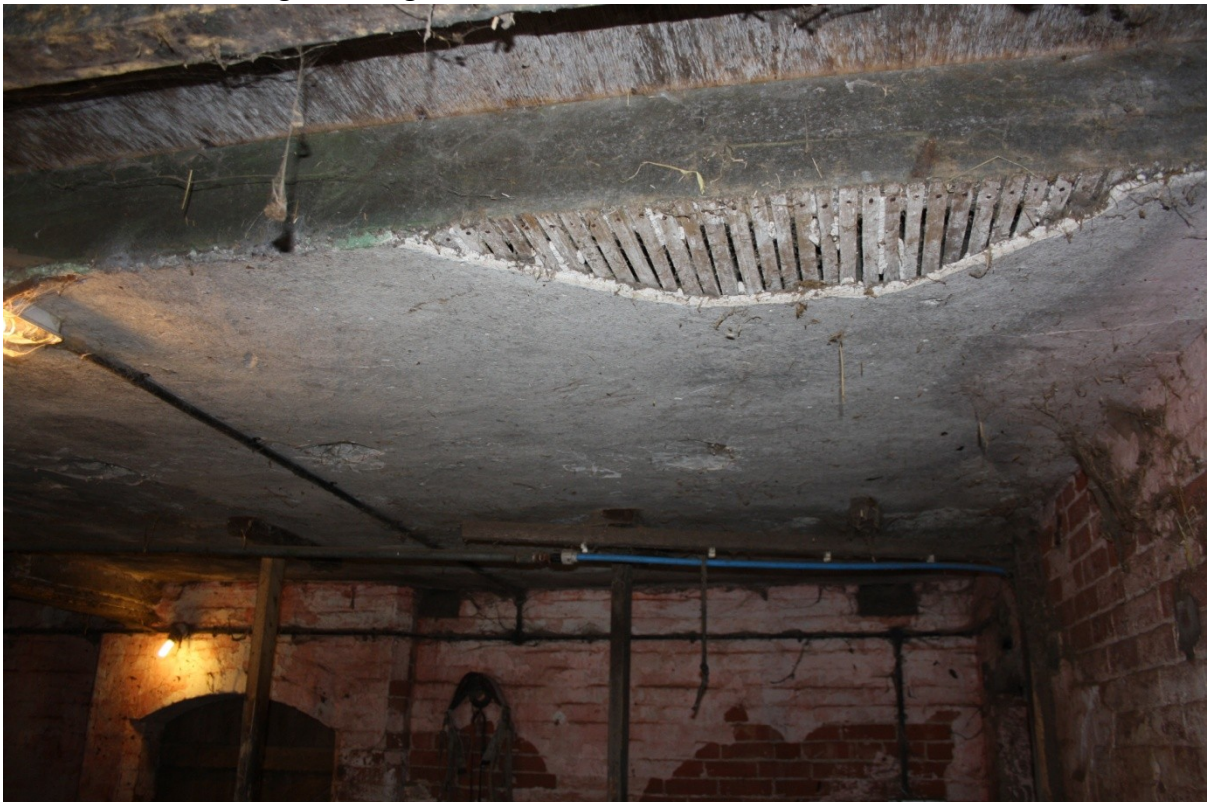
Plate 20: Cow Housing 3, plastered ceiling looking SE.
