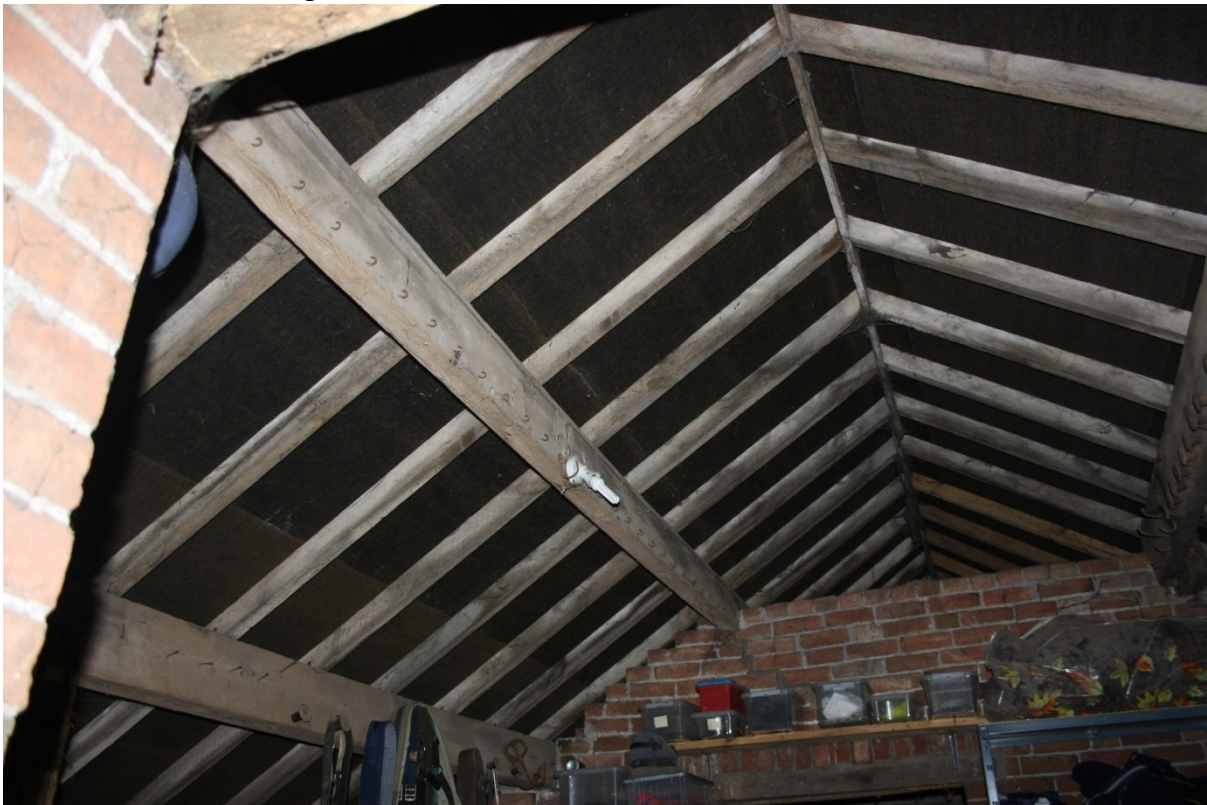
Plate 28: Storage Bay 5 looking N.
