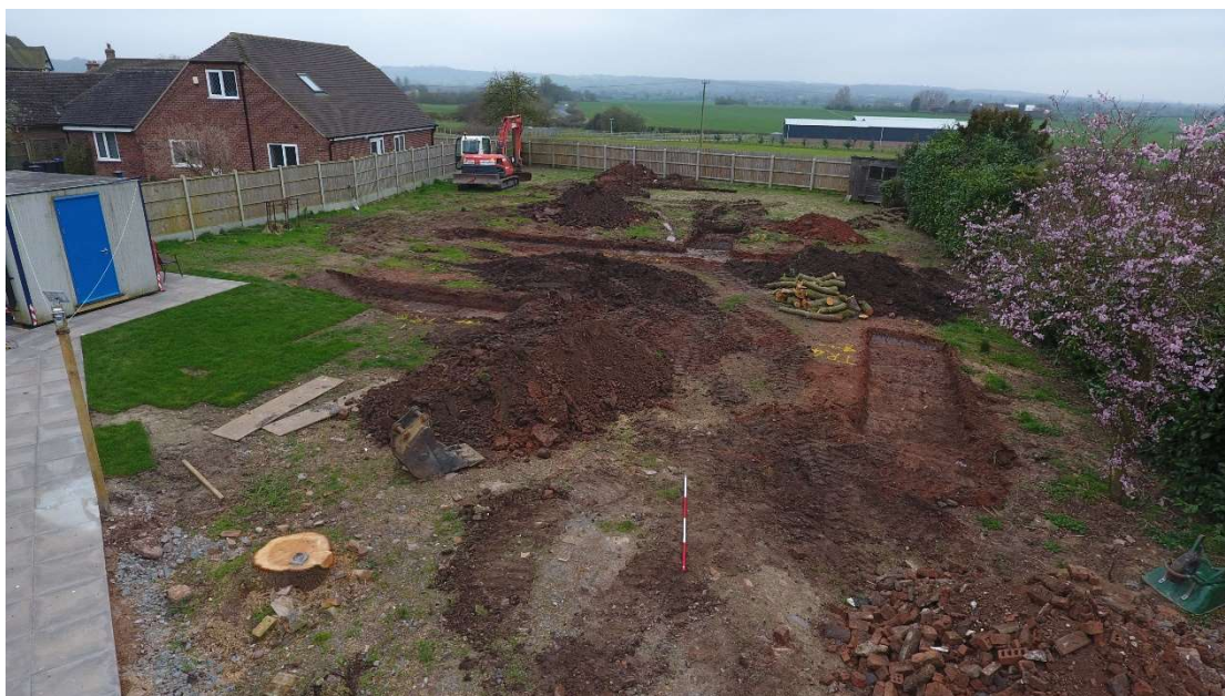
Plate 1: General view of the site, looking southwest.
