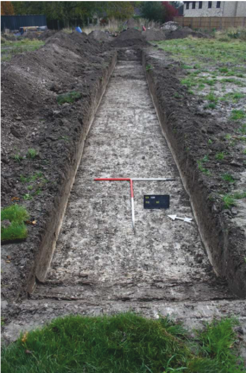
Plate 6: Trench Three looking east.
