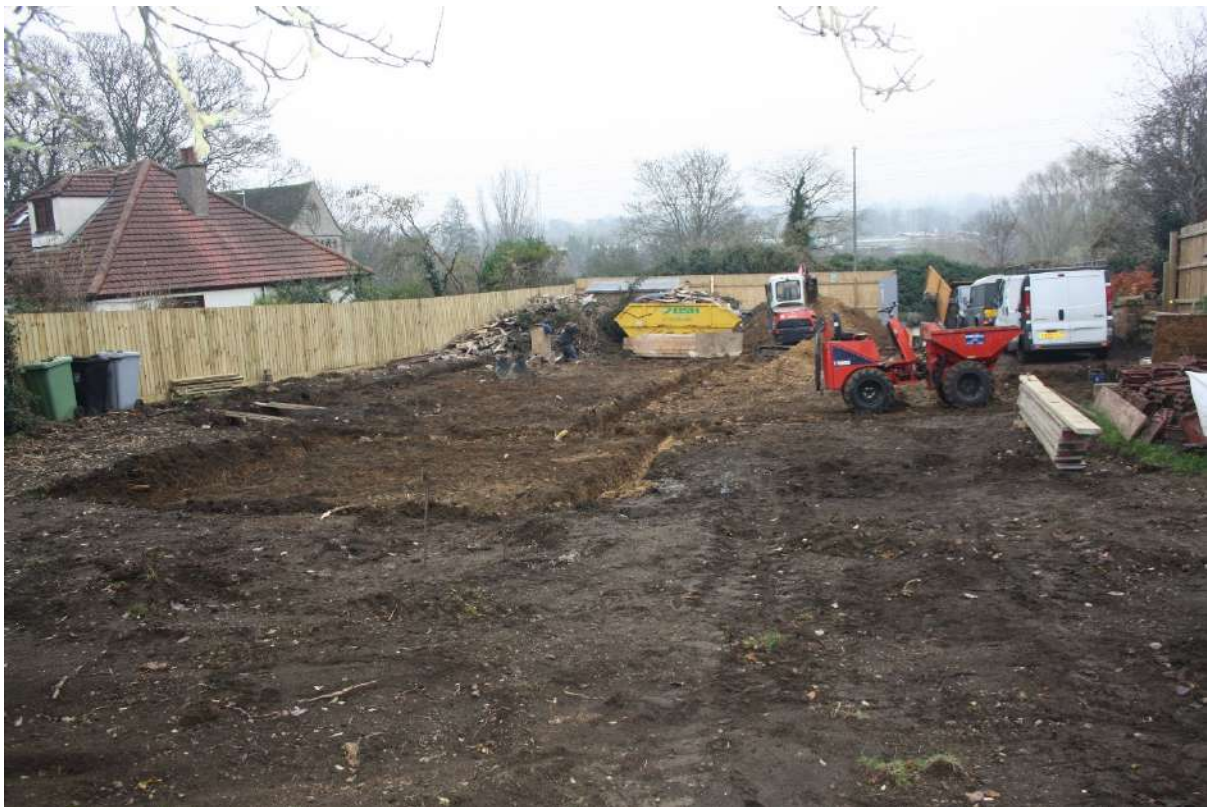
Plate 3: Site post-excavation looking south east.
