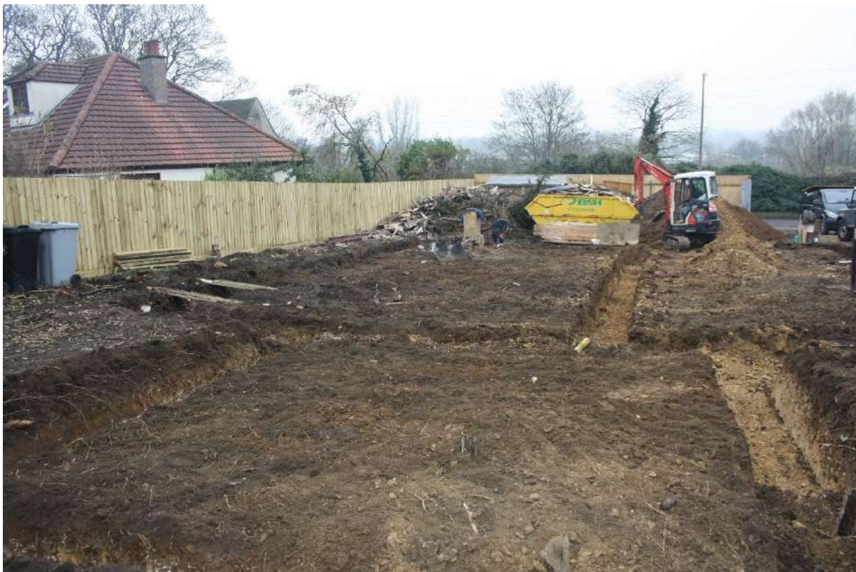
Plate 4: Working shot looking south east.
