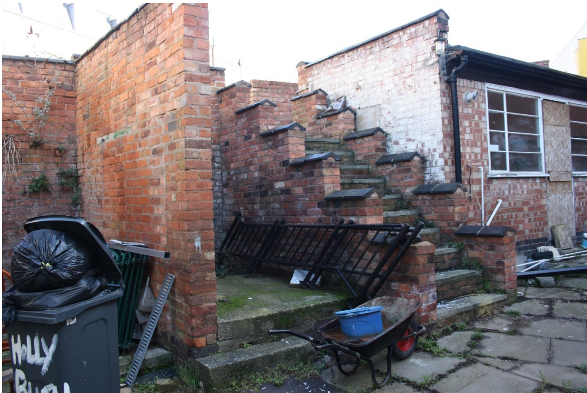
Plate 26: Looking east towards stair access to terraced area.
