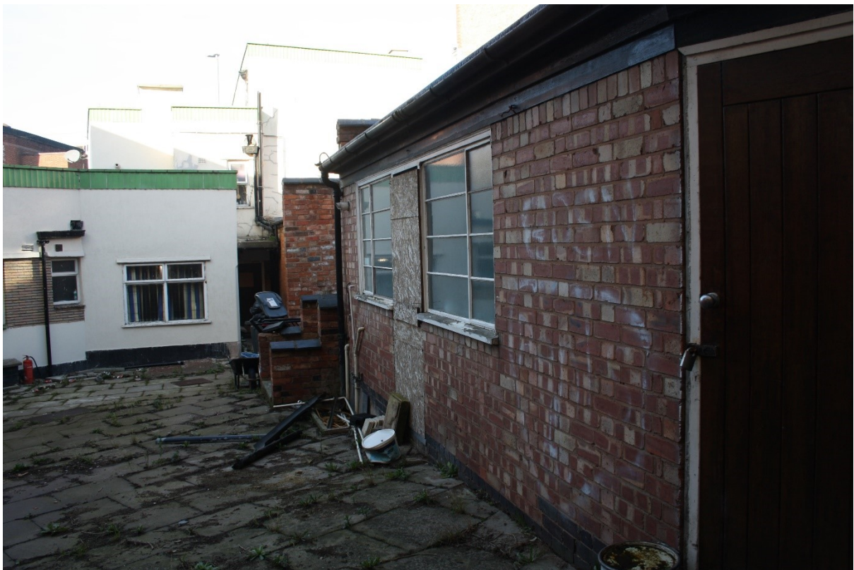
Plate 14: Outbuilding looking north west.
