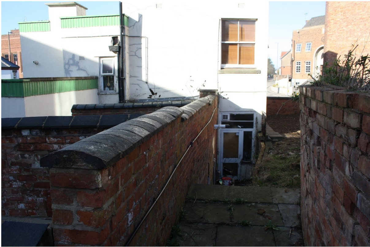
Plate 15: Looking north towards Holly Bush restaurant from terraced area.
