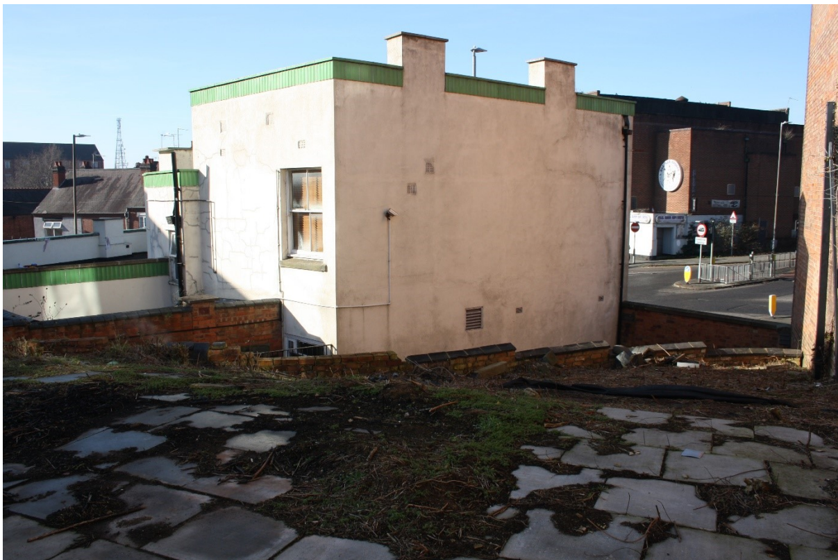
Plate 16: Holly Bush Restaurant looking north west from terrace area.
