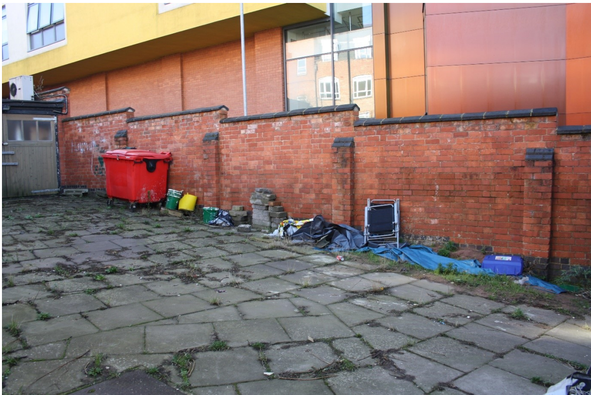
Plate 28: Looking south east towards boundary and adjacent college building.
