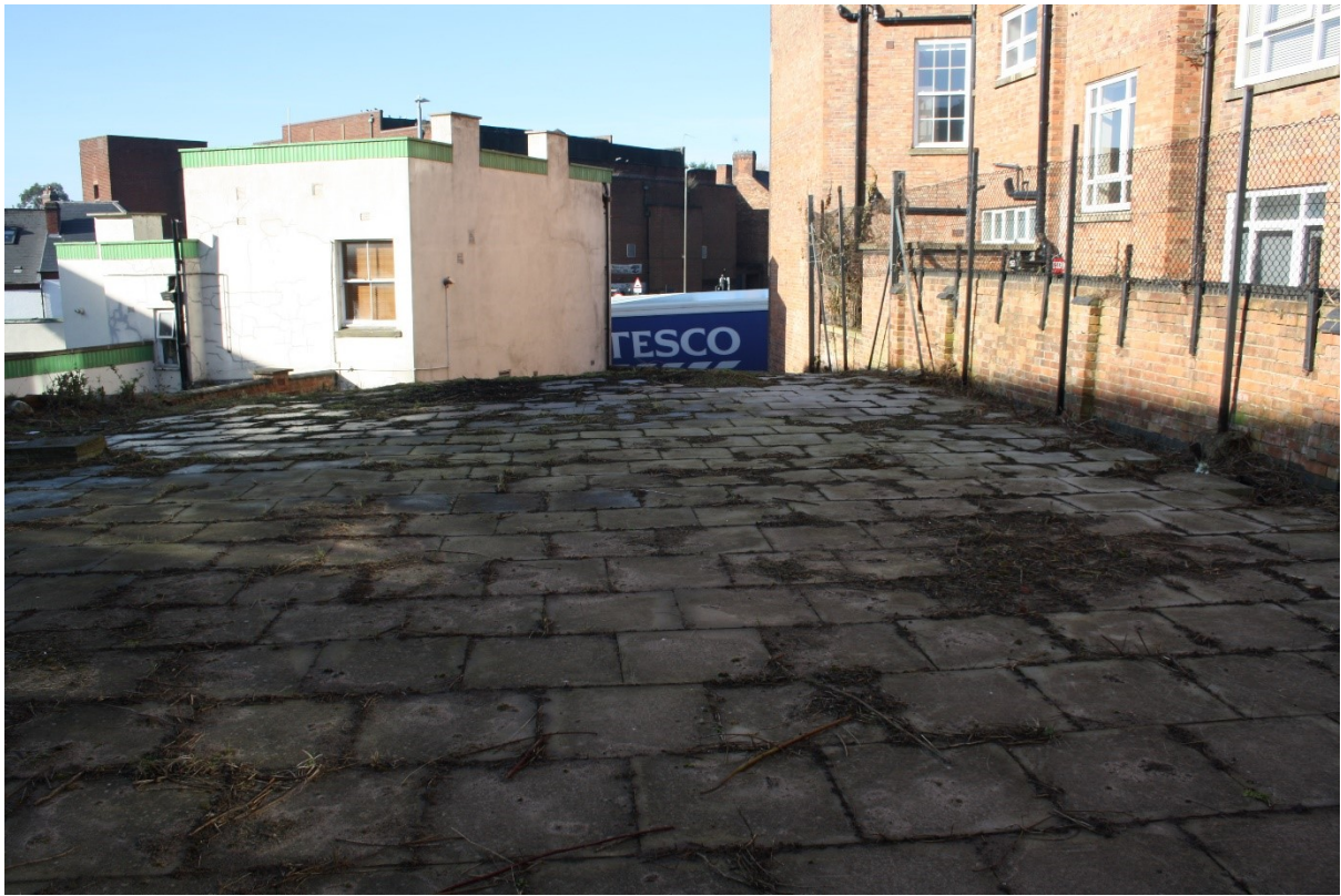
Plate 21: Terraced area looking north west.
