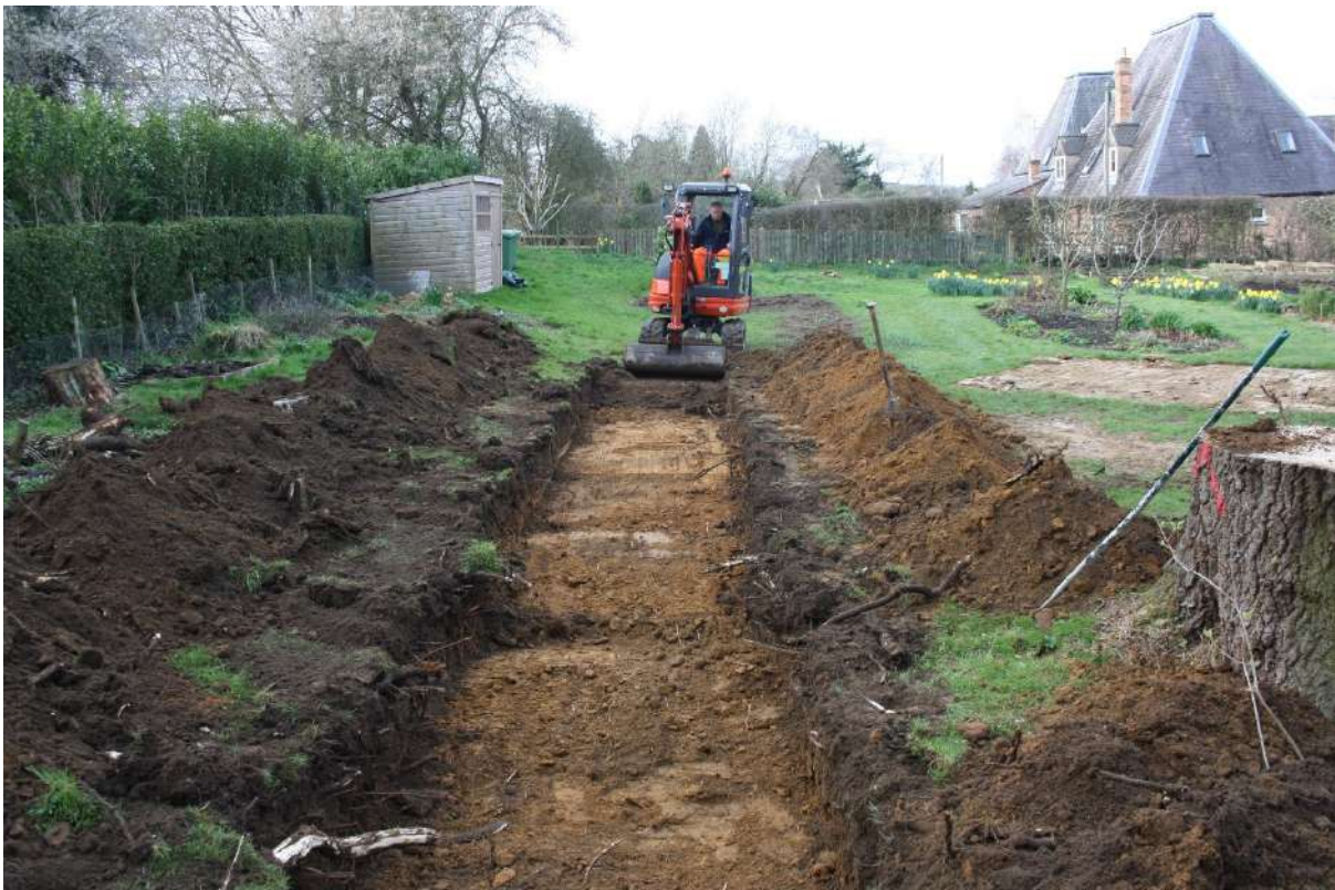
Plate 2: Working shot Trench 1 looking south west.
