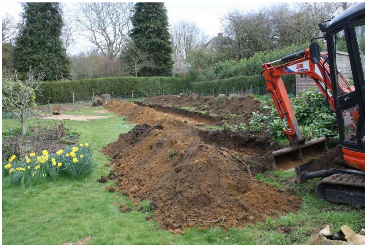
Plate 7: Overall site view of trenches looking east.
