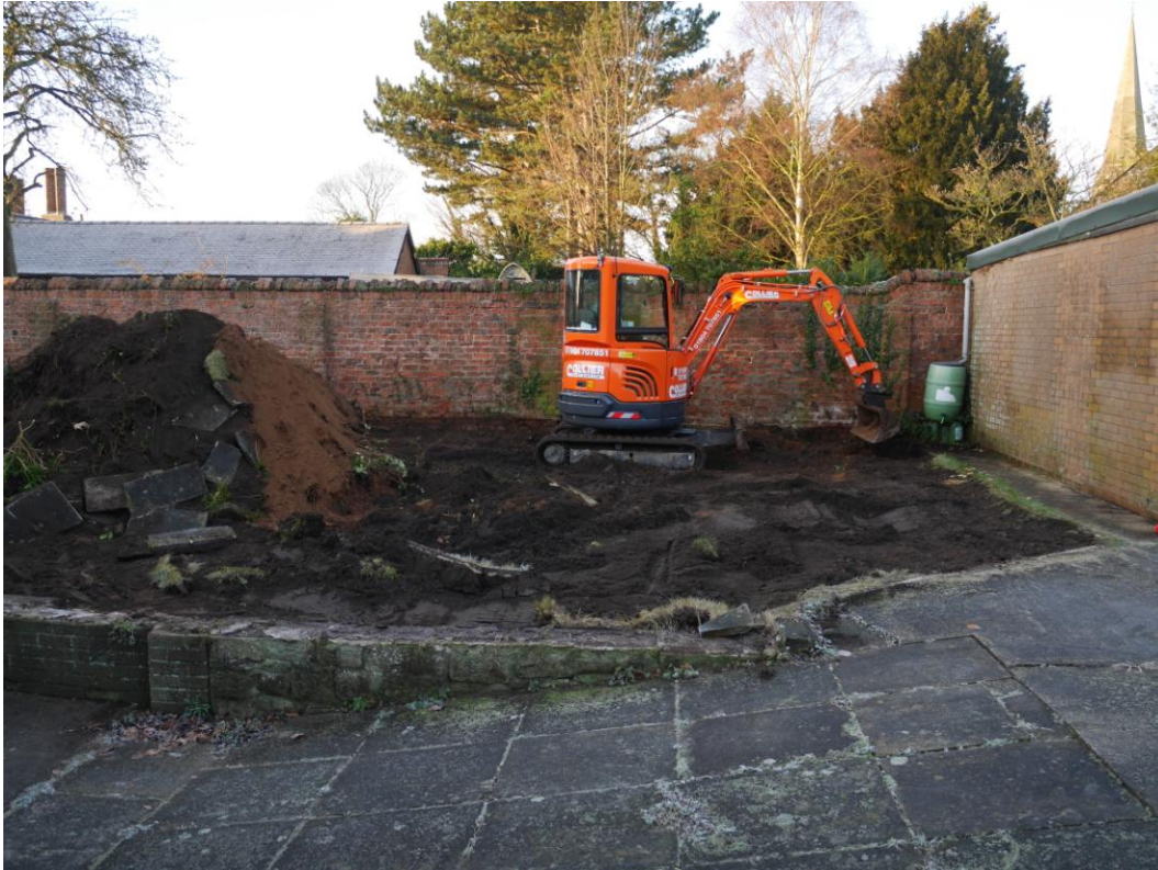
Photograph 1: The removal of the garden / top soil. Facing west
