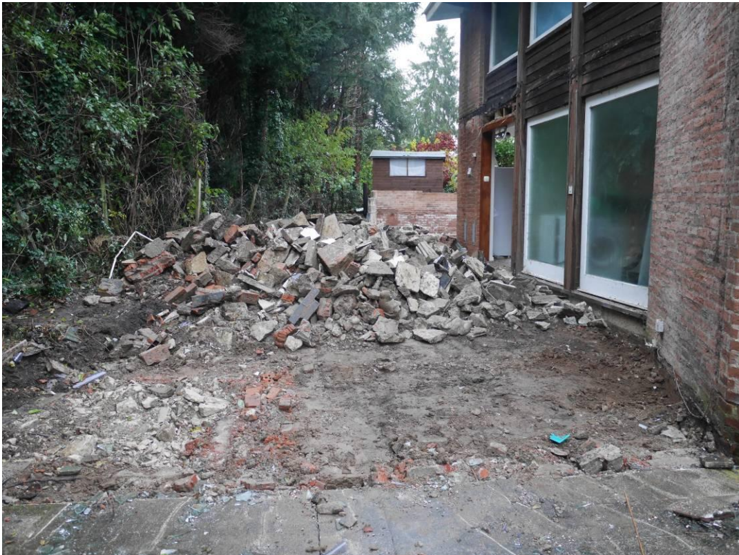
Photograph 1: Remains of the concrete ground floor. Facing northeast
