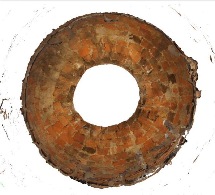
Plate 51: Domed well/cistern [85] internal details
