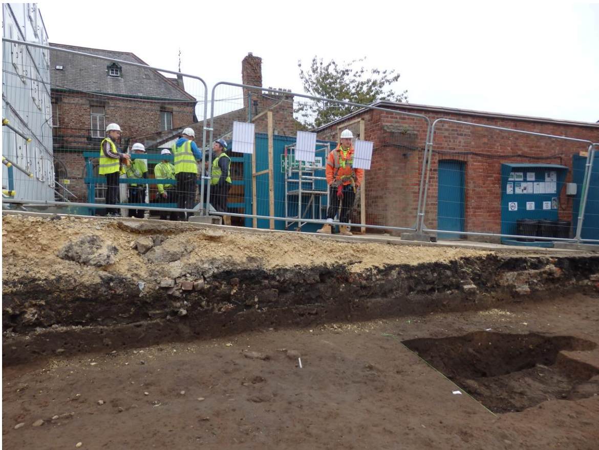
Plate 56: Information posters in use by construction team members
