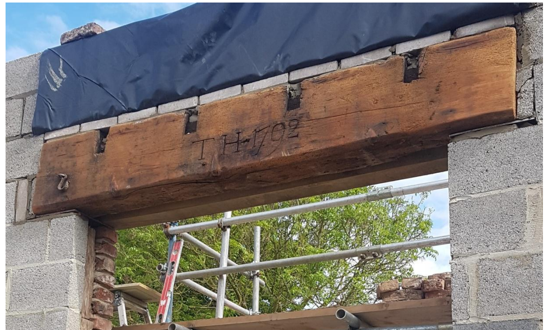
Figure 3: Original beam retained, by the owner, from the demolished 18th century outbuilding. Presently, repositioned as a window lintel, in the new build. Inscribed TH 1792- Thomas Hudson, Farmer residing at the plot during the late 18th to early 19th century.
