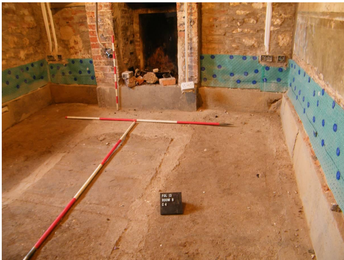
Figure 4: Room B, looking east, showing the under-floor concrete layer
