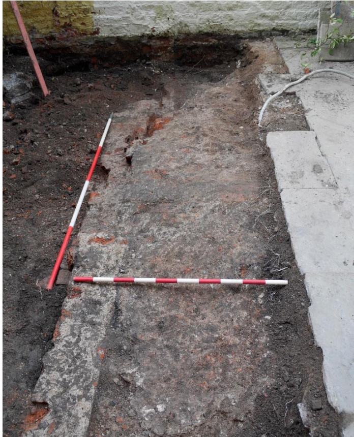
Figure 9: Wall (8) and cellar roof (9).
