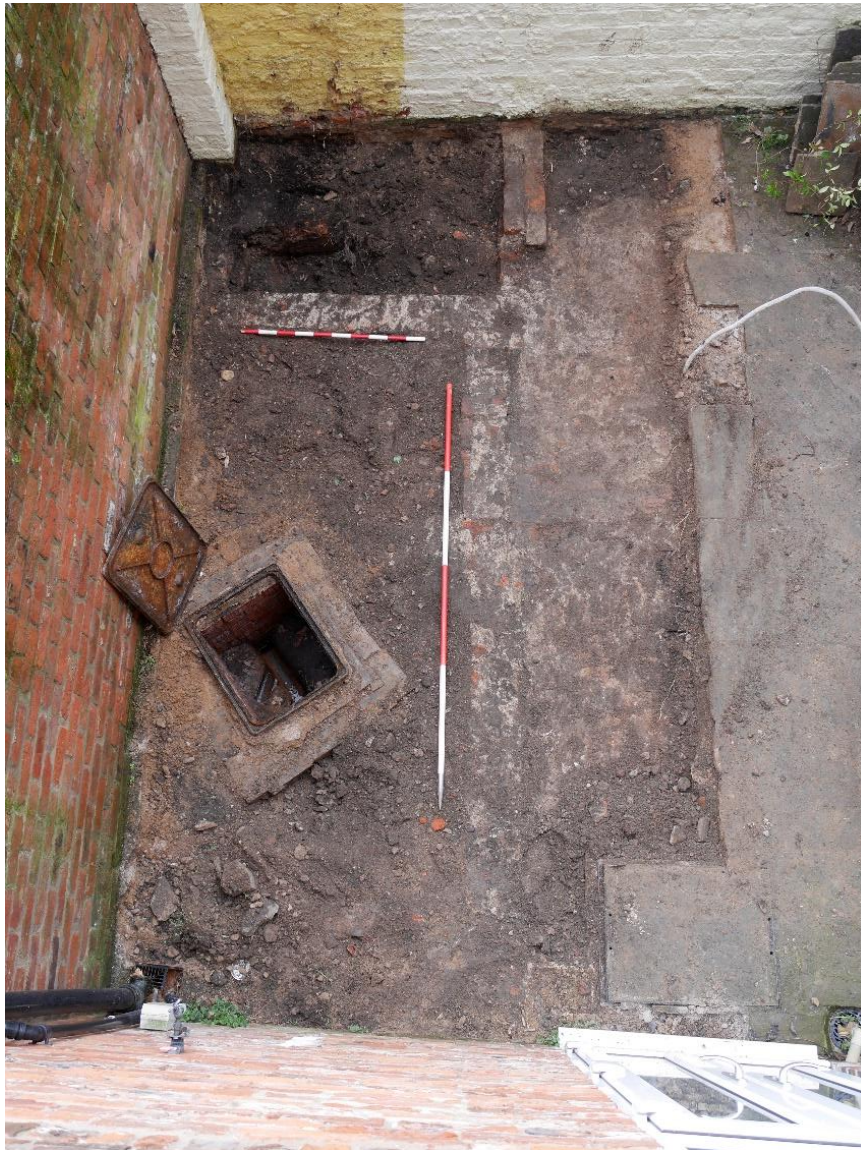
Figure 7: View of the site after the removal of the floor sandstone slab.
