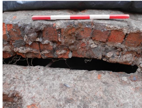
Figure 12: Exposed barrel vaulted cellar roof at garden height.
