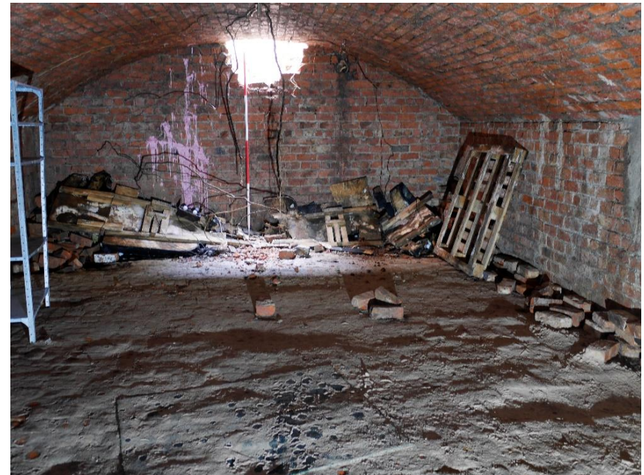
Figure 10: Internal view of the single nave barrel vaulted cellar.
