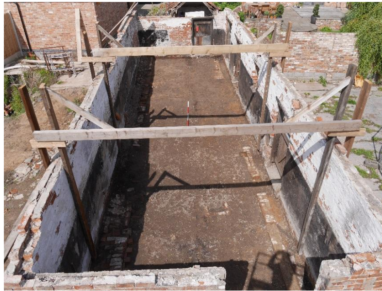
Figure 19: Internal view of Cow House looking north.
