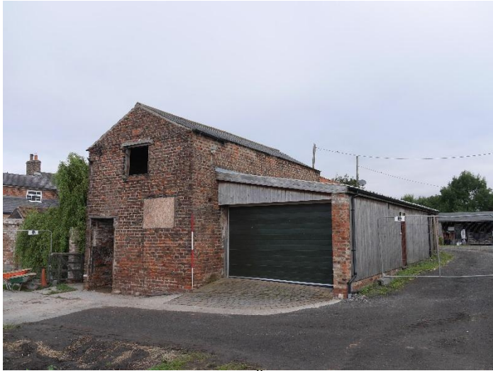
Figure 11: Combination Barn and 20 th Century Garage Addition.
