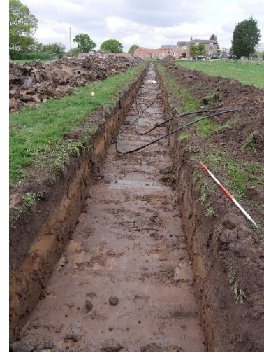
Figure 35: Trench 3 looking east.
