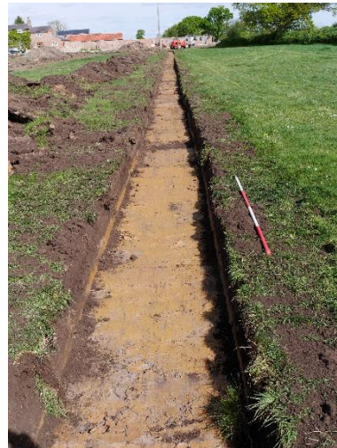
Figure 38: Trench 6 looking east.
