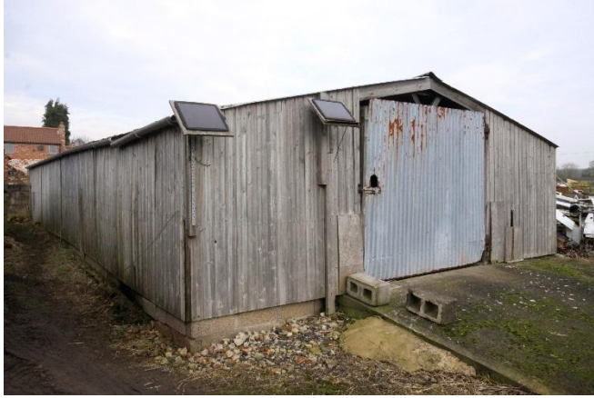
Figure 24: Storage Building 1 looking north-east.
