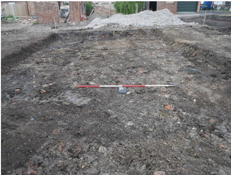
Figure 21: Post stripping in the Farmyard, Contexts (24) and (26).
