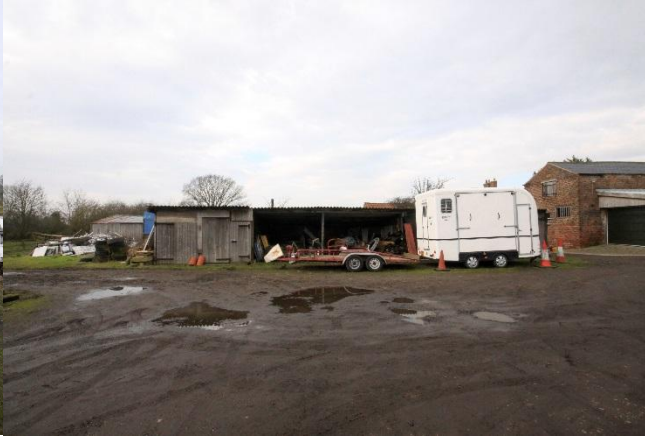
Figure 25: Storage Building 2 looking west.
