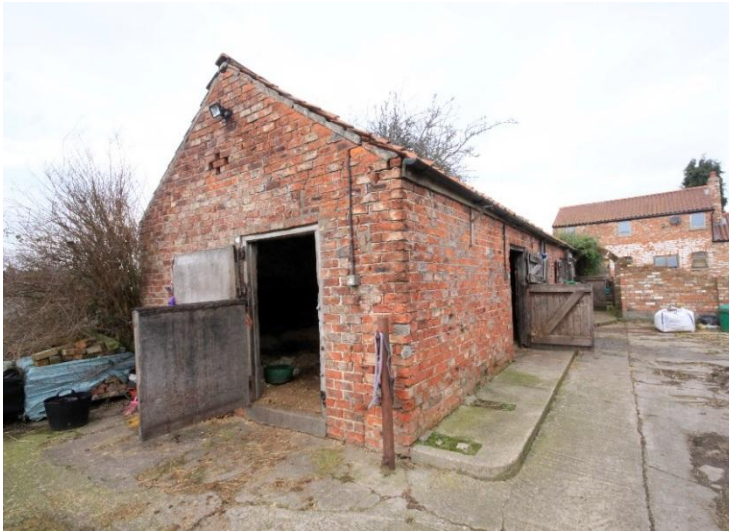
Figure 15: South and east facing elevations of the Cow House.
