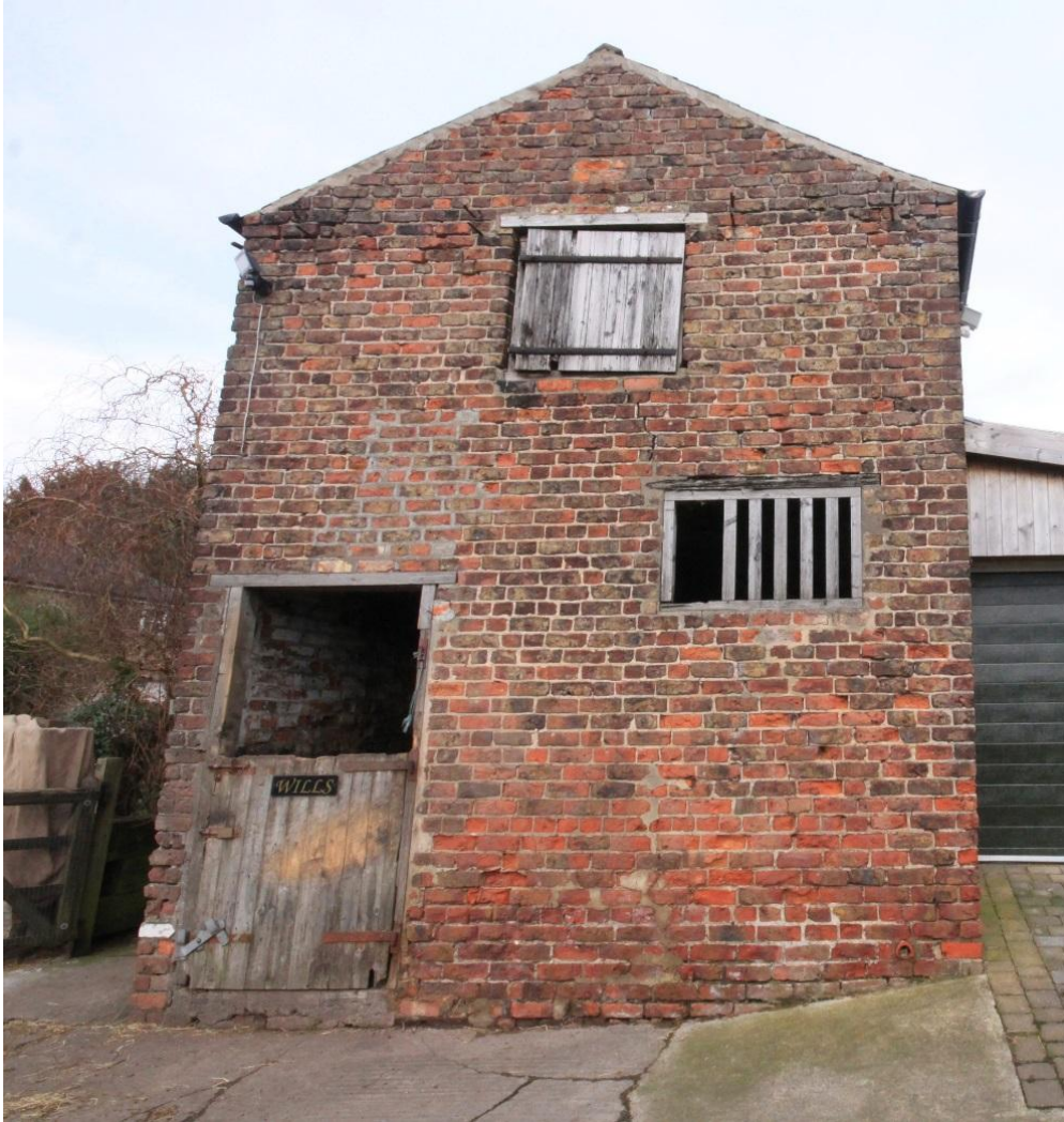
Figure 9: South Facing Elevation of the Combination Barn.
