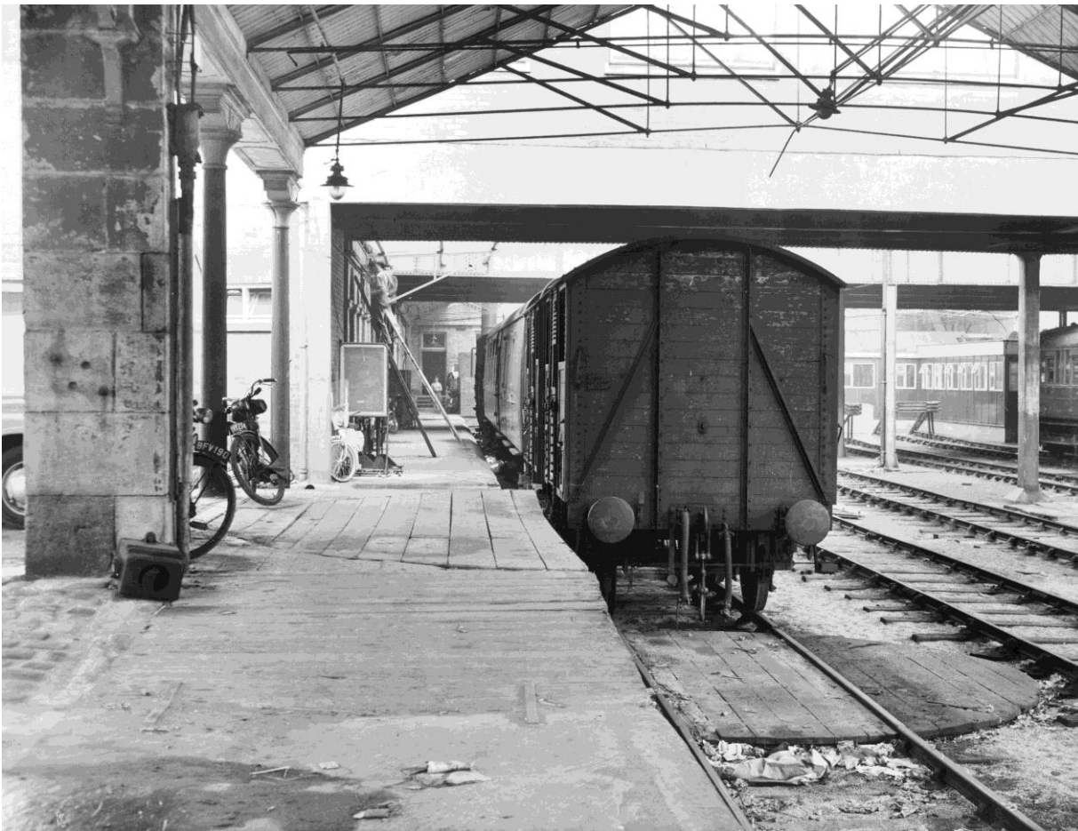
Figure 75: General View of wooden turntable and cutaway platform © Crown copyright. Historic England Archive
