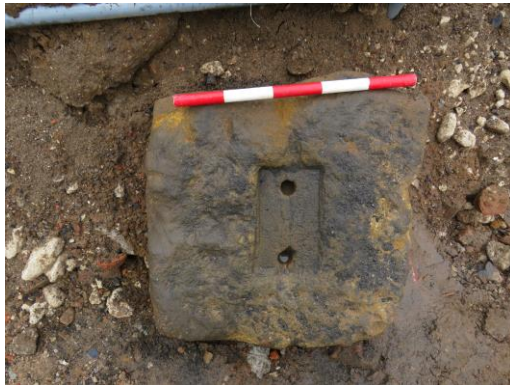
Figure 67: Railway sleeper block. The rail chair would be affixed with timber trenails
