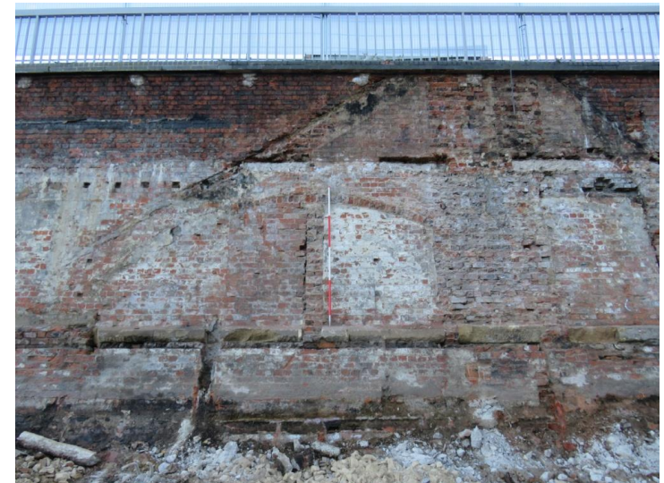
Figure 65: Wide span semi-circular brick arch (523) and flue scarring (505) and (506)
