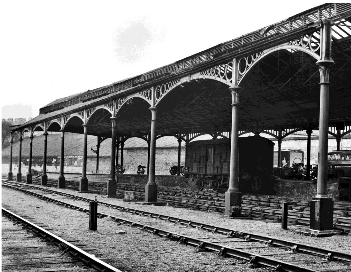
Figure 74:OP01486 General View showing arrival platform, roofing and ironwork © Crown copyright. Historic England Archive
