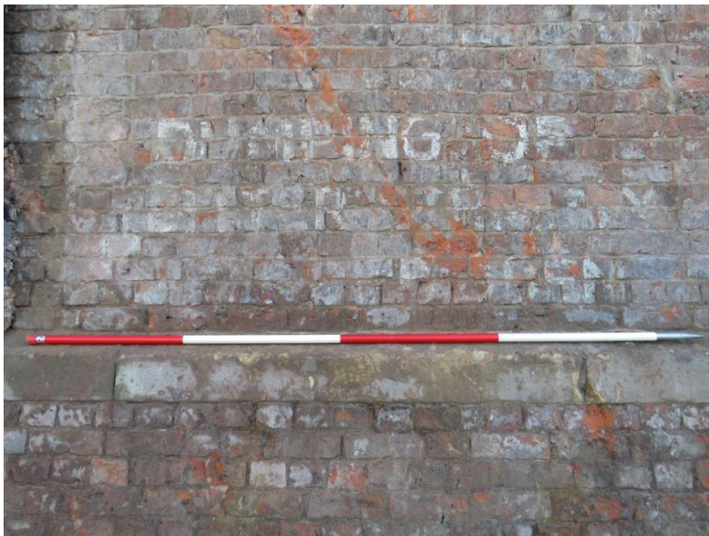
Figure 63: Wall base plinth (500) and beveled sandstone plinth with Phase 2 Ghost sign (498)
