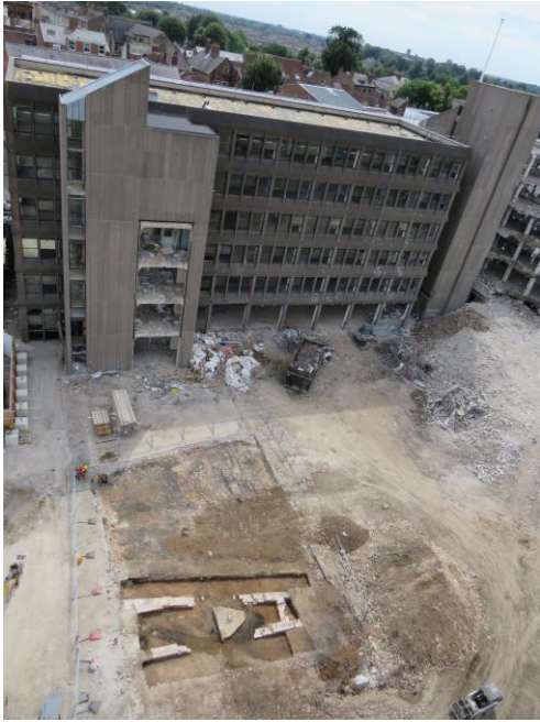
Figure 1: Hudson House demolition and the Old York Station Departure Platform
