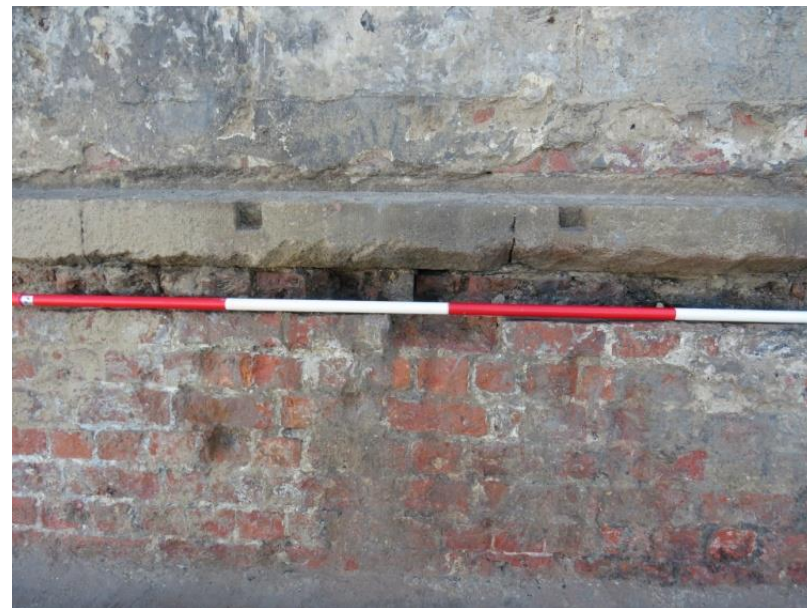
Figure 64: Wall base plinth (500) Phase 2 rectangular beam slots (501)
