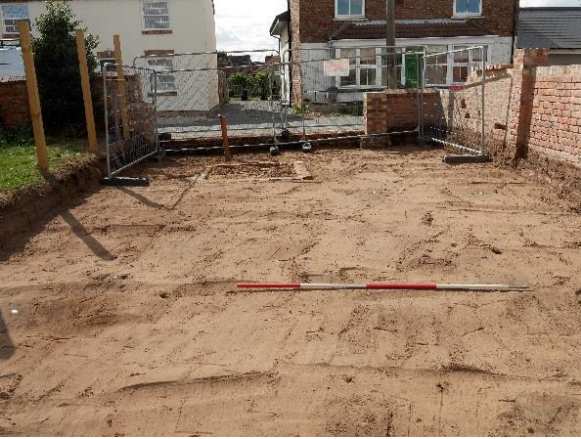
Photo 17: Access road post stripping facing west.
