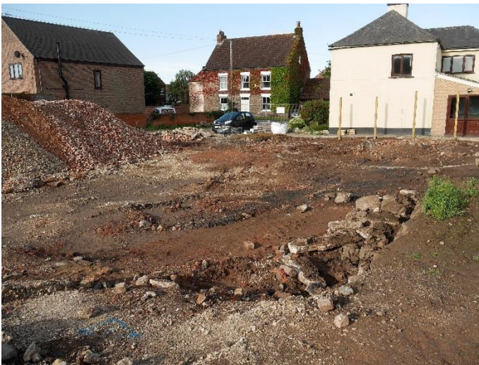
Photo 2: Gable end of farmhouse looking south.
