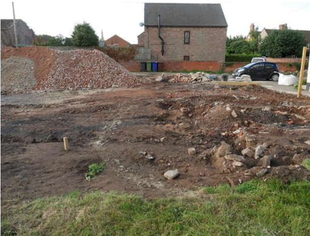
Photo 5: Post stripping of concrete surface, Context (3).
