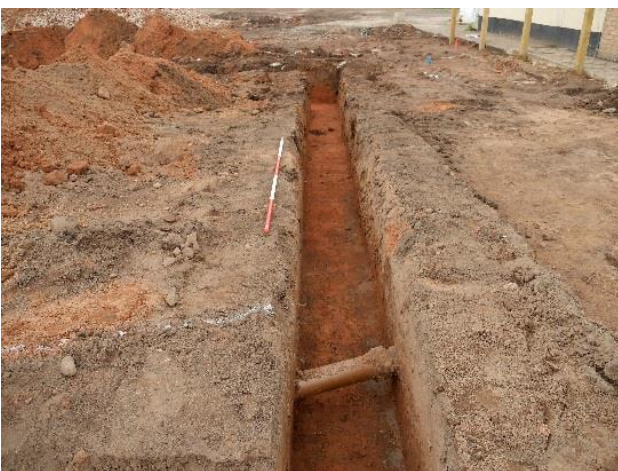
Photo 11: Foundation trenches for PlotV1.
