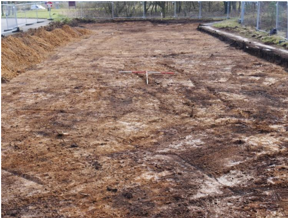
Figure 3: Car Park 1 post machine stripping
