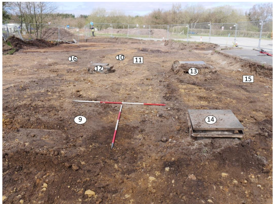
Figure 7: Car Park 2 features related to water and sewage systems
