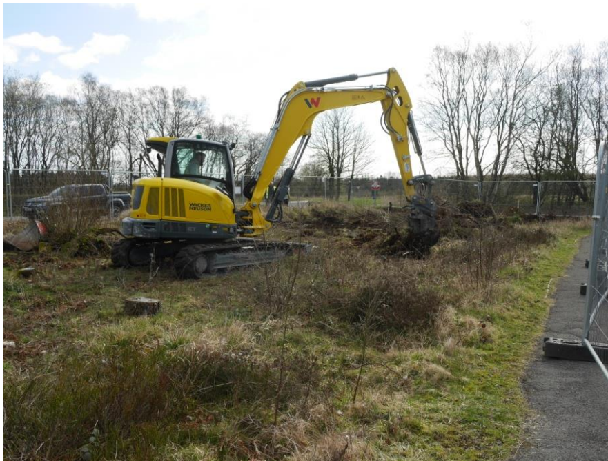
Figure 1: Groundwork's at Sutton Bank, Thirsk
