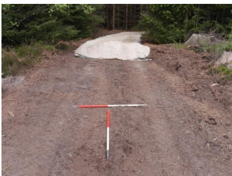
Photograph 3: Cycle Track facing east.
