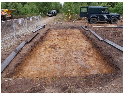
Photograph 21: Cycle Bridge trench facing west.
