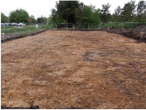
Photograph 29: Car Park area stripped facing south-west.
