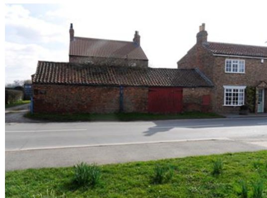
Image 6: Outbuildings constructed abutting Anvil Cottage.
