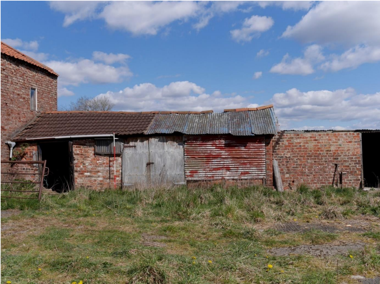
Image 27: Northwest facing elevation of the Multi Bay Shelter Shed.
