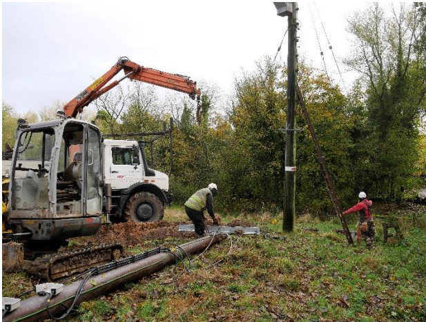
Figure 3: Groundworks involved the removal of an electricity pole.
