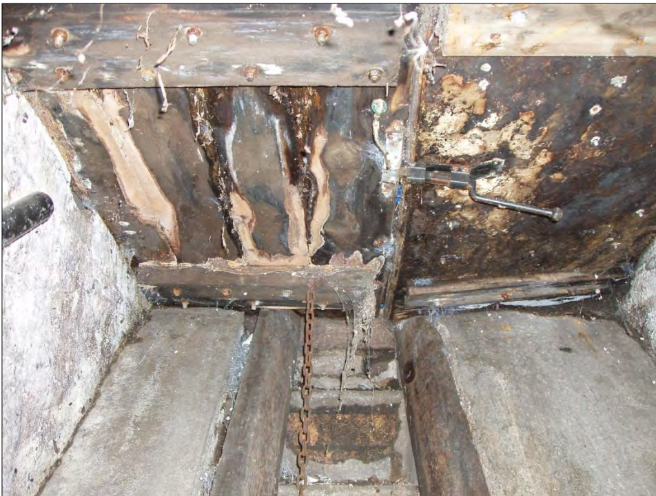
Photograph 5 Detail of Wooden Hatch at Top of Barrel Shute
