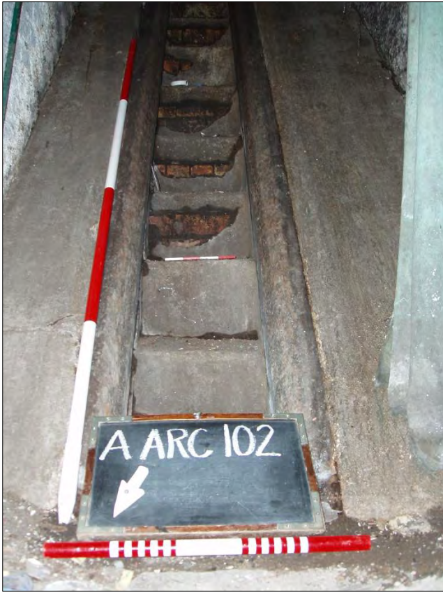
Photograph 5 Detail of Wooden Hatch at Top of Barrel Shute
