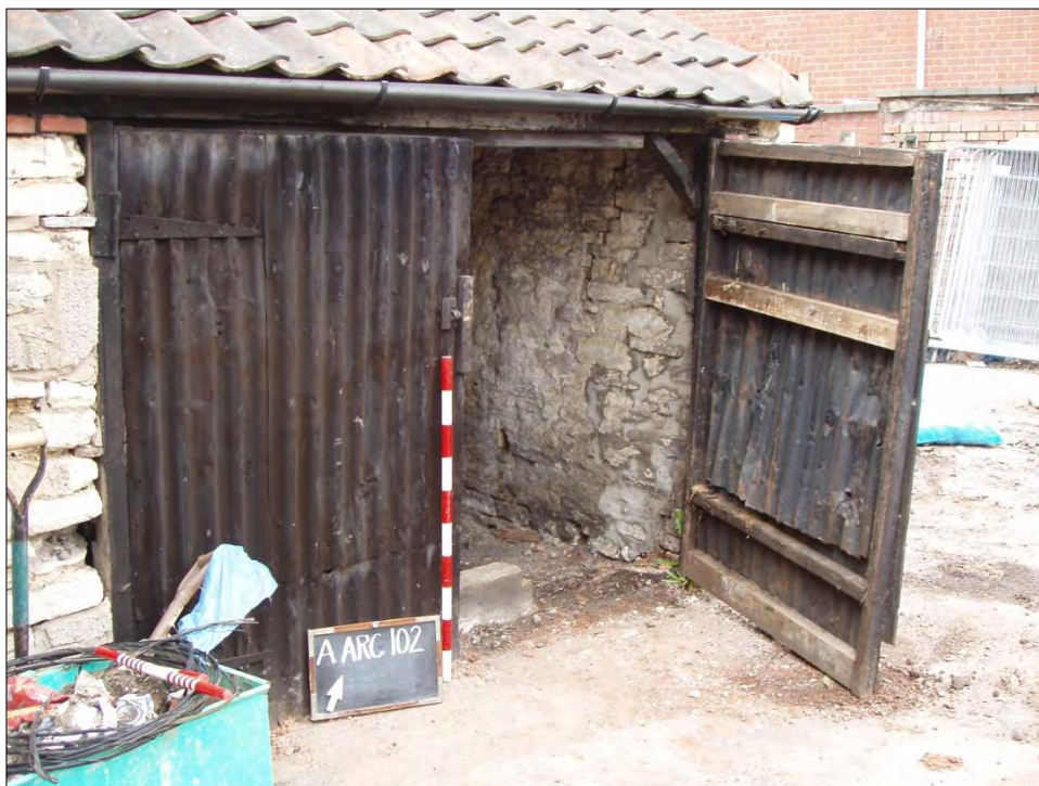
Photograph 45 NNW Facing View of Corrugated Iron Doors (Scale 1 x 1m)
