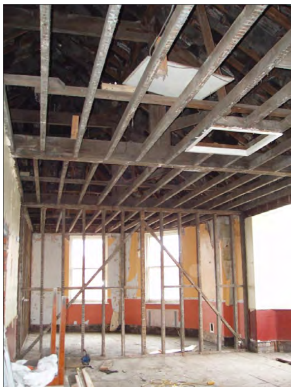
Photograph 28 Detail of Wooden Joists SE Facing View
