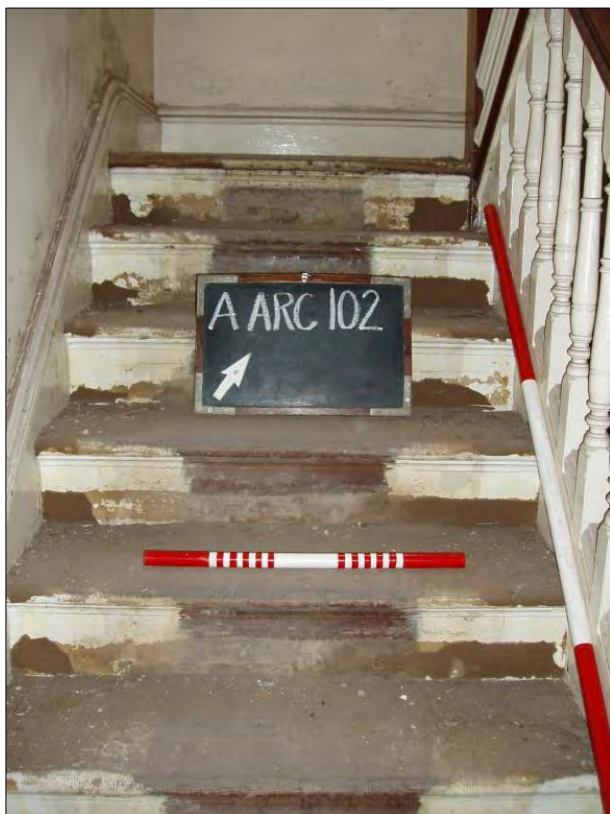
Photograph 30 Half Landing Stair with Square Base Baluster From Ground to First Floor (Scales 1 x 2m & 1 x 500mm)
