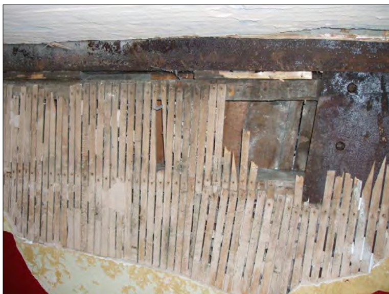
Ground Floor Room 2
