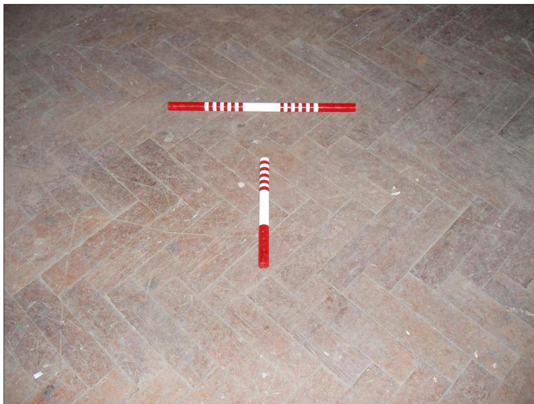
Photograph 21 Detail of Herringbone Parquet Flooring (Scales 1 x 500mm & 1 x 300mm)
