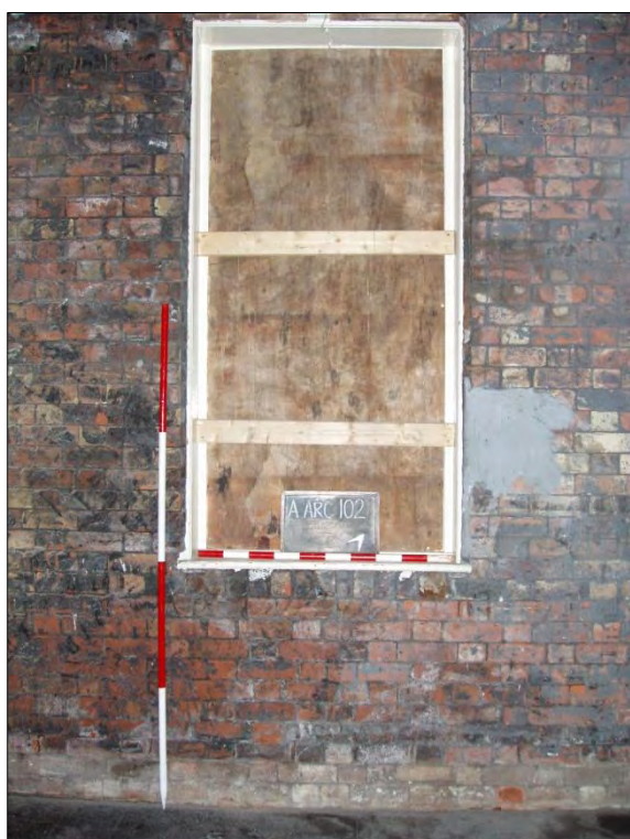
Photograph 10 Detail of Wooden Window Frame (Scales 1 x 2m & 1 x 1m)
