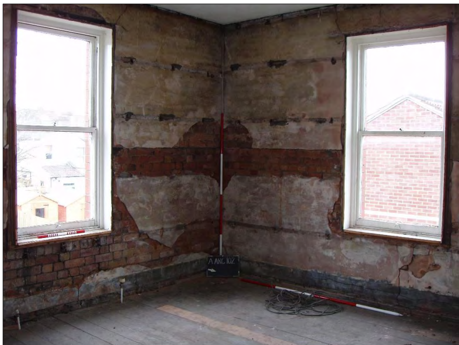
Photograph 33 WSW Facing View (Scales 2 x 2m)
