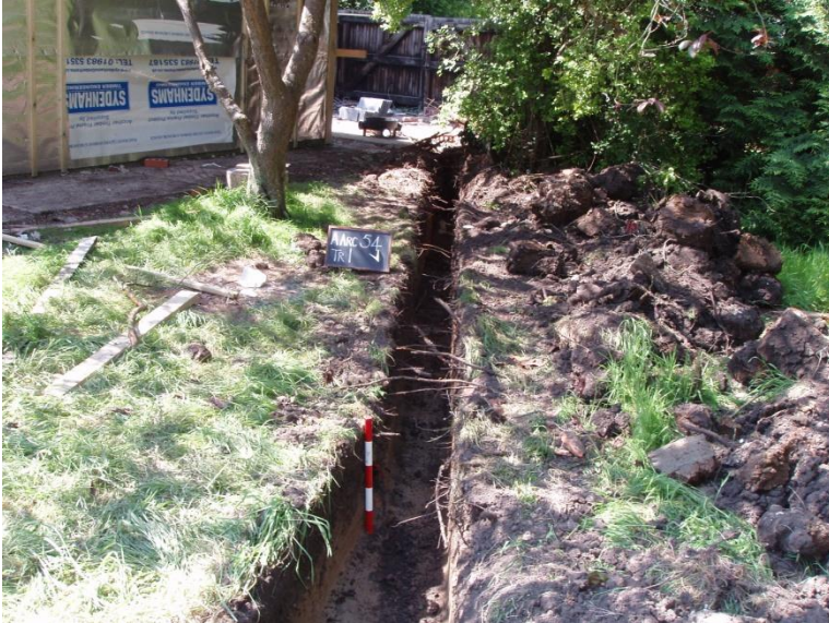
Photograph 11: NE Facing View of Service Trench (Scale 1 x 1m)
