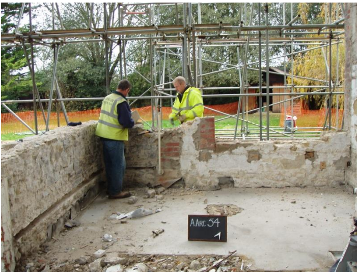
Photograph 5: Demolition of Lower Courses by Hand
