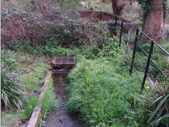
Photograph 8 Water Tank c. 5m from Project Site NW Boundary
