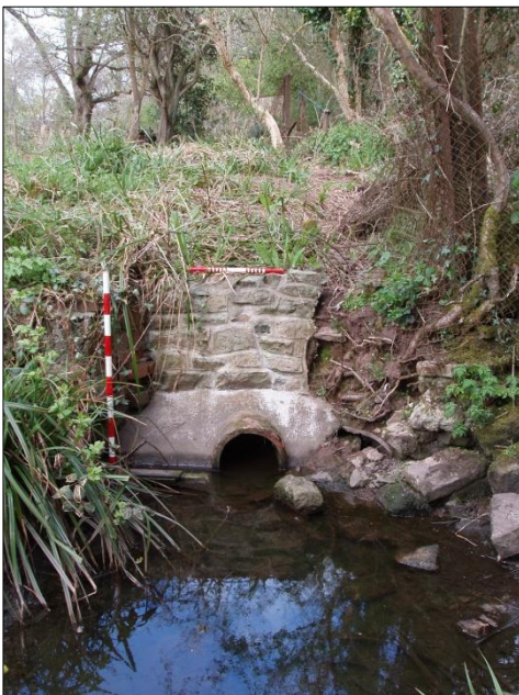
Photograph 9 Possible Outlet to Overflow Detailed in Photos 6 & 7 (Scales 1 x 1m & 1 x 500mm)
