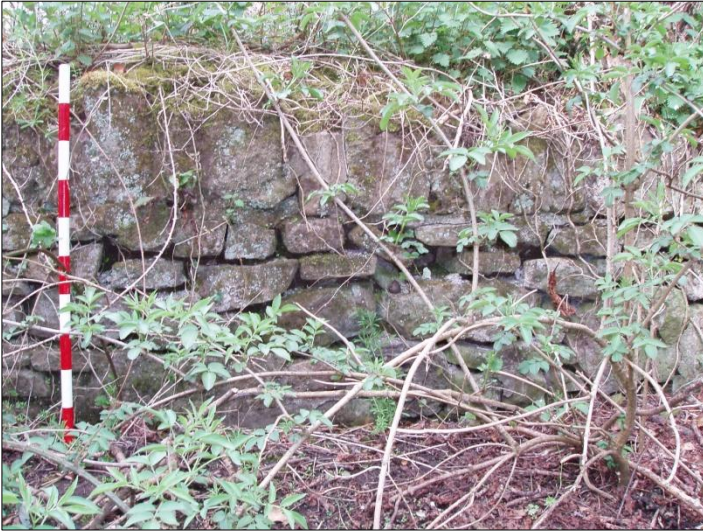
Photograph 11 NNE Facing View of Single Skin Stone Walling, Facing Earthen Bank Opposite Above (Scale 1 x 1m)
