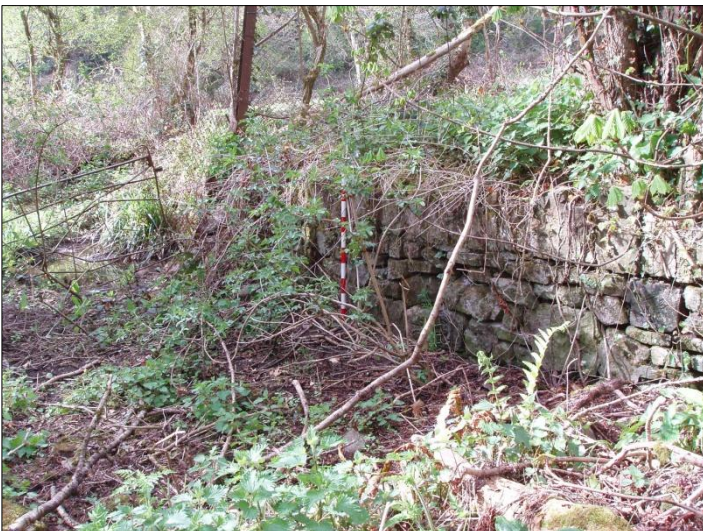
Photograph 11 NNE Facing View of Single Skin Stone Walling, Facing Earthen Bank Opposite Above (Scale 1 x 1m)
