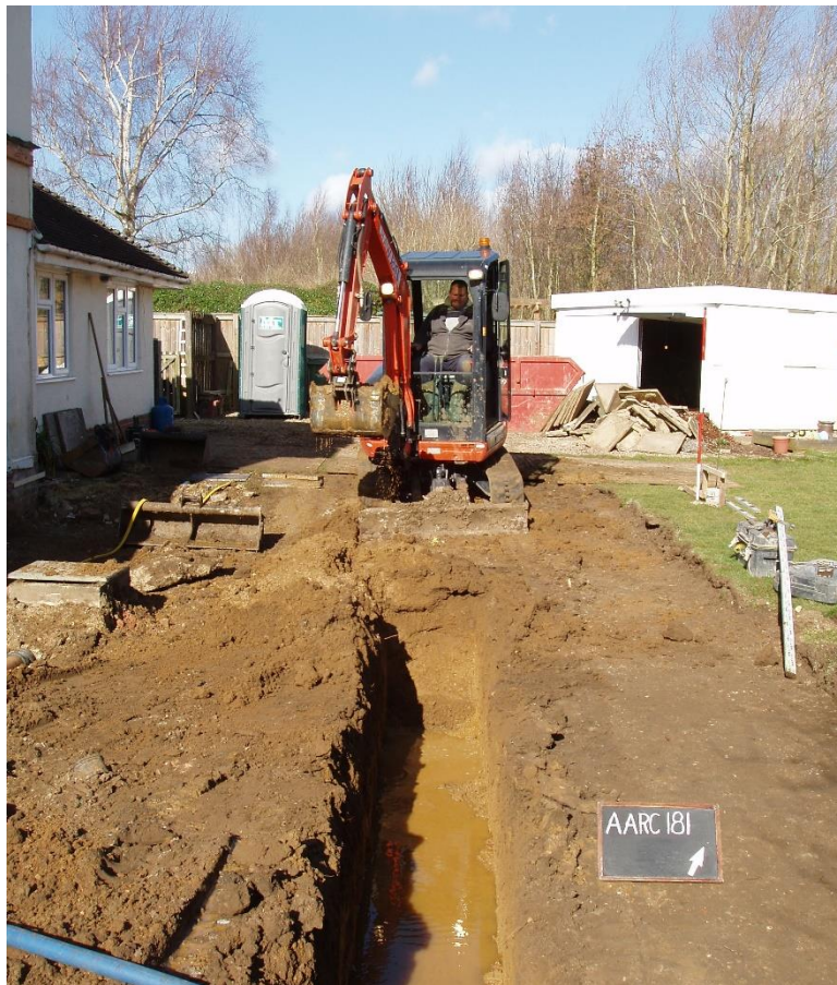
Photo 2 NNW facing view of foundation trench under excavation
