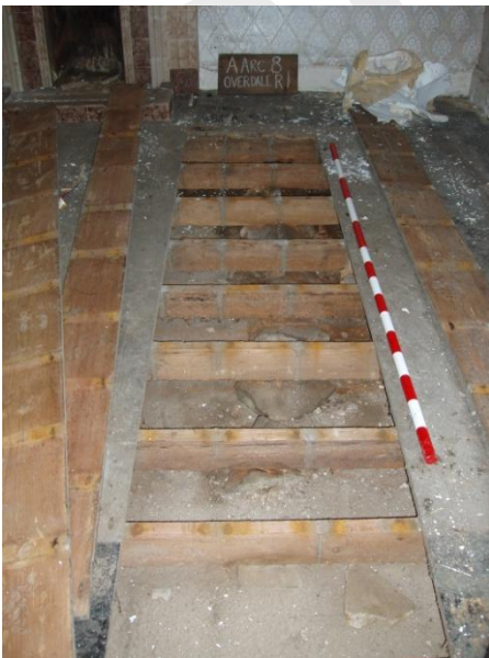
Plate 12. Floor boards and joists, Room 1. (2m Scale)
