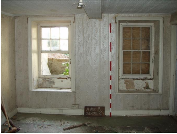
Plate 7. Recessed sash window with deep sill/seat, Room 3 (2m Scale)
