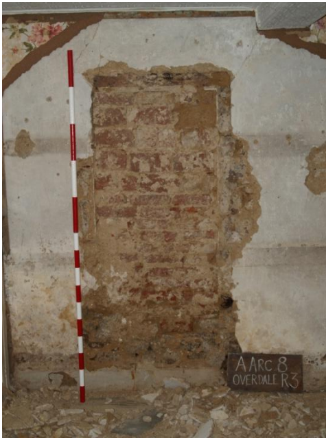
Plate 8. Bricked up window, rear wall of Room 3 (2m Scale)
