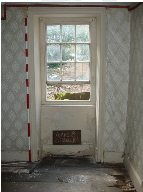
Plate 6. Recessed sash window, Room 1. (2m Scale).
