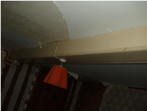
Plate 11. Central Beam. Room 1.
