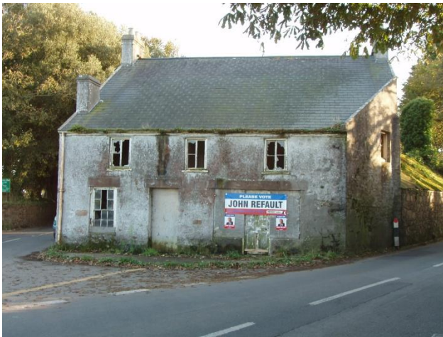
Plate 1. North facing facade, Overdale, Le Carrefour a Cendre.
