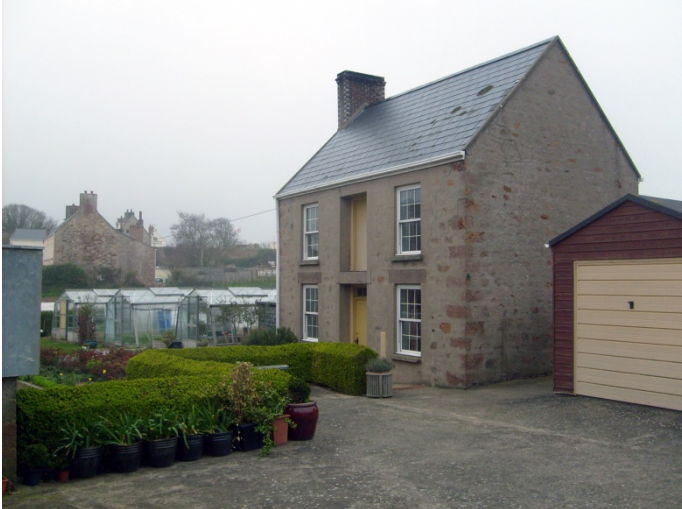
Fig 6: SSE facing cottage, with ENE facing gable end
