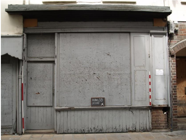
Photo 3 Facade 14 Hilgrove Street (Scales 1 x 2m & 1 x 1m)
