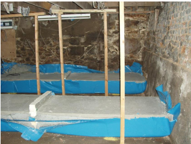
Photo 4 Cellar View with Concrete Rafts 14 Hilgrove Street
