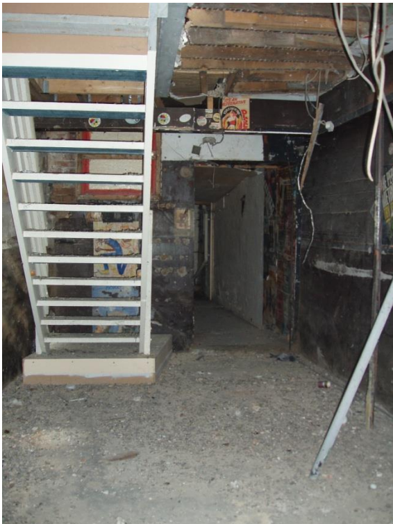
Photo 2 Interior View North Facing 12 Hilgrove Street
