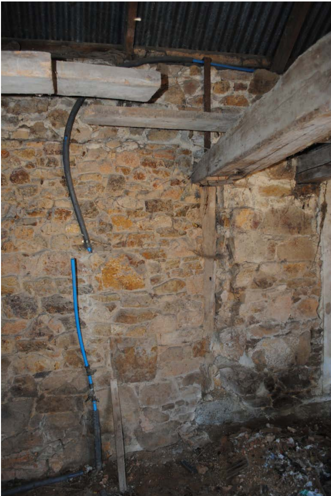
Photo 14: View of internal northern wall of outbuilding showing extant post and joist also visible from La Rue du Ponterrin
