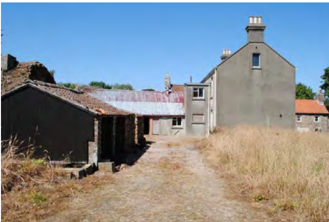
Photo 4: Ruined Building showing fireplace and small entrance from east
