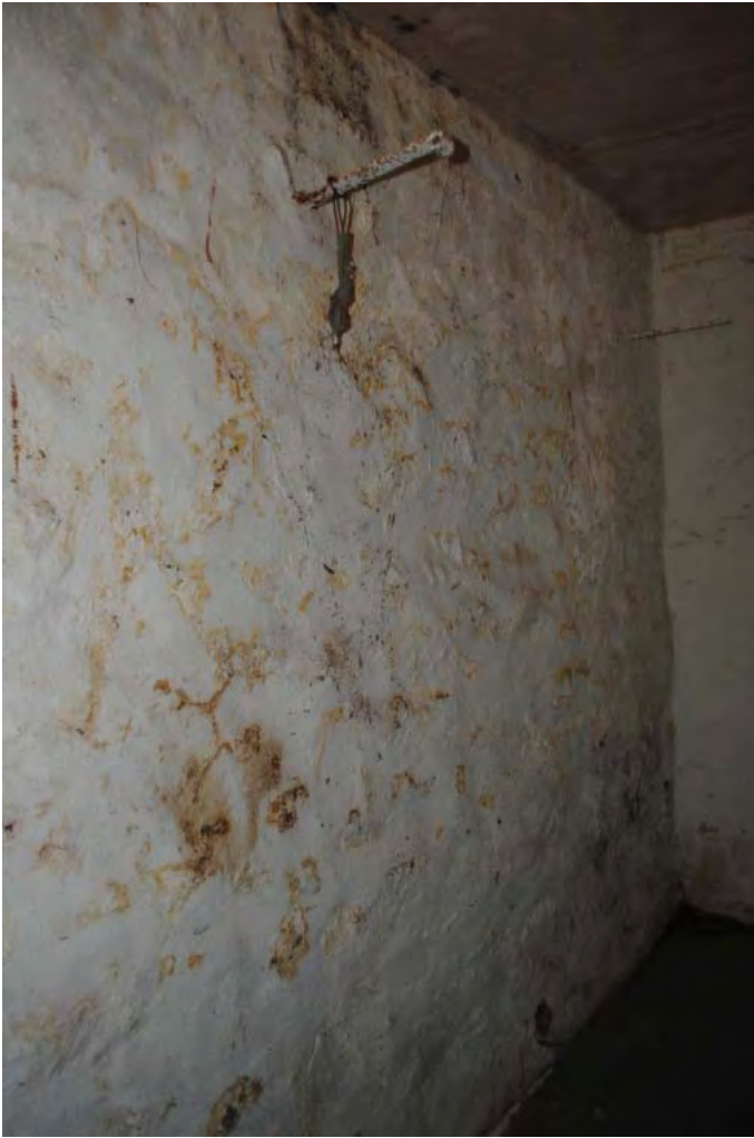
Photo 8: Outbuilding to the rear (west) of Ruined Structure, now painted
