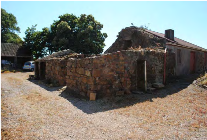
Photo 6: Ruined building from N
